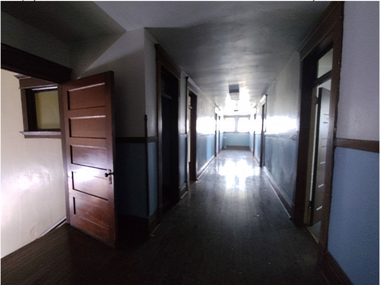
Photograph 46. View: third floor hallway interior, facing northeast WV_RandolphCo_OddFellowsHome_0046
