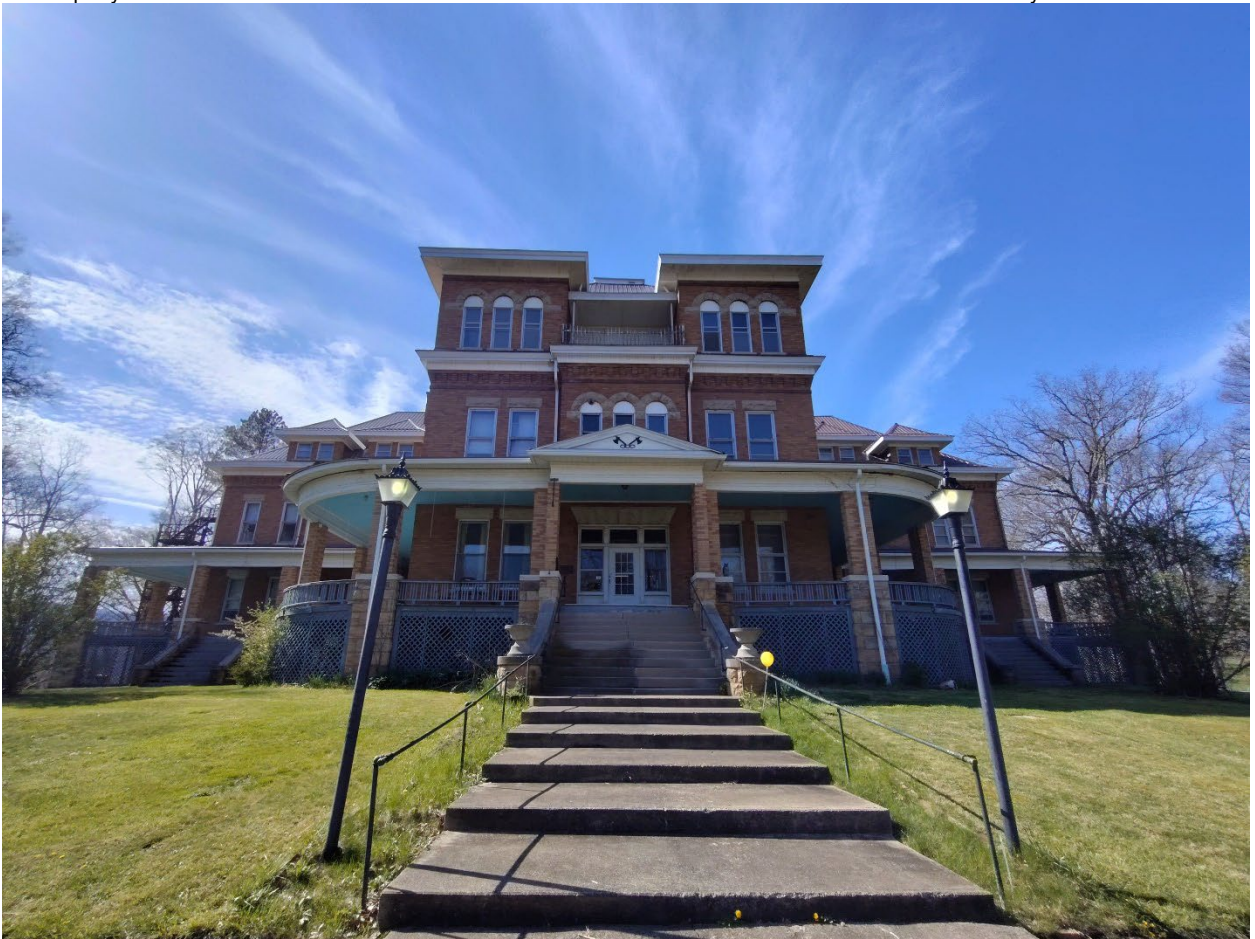
Photograph 2. View: front façade/southeast elevation, facing northwest WV_RandolphCo_OddFellowsHome_0002
