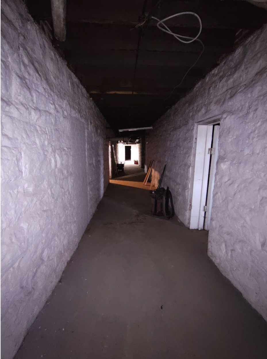
Photograph 57. View: basement hallway interior, facing northeast WV_RandolphCo_OddFellowsHome_0057
