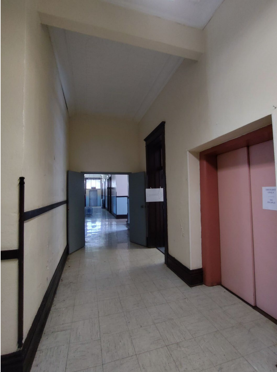
Photograph 22. View: first floor hallway interior, facing southwest WV_RandolphCo_OddFellowsHome_0022
