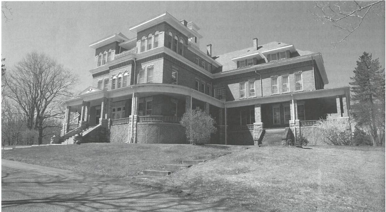
Figure 16: Historic photo, front façade with modified columns and roof, 2003.
