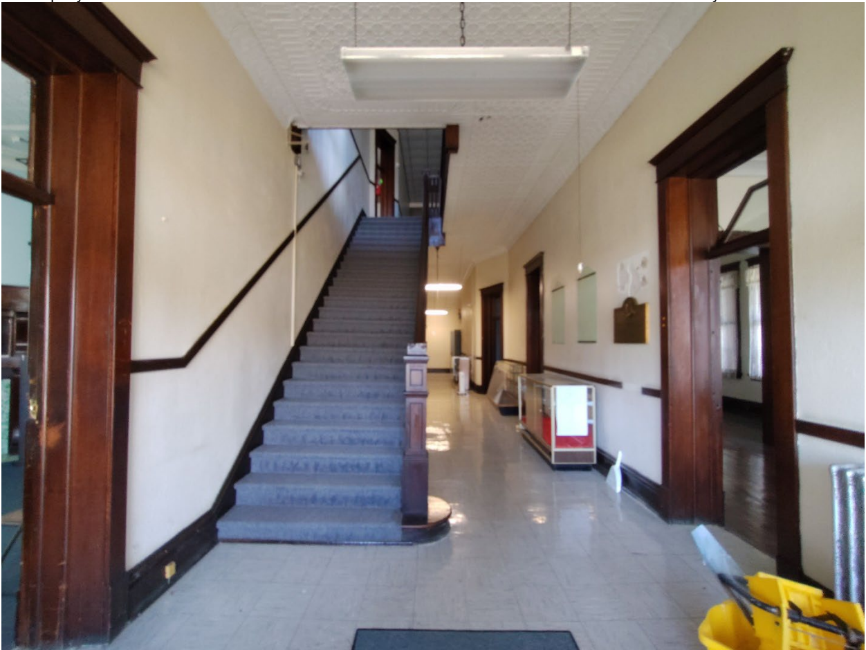
Photograph 18. View: foyer interior, facing northwest WV_RandolphCo_OddFellowsHome_0018
