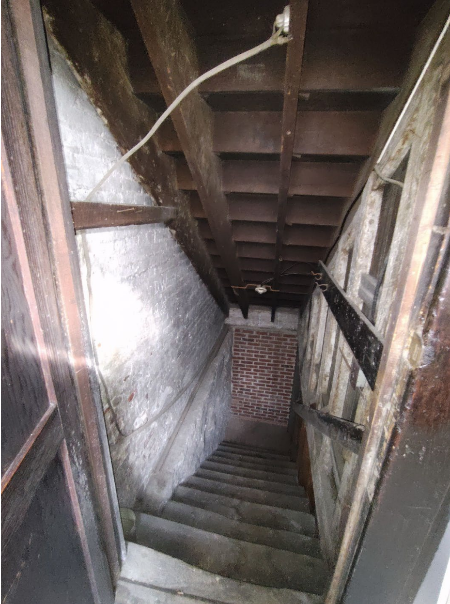
Photograph 55. View: basement stairwell interior, facing southeast WV_RandolphCo_OddFellowsHome_0055
