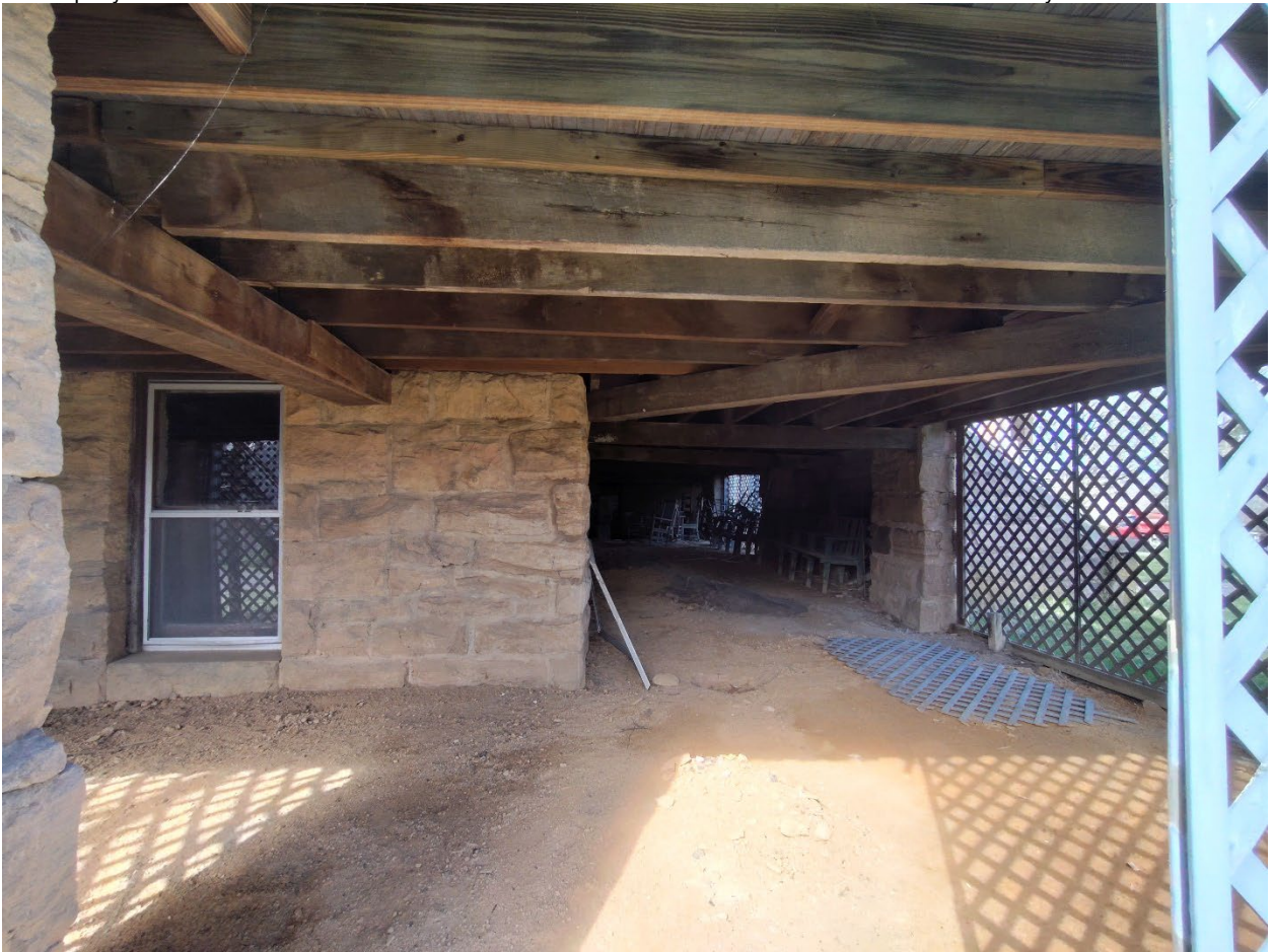
Photograph 10. View: south corner foundation exterior (under porch), facing northeast WV_RandolphCo_OddFellowsHome_0010
