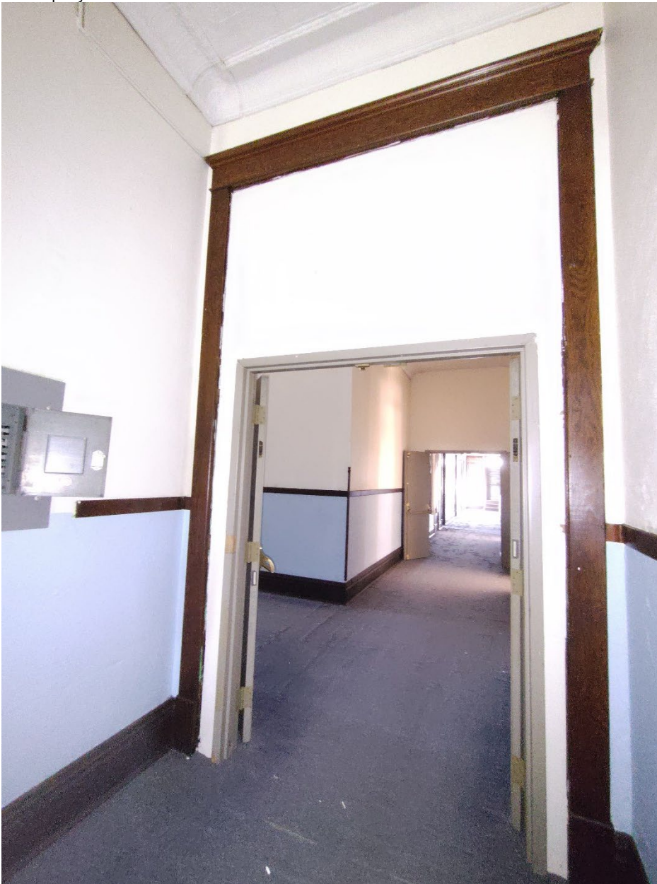
Photograph 37. View: second floor hallway interior, facing southwest WV_RandolphCo_OddFellowsHome_0037
