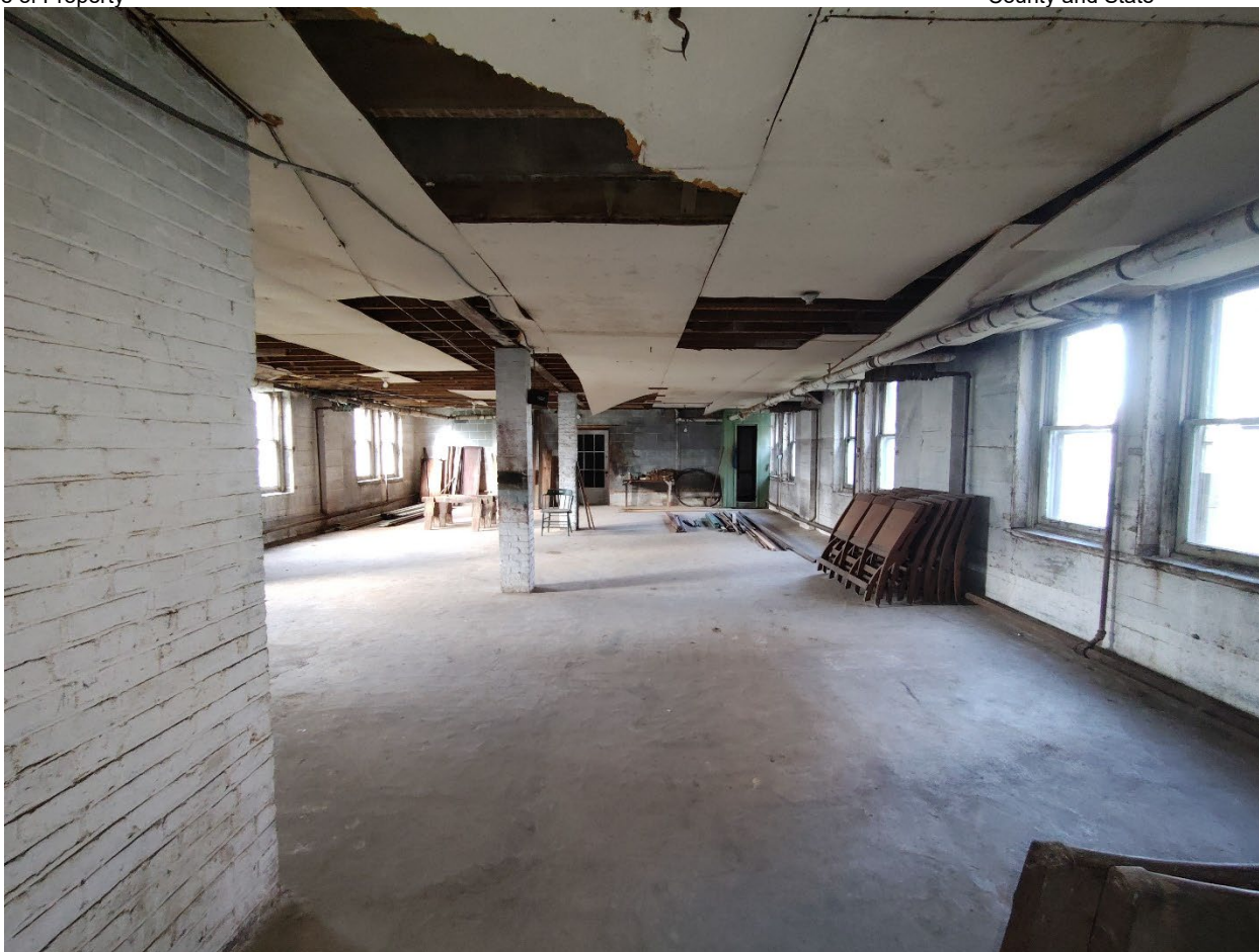
Photograph 60. View: basement interior, facing northeast WV_RandolphCo_OddFellowsHome_0060
