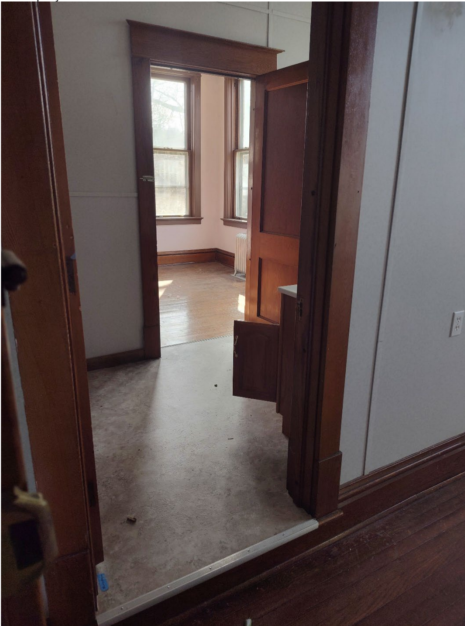
Photograph 43. View: second floor bathroom interior, facing west WV_RandolphCo_OddFellowsHome_0043
