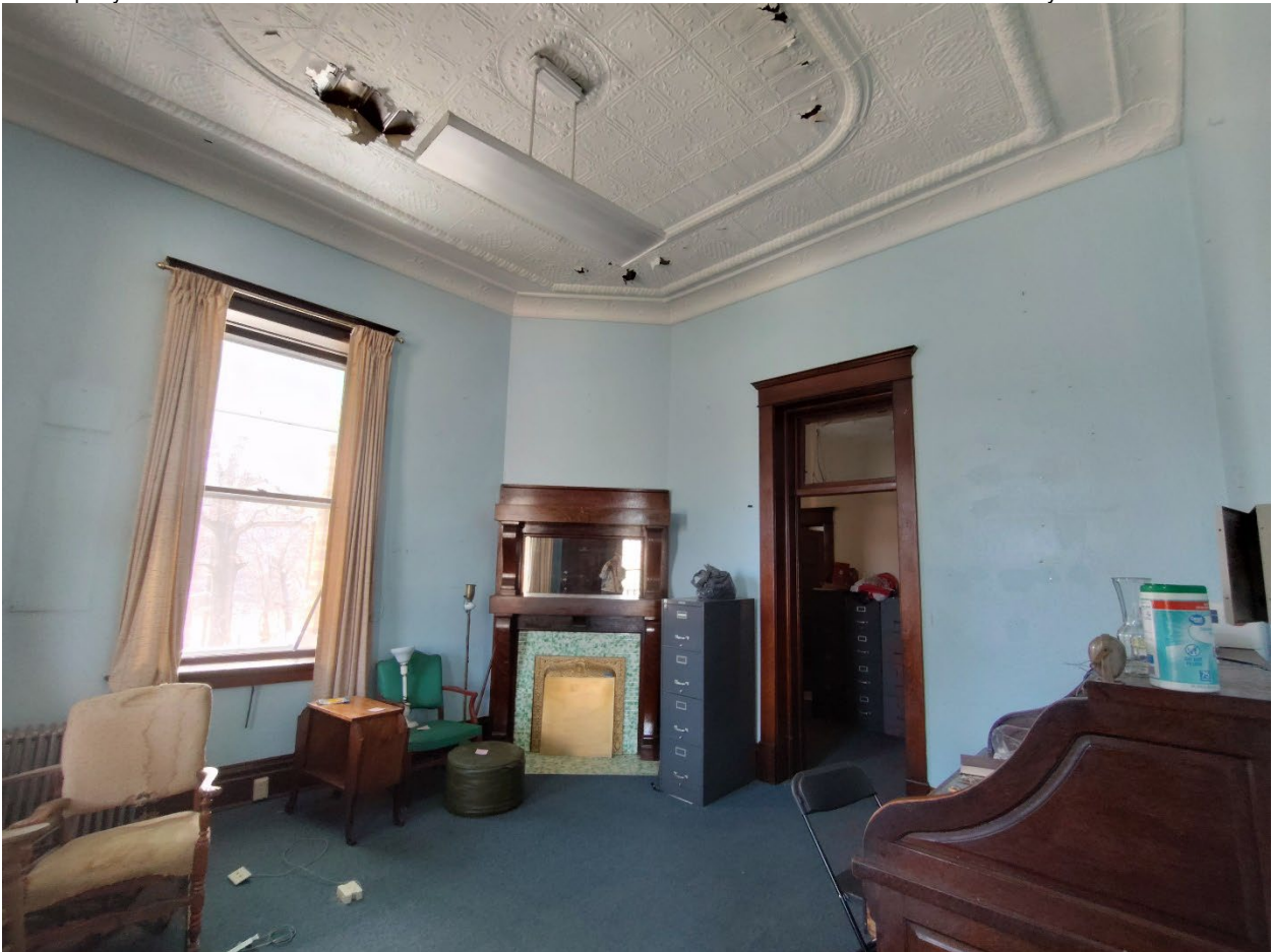
Photograph 20. View: first floor parlor interior, facing west WV_RandolphCo_OddFellowsHome_0020
