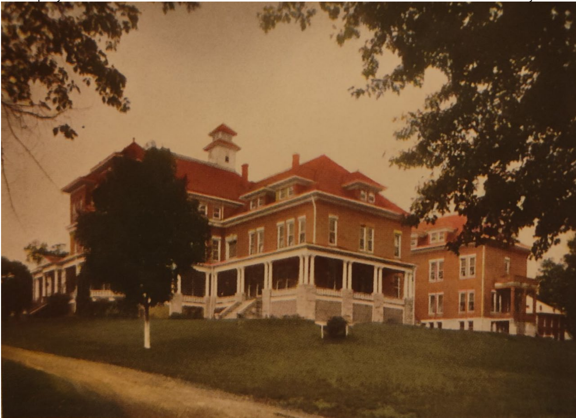
Figure 14: Historic photo, northeast elevation with recently completed addition and carriage house visible at rear, 1927.
