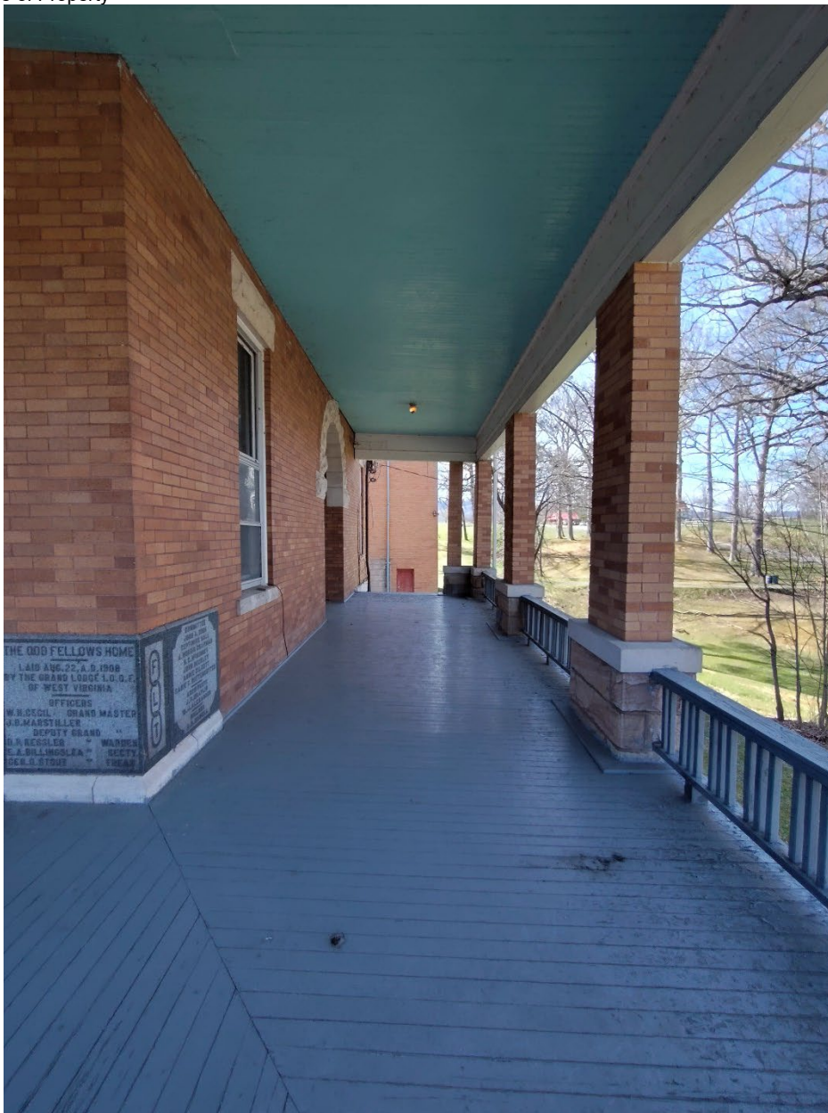
Photograph 5. View: east corner exterior, facing northwest WV_RandolphCo_OddFellowsHome_0005
