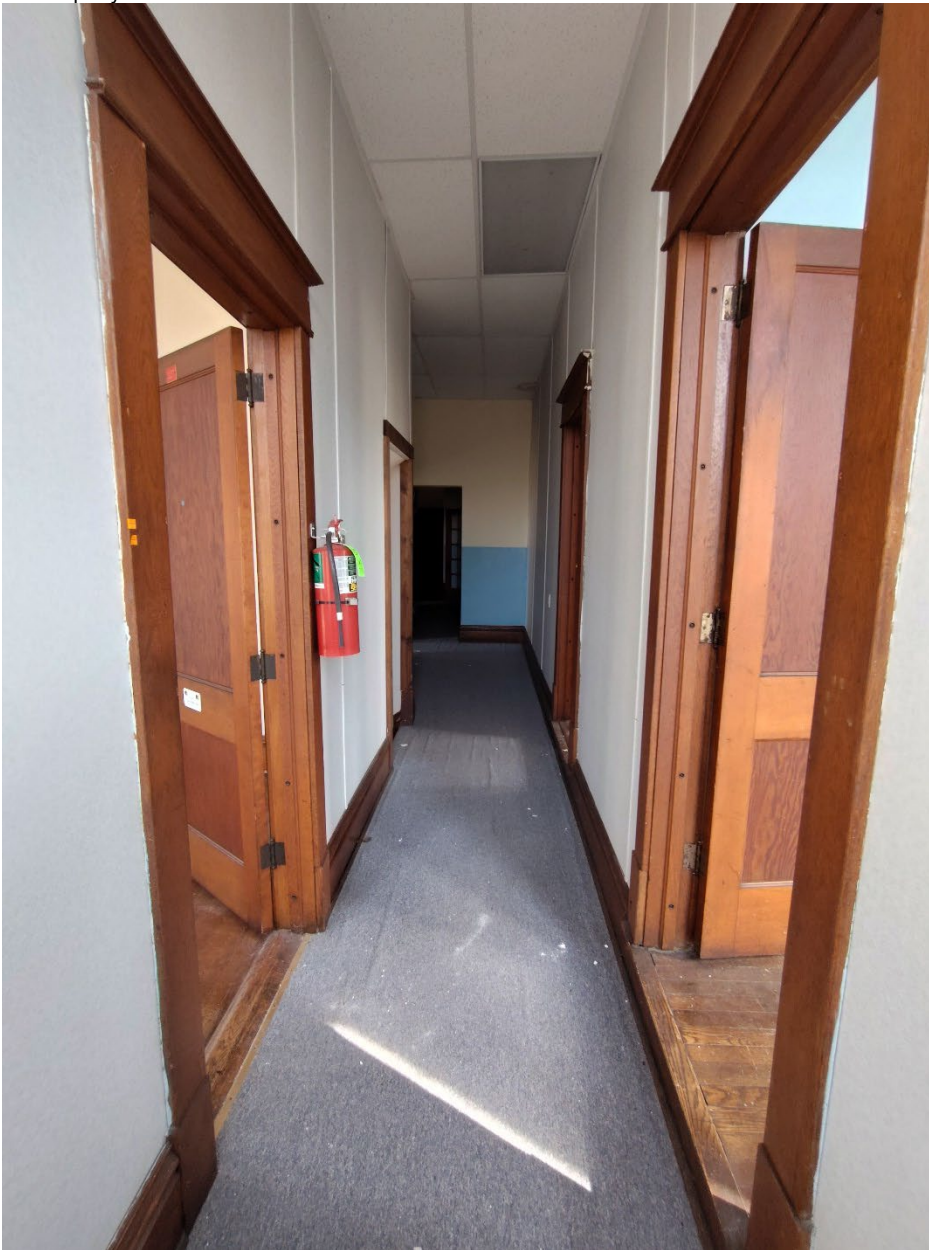
Photograph 44. View: second floor hallway interior, facing southeast WV_RandolphCo_OddFellowsHome_0044
