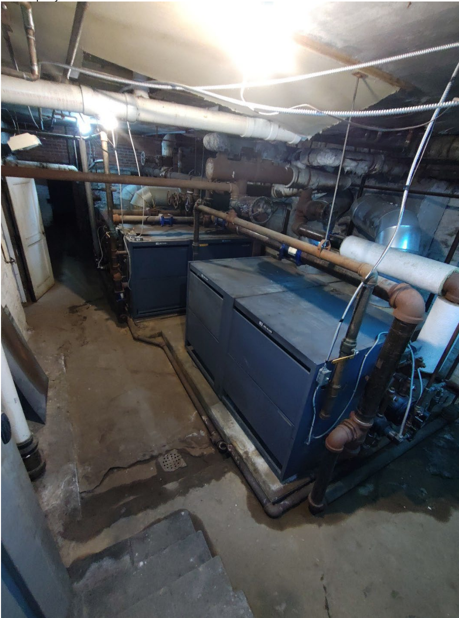
Photograph 56. View: basement interior, facing southwest WV_RandolphCo_OddFellowsHome_0056
