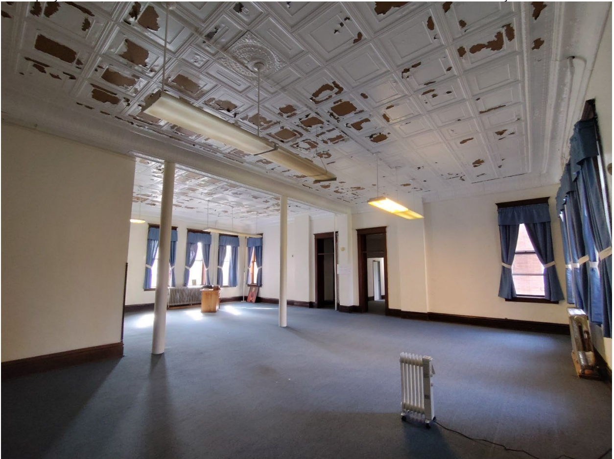
Photograph 28. View: first floor interior, facing west WV_RandolphCo_OddFellowsHome_0028
