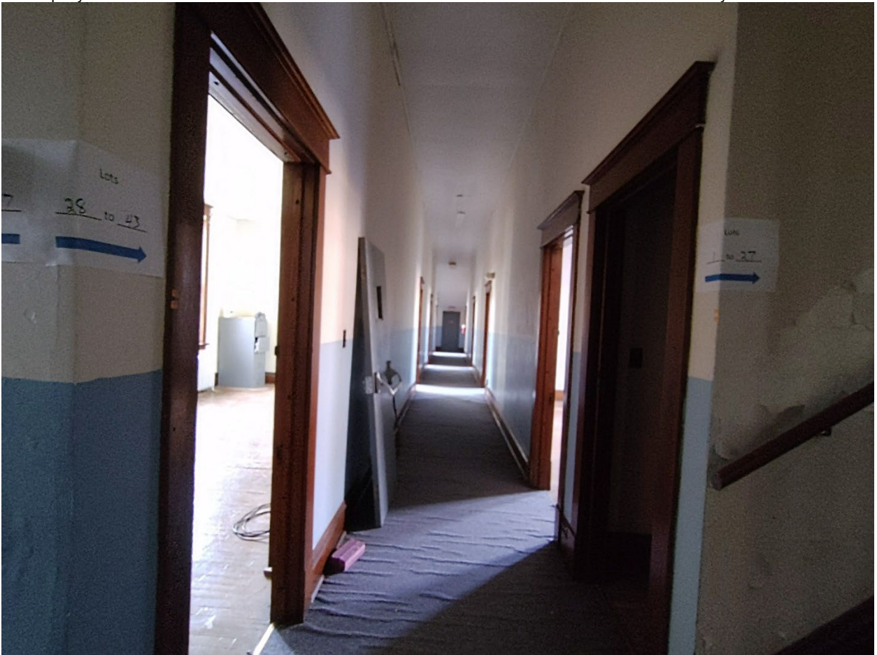
Photograph 41. View: second floor hallway interior, facing northeast WV_RandolphCo_OddFellowsHome_0041
