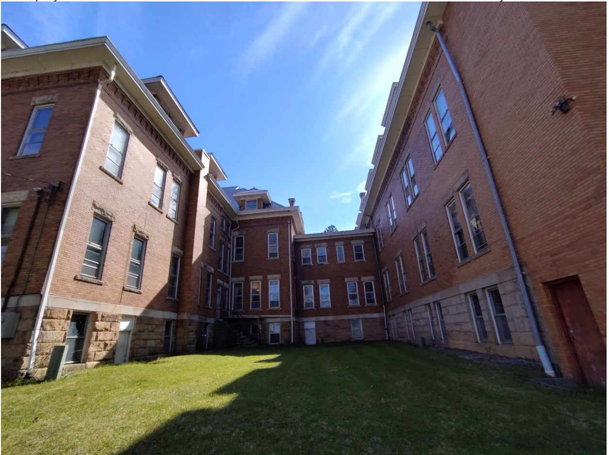
Photograph 7. View: northeast elevation, facing southwest WV_RandolphCo_OddFellowsHome_0007
