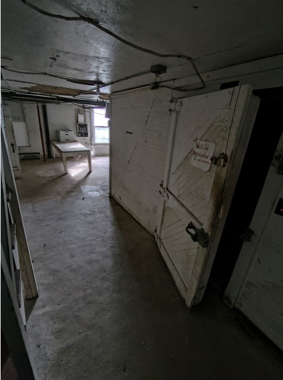
Photograph 59. View: basement interior, facing southwest WV_RandolphCo_OddFellowsHome_0059
