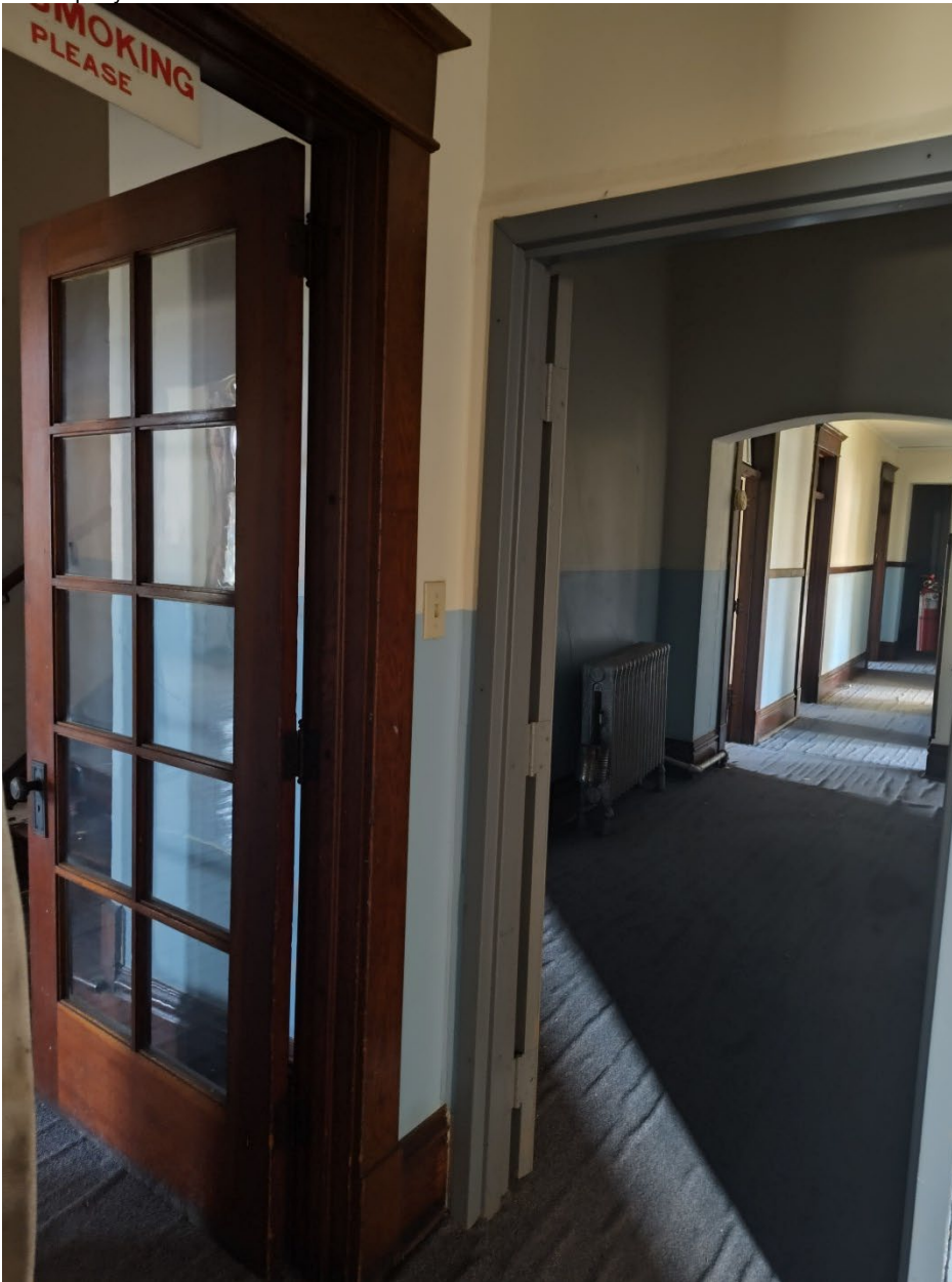
Photograph 40. View: second floor hallway interior, facing east WV_RandolphCo_OddFellowsHome_0040
