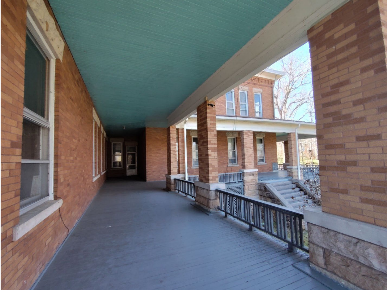
Photograph 4. View: east corner exterior, facing northwest WV_RandolphCo_OddFellowsHome_0004
