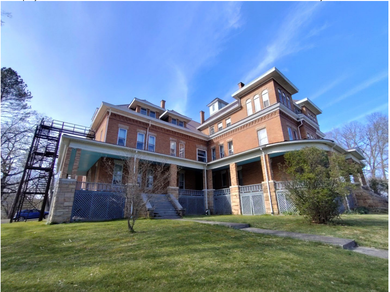
Photograph 11. View: south corner exterior, facing north WV_RandolphCo_OddFellowsHome_0011
