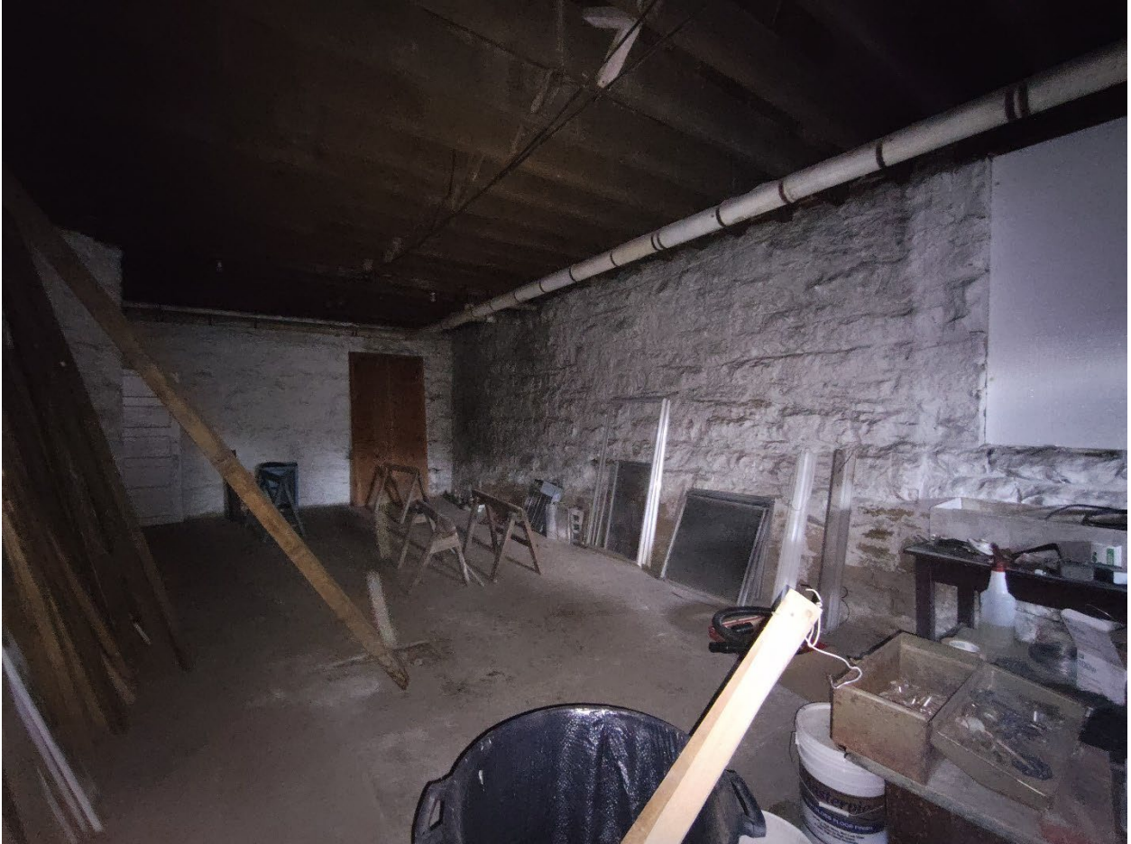
Photograph 58. View: basement interior, facing northeast WV_RandolphCo_OddFellowsHome_0058
