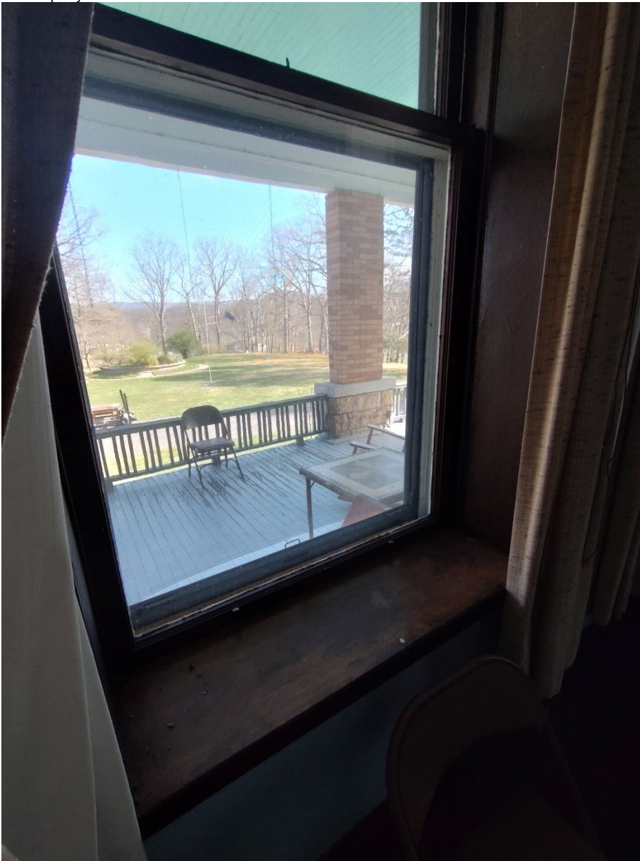
Photograph 21. View: first floor interior window detail, facing southeast WV_RandolphCo_OddFellowsHome_0021
