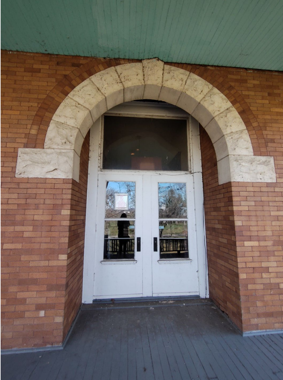
Photograph 6. View: northeast elevation, facing southwest WV_RandolphCo_OddFellowsHome_0006
