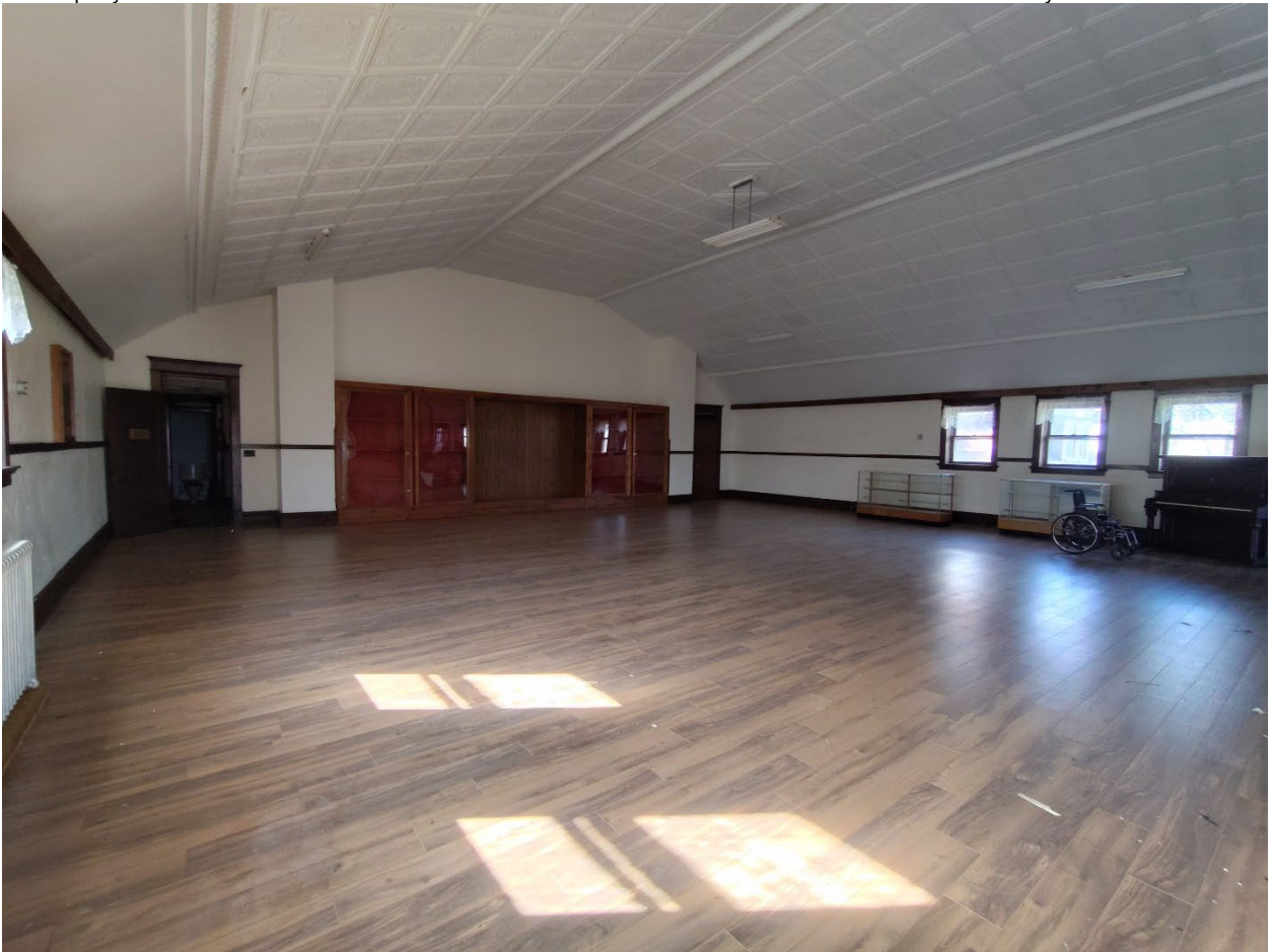
Photograph 49. View: third floor meeting hall, facing north WV_RandolphCo_OddFellowsHome_0049
