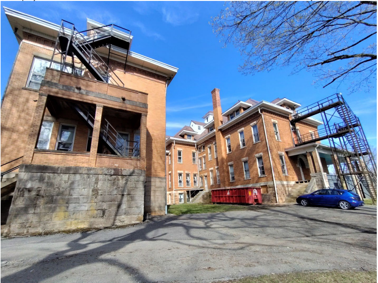
Photograph 9. View: southwest elevation, facing east WV_RandolphCo_OddFellowsHome_0009
