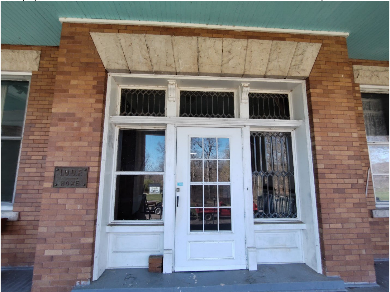
Photograph 3. View: front façade/southeast elevation, facing northwest WV_RandolphCo_OddFellowsHome_0003
