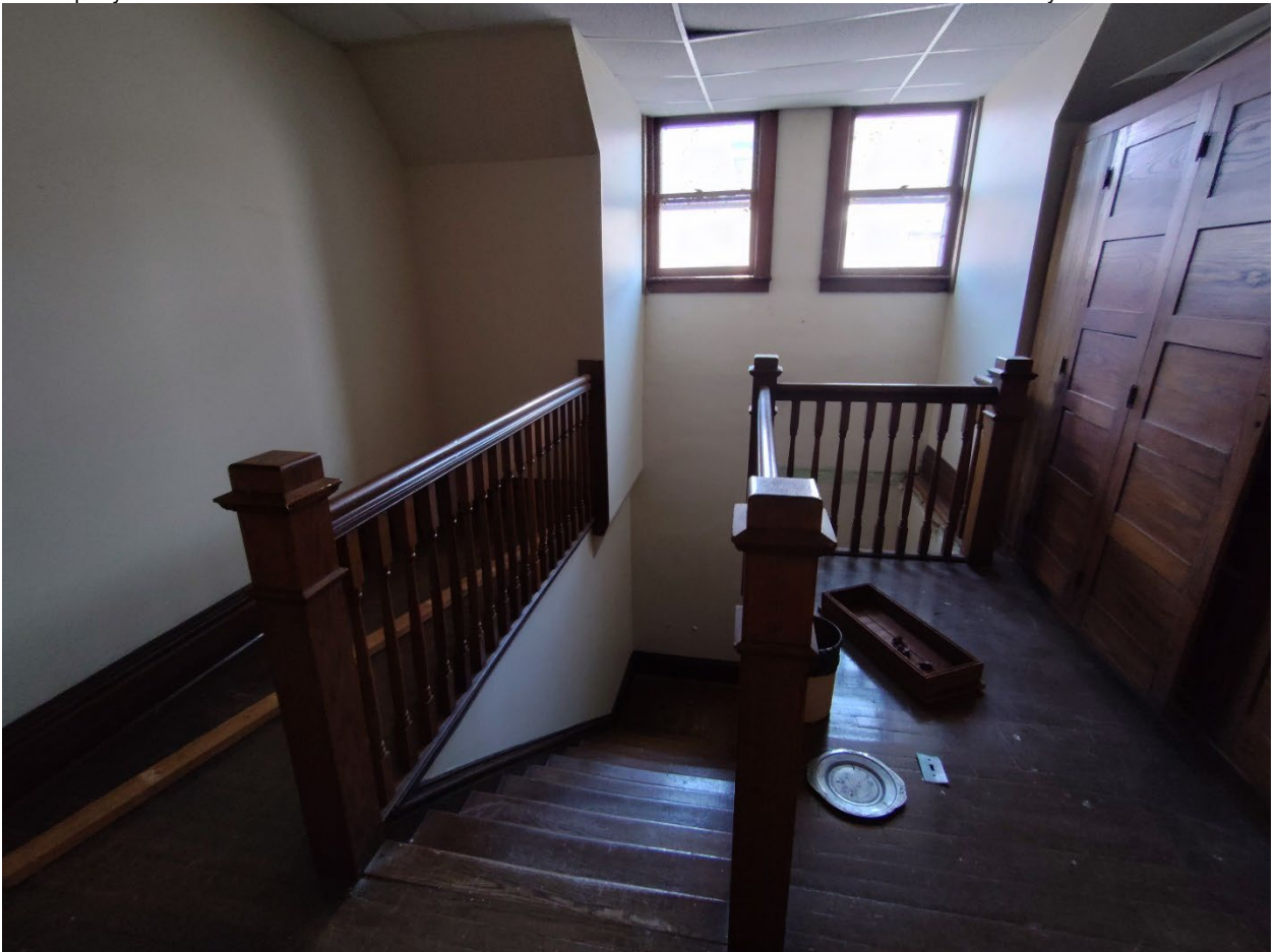
Photograph 52. View: third floor stairwell, facing southeast WV_RandolphCo_OddFellowsHome_0052
