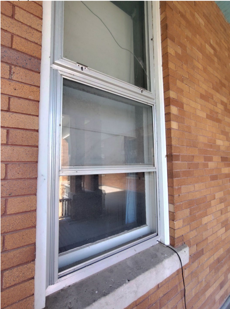
Photograph 12. View: southeast elevation window detail, facing north WV_RandolphCo_OddFellowsHome_0012
