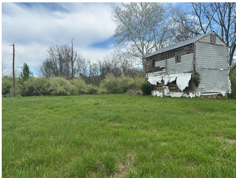
WV_Hampshire_Edwards' Fort_Photo 003, site setting and log Poston house, looking northeast, April 18, 2026.
