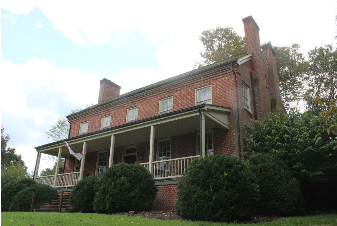
Photo 4. North and west elevations, oblique view, camera facing SE.
