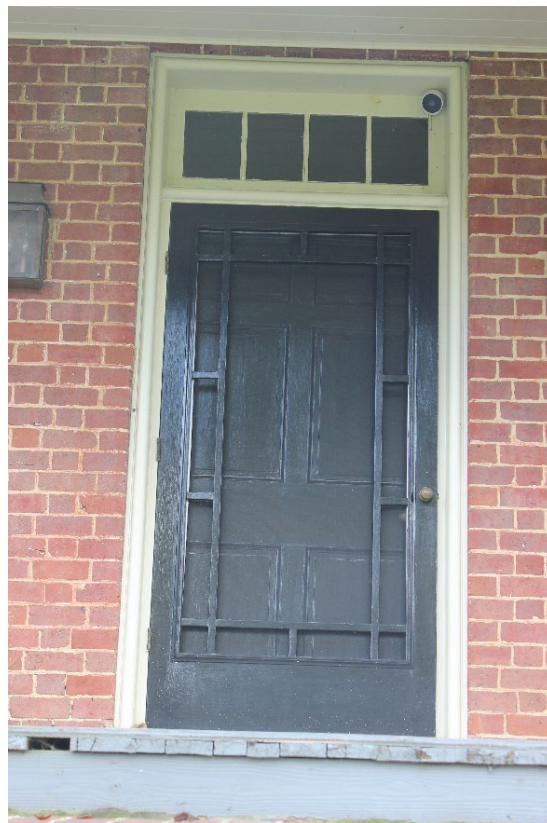
Photo 6. Front door on north elevation, camera facing S.
