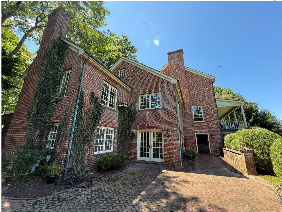
Photo 5. East addition, camera facing W.
