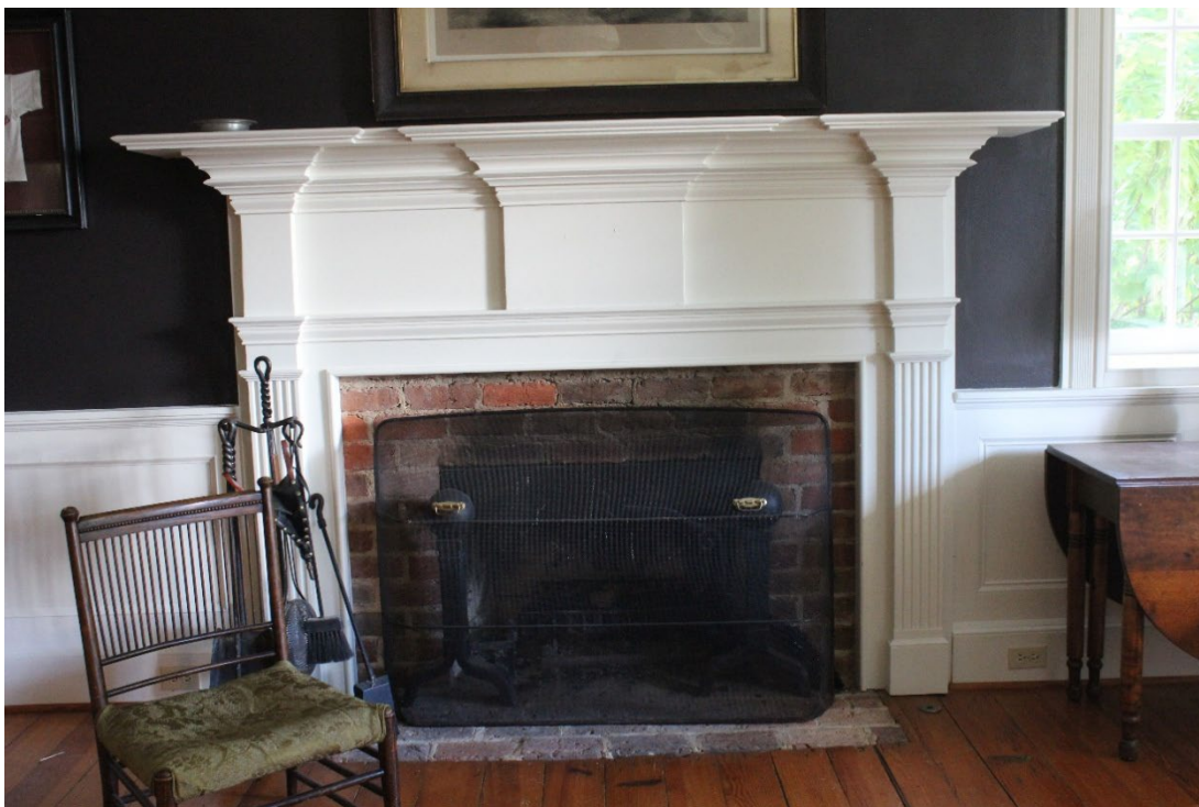
Photo 8. Interior detail of fireplace in west first floor parlor.
