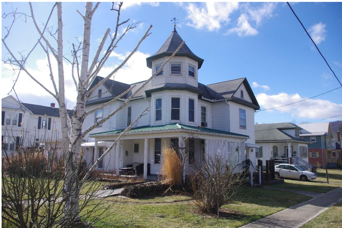
Photograph 26. 85 N Bolton (Map No. 99), camera facing southwest.
