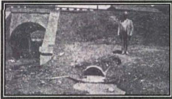
Fig 10 The work of the Pietro Company extended to the laying of culverts and sewers as well as paving. Here Thoney Pietro is shown beside a recently-installed drainage culvert.
