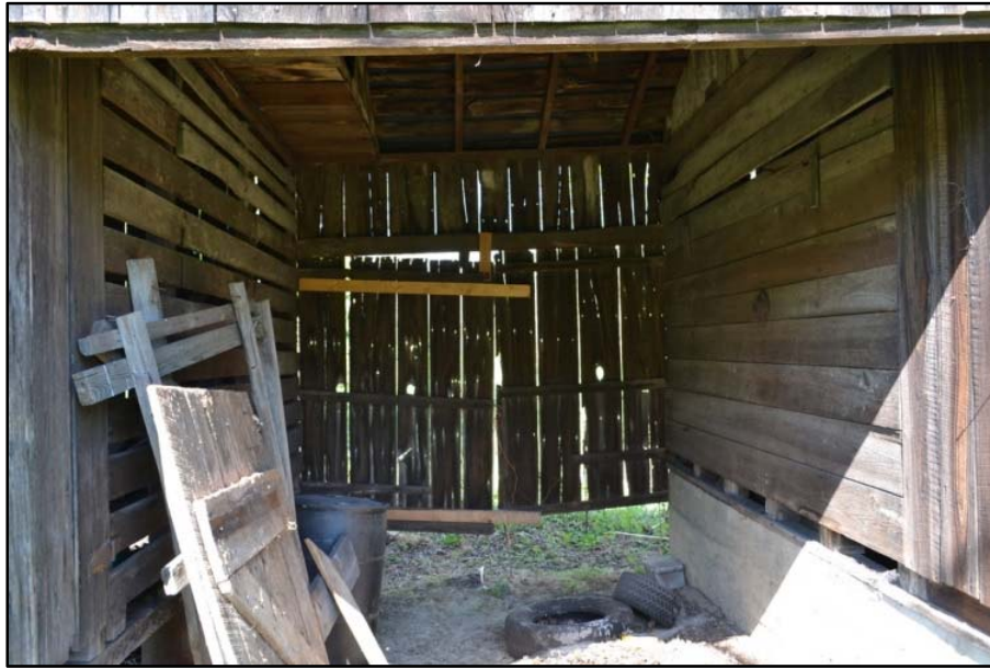
Figure 19 Drive-through of the corncrib.
