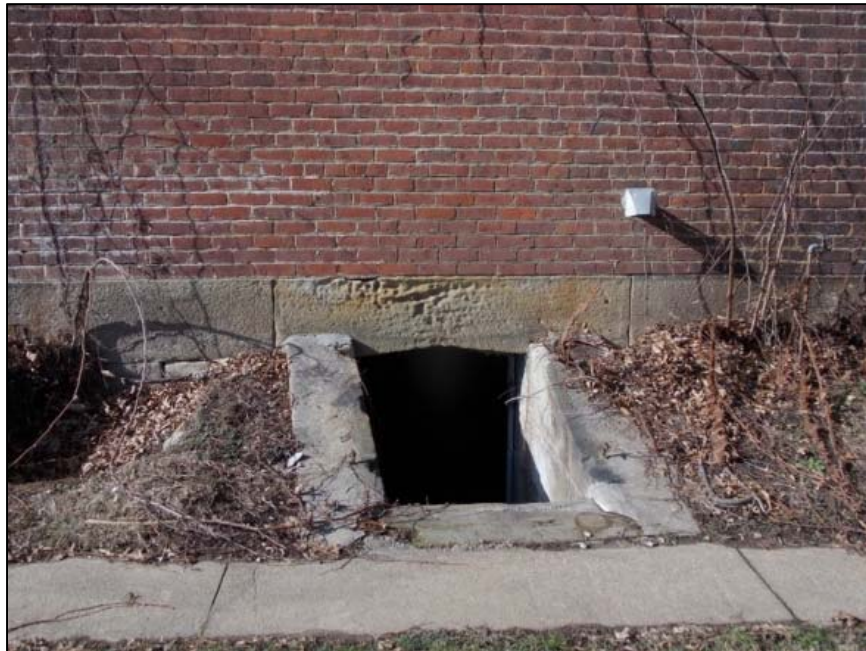
Figure 11 Cellar entry on south gable end of house.
