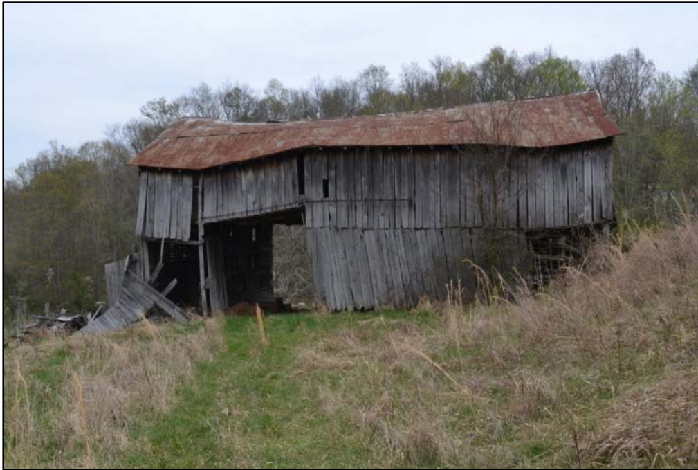
Figure 75 The barn at WA-0201
