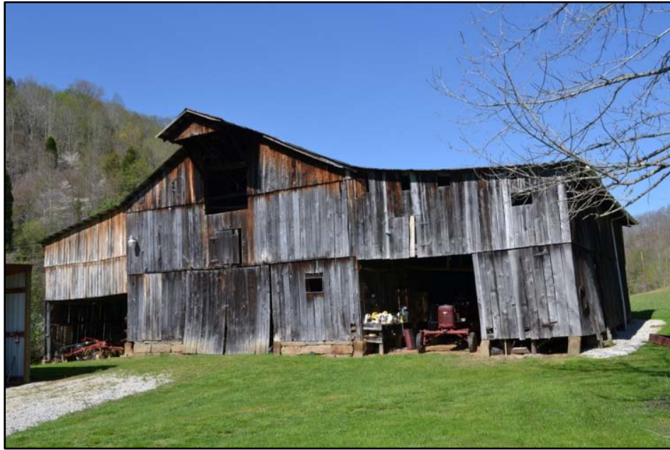
Figure 88 Transverse frame barn with side shed additions, WA-0212.
