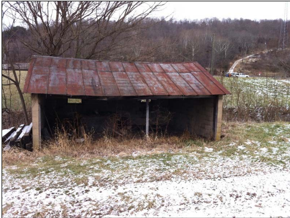
Figure 22 Resource 9, facing east.
