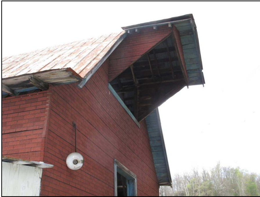
Figure 95 Hay hood at WA-0224.
