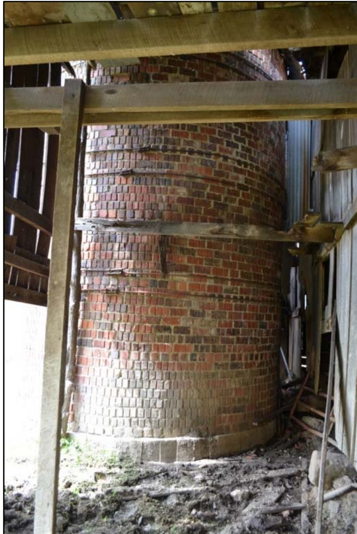
Figure 119 Circa 1937 silo made from brick pavers at WA-0199.
