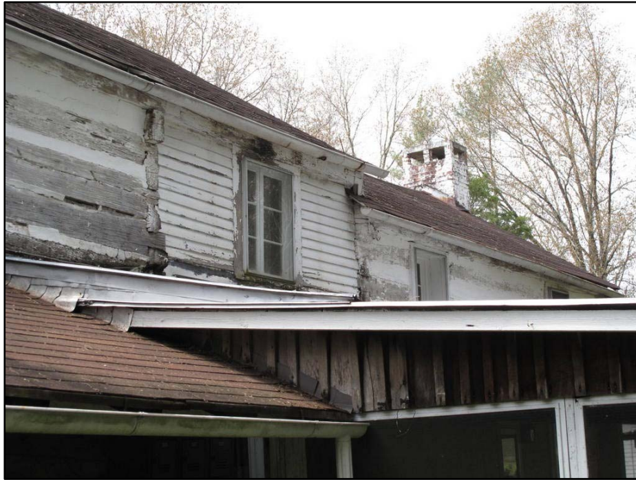
Figure 46 Detail of the enclosed dogtrot between the two pens, WA-0223.
