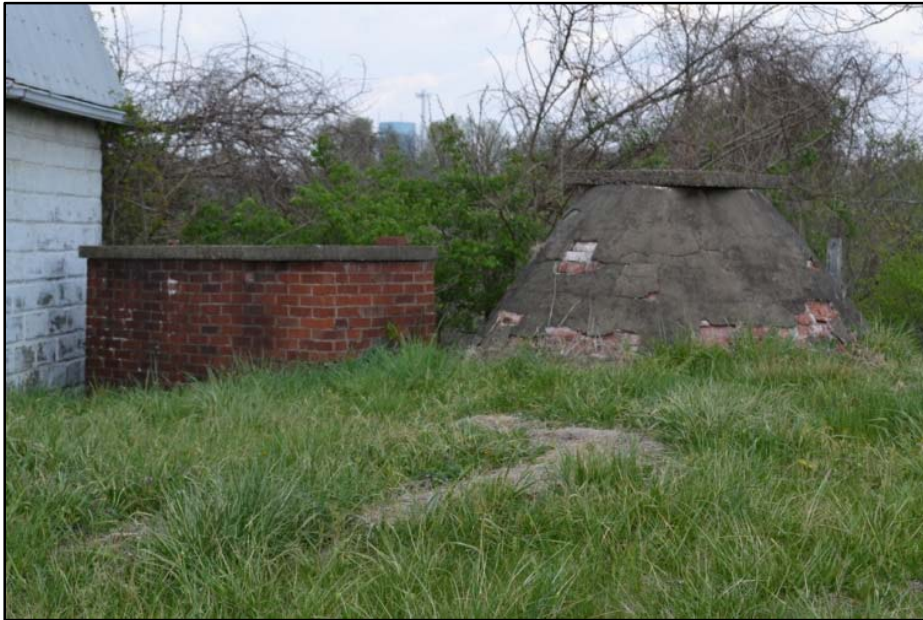
Figure 131 Beehive cistern and filter at WA-0204.
