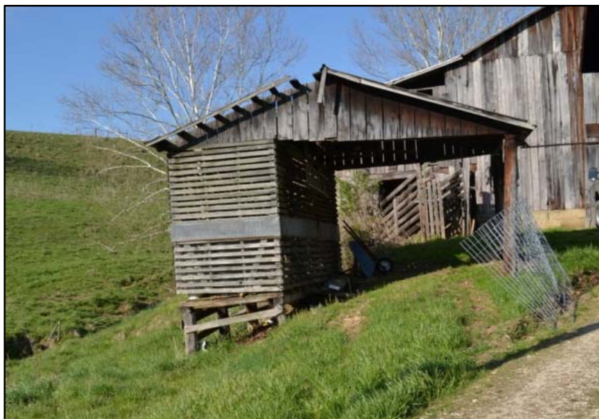
Figure 107 Single crib corncrib with shed roof addition at WA-0209.
