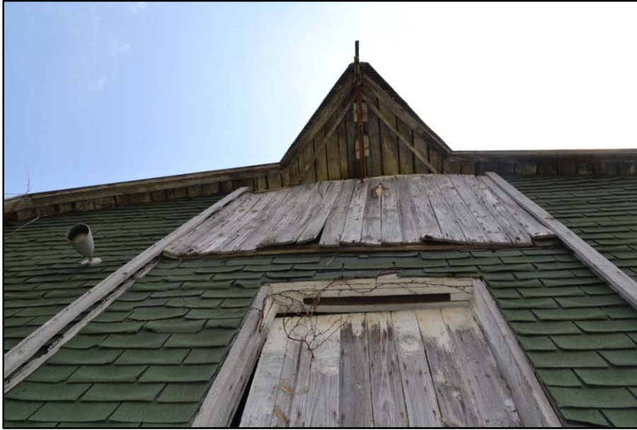
Figure 91 Hay hood at WA-0204.
