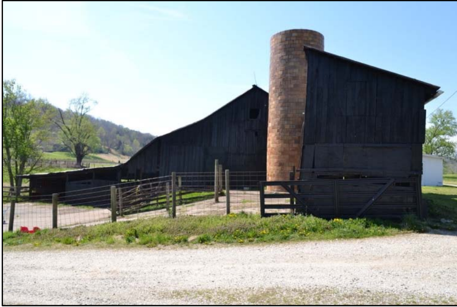
Figure 32 Bank barn (Resource 7), Facing south.
