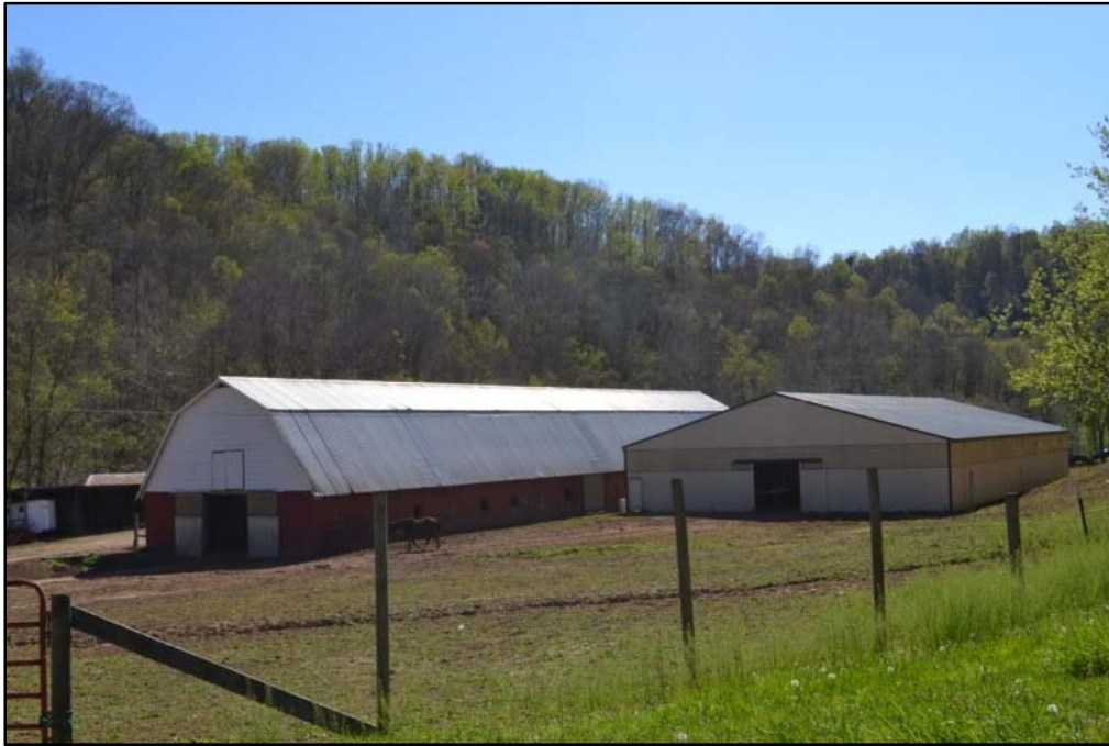
Figure 97 The dairy barn at WA-0220 is on left in the photo.
