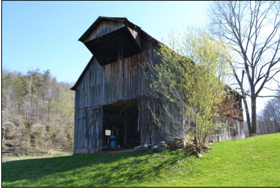
Figure 85 Gable end with hay hood of the transverse frame barn at WA-0211.
