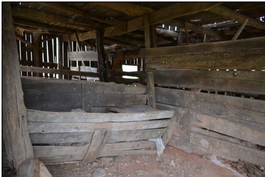
Figure 77 One of the built-in troughs/mangers at WA-0201.
