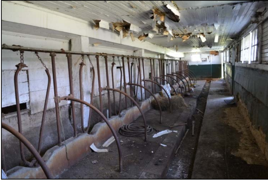
Figure 36 Milking parlor on west side of barn.
