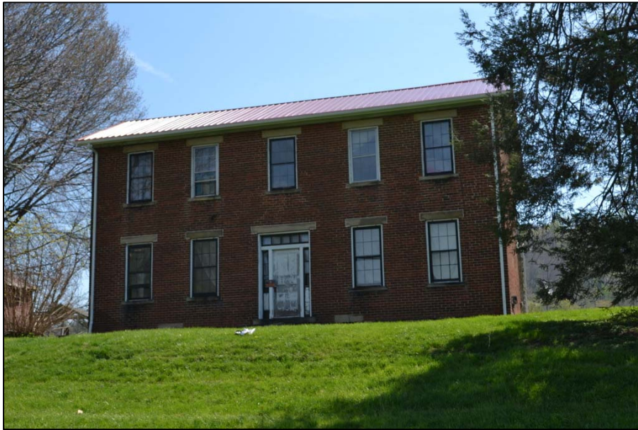
Figure 8 Façade, facing east.
