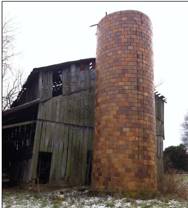
Figure 27 North gable end of barn and silo
