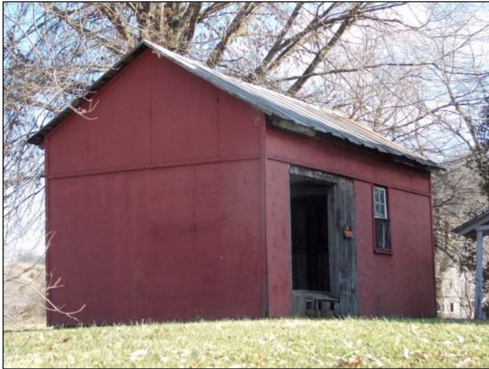
Figure 166 Domestic outbuilding (Resource 4), facing southeast.
