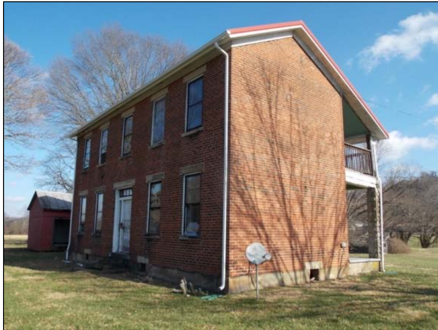
Figure 12 Façade and south gable end.
