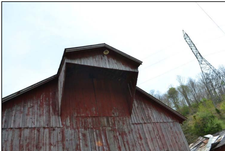
Figure 94 Hay hood at WA-0200.
