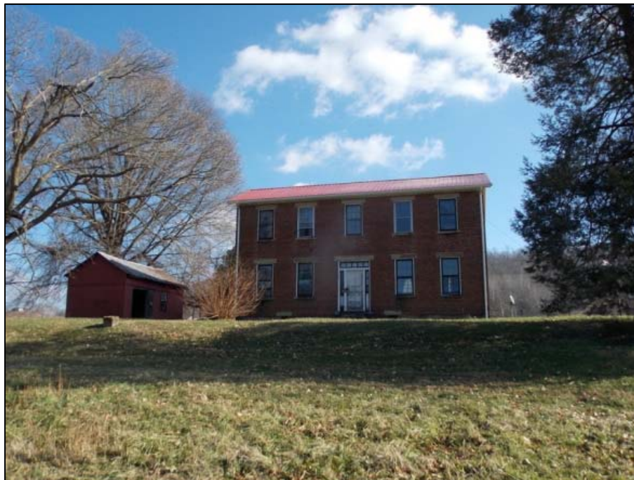
Figure 7 Façade of Roswell Cyrus House (Resource 5) and domestic outbuilding, facing east.
