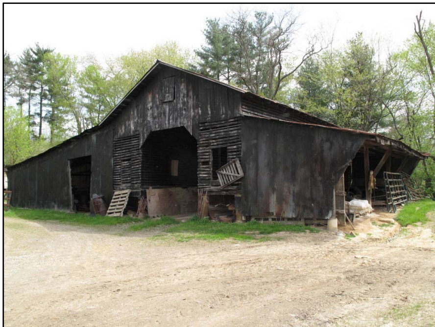
Figure 114 Drive-through corncrib with side shed additions at WA-0223.
