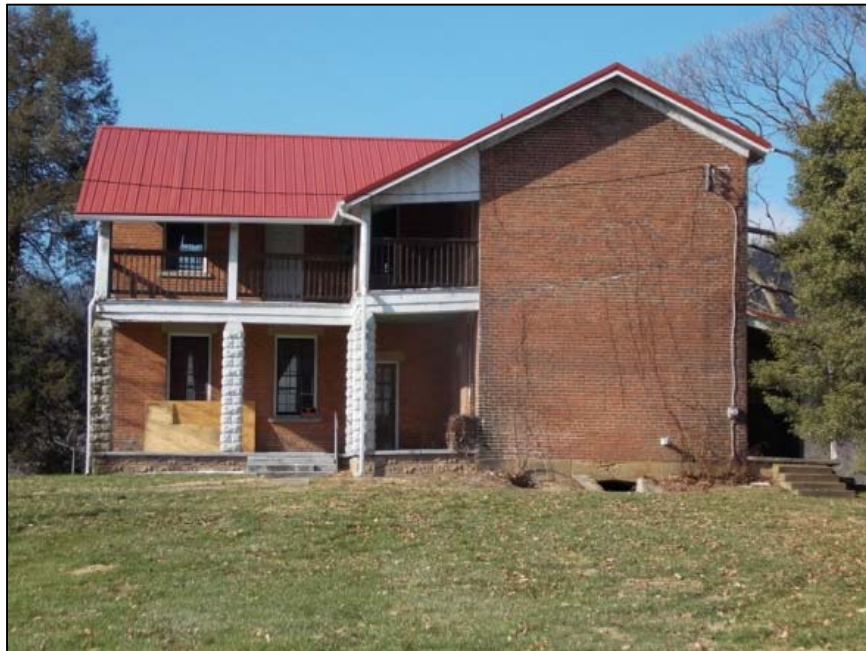
Figure 144 East elevation of main block and ell.
