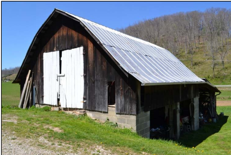
Figure 81 Bank barn at WA-0217. This barn demonstrates both the English and Transverse Frame plans.
