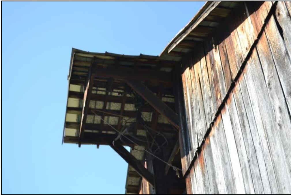
Figure 90 Front gable braced hay hood with hay rake extant, at WA-0212.
