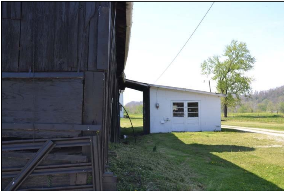
Figure 33 Concrete block milk house on west side of barn.
