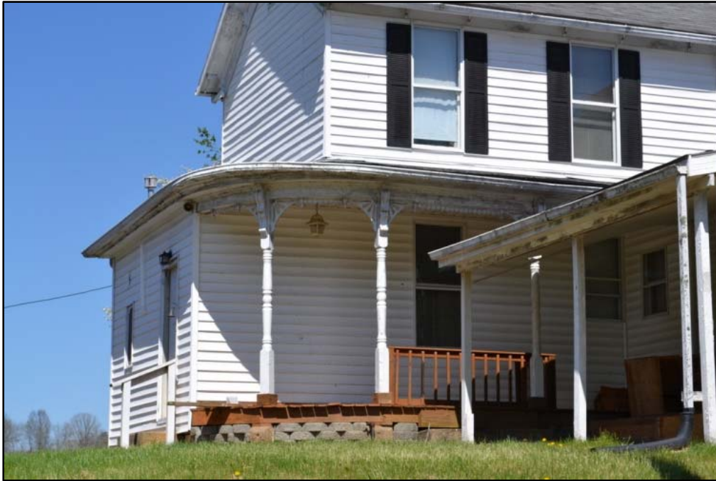
Figure 47 The brackets, turned and chamfered porch posts and sawtooth frieze are all machine made elements applied to the curved porch of the late-19 th century house at WA-0214.
