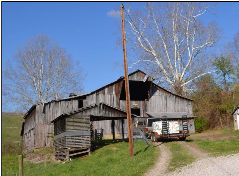
Figure 89 Transverse frame barn with enclosed side shed additions, WA-0209.
