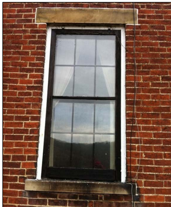
Figure 9 Detail of window and sill.
