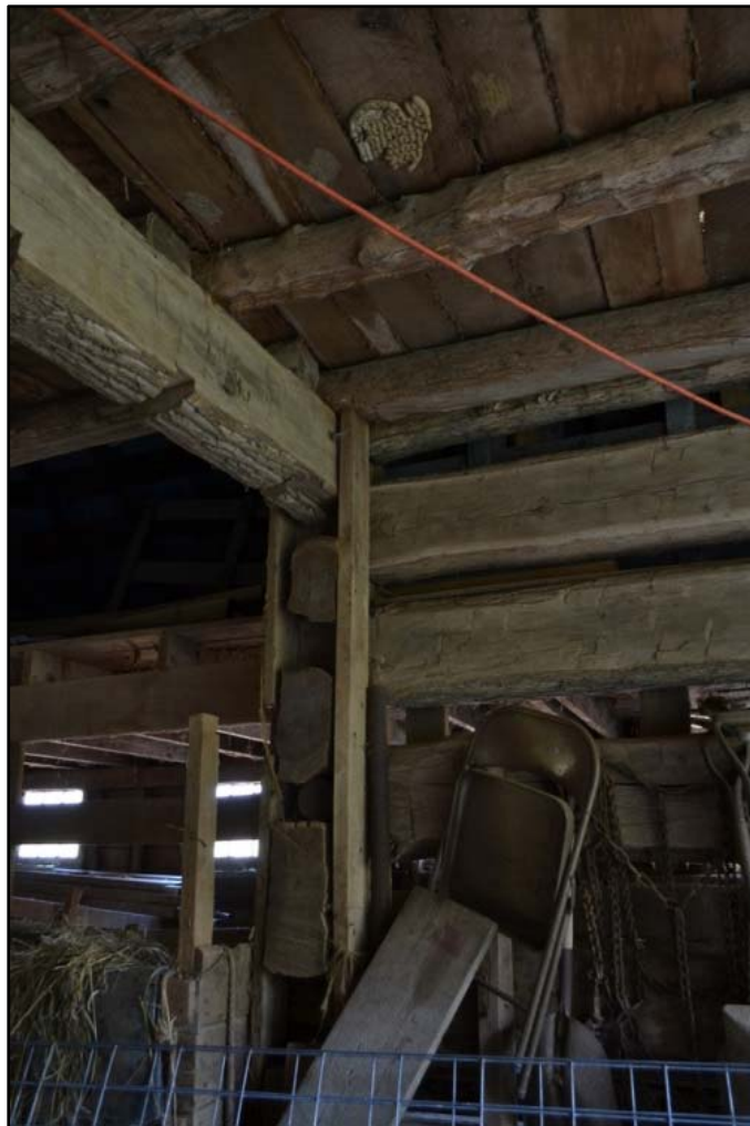
Figure 74 A portion of the log crib inside the barn at WA-0210.
