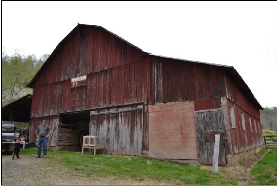
Figure 100 The transverse stock barn at WA-0203 had a milking parlor added in the mid-20 th century (shed roof addition on right in photo).
