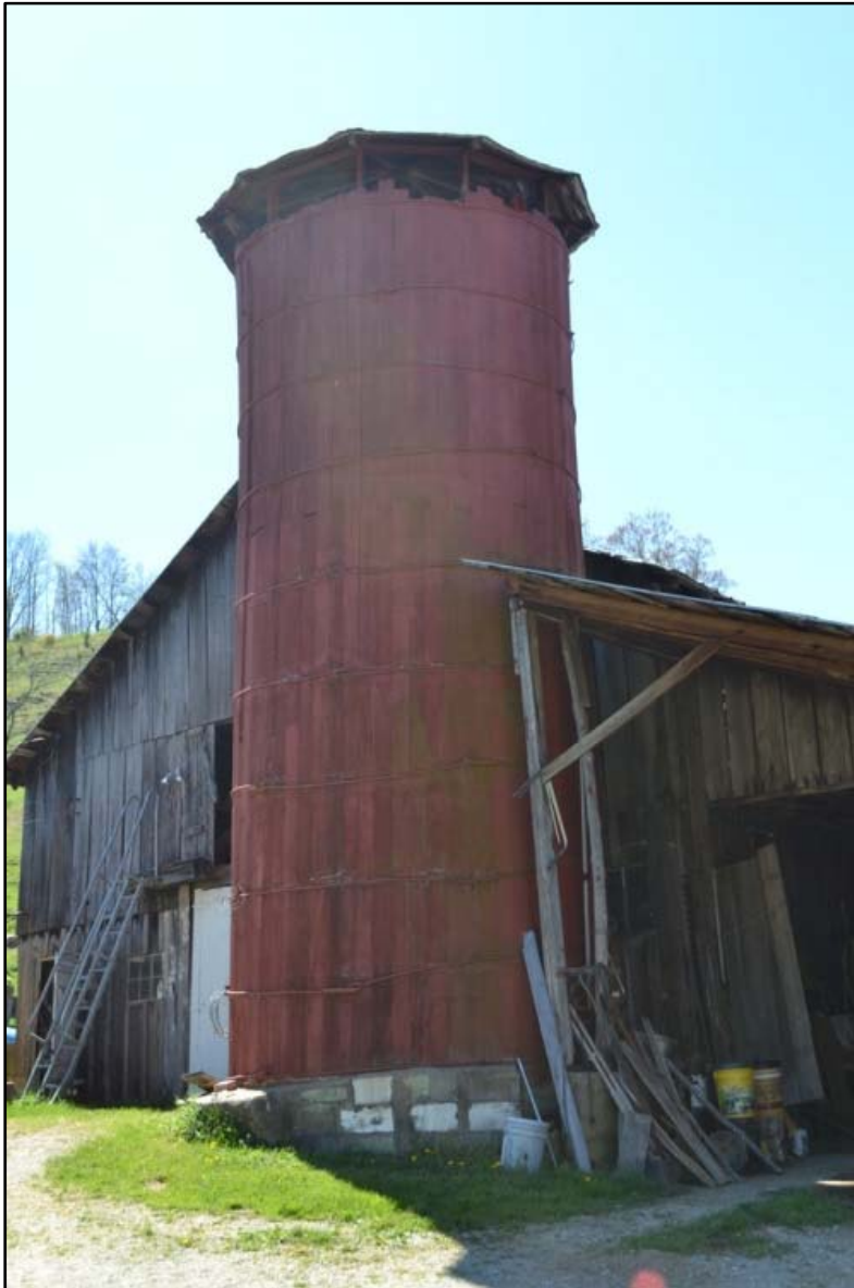
Figure 120 Wooden stave silo at WA-0217.
