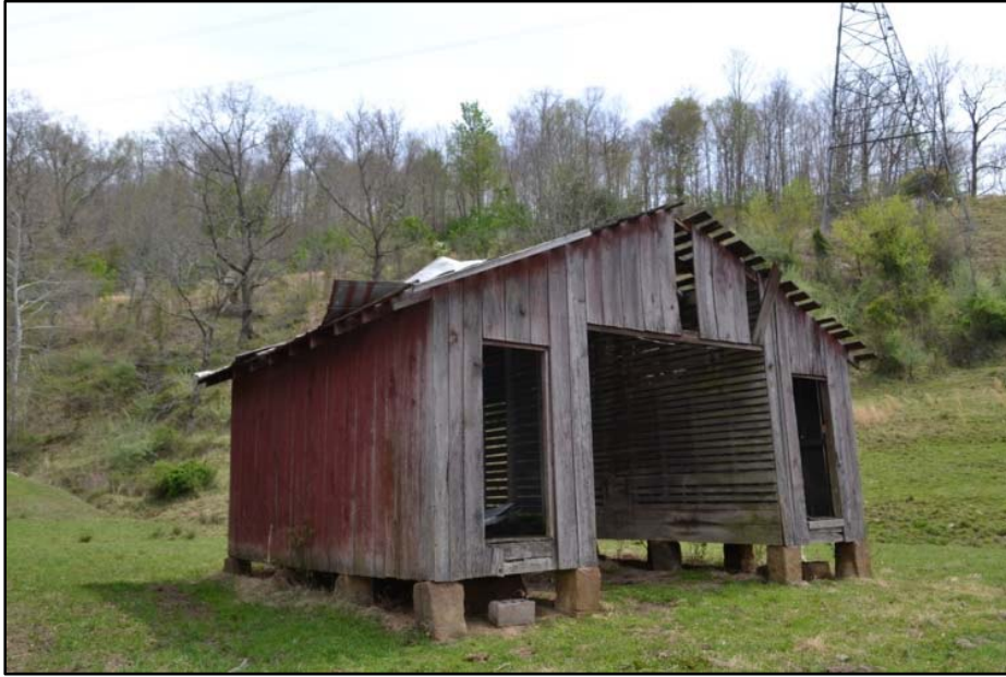
Figure 111 A typical gable-oriented drive-through corncrib at WA-0200.
