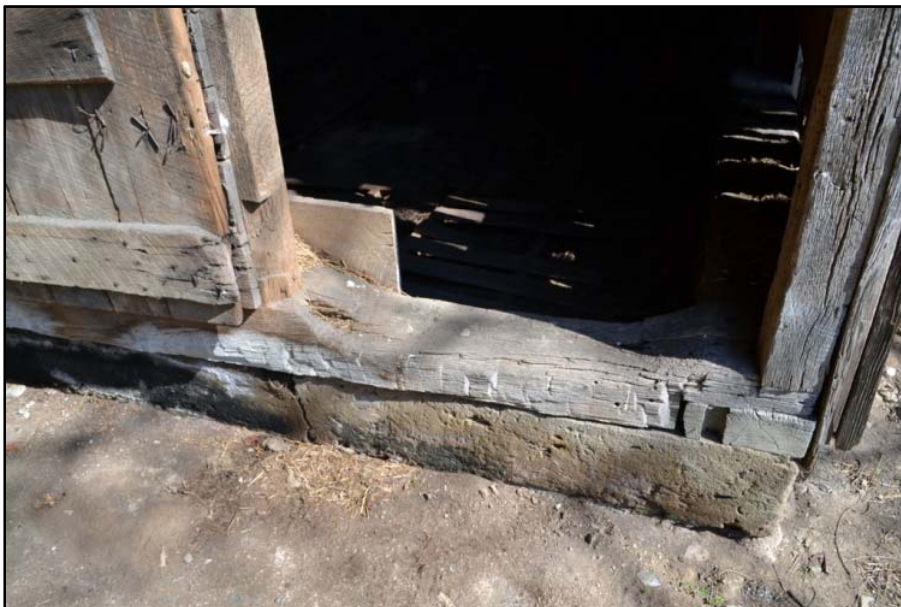
Figure 25 Sills with hewn marks in lower level of barn.
