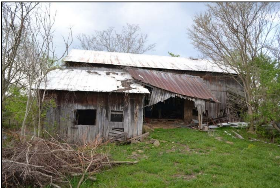
Figure 83 The bank barn at WA-0204 illustrates the English plan entrance. The shed addition to the left of the main entry was used to stable two work horses.
