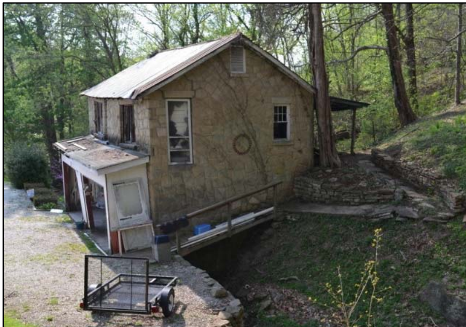
Figure 60 Partially banked garage and apartment at WA-0207.
