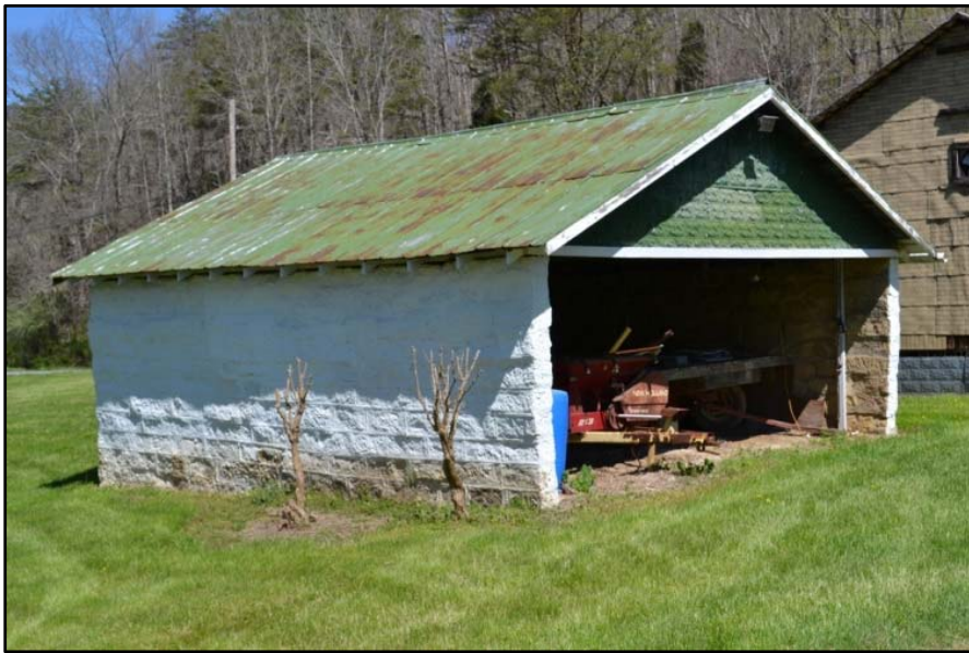
Figure 64 This rusticated concrete block garage with its exposed rafter tails, associated with WA-0215, displays the influence of the Craftsman style.
