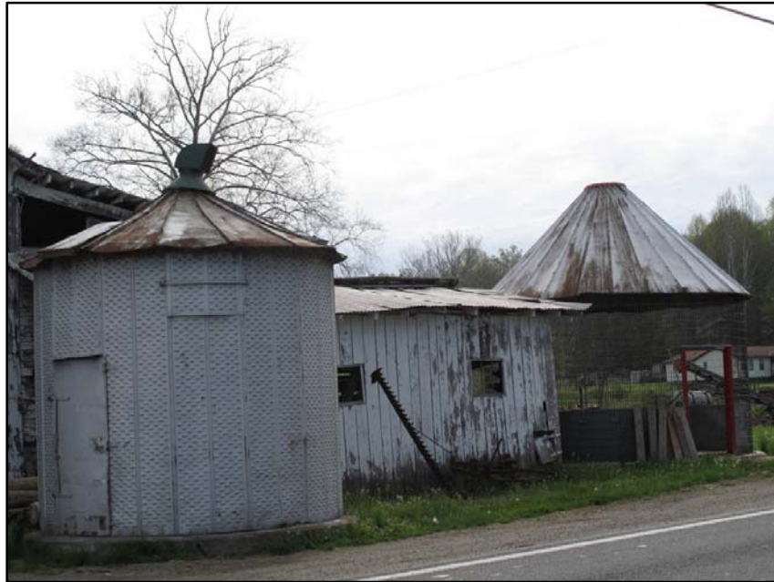
Figure 117 Three different types of corncribs are shown at WA-0221 – a metal crib, a wooden crib (the side facing the road has been modified) and a wire mesh crib.
