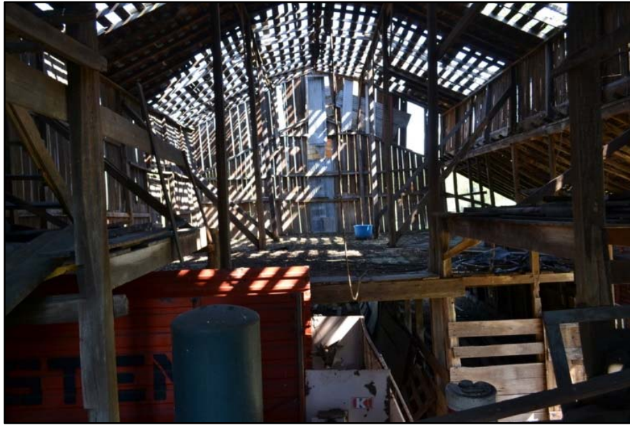
Figure 29 Looking north in loft, upper level of barn.
