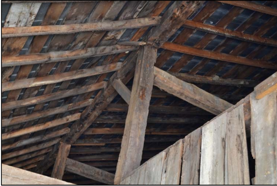
Figure 34 Hewn timbers in barn.
