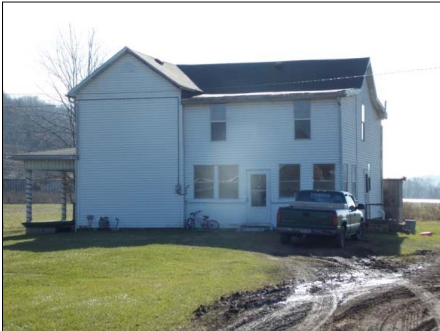
Figure 40 North elevation, showing ell.
