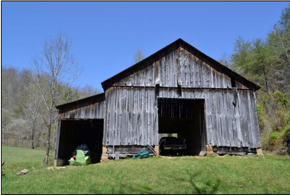
Figure 87 Transverse frame barn with side shed addition at WA-0216. This barn dates to the first quarter of the 20 th century.
