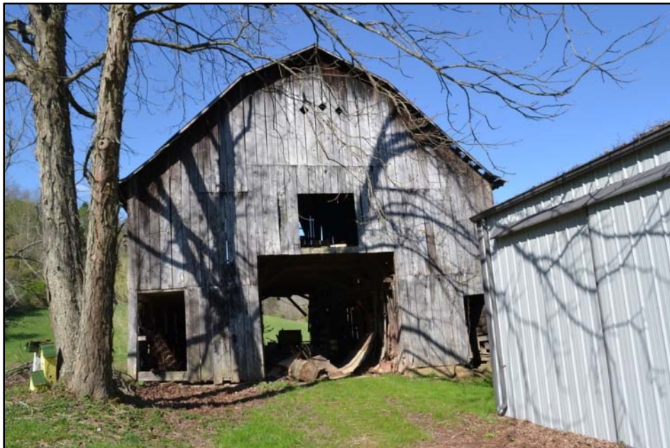
Figure 86 The other gable end of the WA-0211 barn.
