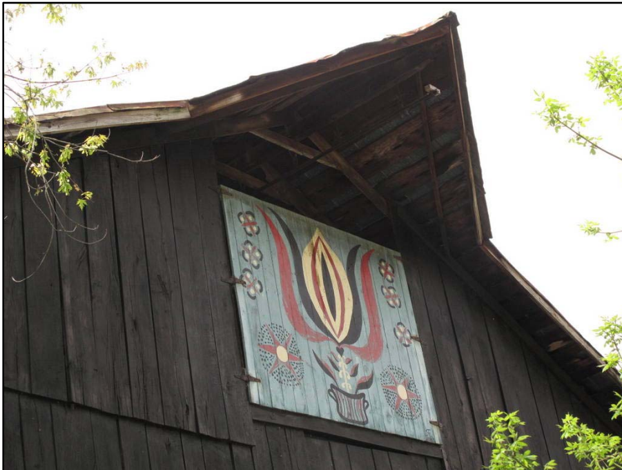
Figure 92 Hay hood at WA-0223.
