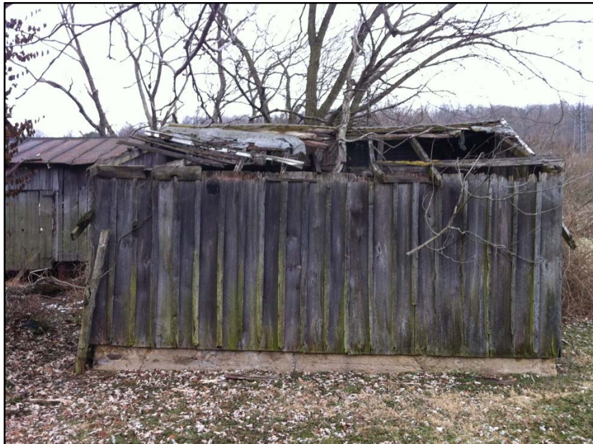
Figure 20 Resource 3, facing east.
