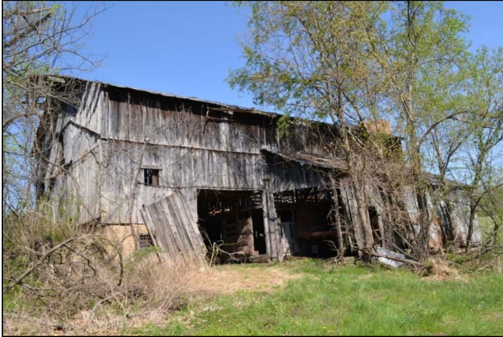
Figure 23 East elevation of barn.
