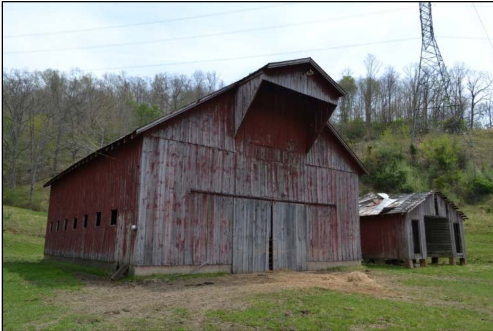
Figure 84 Transverse frame barn at WA-0200. This barn, which rests on a concrete block foundation, dates from the mid-1950s.
