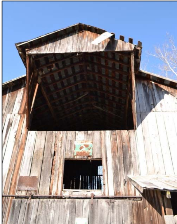
Figure 93 Hay hood at WA-0209.
