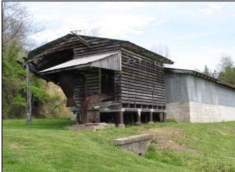
Figure 108 The single crib corncrib at WA-0224 has a gable overhang, and is set up with a machine-powered cornsheller, which is shielded from the weather by a shed roof overhang.
