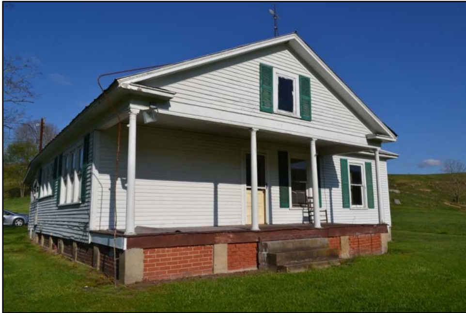
Figure 69 This asymmetrical, front gable dwelling at WA-0209 has the orientation and porch of a southern bungalow, with Colonial Revival stylistic details.
