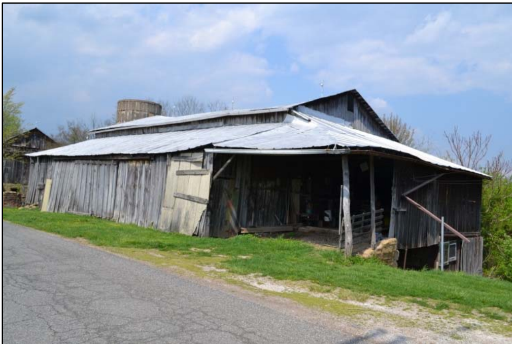
Figure 79 One of two bank barns at WA-0206. This barn has shed additions on the west and south elevations, and a concrete stave silo at the north gable end.
