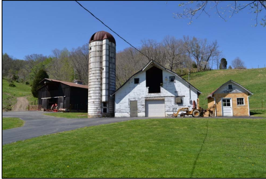
Figure 121 Stock barn, concrete stave silo, dairy barn and milk house at WA-0219.
