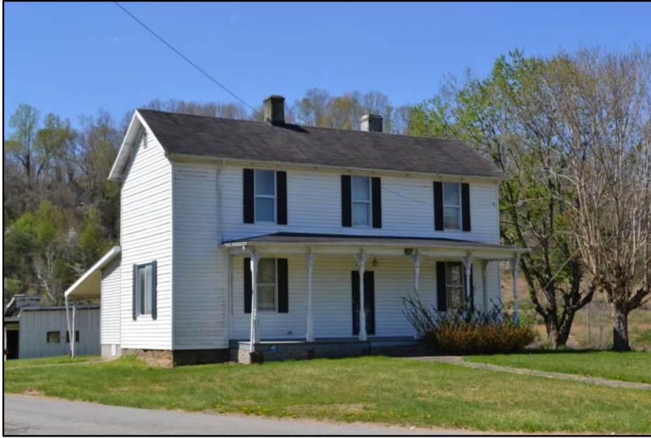
Figure 56 Late-nineteenth century house at WA-0214.
