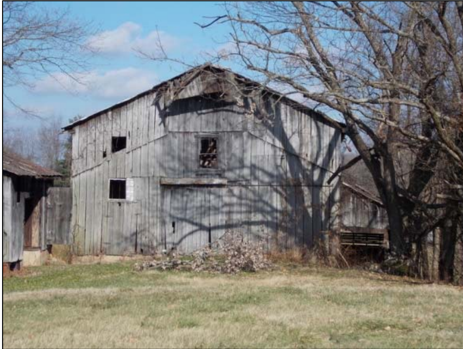
Figure 24 South gable end of barn.
