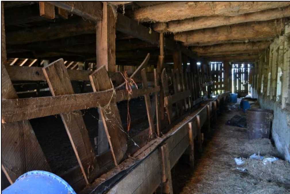
Figure 37 Built-in mangers and hay racks in original central portion of barn.
