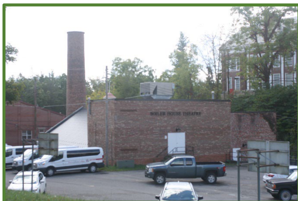
The original boiler room/heating plant for the College (Resource No. 29) has been converted into a theater.
