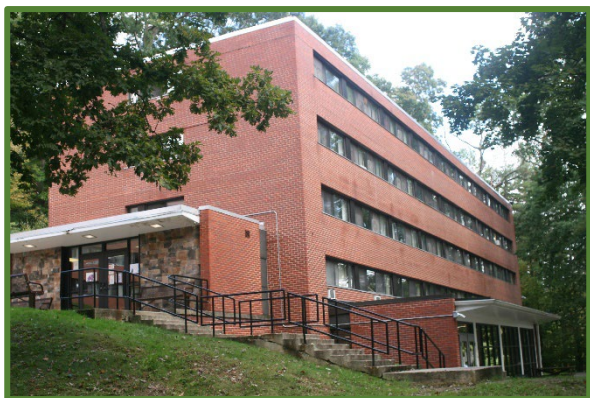
Gribble Residence Hall, built 1958 (Resource No. 17), is the earliest of the various buildings built during the 1950s-1970s expansion of the College.
