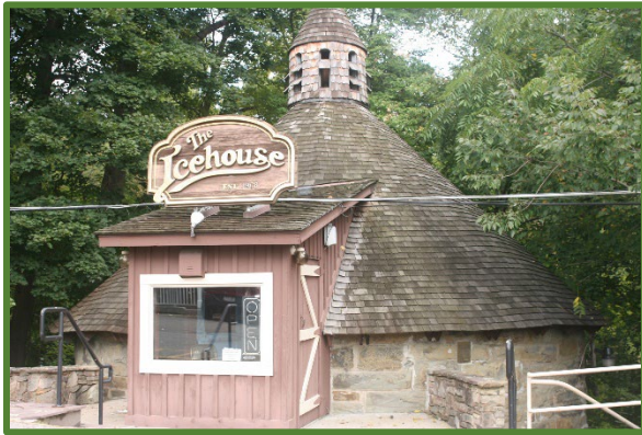
The Icehouse, c. 1890, dates from the pre-College years of the district. The vestibule was a 1967 modification.
