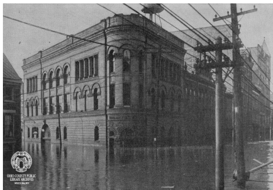
Fig. 6. Riverside Iron Works Building before the 4th story addition, 1913. (Ohio County Public Library)
