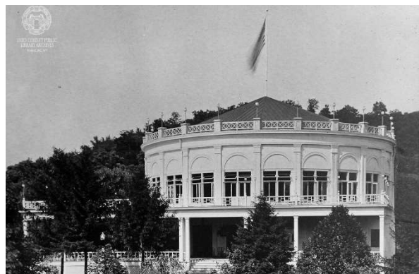
Fig. 3. Wheeling Park Casino, 1905. (Ohio County Public Library)
