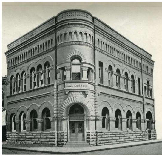
Fig. 9. Merchants' National Bank, Clarksburg, 1911. (West Virginia History On View)
