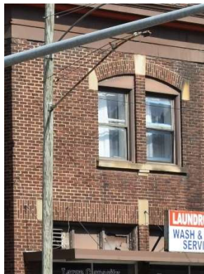
Fig. 13. Detail of lintels at P.F. King Garage, 2019.
