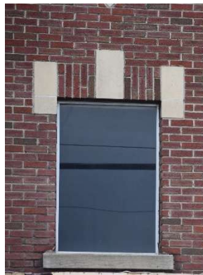
Fig. 14. Detail of lintel at 12th Street Garage, 2019.
