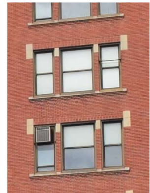
Fig. 16. Detail of lintels at Hawley Building, 2019.
