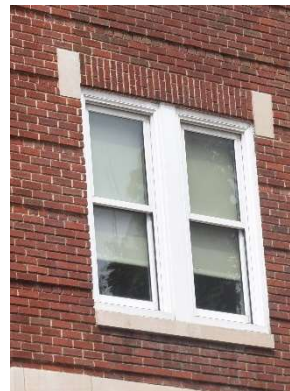
Fig. 15. Detail of lintel at Riley Building, 2019.
