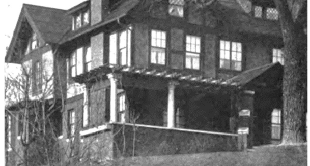
Fig. 26. Detail of Eckhard house with extended pergola porch, c.1912. (Ohio Architect 1912)
