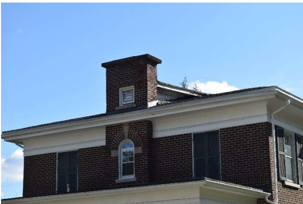
Fig. 29. Detail of window in chimney of the Naylor house, 2019.
