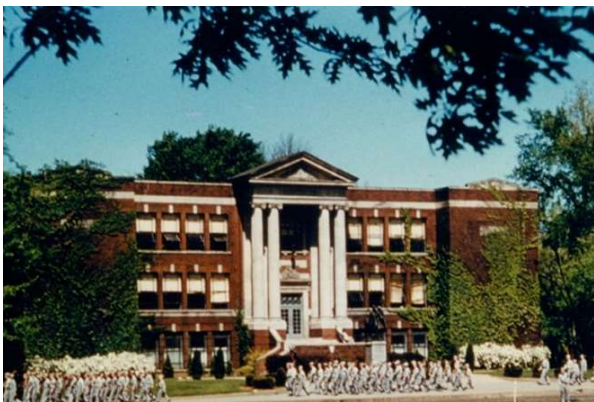
Fig. 9. Linsly Institute, Wheeling, 1958. (Ohio County Public Library)
