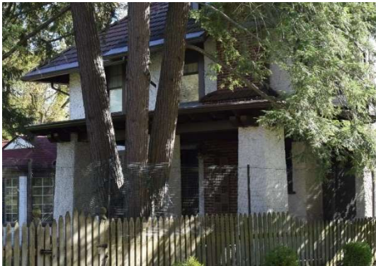
Fig. 27. Detail of battered porch posts at Merriman residence, 2019.
