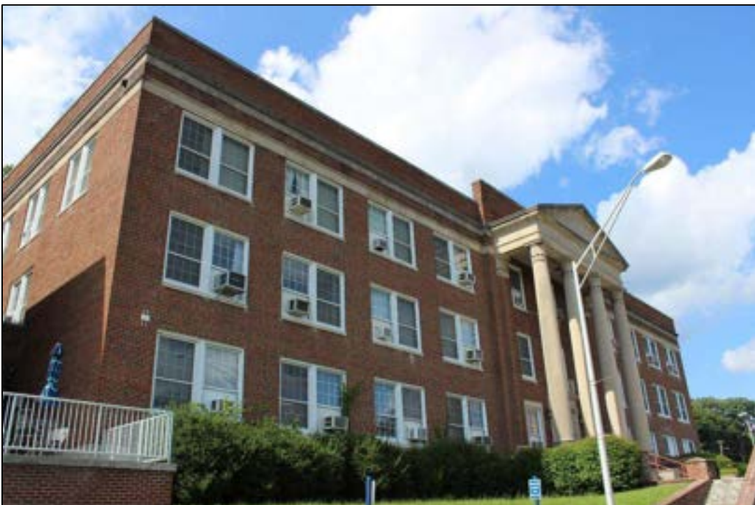
Photograph 2. MC-1892, Conley Hall, Bluefield State College, Facing Northeast.
