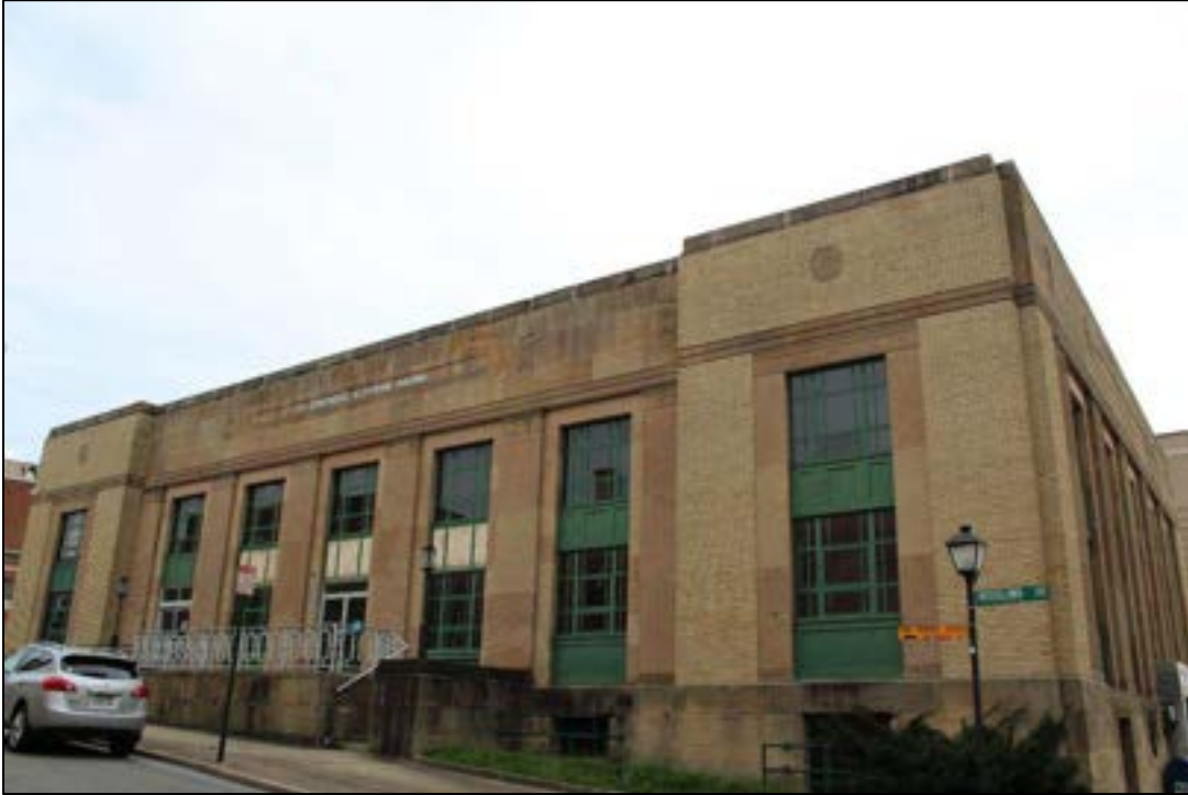
Photograph 1. RG-0014-0074, Post Office, 400 Neville St., Post Office, Facing South.
