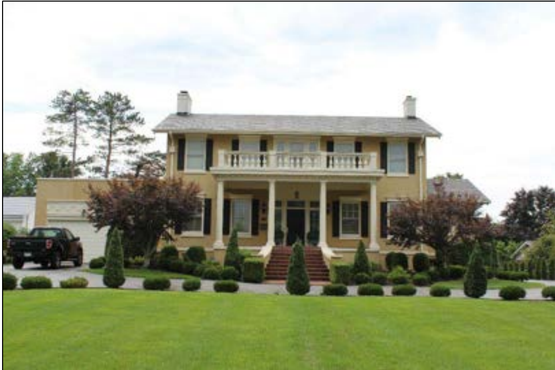
Photograph 1. MC-0882, Toney House, 2116 Reid Ave., Facing Southwest.
