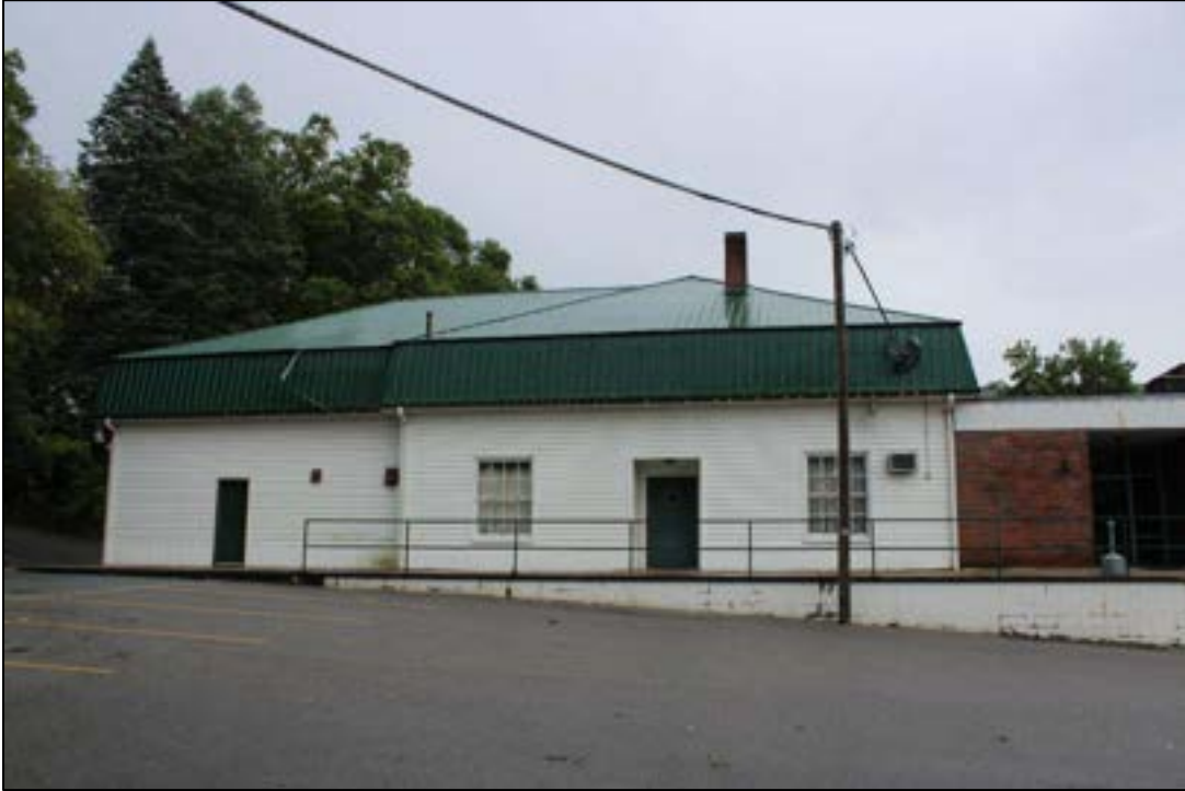
Photograph 1. MC-0869, Bluefield Elks Country Club, 1501 Whitethorn St., Facing Southeast.
