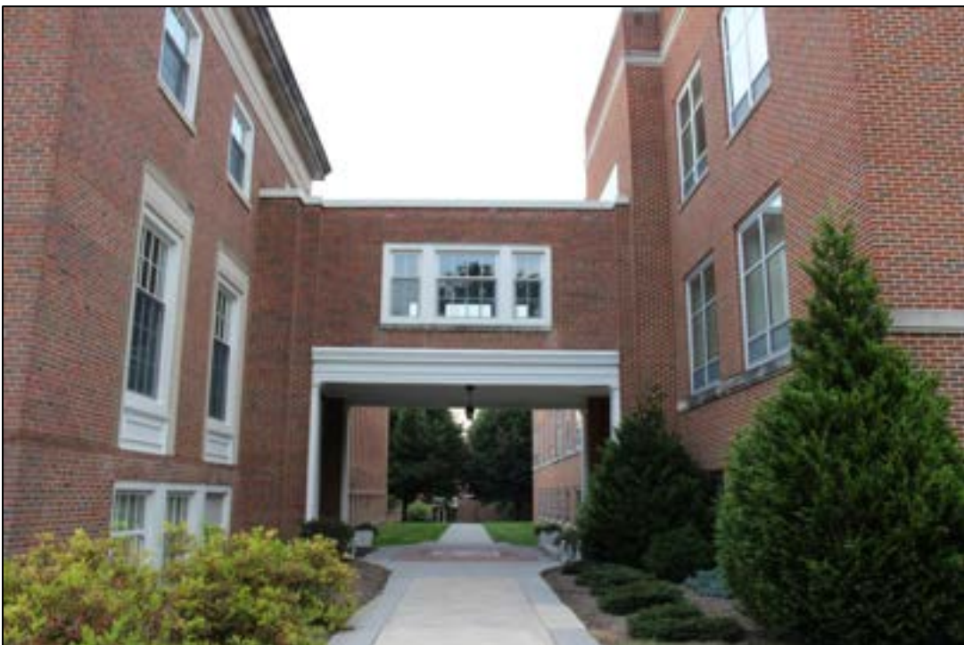
Photograph 4. MC-1968-0001, Concord College Administration Building, Concord College., Facing North.
