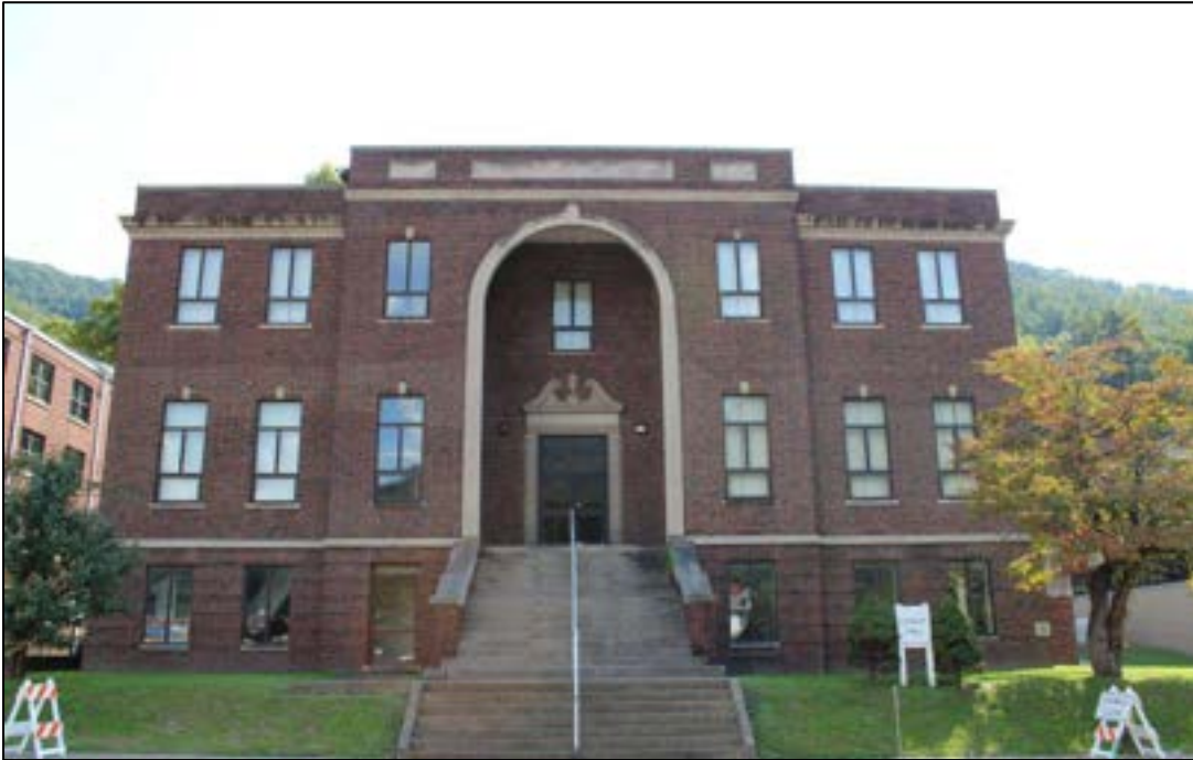
Photograph 1. FA-0006-0031, Conley Hall, S. Adams St., Facing South.
