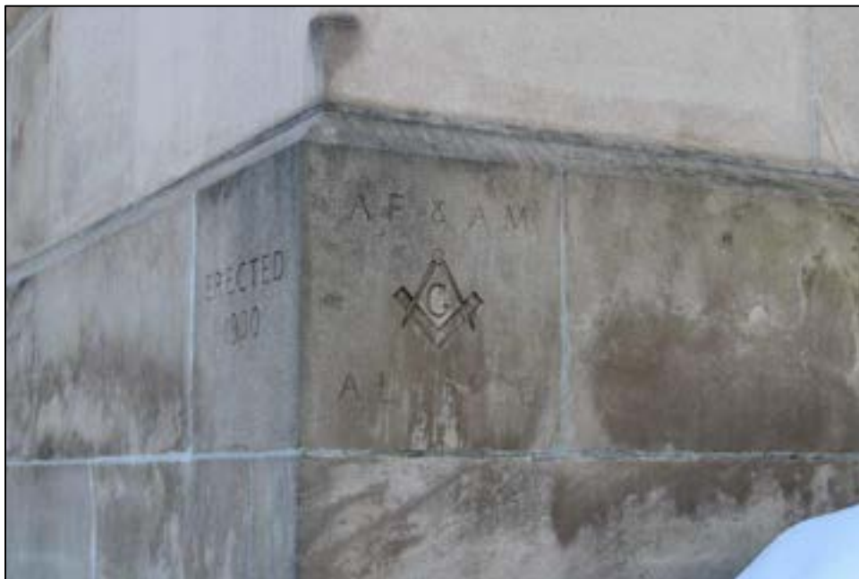
Photograph 6. MC-1969, Mercer County Courthouse, 1501 Main St., Cornerstone Detail.
