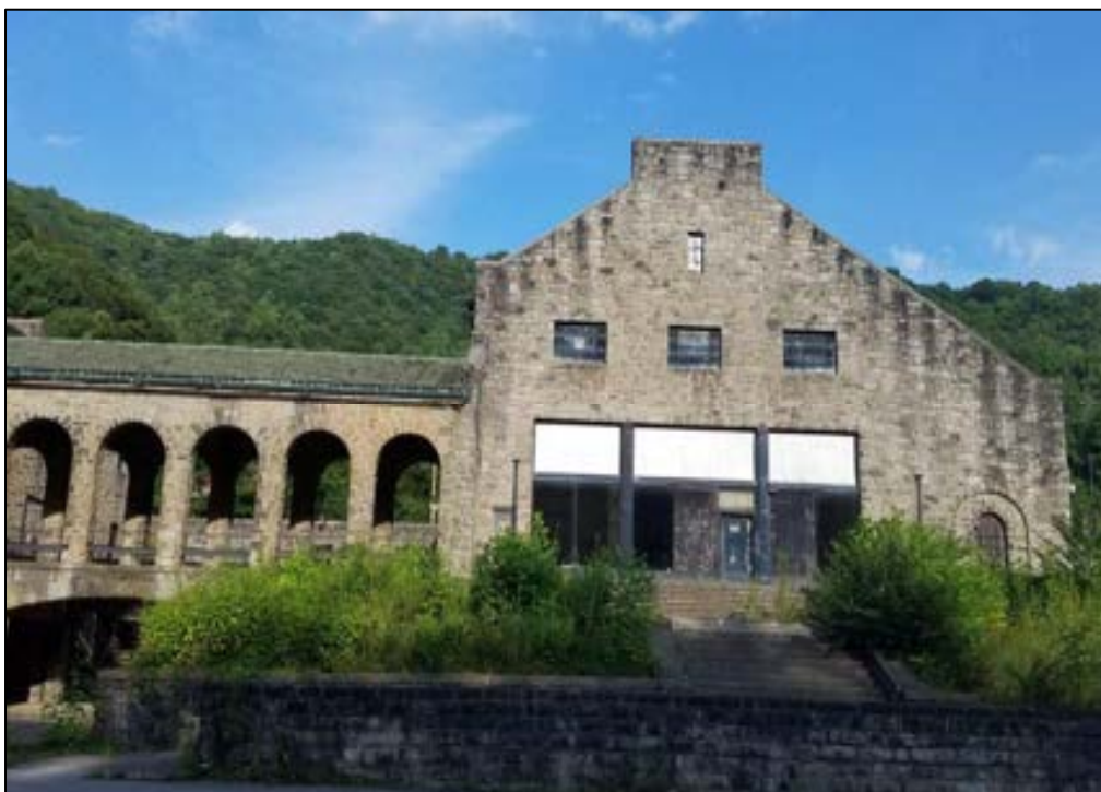
Photograph 4. WM-0001, Itmann Coal Company Store, State Route 10/16, Facing Southeast.
