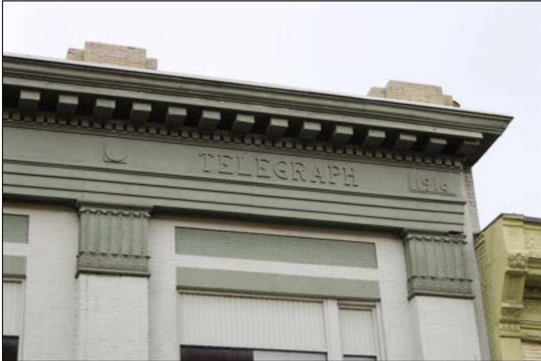
Photograph 3. MC-1170, Bluefield Daily Telegraph, 392 Bland St., Cornice Detail, Facing West.
