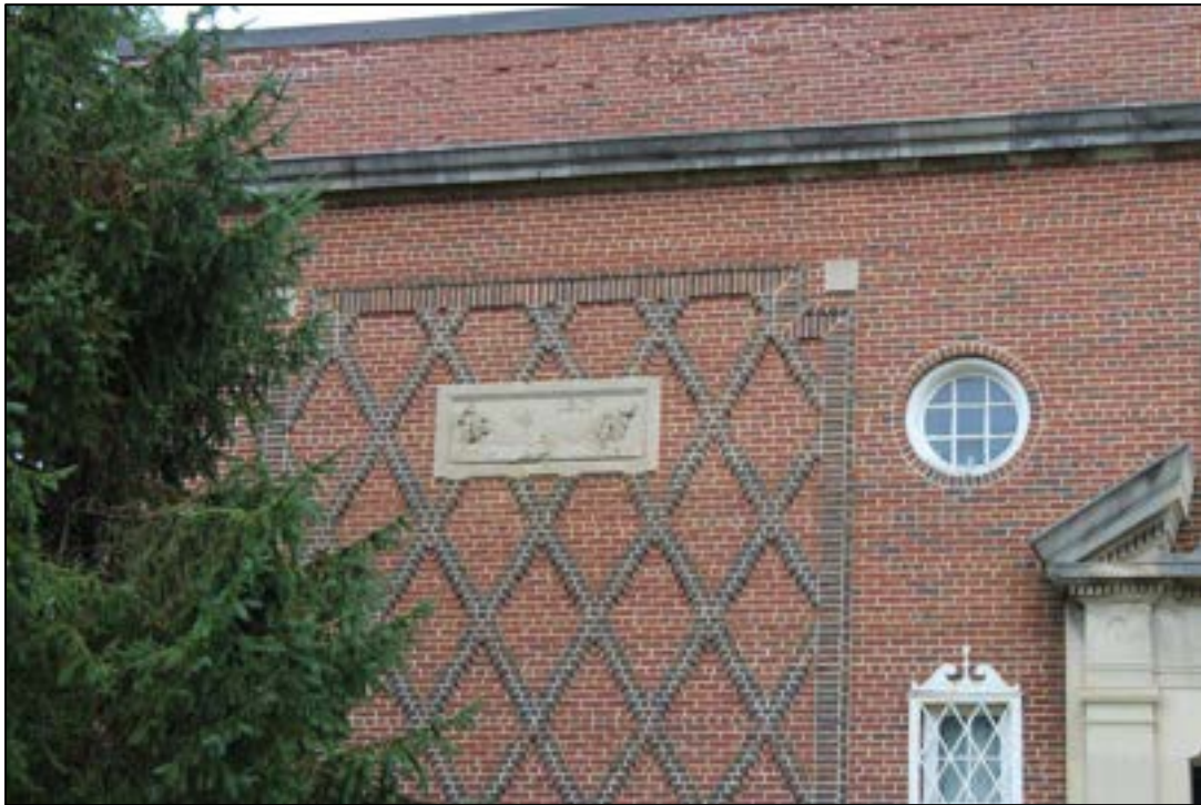
Photograph 5. MC-1967, Memorial School, 319 Memorial Ave., Facade (Southeast Elevation) Detail, Facing Northwest.
