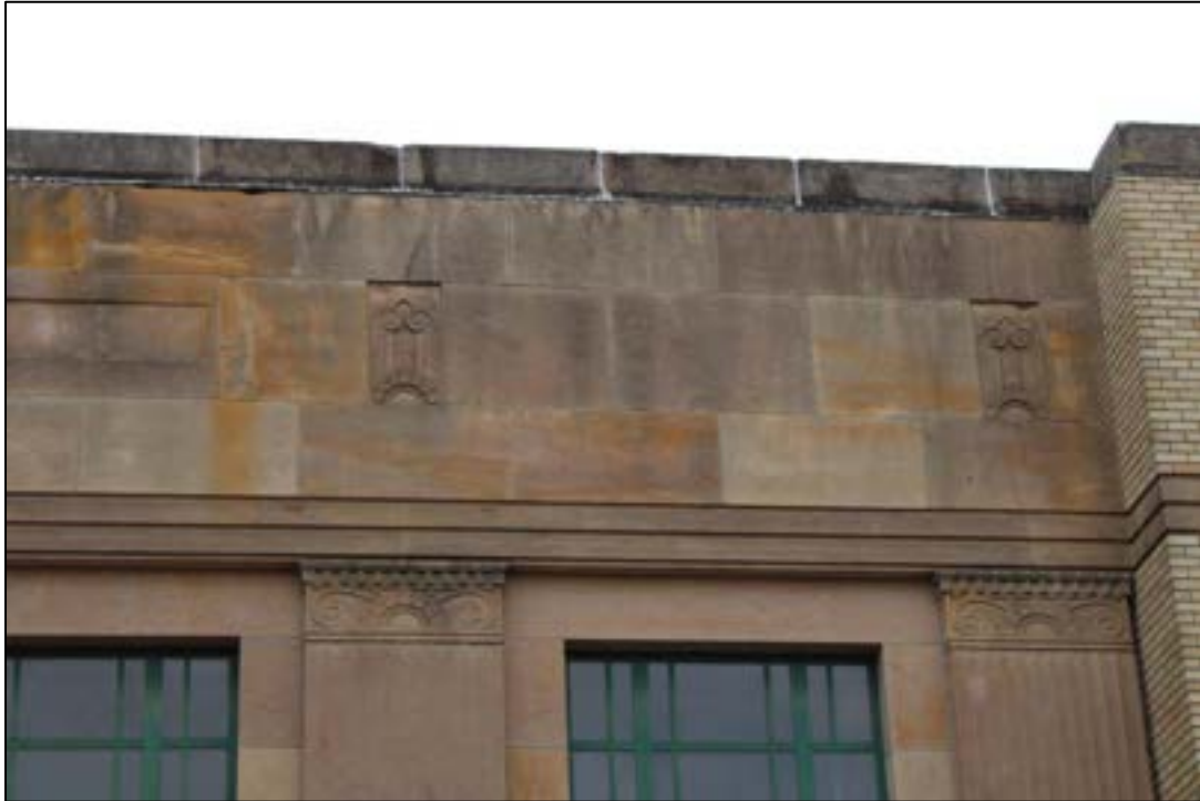
Photograph 5. RG-0014-0074, Post Office, 400 Neville St., Post Office, Facing Southwest.
