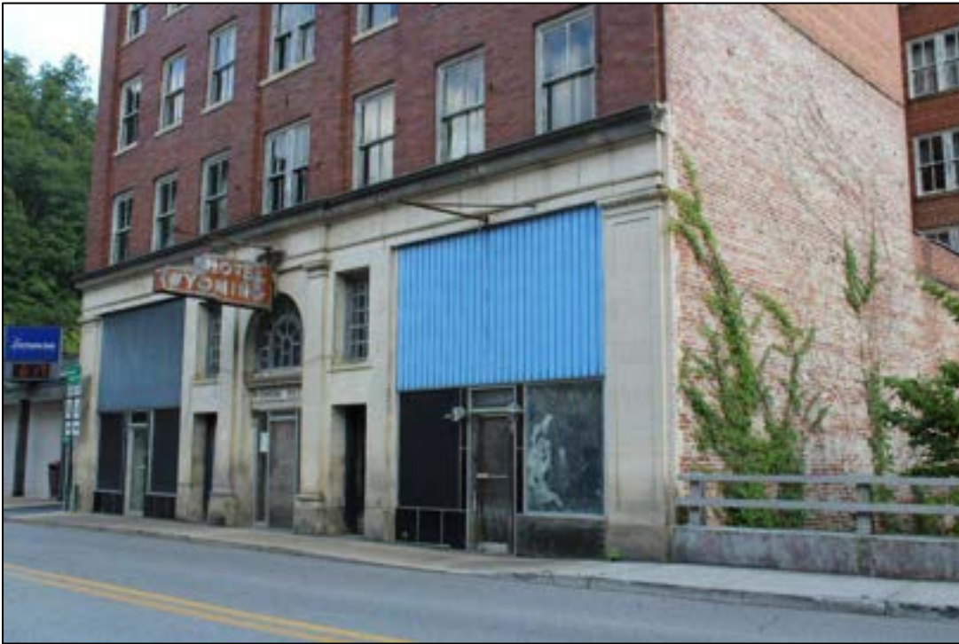
Photograph 4. WM-0337, Hotel Wyoming, First Street, First Floor Detail, Facing Southeast.
