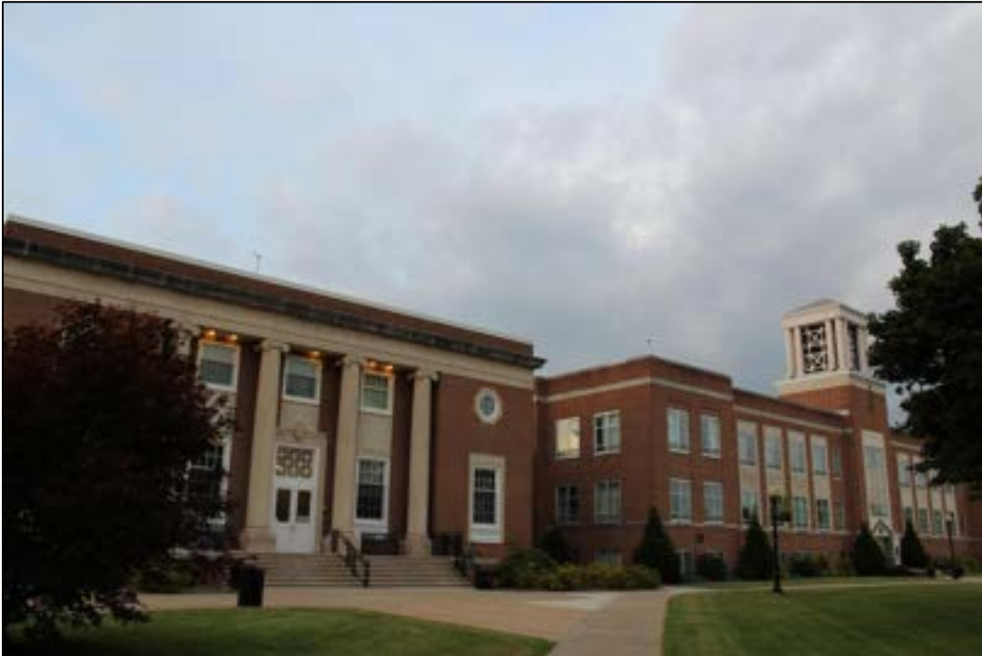
Photograph 3. MC-1968-0001, Concord College Administration Building, Concord College., Facing Northeast.
