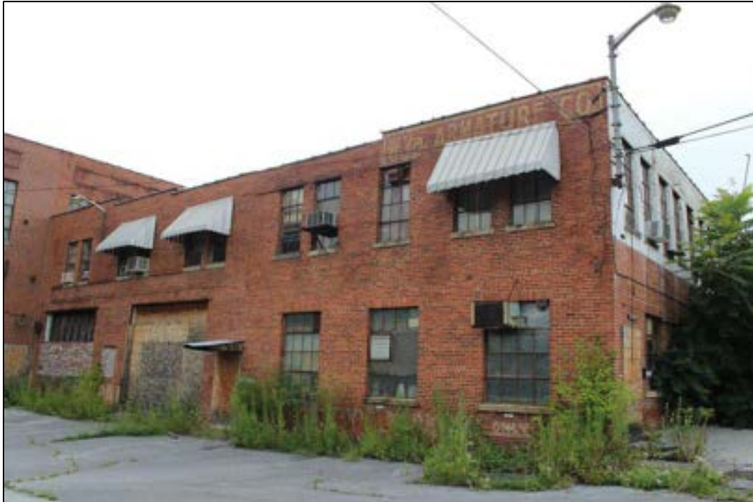
Photograph 1. MC-1962, National Armature and Electric Building, 2 Pine St., Facing North.
