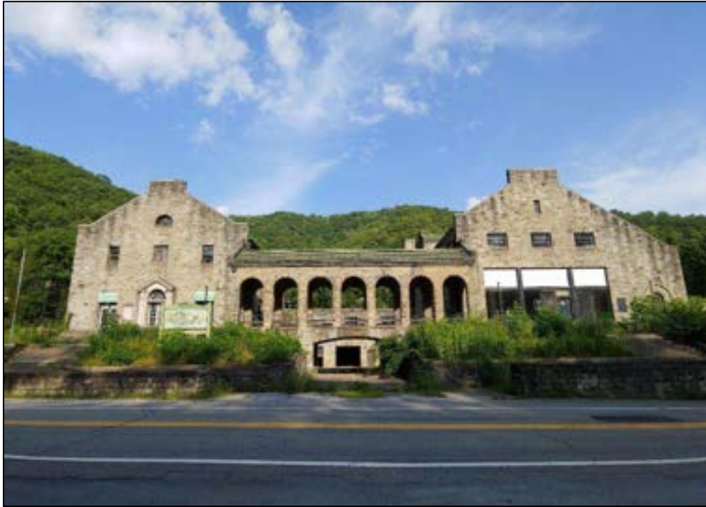
Photograph 1. WM-0001, Itmann Coal Company Store, State Route 10/16, Facing Southeast.
