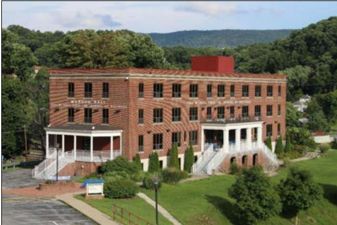
Photograph 1. MC-1894, Mahood Hall, Bluefield State College, Facing East.
