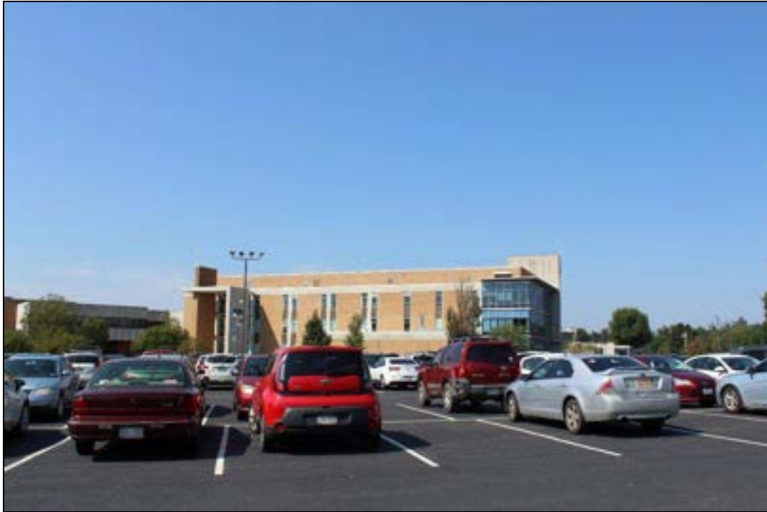
Photograph 3. WD-3257, Main Administration Building, 300 Campus Dr., Facing West.
