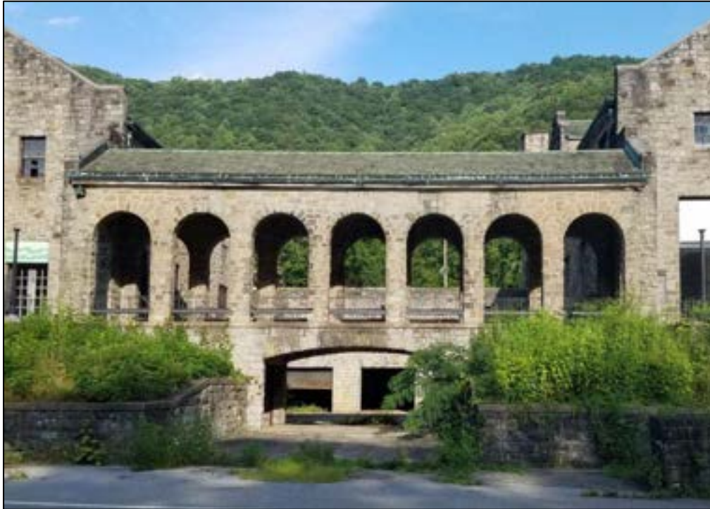
Photograph 3. WM-0001, Itmann Coal Company Store, State Route 10/16, Facing Southeast.
