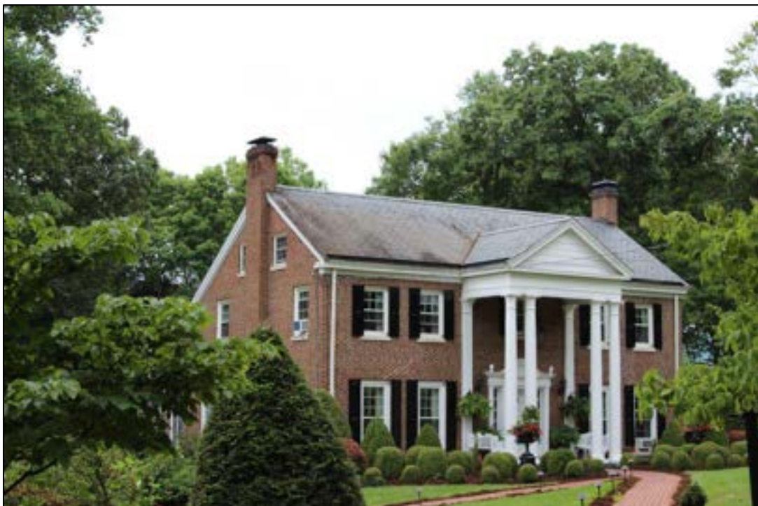
Photograph 2. MC-1097, Kingdon House, 618 Mountain View Ave., Facing Southwest.
