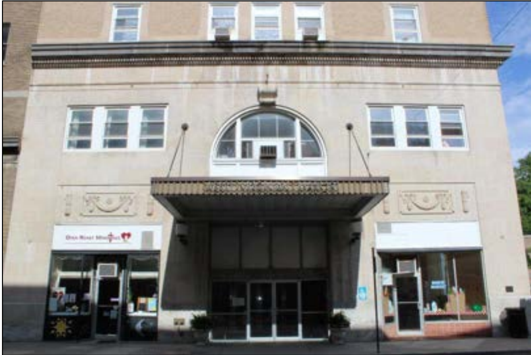
Photograph 3. MC-1189, The West Virginia Hotel, 415 Federal St., Facing East.
