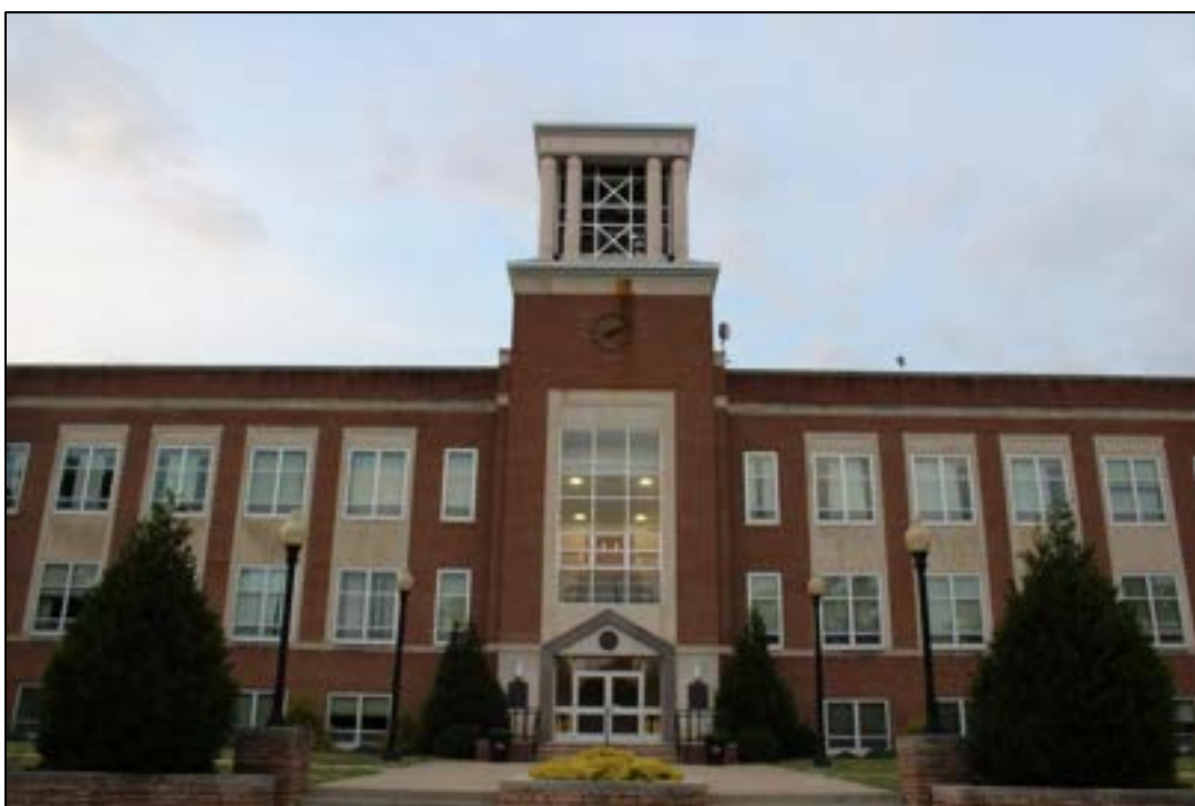
Photograph 2. MC-1968-0001, Concord College Administration Building, Concord College., Facing North.
