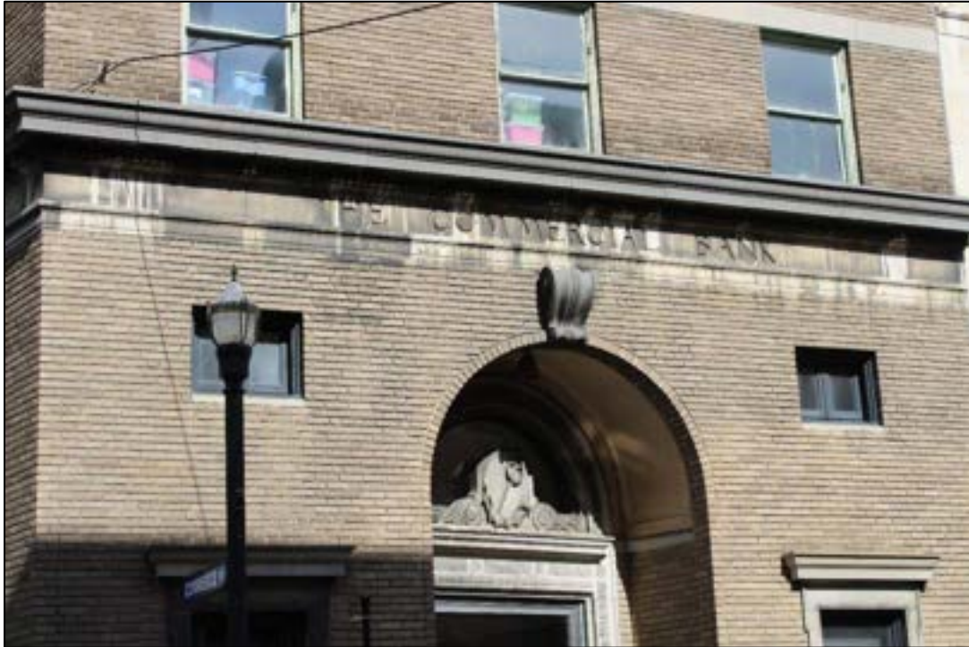
Photograph 3. MC-1190, The Commercial Bank, 401 Federal St., Facing Southeast.
