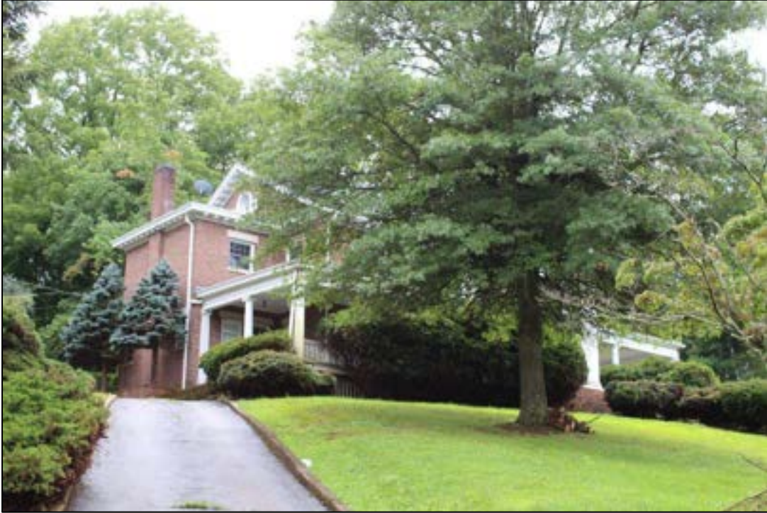
Photograph 3. MC-1964, Garrett House, 109 Spring Grove Ave., Facing South.
