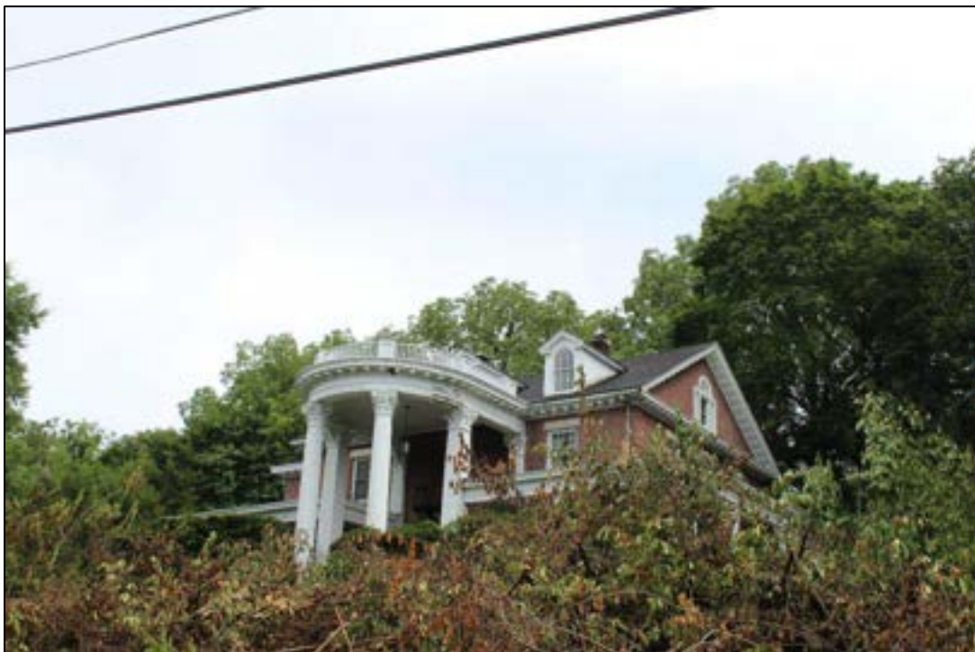
Photograph 2. MC-1964, Garrett House, 109 Spring Grove Ave., Facing Southeast.
