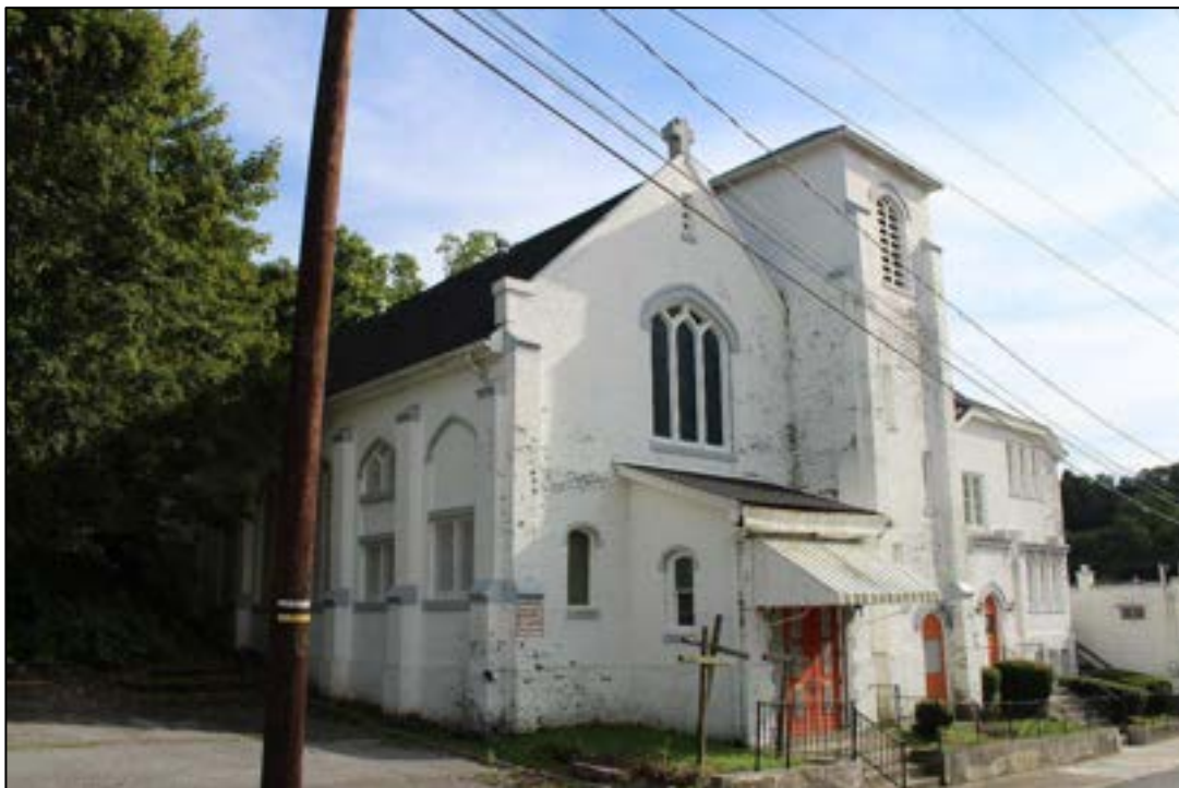
Photograph 2 MC-1215, John Stewart United Methodist Church, 102 Jones Street, Church, Facing Southwest.
