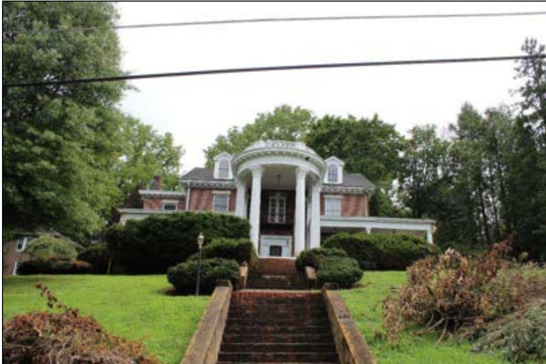
Photograph 1. MC-1964, Garrett House, 109 Spring Grove Ave., Facing Southeast.
