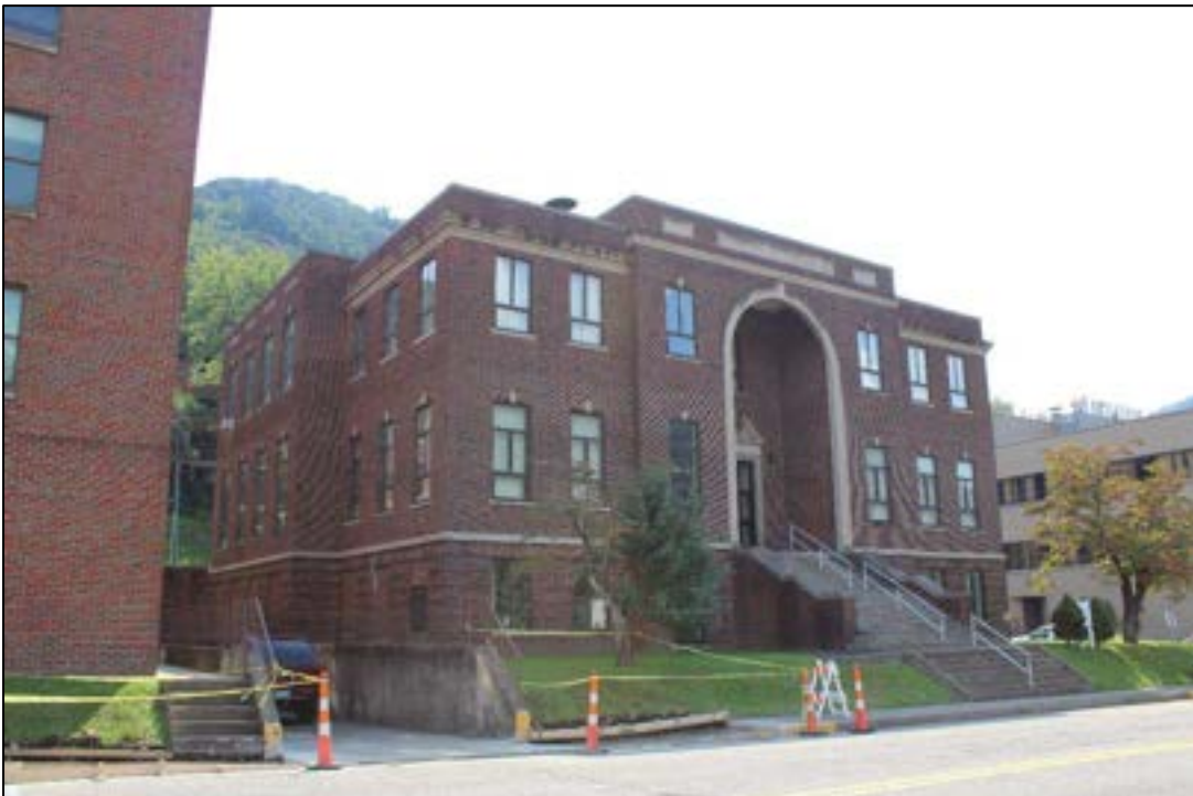
Photograph 2. FA-0006-0031, Conley Hall, S. Adams St., Facing Southwest.
