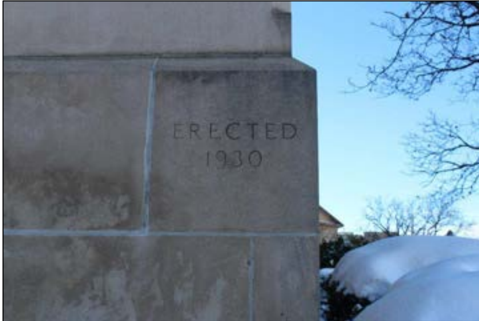
Photograph 5. MC-1969, Mercer County Courthouse, 1501 Main St., Cornerstone Detail.
