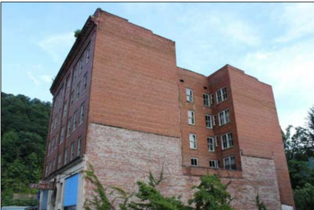
Photograph 3. WM-0337, Hotel Wyoming, First Street, Hotel, Facing Southeast.
