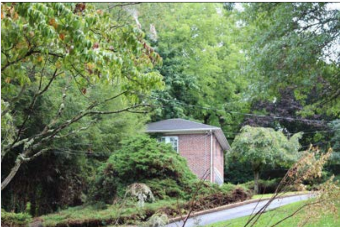
Photograph 4. MC-1964, Garrett House, 109 Spring Grove Ave., Facing Southeast.
