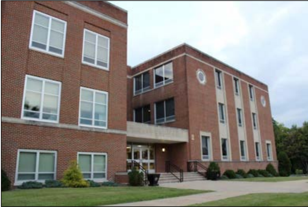
Photograph 5. MC-1968-0001, Concord College Administration Building, Concord College., Facing Northeast.
