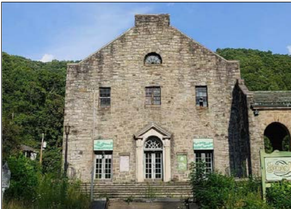
Photograph 2. WM-0001, Itmann Coal Company Store, State Route 10/16, Facing Southeast.
