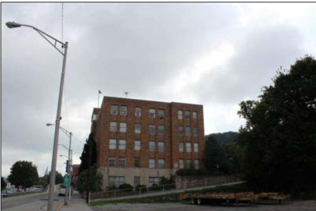
Photograph 2. MC-1142, Norfolk & Western Railroad Building, 800 Princeton Ave., Facing East.
