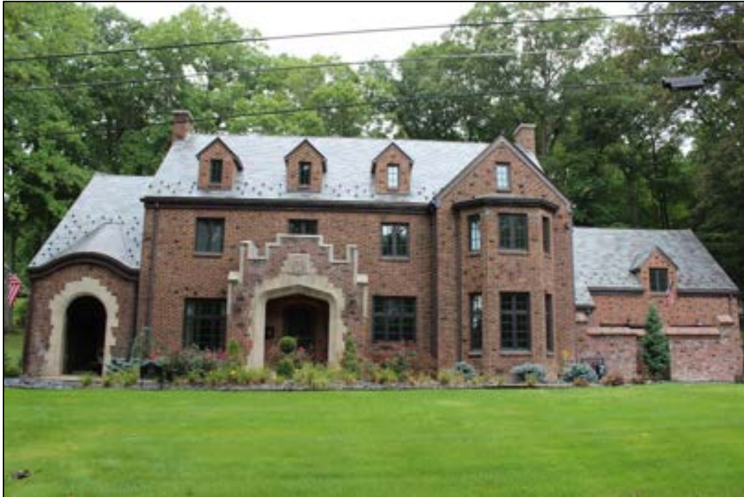
Photograph 1. MC-1015, Cooper House, 909 Edgewood Rd., Facing Northwest.
