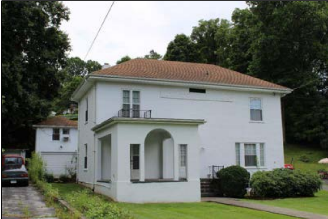
Photograph 1. MC-1091, Mahood House, 2306 Bland Rd., Facing Southwest.
