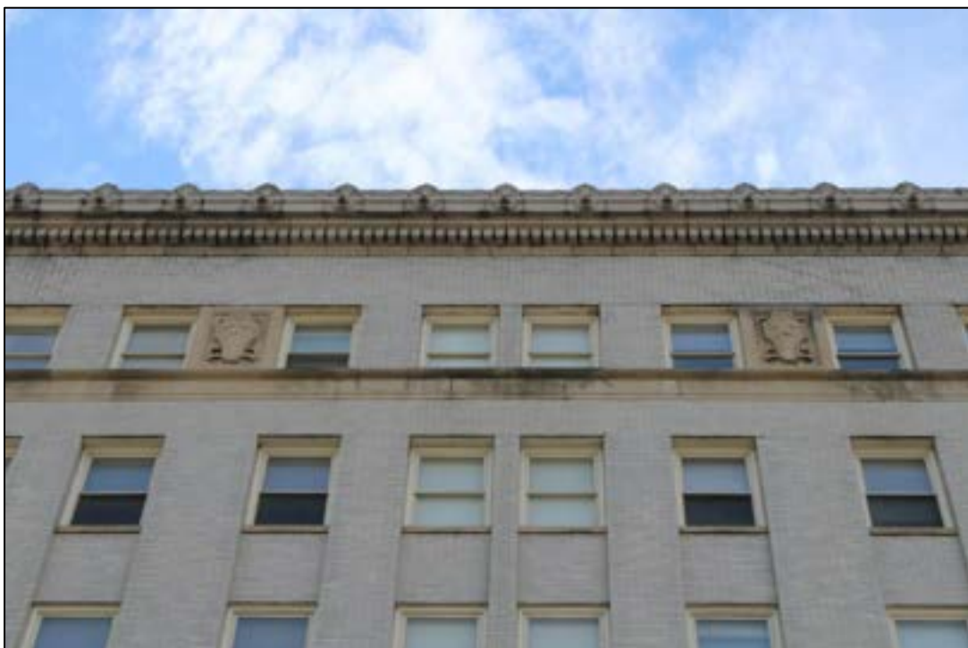
Photograph 4. MC-1174, Perry Building, 525 Bland St., Facing Northeast.
