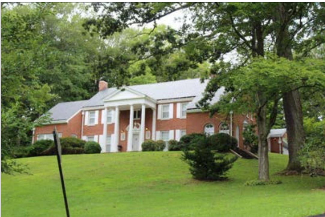
Photograph 2. MC-1966, Kingdon House, 625 Mountain View Ave., Facing Northwest.
