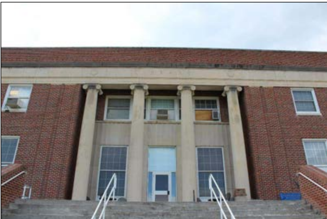
Photograph 2. MC-1893, Wendell G. Hardway Library, Bluefield State College, Facing Northwest.
