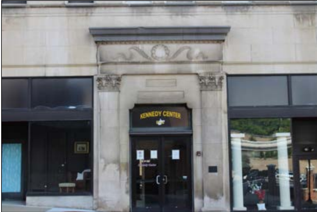
Photograph 3. MC-1174, Perry Building, 525 Bland St., Facing Northeast.
