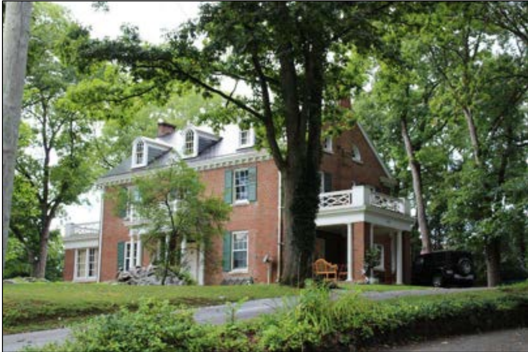
Photograph 3. MC-0870, Farquarson House, 1420 Lebanon St., Facing Northwest.
