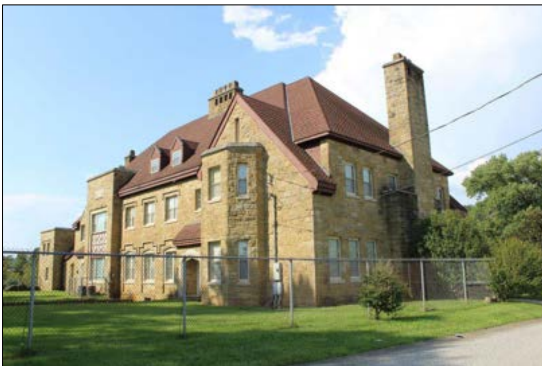
Photograph 4. CB-2758, Prichard School, 2619 Raceview Drive, Primary Dwelling, Facing Northwest.
