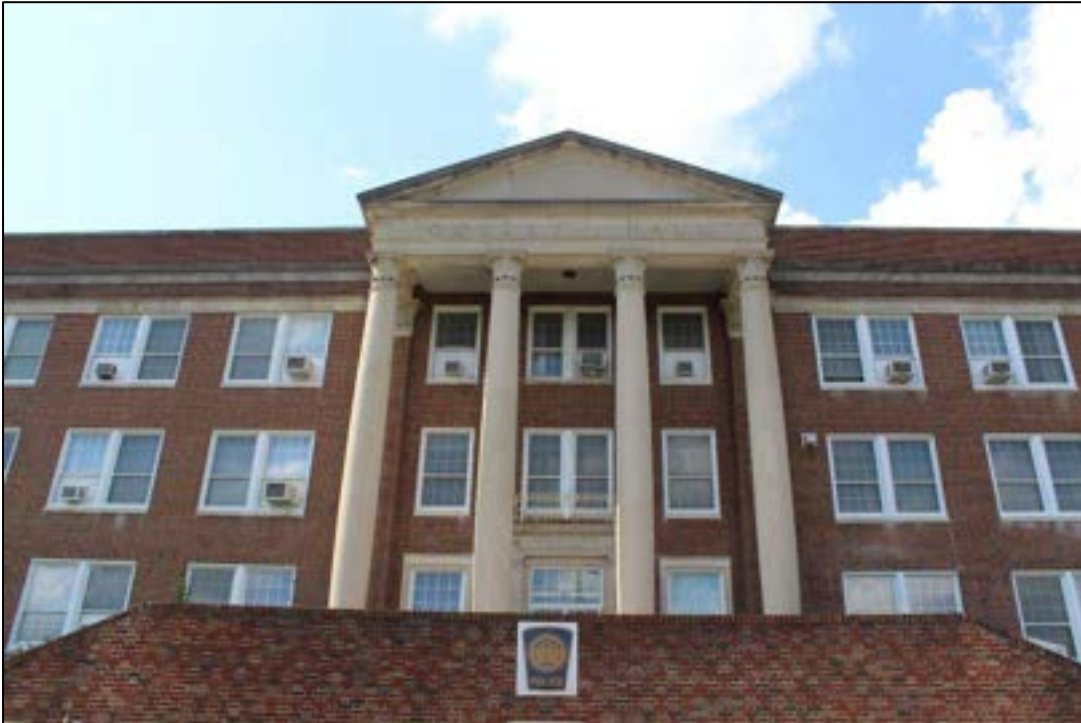
Photograph 1. MC-1892, Conley Hall, Bluefield State College, Facing Northwest.
