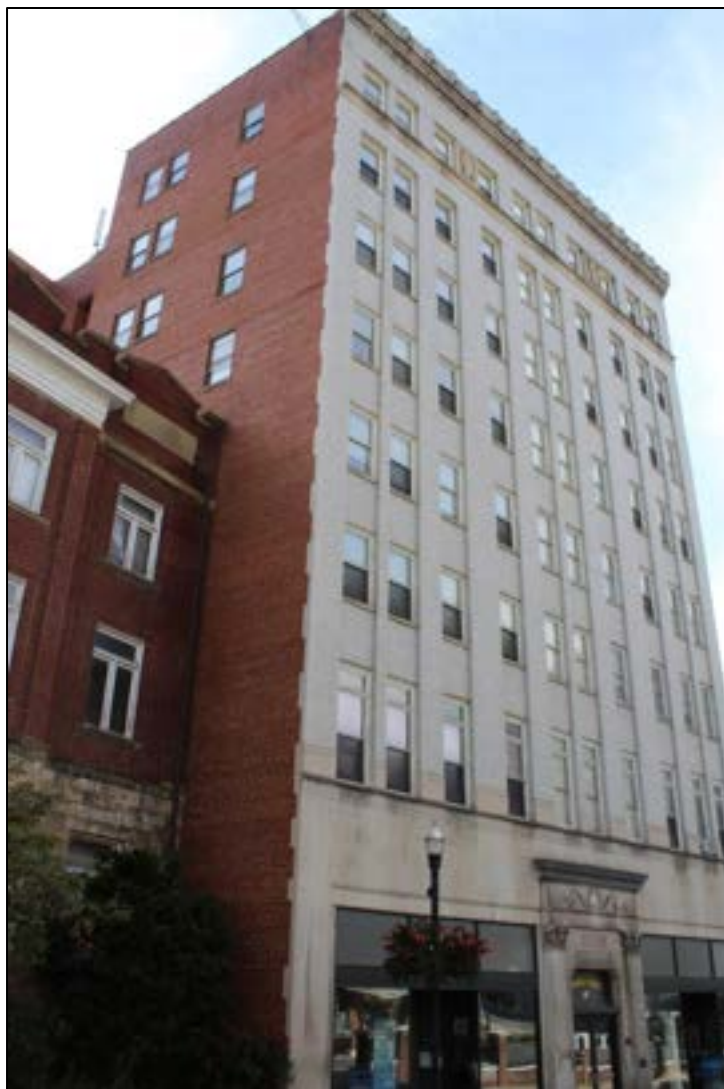
Photograph 2. MC-1174, Perry Building, 525 Bland St., Facing Southeast.
