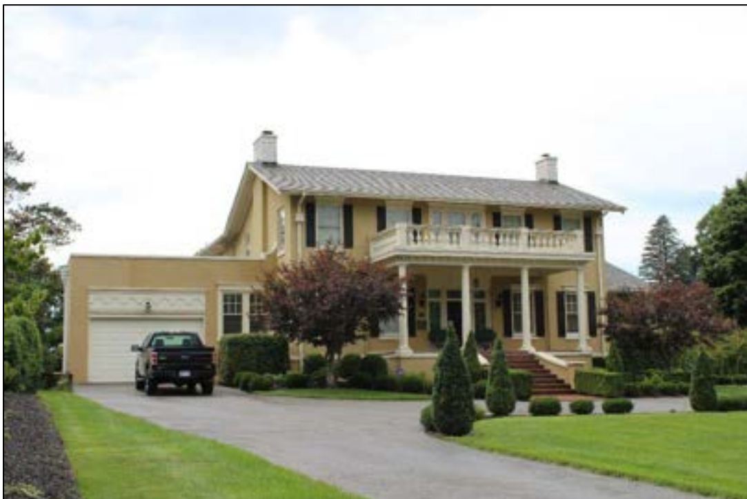
Photograph 2. MC-0882, Toney House, 2116 Reid Ave., Facing West.
