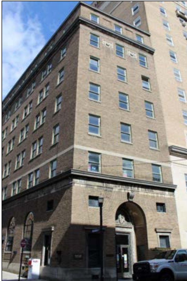
Photograph 2. MC-1190, The Commercial Bank, 401 Federal St., Facing Southeast.
