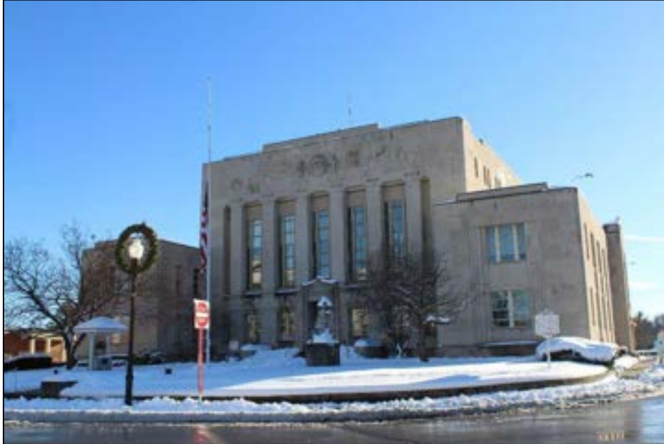
Photograph 3. MC-1969, Mercer County Courthouse, 1501 Main St., Facing Northwest.
