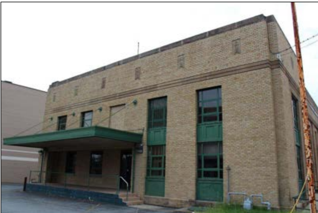
Photograph 4. RG-0014-0074, Post Office, 400 Neville St., Post Office, Facing West.
