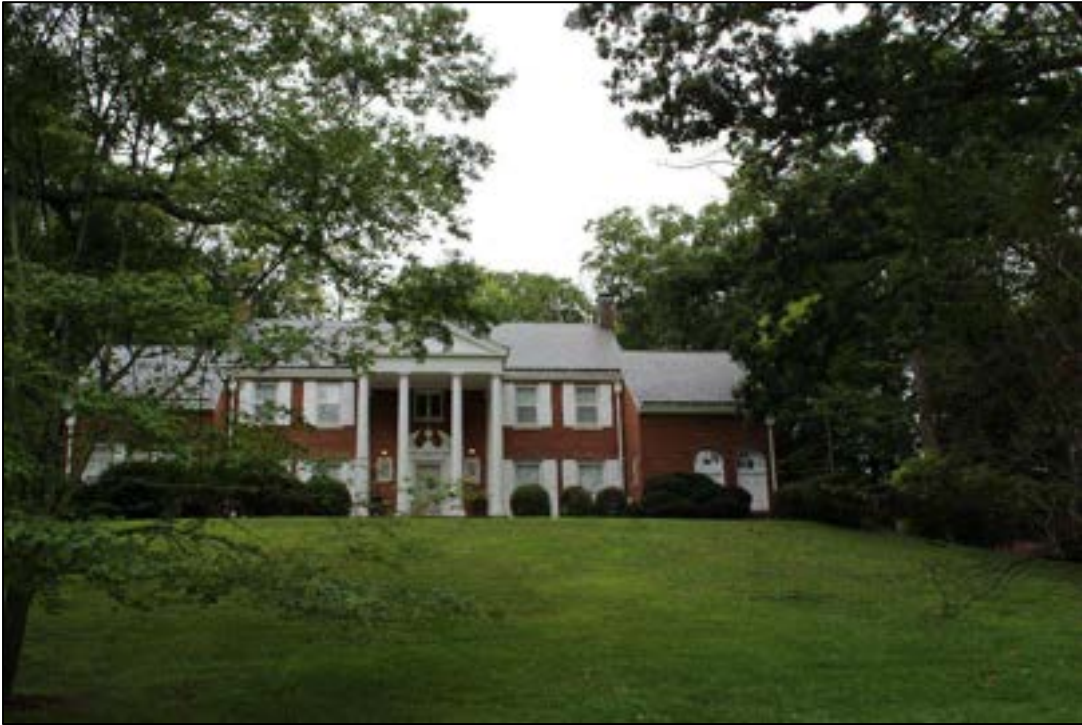
Photograph 1. MC-1966, Kingdon House, 625 Mountain View Ave., Facing Northwest.
