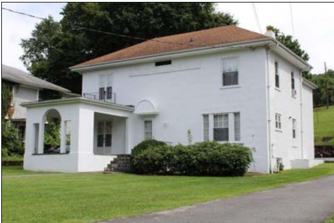
Photograph 2. MC-1091, Mahood House, 2306 Bland Rd., Facing Southeast.
