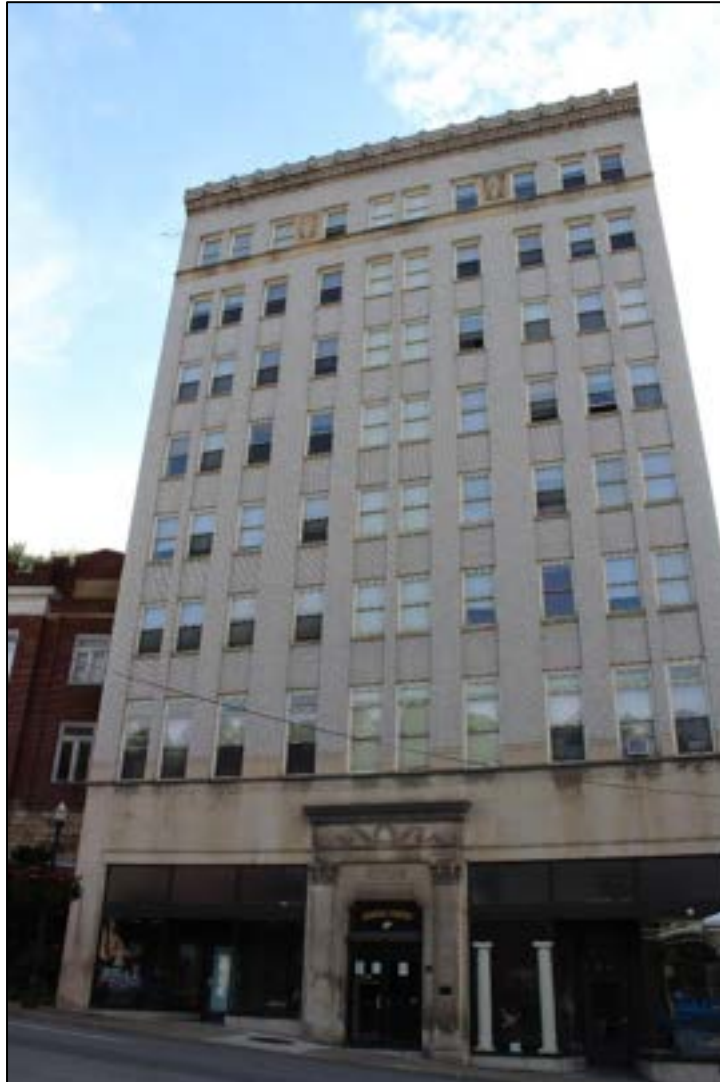
Photograph 1. MC-1174, Perry Building, 525 Bland St., Facing Northeast.
