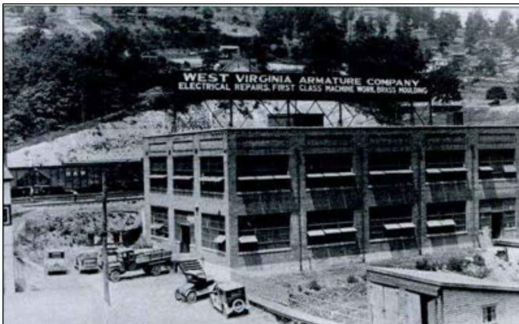
Figure 1. MC-1962, National Armature and Electric Building, Historic Photograph c.1930s. Source: Frank Davis from William Archer's "Bluefield in the 1940s", Arcadia Publishing, 2009.
