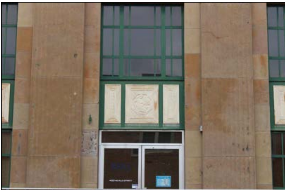
Photograph 6. RG-0014-0074, Post Office, 400 Neville St., Post Office, Facing Southwest.
