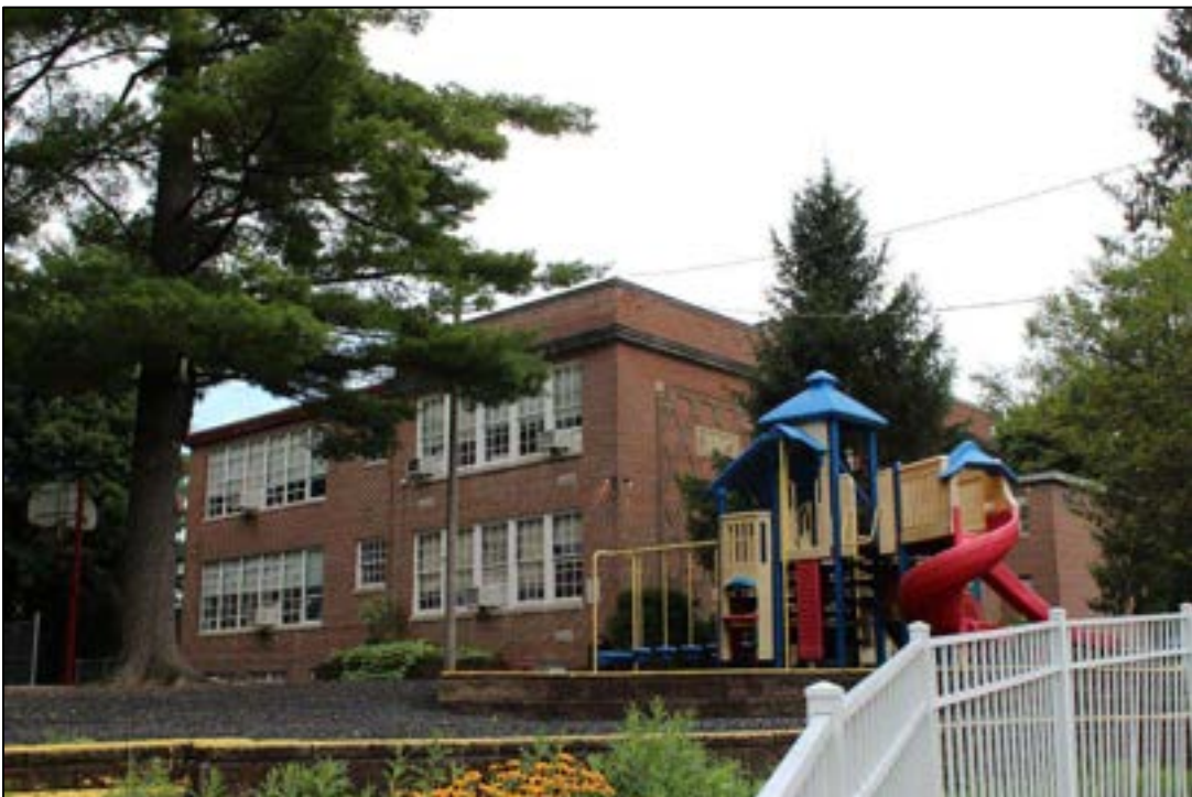
Photograph 4. MC-1967, Memorial School, 319 Memorial Ave., Facing Northeast.
