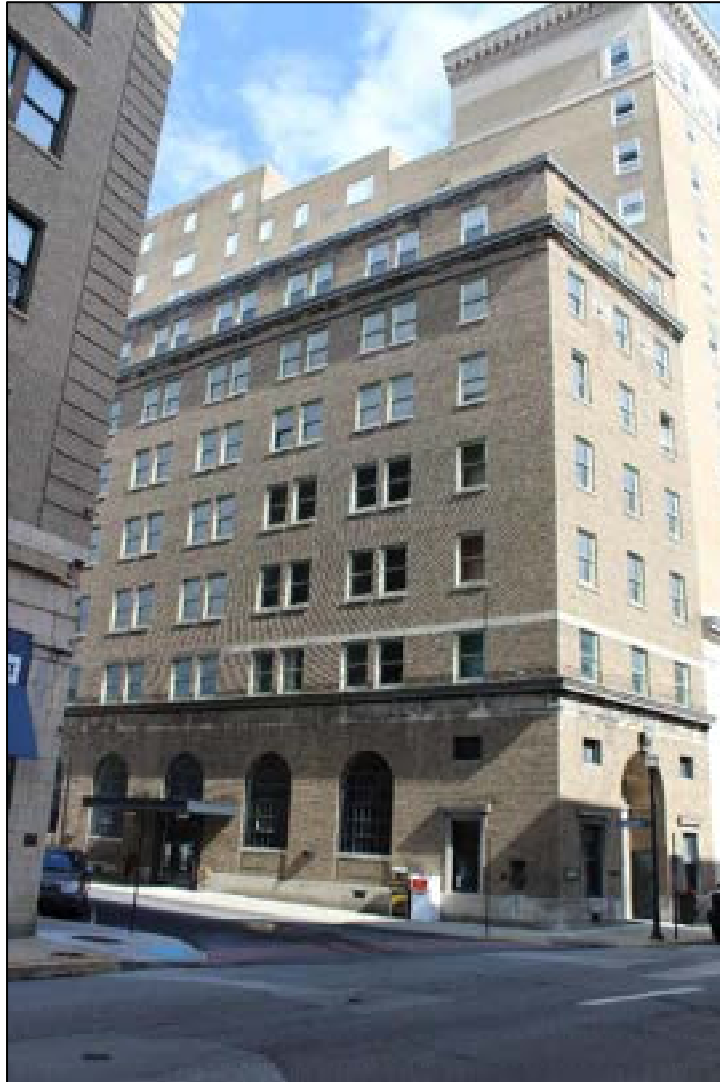
Photograph 1. MC-1190, The Commercial Bank, 401 Federal St., Facing Southeast.
