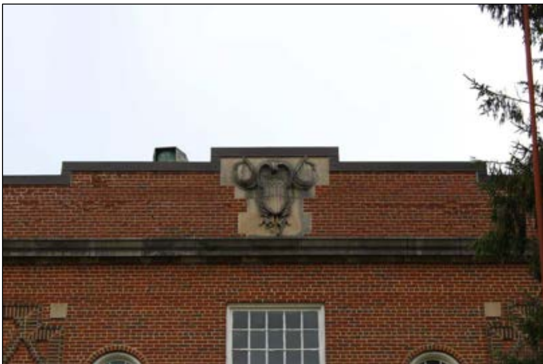
Photograph 6. MC-1967, Memorial School, 319 Memorial Ave., Facade (Southeast Elevation) Detail, Facing Northwest.
