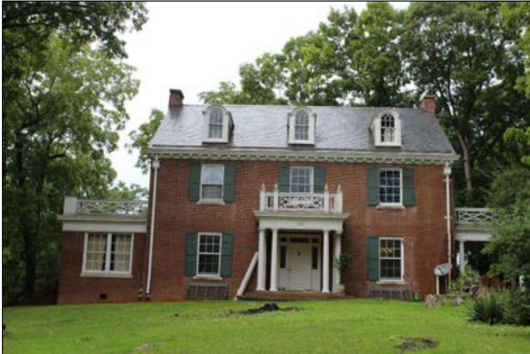
Photograph 1. MC-0870, Farquarson House, 1420 Lebanon St., Facing Northwest.
