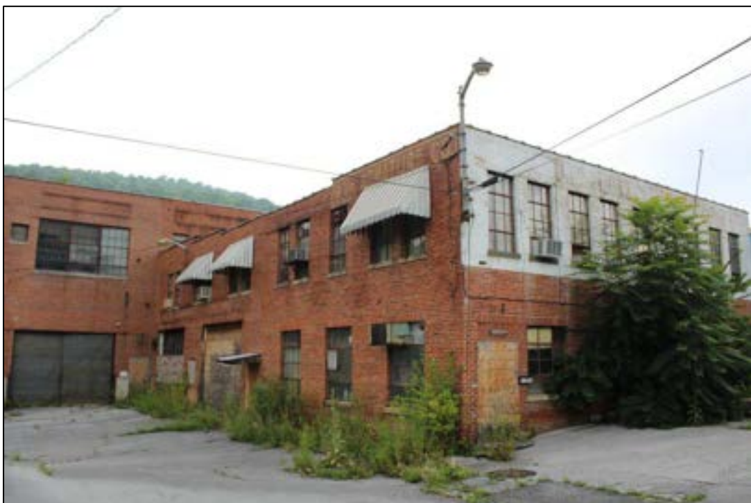
Photograph 2. MC-1962, National Armature and Electric Building, 2 Pine St., Facing Northwest.
