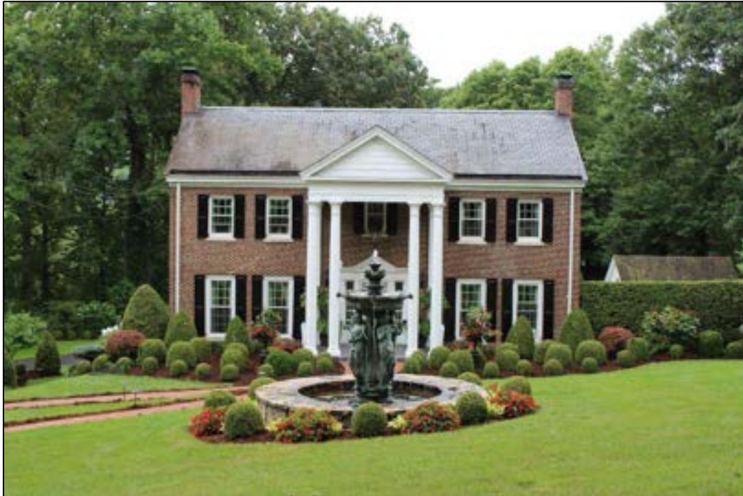
Photograph 1. MC-1097, Kingdon House, 618 Mountain View Ave., Facing South.
