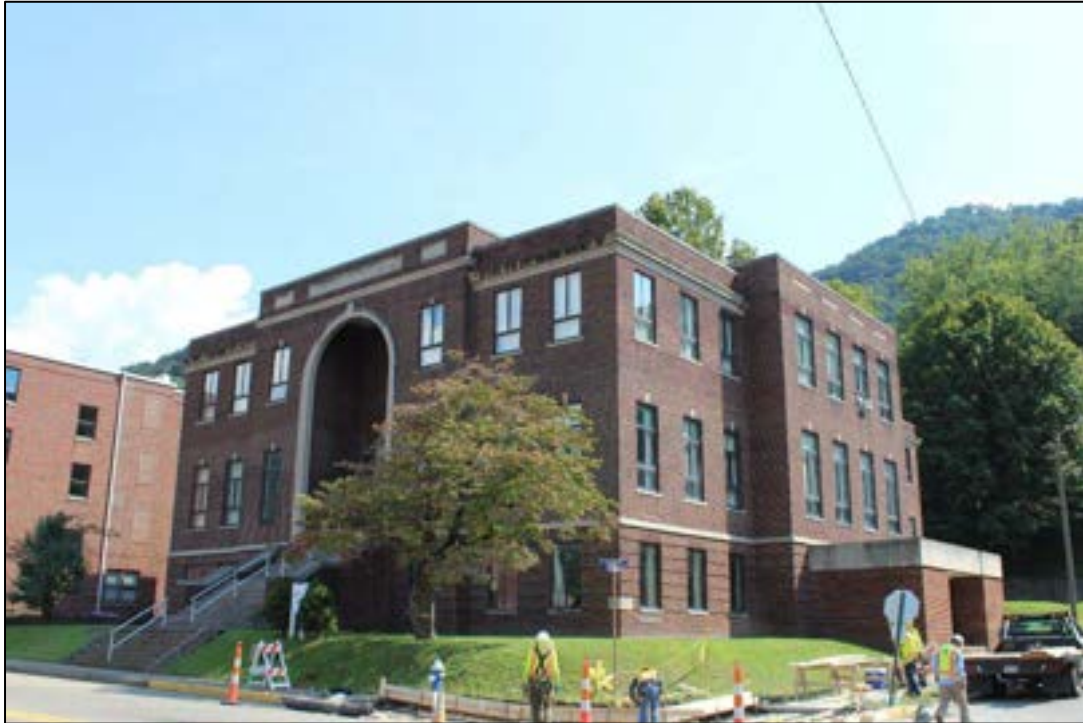
Photograph 3. FA-0006-0031, Conley Hall, S. Adams St., Facing Southeast.
