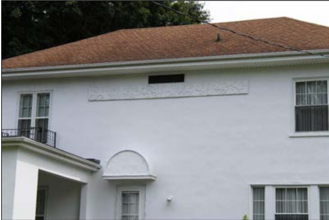
Photograph 3. MC-1091, Mahood House, 2306 Bland Rd., Facing Southeast.
