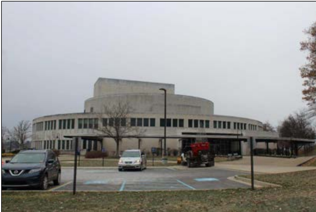
Photograph 1. MG-1259, Creative Arts Center, 1 Fine Arts Dr., Facing Northeast.
