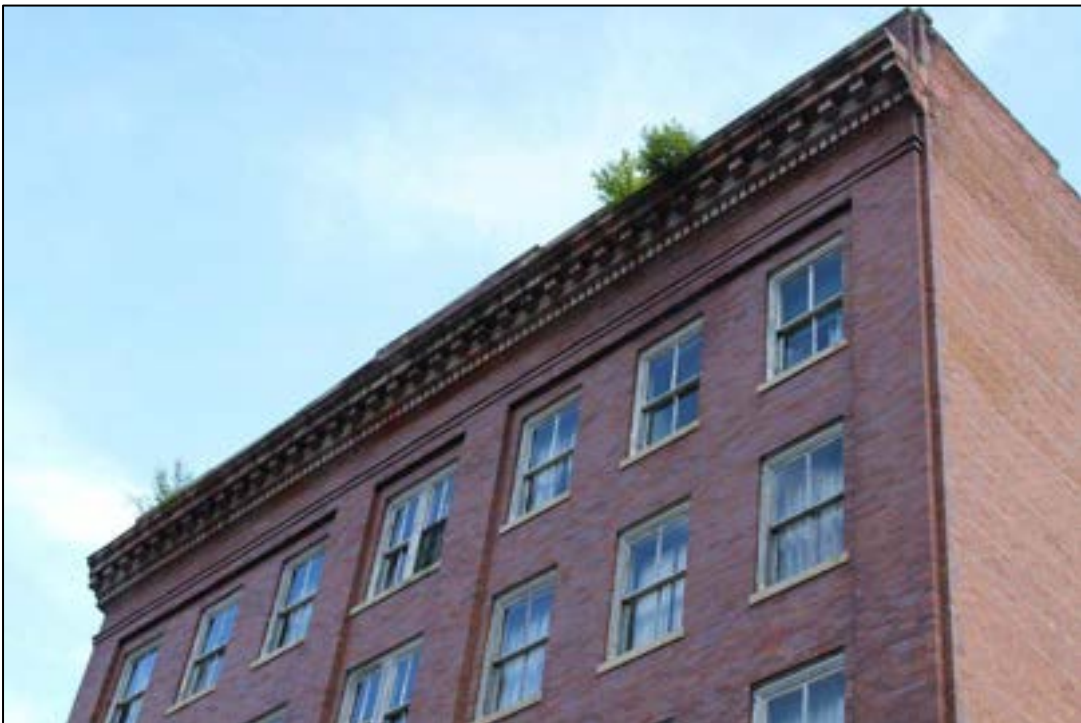
Photograph 5. WM-0337, Hotel Wyoming, First Street, Cornice Detail, Facing Southeast.
