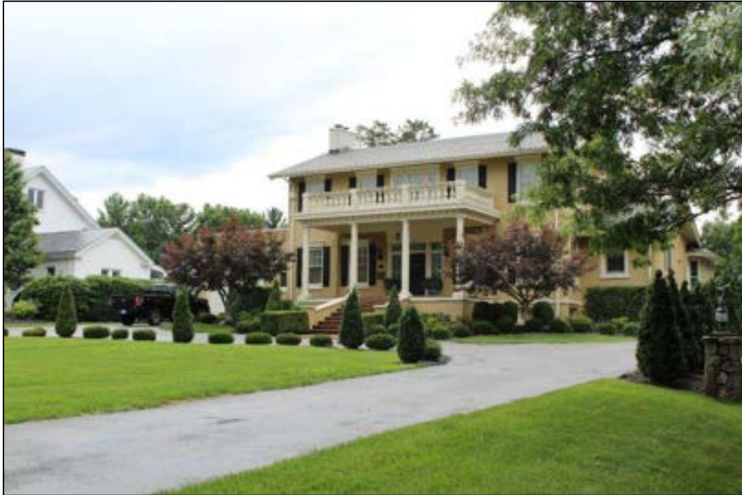
Photograph 3. MC-0882, Toney House, 2116 Reid Ave., Facing Southwest.
