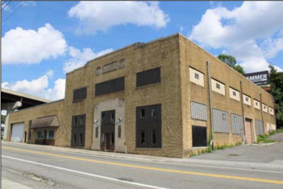
Photograph 1. MC-1303, Coca-Cola Manufacturing Building, 1217 Bluefield Avenue, Facing East.
