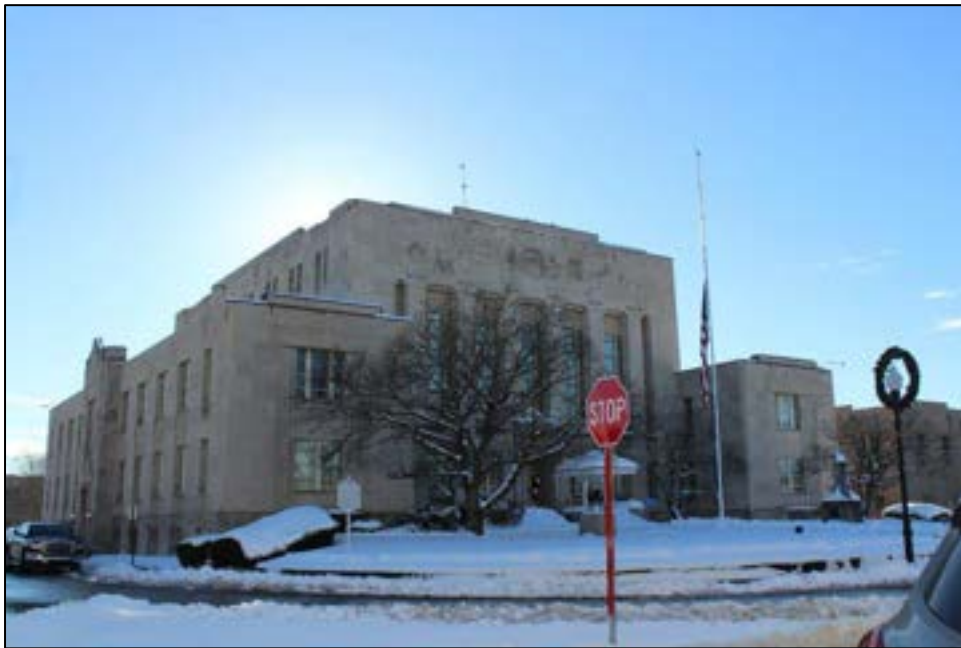
Photograph 2. MC-1969, Mercer County Courthouse, 1501 Main St., Facing Northeast.
