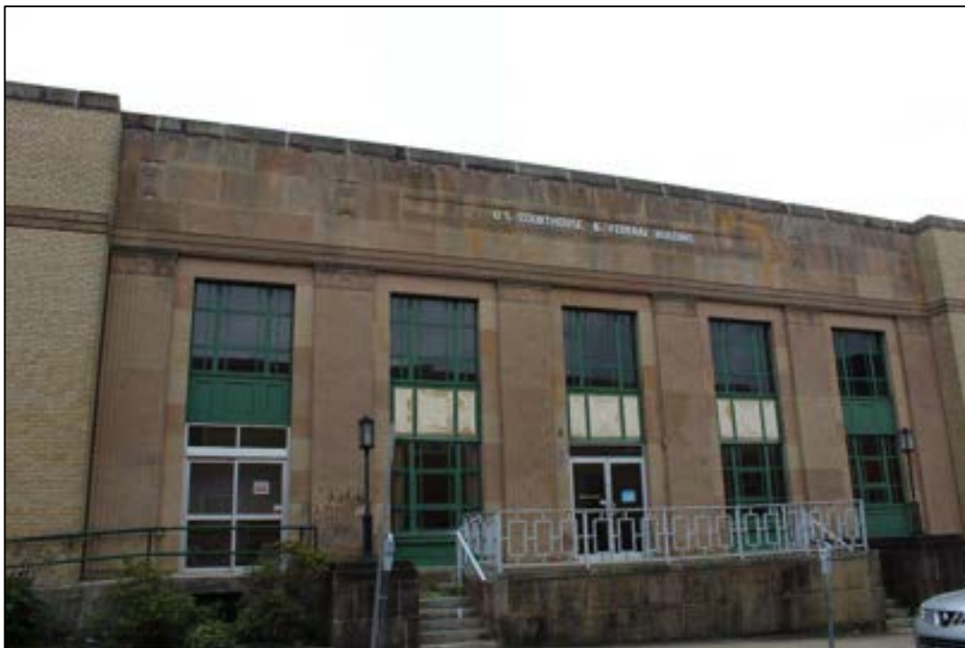
Photograph 2. RG-0014-0074, Post Office, 400 Neville St., Post Office, Facing West.
