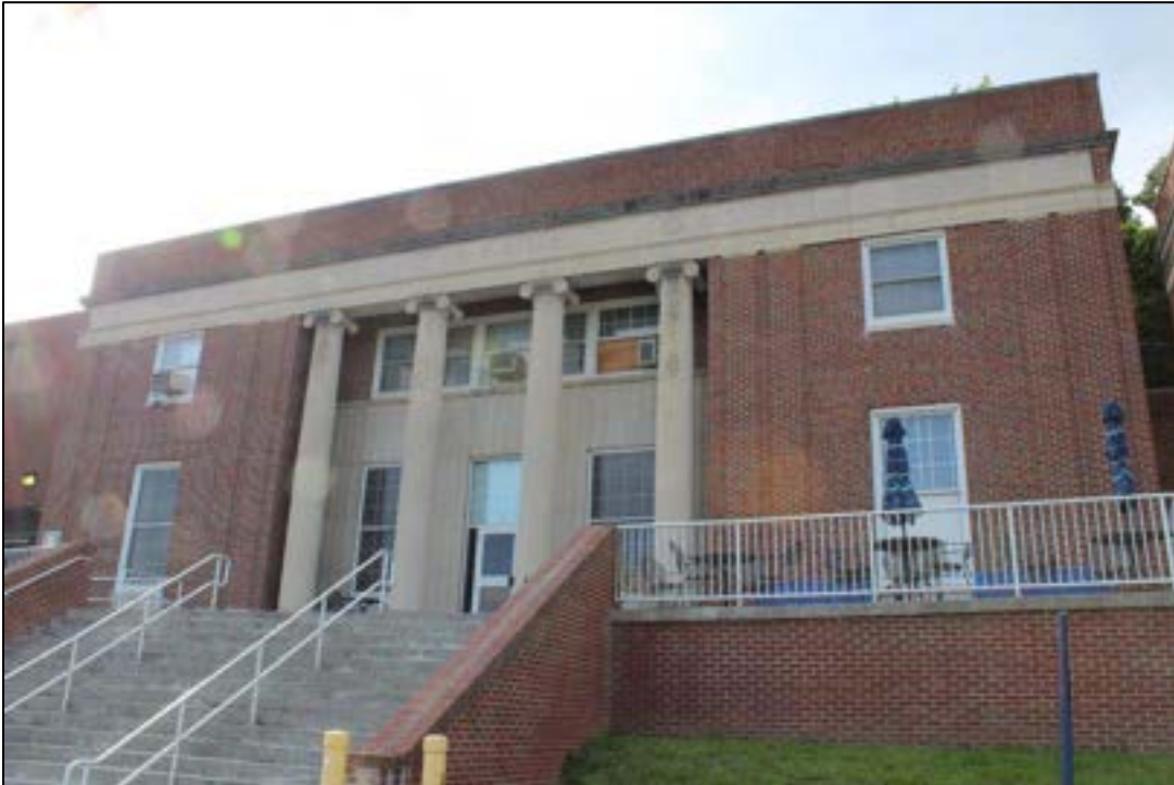
Photograph 1. MC-1893, Wendell G. Hardway Library, Bluefield State College, Facing Northwest.
