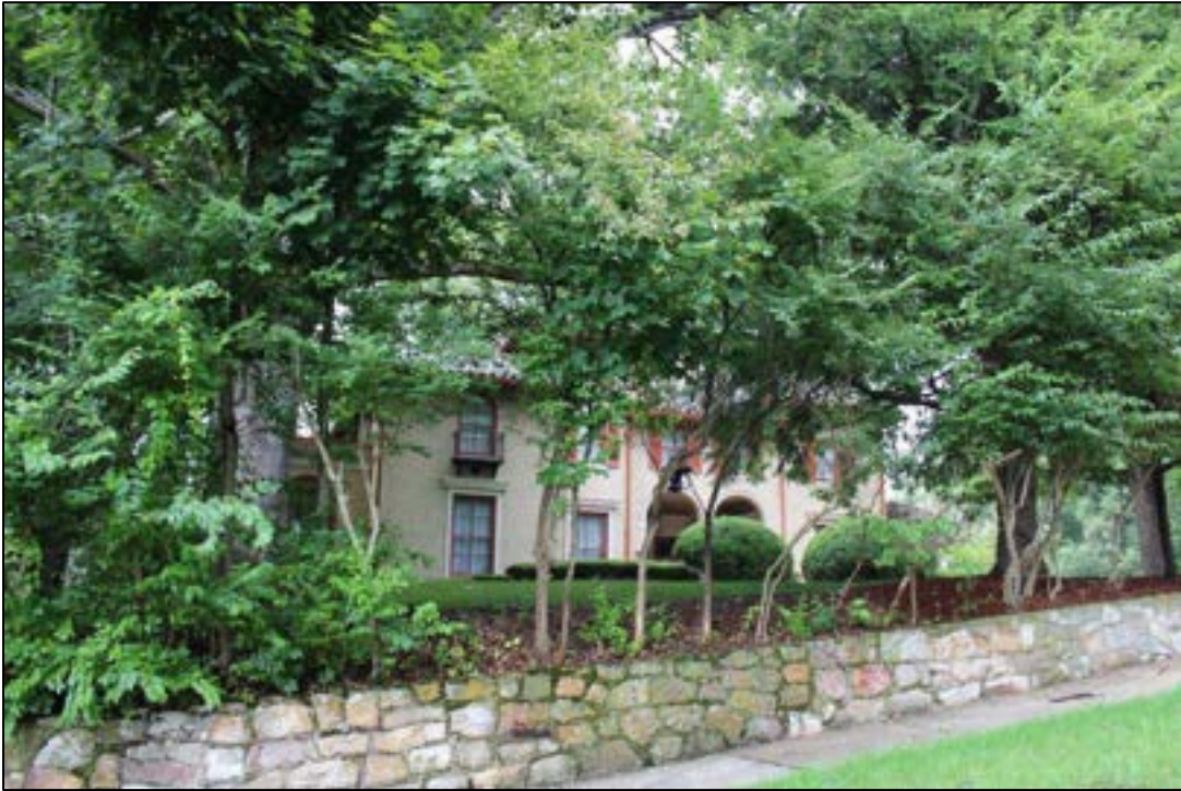
Photograph 1. MC-1970, Bodell House, 1430 Whitethorn St., Facing Northeast.
