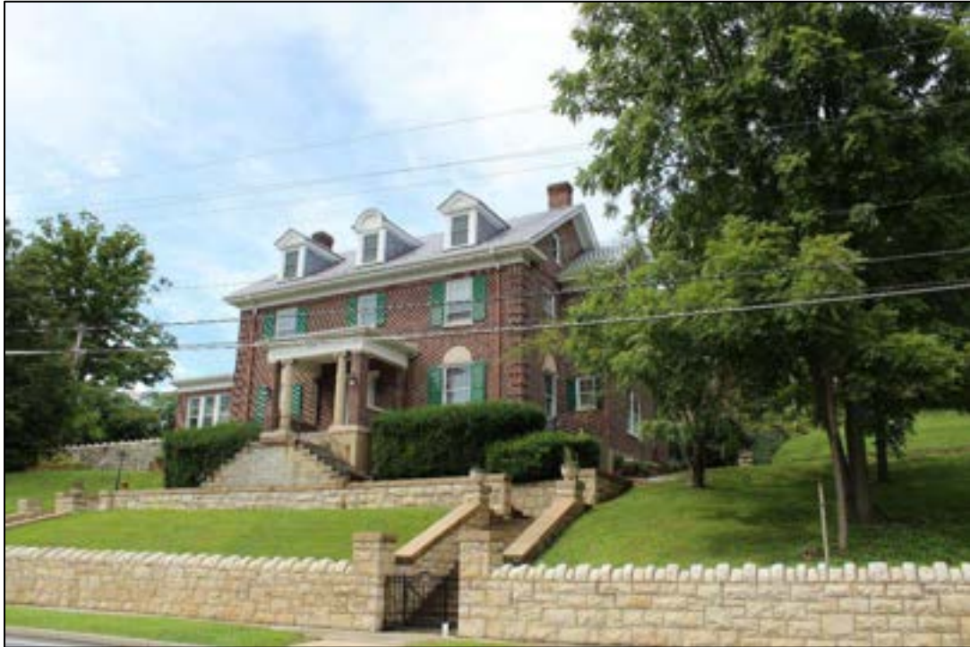
Photograph 3. MC-1965, Barger House, 2009 Bland Rd., Facing Northwest.
