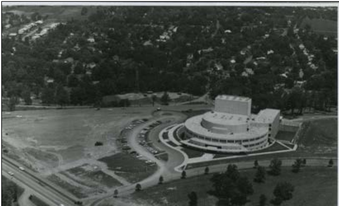
Figure 1. Creative Arts Center, West Virginia University, c.1965-1971 Source: WVU Photo Lab
