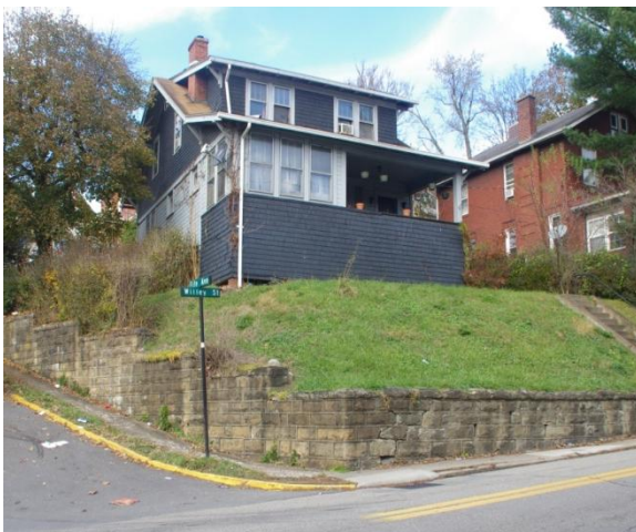
Fig. 25. 701 N Willey St and Fife Ave MG-2396
