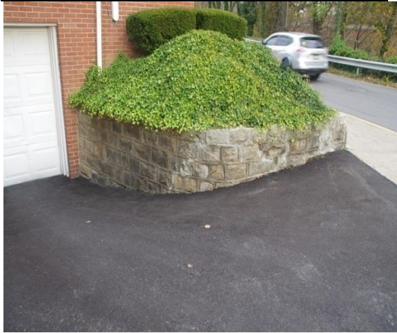
Fig. 72.153 Spruce Street/Kirk Street
