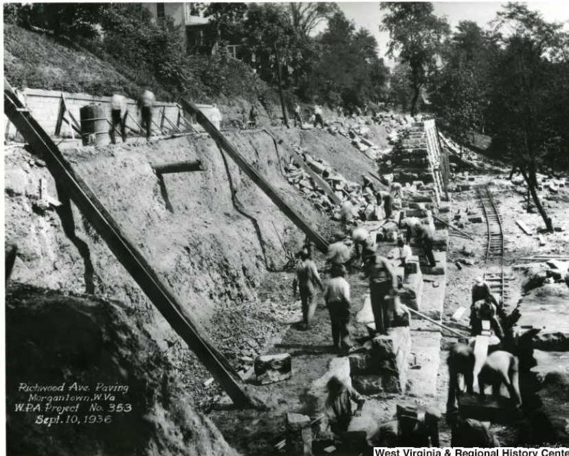
Construction of the lower Richwood Avenue wall.
