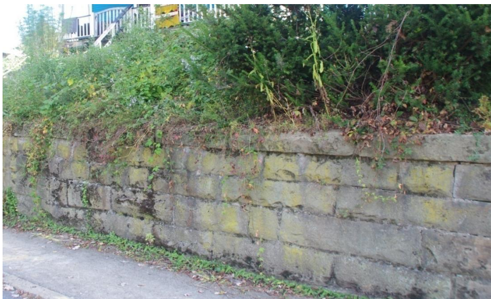
Fig. 6.Larger stones used for wall at 728 Richwood Avenue - Vol.II
