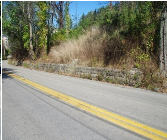
Fig. 40. 987 N Willey St-MG-2407 Willey Street Wall Project
