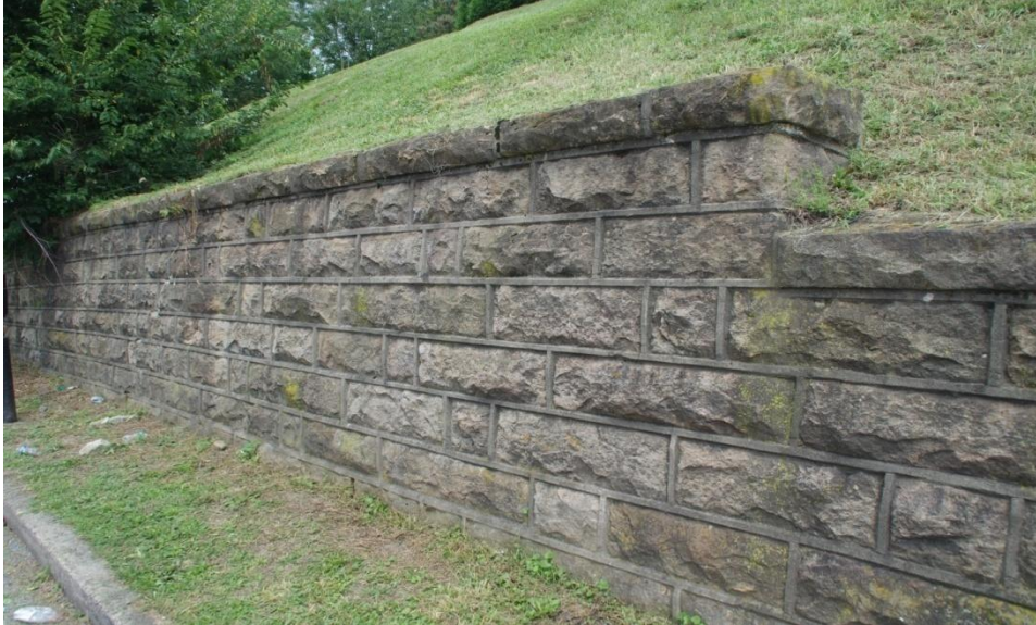
Fig. 1.Fife Avenue wall showing 2 and 3 stretcher coursing
