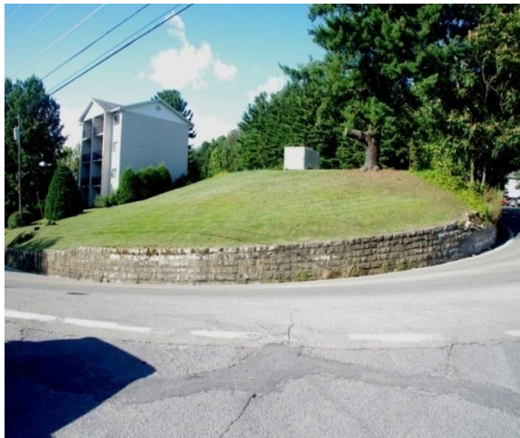
Fig. 39. 995 N Willey St-MG-2408 Willey Street Wall Project
