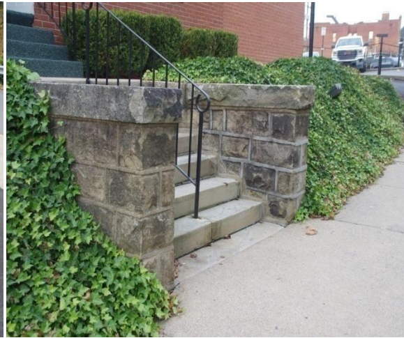
Fig. 73.153 Spruce Street/Kirk Street
