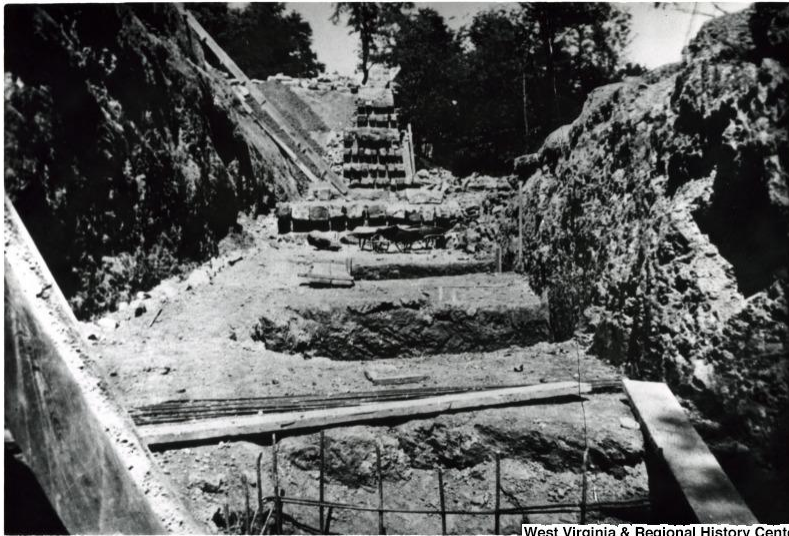
Digging the foundation for the Richwood Avenue wall.
