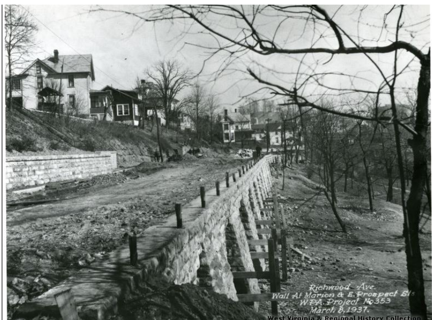
The completed Richwood Avenue walls.
