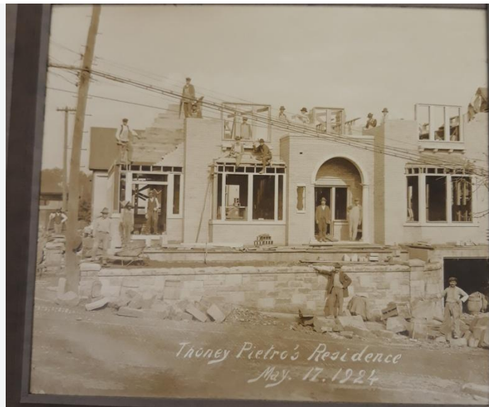
106 Wilson Street, 1924, Morgantown, WV.
