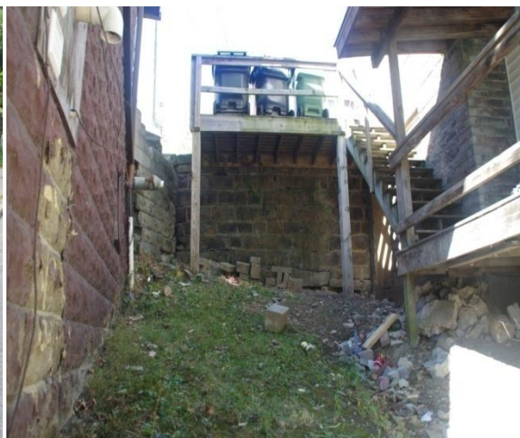
Fig. 34.670 N Willey St -East Side of St MG-2409
