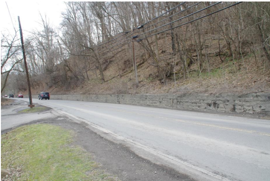
Figure 34 HPI Form MG-1924 - View Facing Northwest
