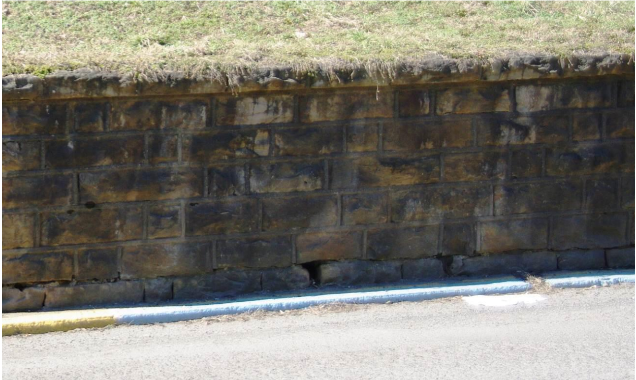
Figure 1: Eighth Street wall showing 2 and 3 stretcher coursing
