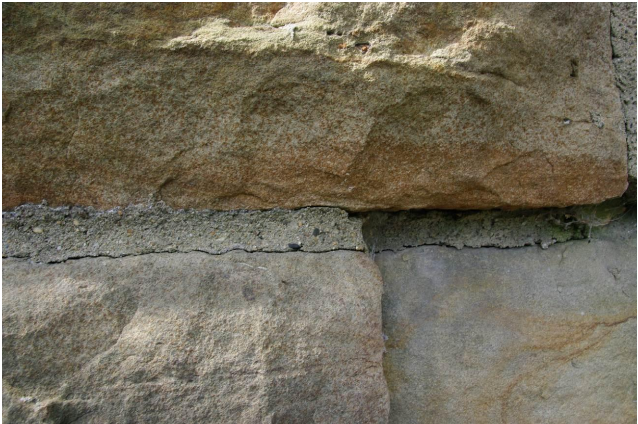
Figure 3: Concave joint used in Richwood Avenue wall
