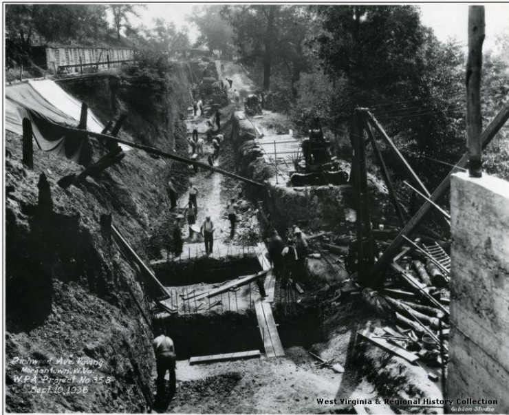
Figure 24 Richwood Avenue Paving, Morgantown, WV WPA Project 353
