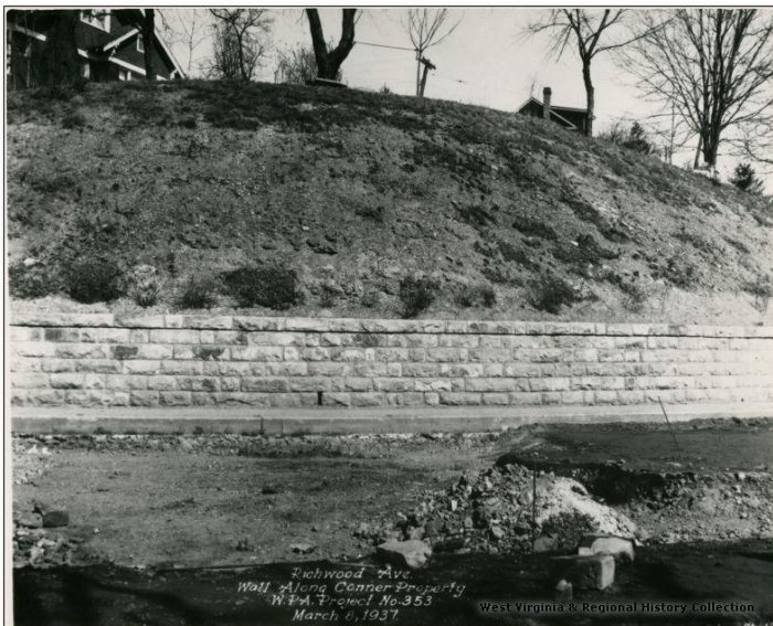
Figure 21 Richwood Avenue Wall Along Conner Property, Morgantown, WV WPA Project 353 3/8/1937 West Virginia & Regional History Collection, Photographs, https://wvrhc.lib.wvu.edu .
