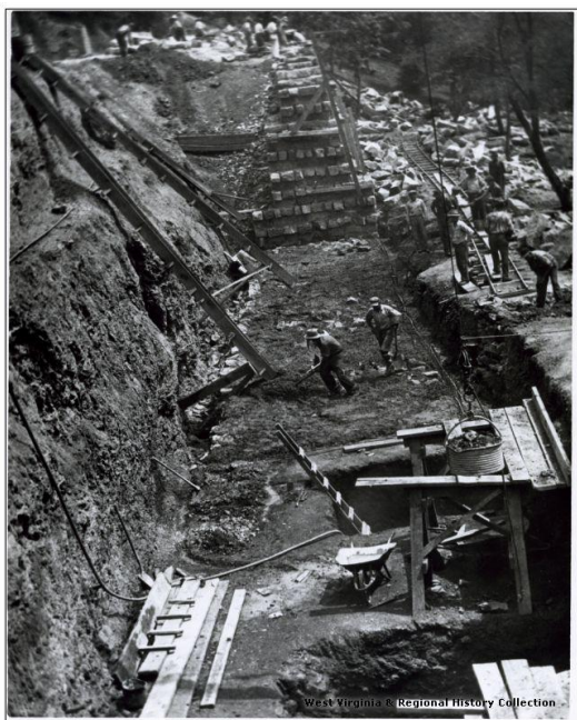
Figure 22 Pietro Company Road Crew at Work on Retaining Wall, Morgantown, WV No Date West Virginia & Regional History Collection, Photographs, https://wvrhc.lib.wvu.edu .
