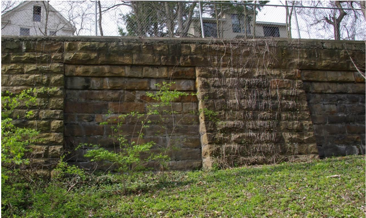
Figure 4: Larger stones of the Richwood Avenue wall
