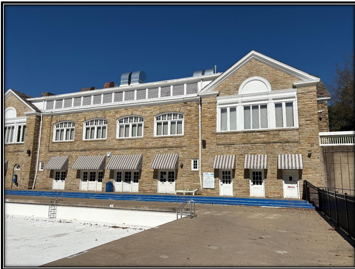
Photograph 7 of 32. The south (rear) elevation of the Pine Room, facing northwest.
