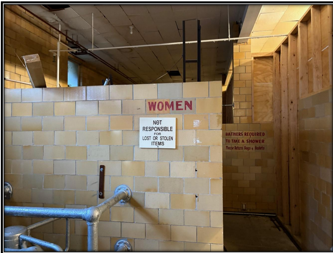
Photograph 13 of 32. The entrance to the women's dressing room, facing southeast.
