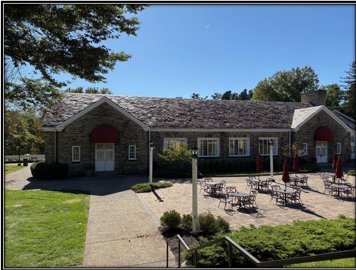
Photograph 2 of 32. The north (front) façade of the Pine Room, facing southwest.
