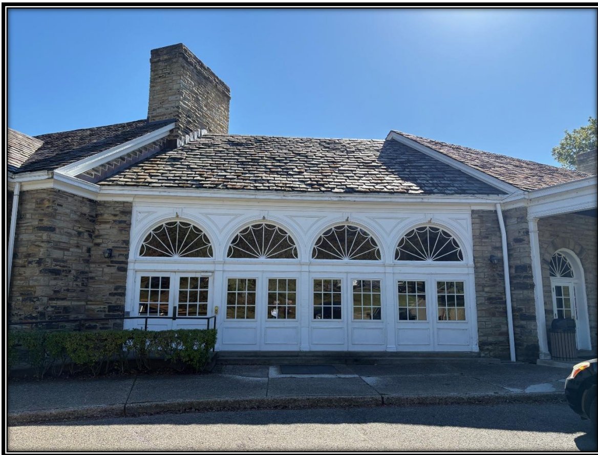
Photograph 15 of 32. The north façade of the hyphen, facing south.
