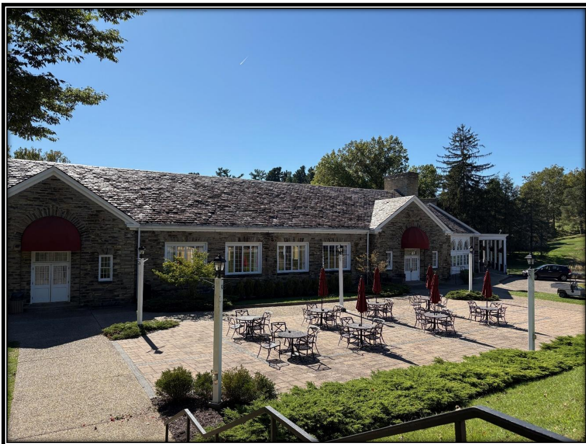
Photograph 1 of 32. The north (front) façade of the Crispin Center, showing all three segments of the building: the Pine Room, hyphen, and Clubhouse, facing southwest.
