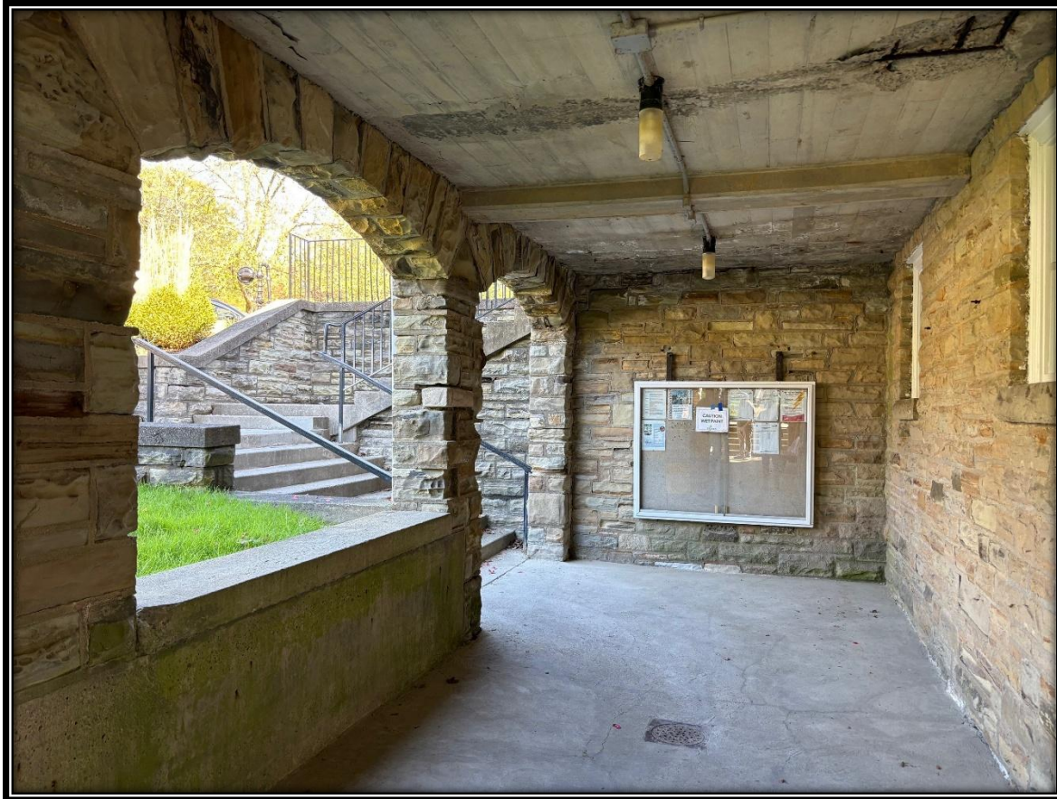
Photograph 20 of 32. View from under the promenade, facing northeast.
