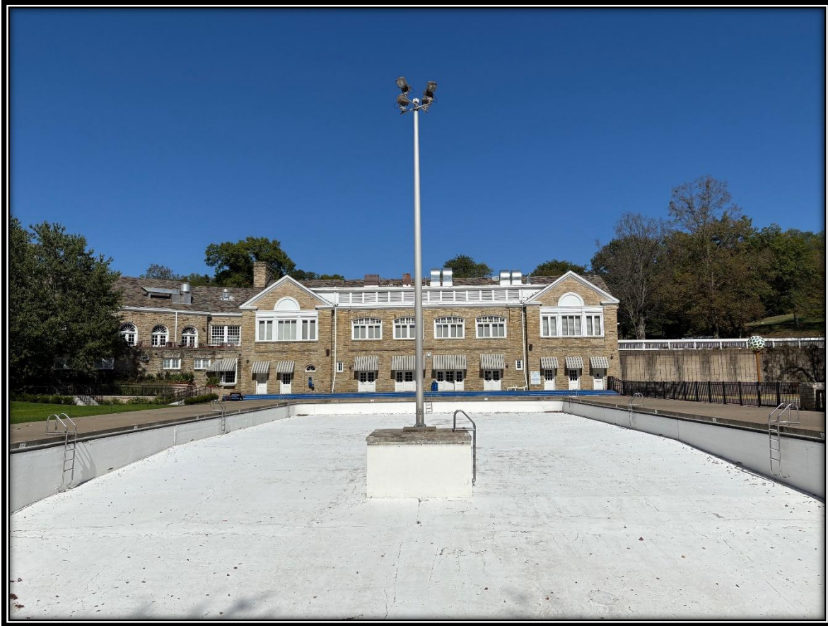
Photograph 6 of 32. The south (rear) elevation of the Crispin Center, facing northeast.
