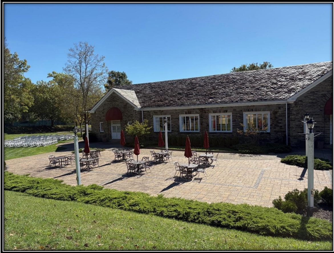
Photograph 3 of 32. The north (front) façade of the Pine Room, facing southeast.
