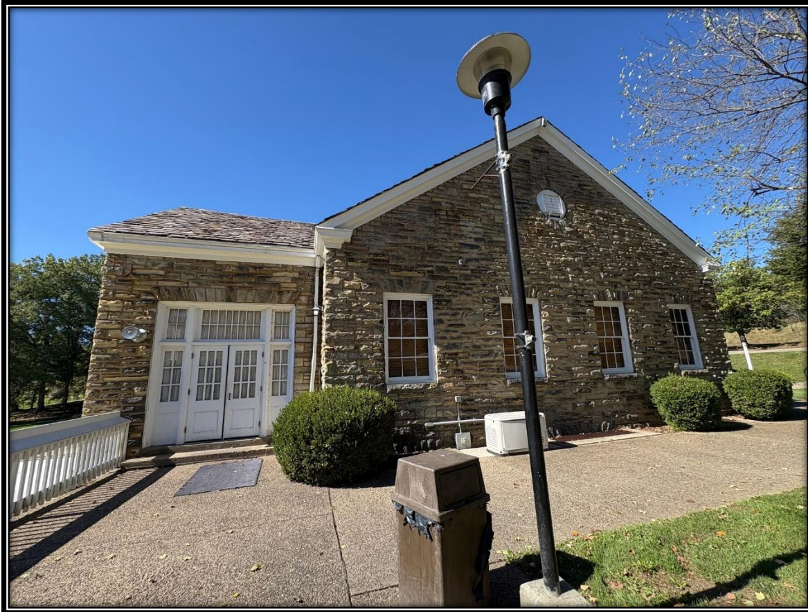
Photograph 5 of 32. The east elevation of the Pine Room, facing northwest.
