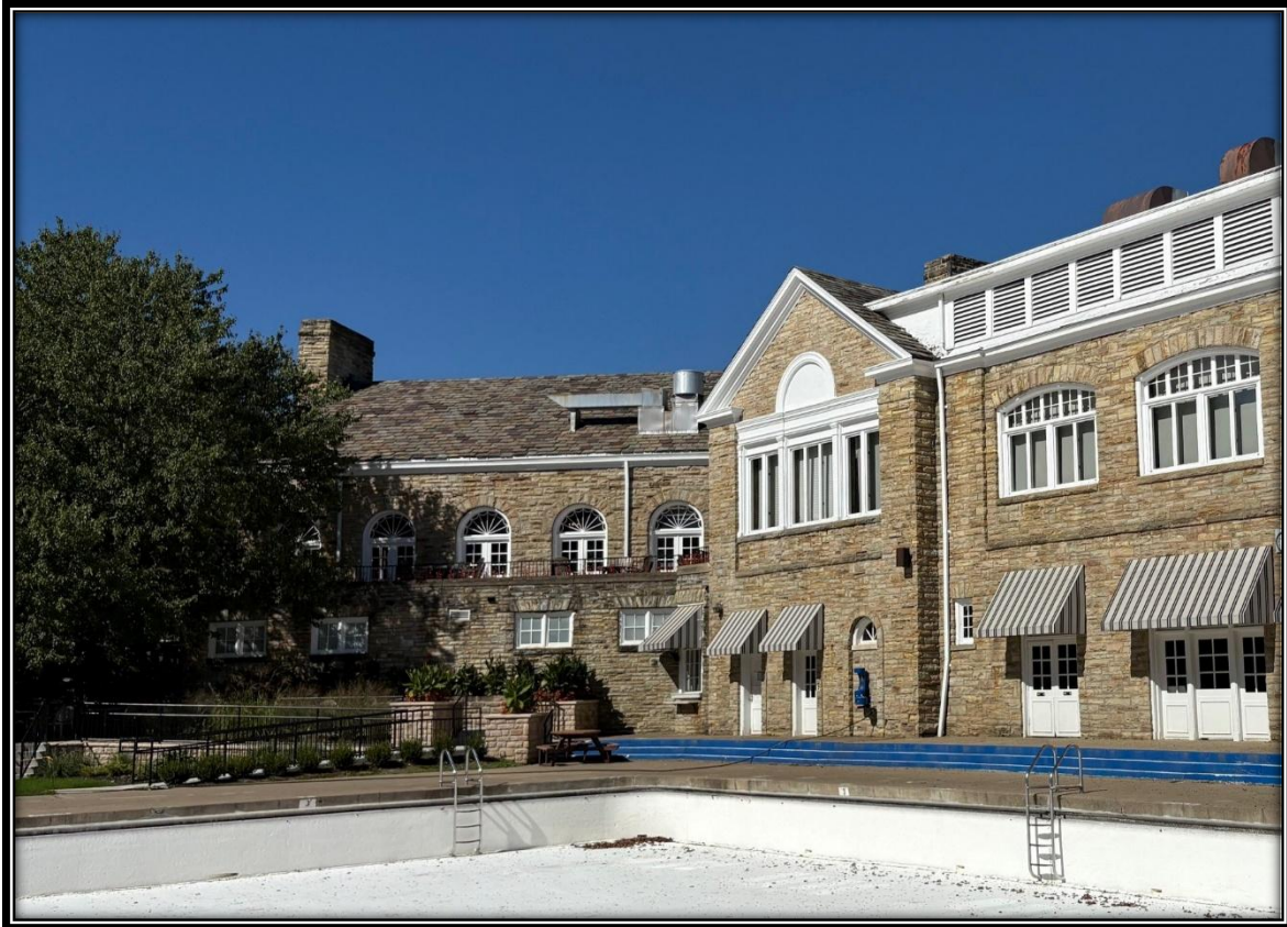
Photograph 22 of 32. The south (rear) elevation of the golf clubhouse, facing northwest.
