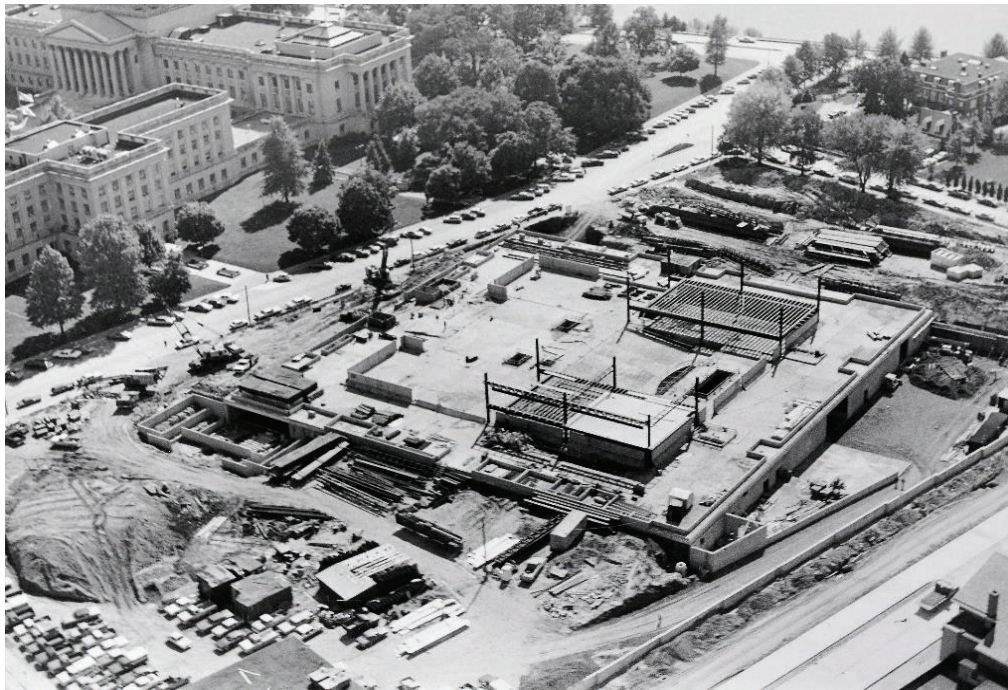
Figure 10 Culture Center under construction in 1973. From Goldenseal magazine, Summer 2016.
