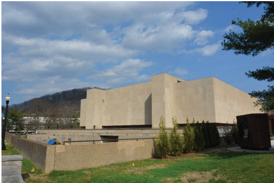
Photo 18 Exterior, west side of Culture Center, camera facing northeast
