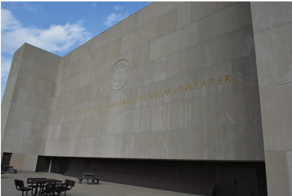
Photo 19 Rear (west) side of Culture Center with state seal engraving, camera facing northeast
