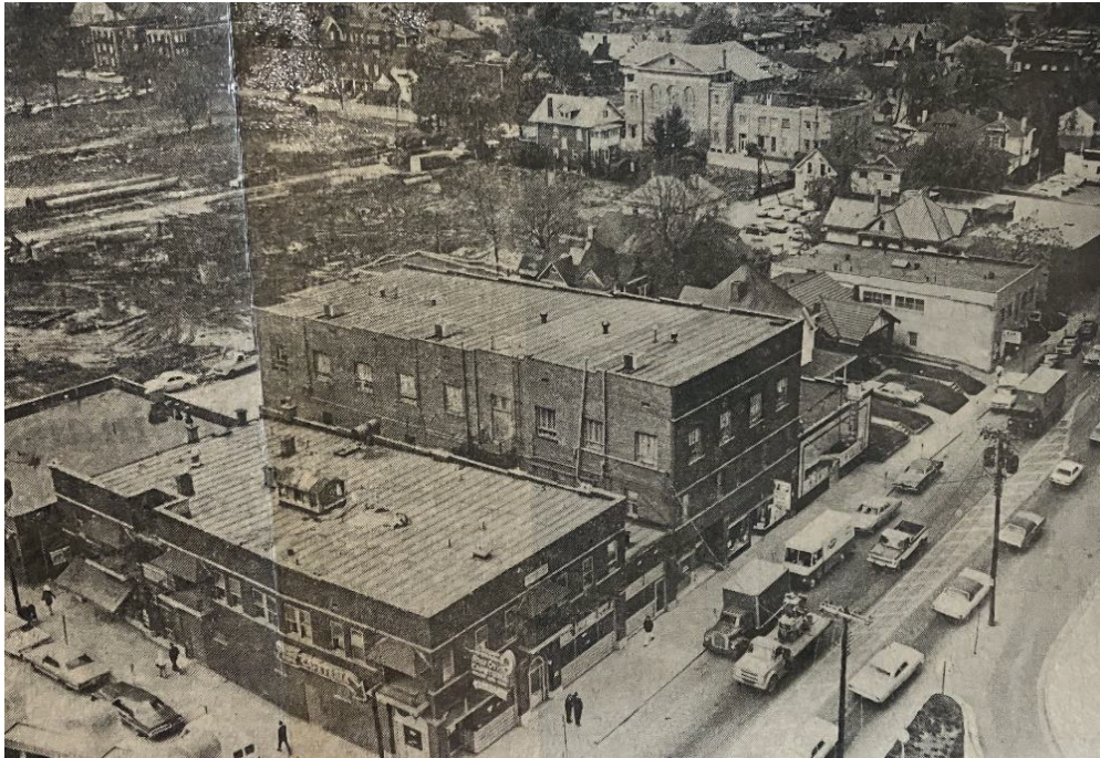
Figure 9 Rose City Block Partly Demolished. From the Charleston Gazette, May 9, 1973.
