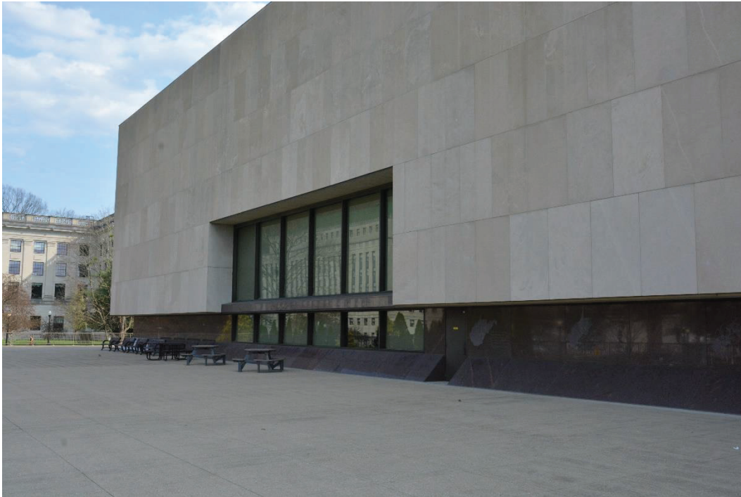
Photo 22 Exterior, north side windows, camera facing southeast
