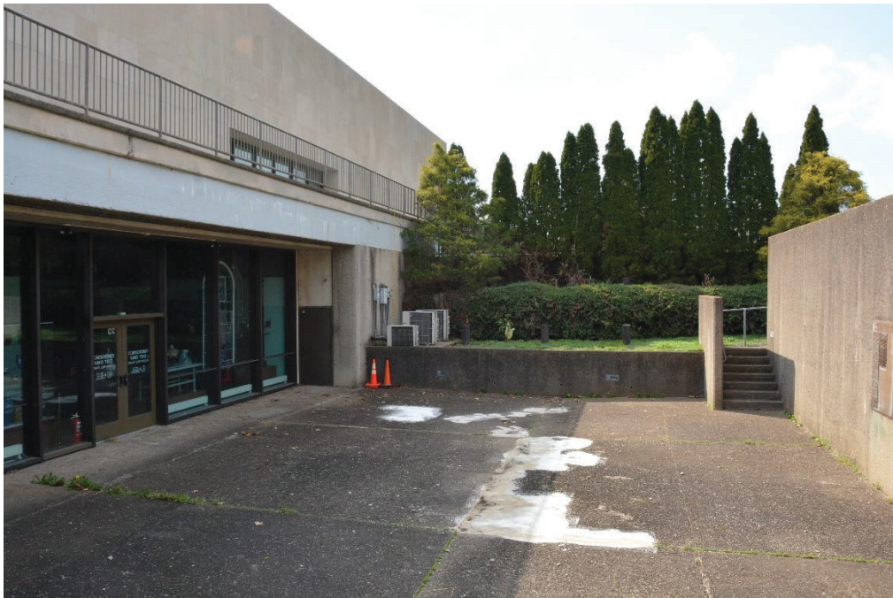
Photo 6 Exterior, northeast lightwell, camera facing west
