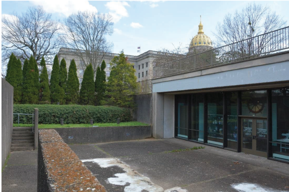
Photo 7 Northeast lightwell, camera facing east
