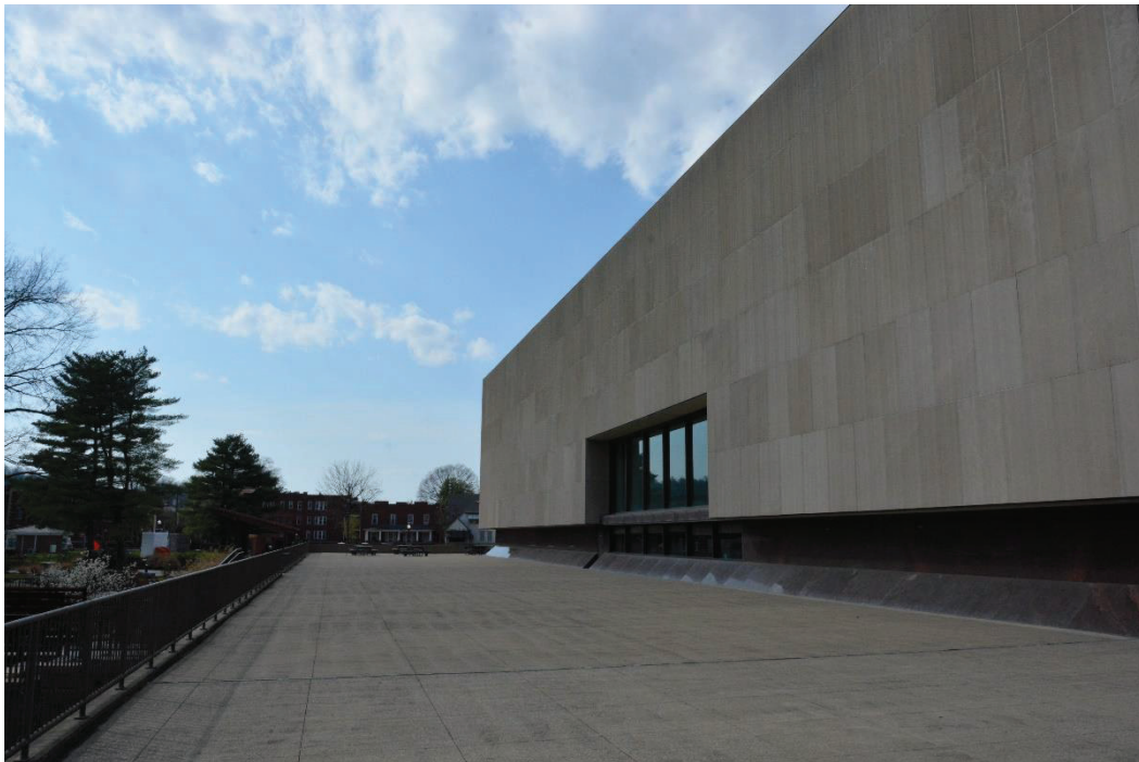
Photo 16 Exterior, south deck of Culture Center, camera facing west
