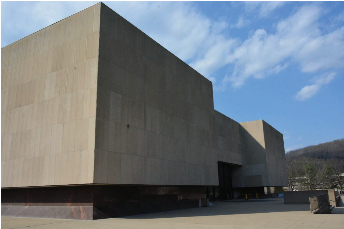
Photo 9 Exterior, front of Culture Center, camera facing northwest
