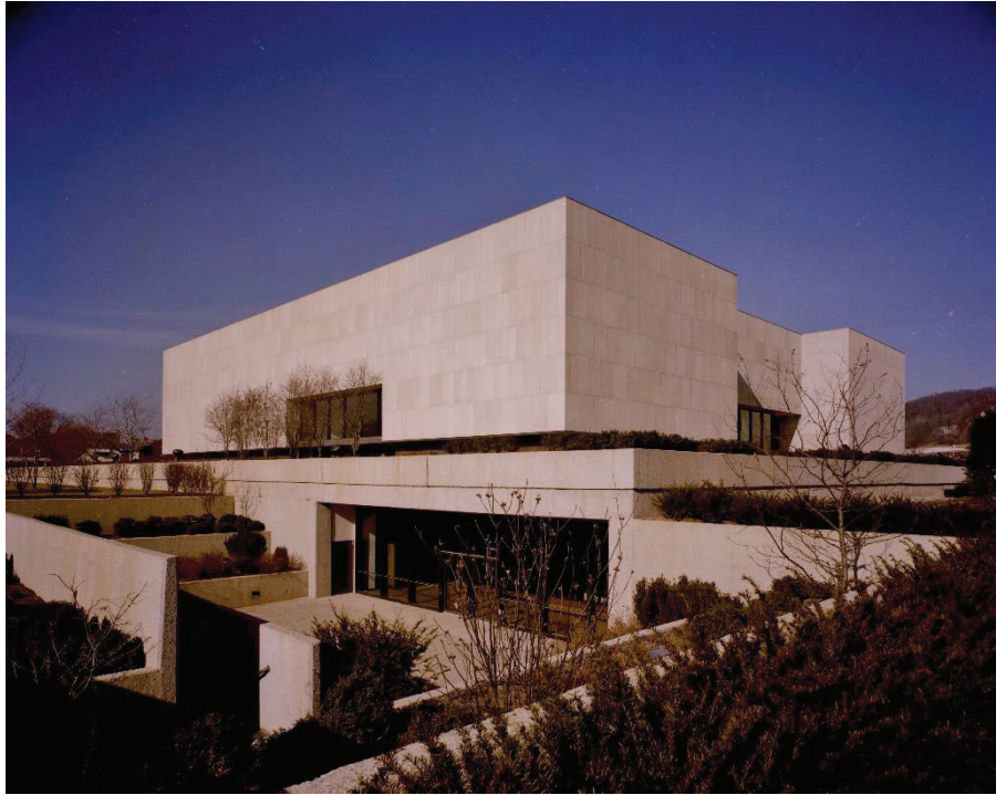
Figure 14 Southeast lightwell in 1976. Courtesy of Silling Associates.
