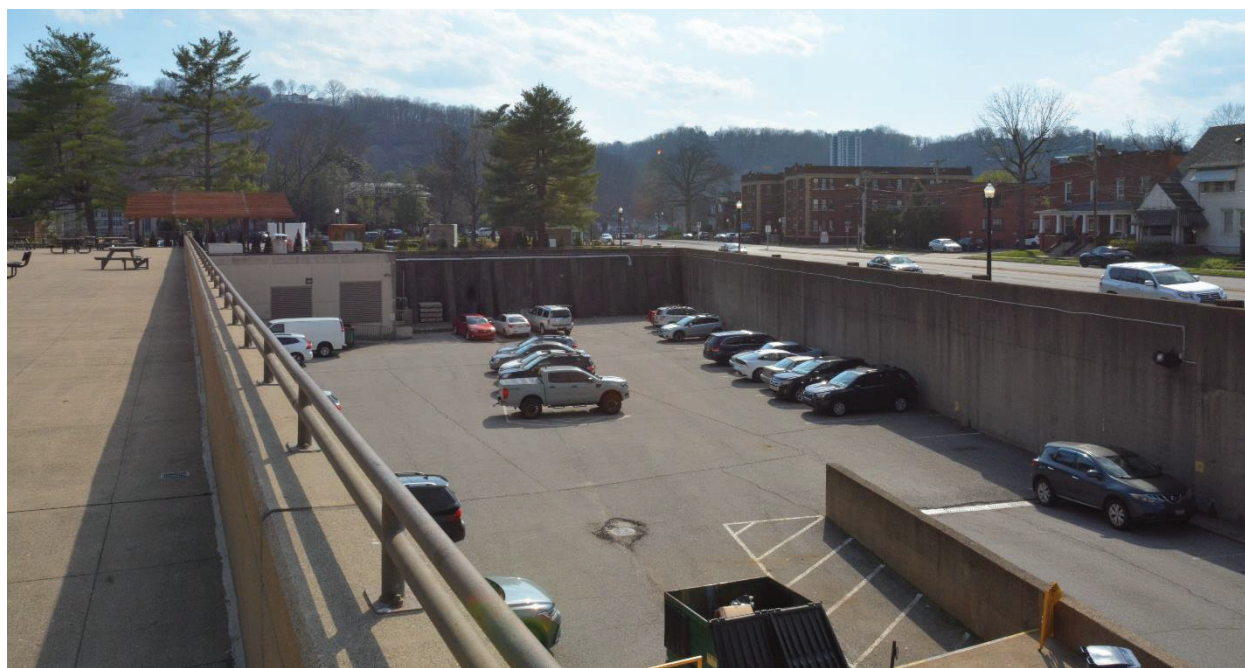
Photo 20 Parking lot and retaining wall, camera facing southwest
