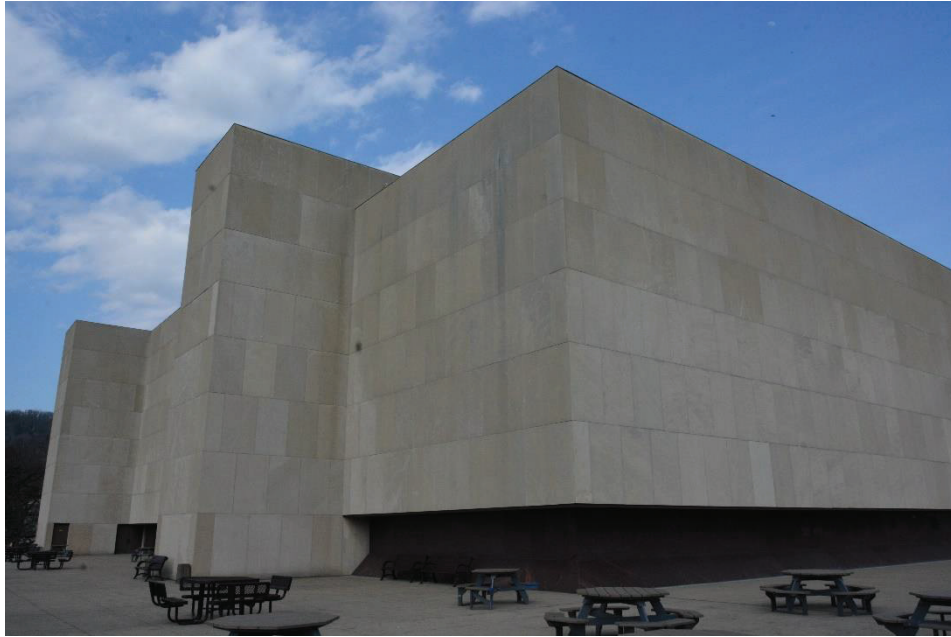
Photo 17 Exterior, southwest corner of Culture Center, camera facing northeast
