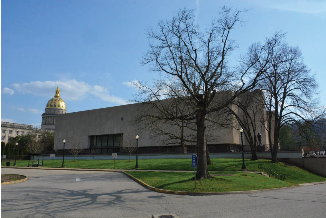
Photo 8 Exterior, northwest side of Culture Center, camera facing southeast
