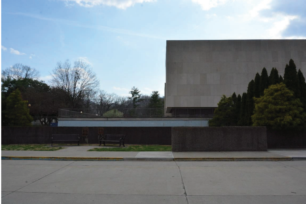
Photo 5 Exterior, northeast corner of Culture Center, camera facing south
