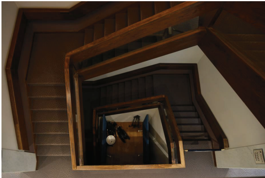
Photo 42 Balcony's north side staircase, camera facing east and downwards
