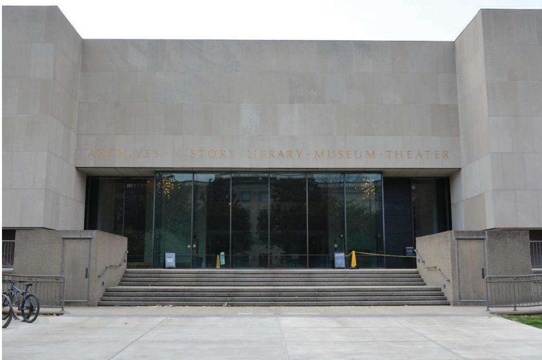
Photo 1 Exterior, front entrance of Culture Center, camera facing west
