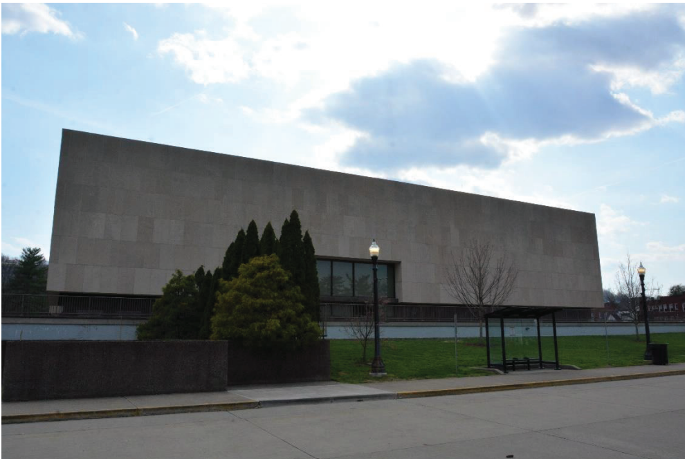
Photo 4 Exterior, north side of Culture Center, camera facing south
