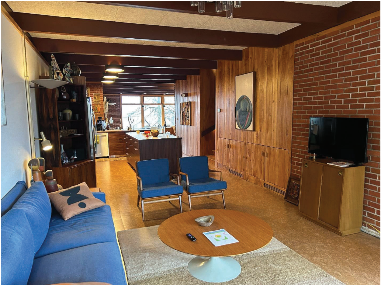
Photo 14 View of the first floor interior taken from end of living room on west side of house. Details of tongue and groove birch wall panels and western brick column. Shows open floor living space flow as living room goes from kitchen into dining room. Camera facing east.
