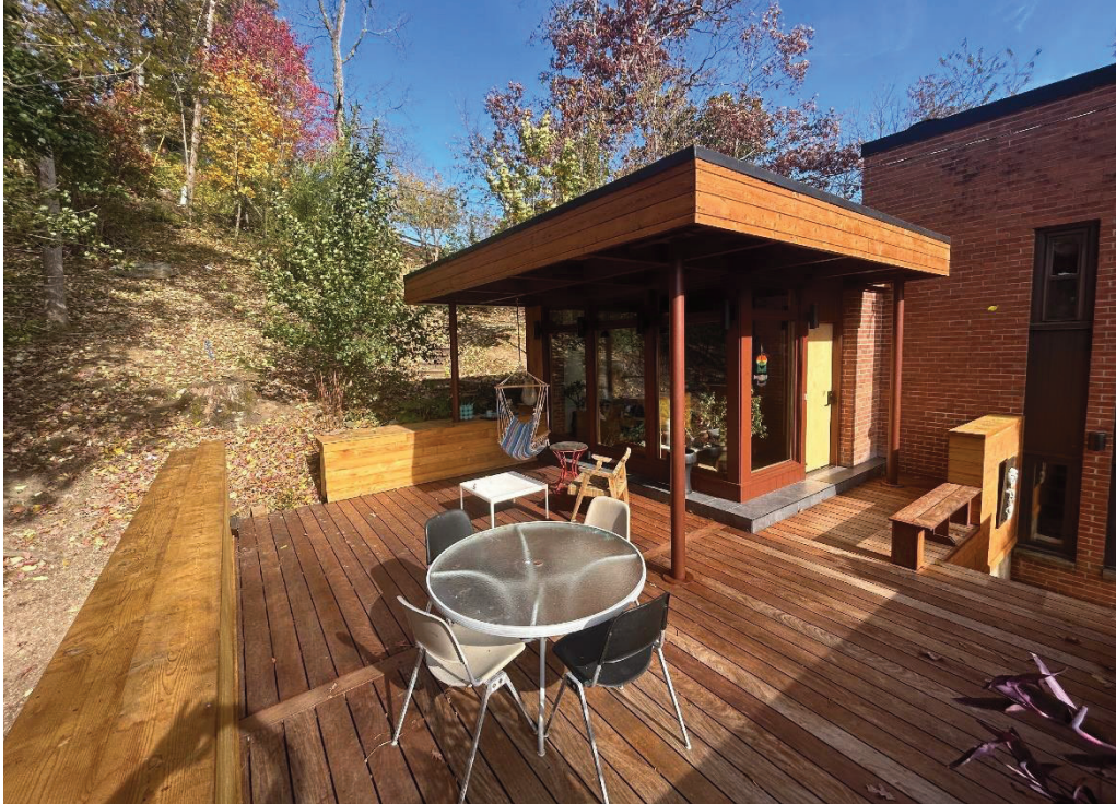
Photo 6 Depicts the deck flooring, sheltered overhang of western wing/living room windows, steel pole supports, western brick column with exterior windows and first floor entry door. Camera facing north.
