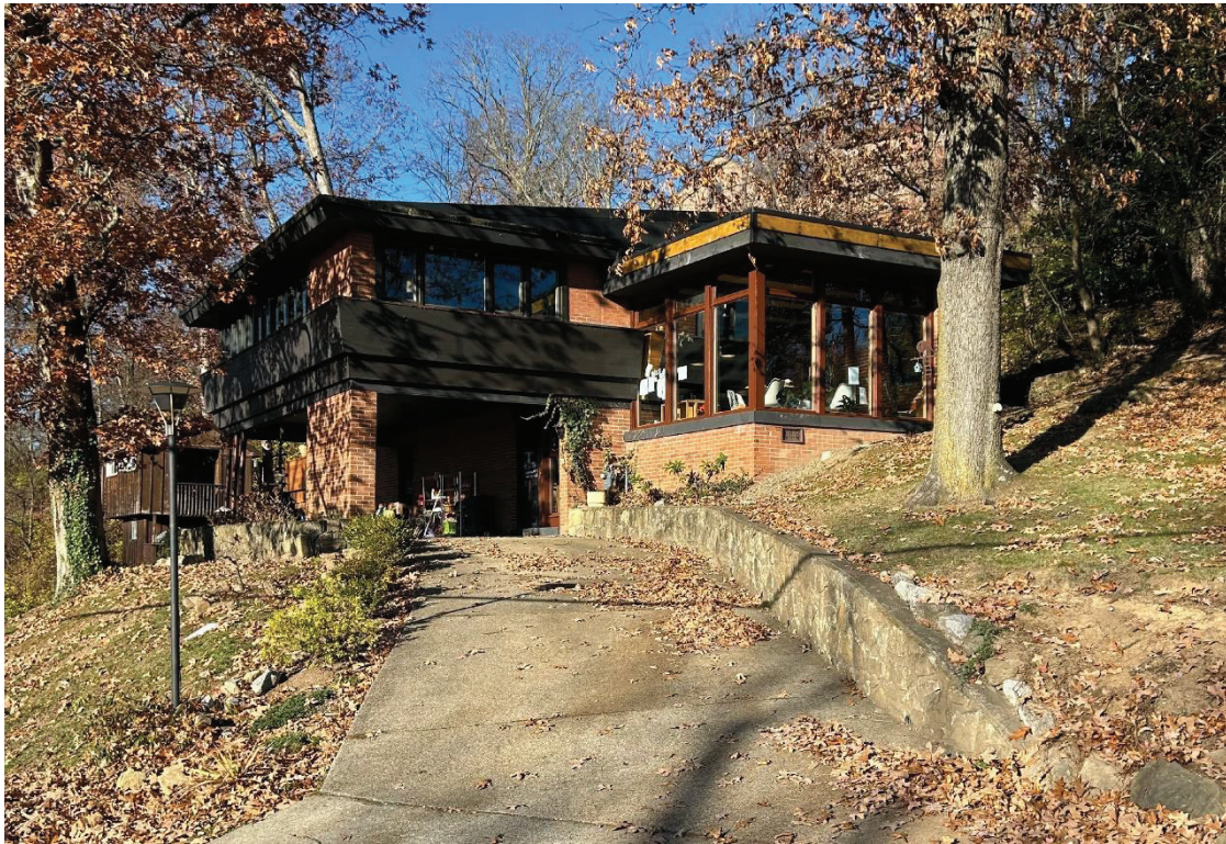
Photo 2 Photo of the house from the driveway with carport, second floor and glass windows of living room visible. Camera facing northwest.
