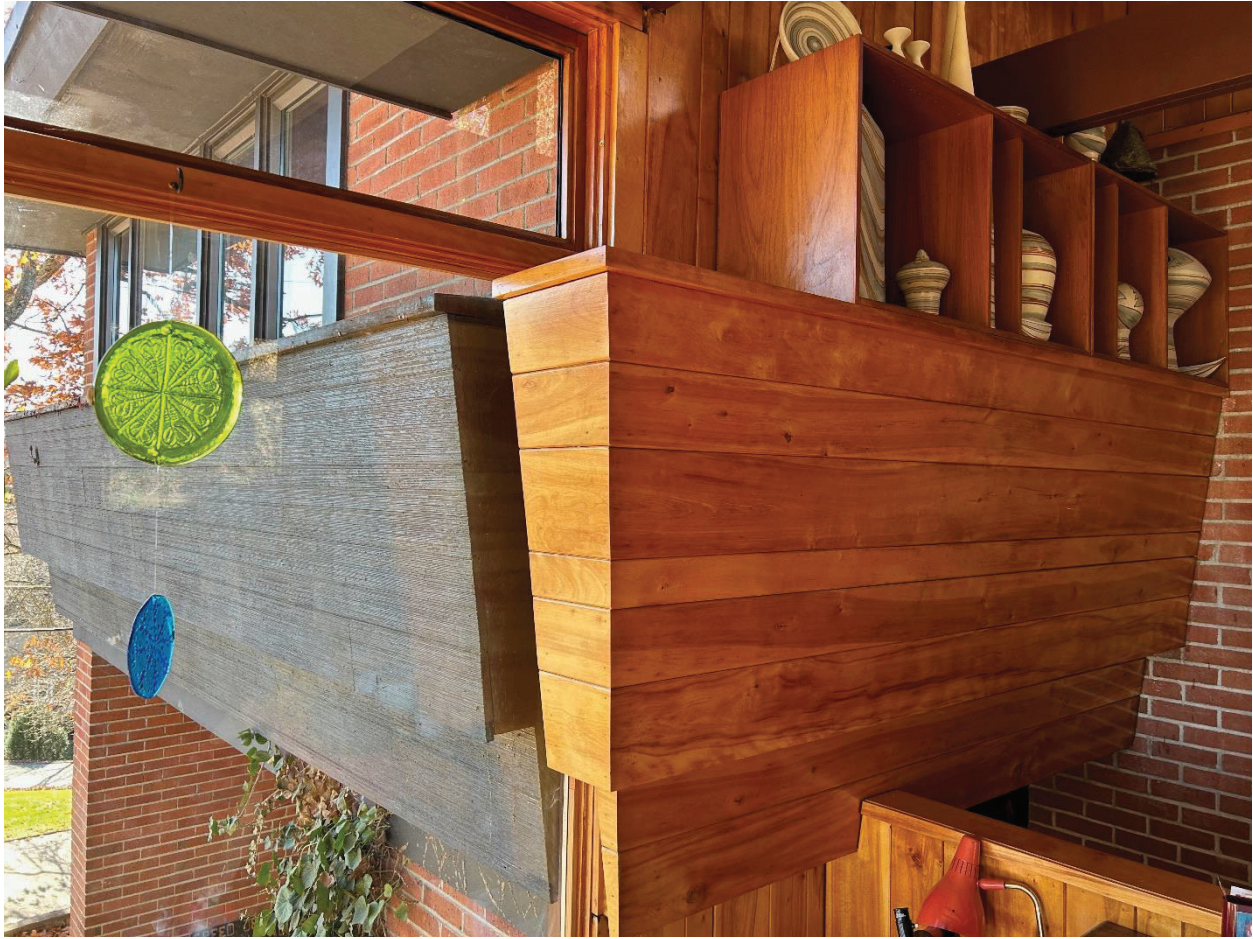
Photo 9 Depicts how the interior birch feature wall meets with the exterior cedar siding at the dining room windows. Showcases the way the interior and exterior lines are blurred. Camera facing southwest.
