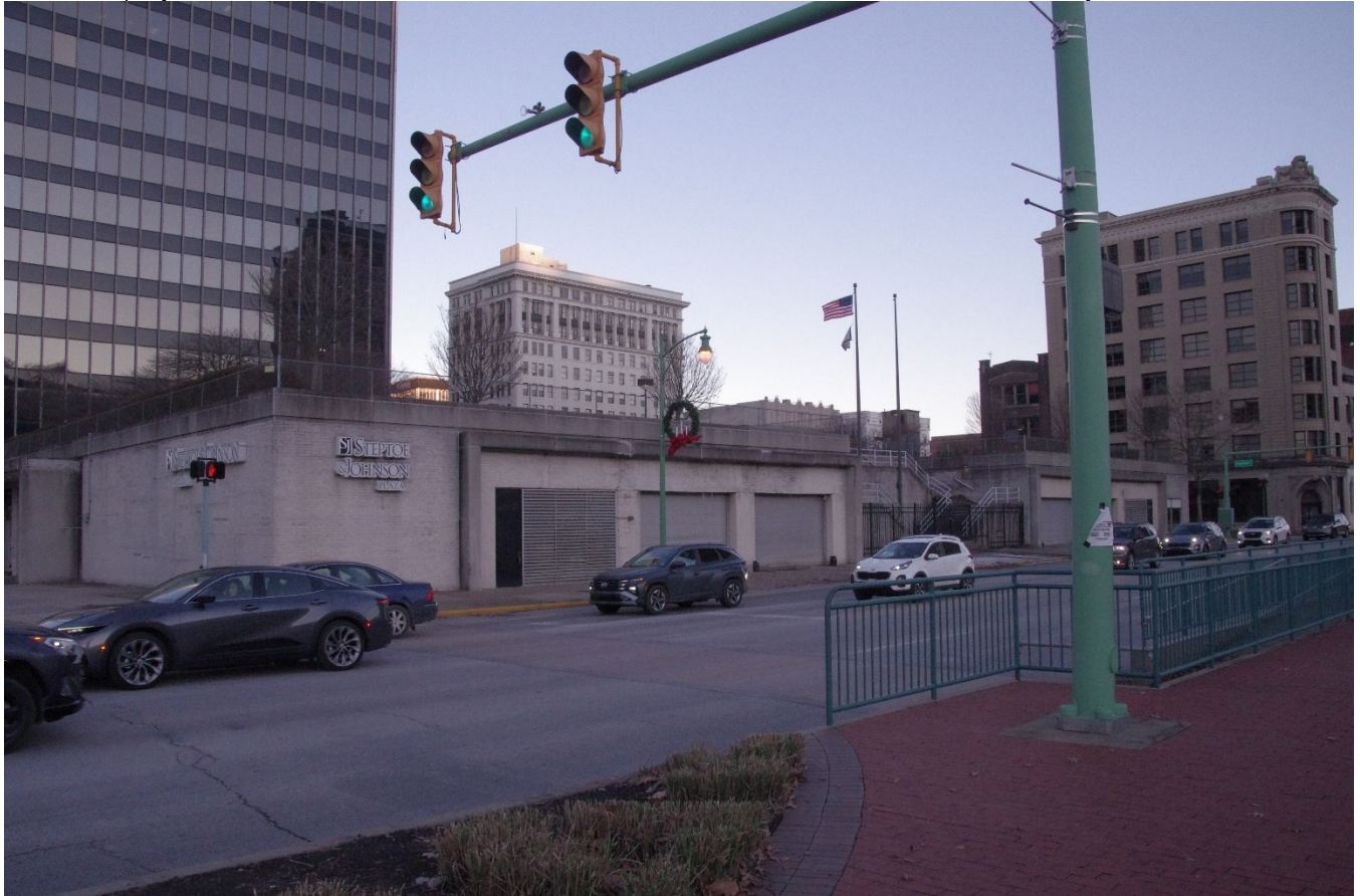
Photo 13 Resource 182. Looking east on Kanawha Boulevard
