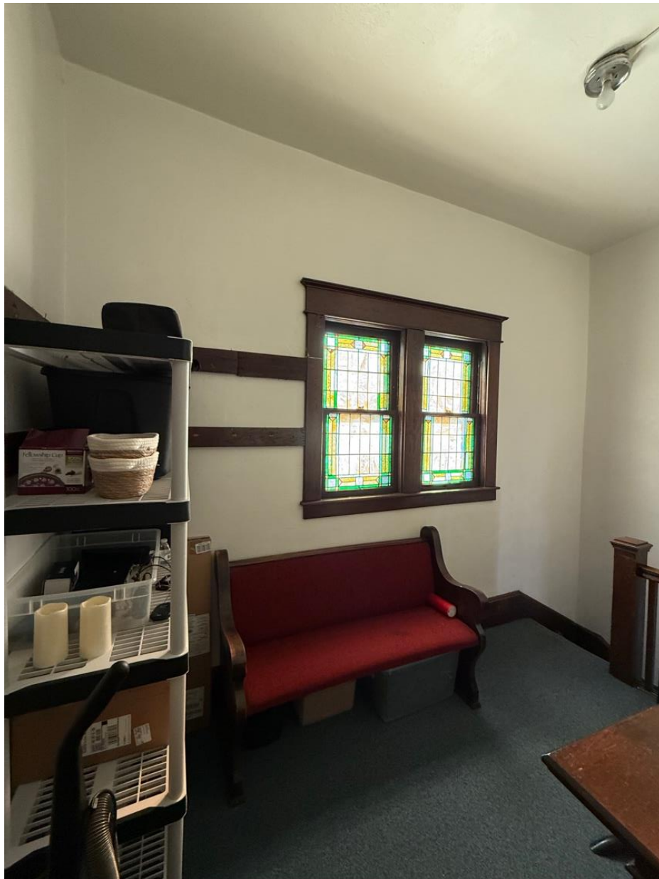
Photo 13: Interior view of a small room in the northwest corner of the first story of the building and the second set of stairs leading to the basement; camera pointed northwest.
