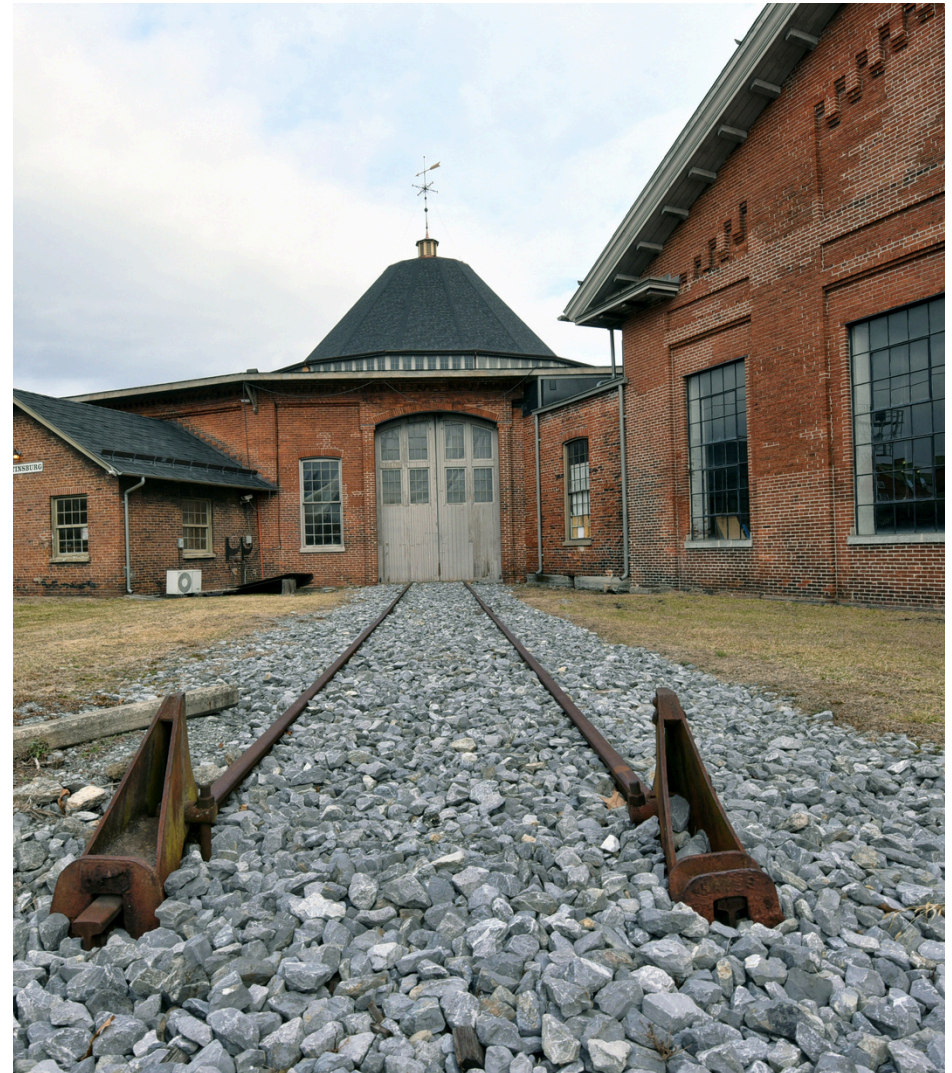
B&O Railroad Martinsburg Shops, Photo courtesy of Steve Brightwell, 2023.
