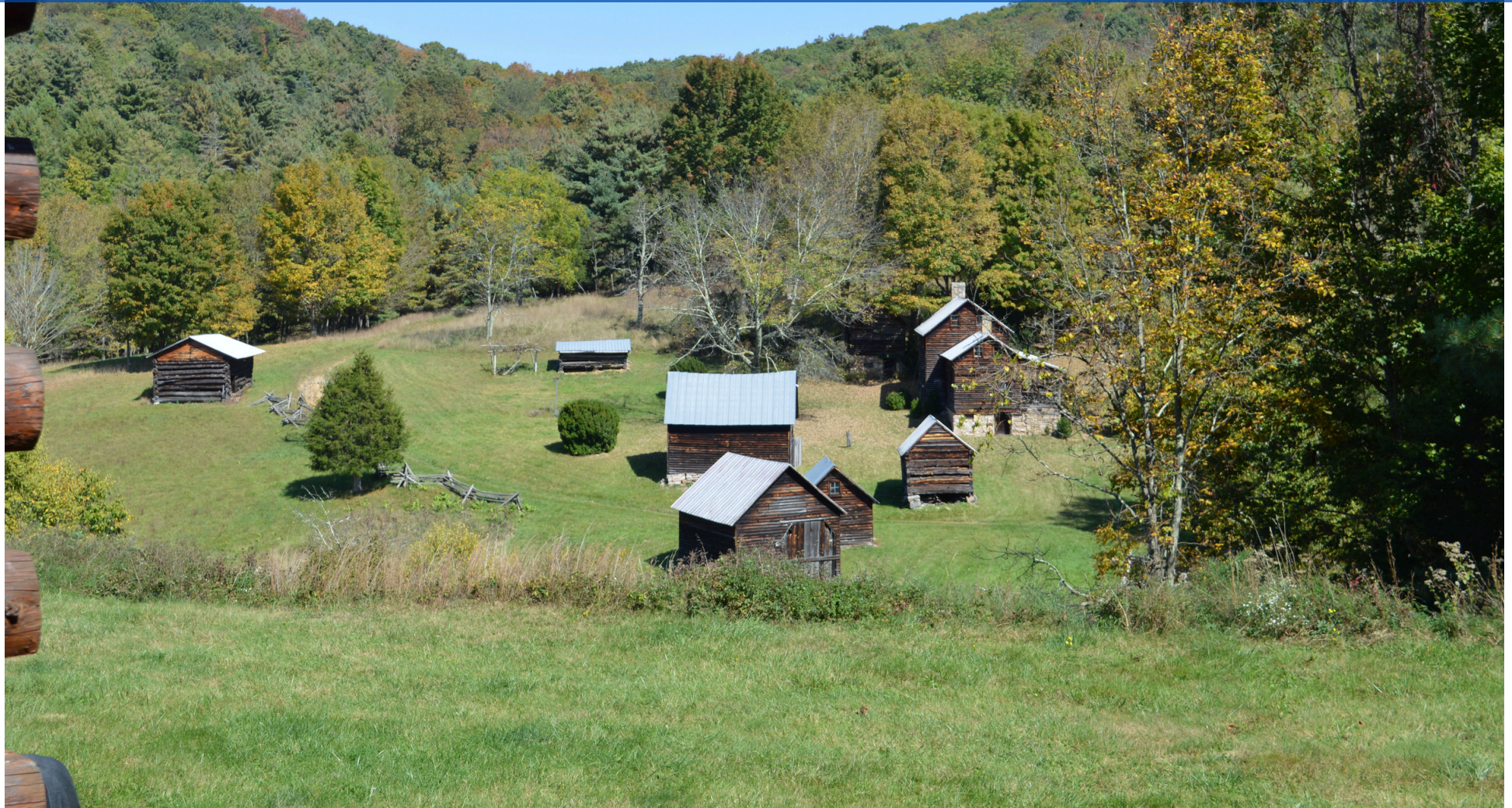
Ananias Pitsenbarger Farm, Photo courtesy of WV SHPO, 2021.
