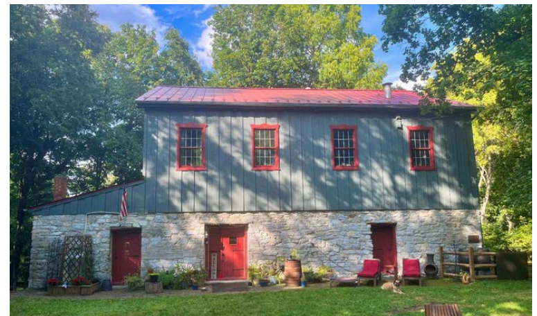
Thomas Shepherd Grist Mill Before & After. Photo courtesy of Andy Beall. Shepherdstown, WV.
