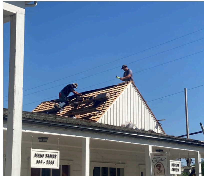
Roof replacement funded by WV SHPO grant in Arthurdale, Photo courtesy of Elizabeth Satterfield, 2023.
