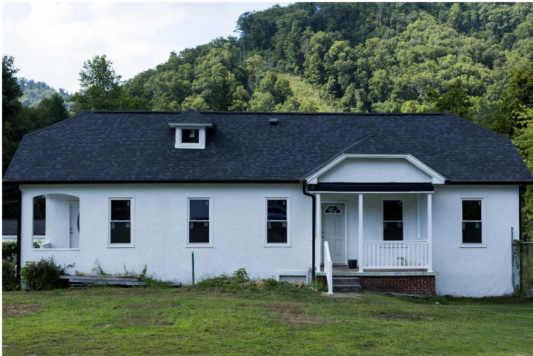
Photo 2 South side of Nurses Home, north elevation
