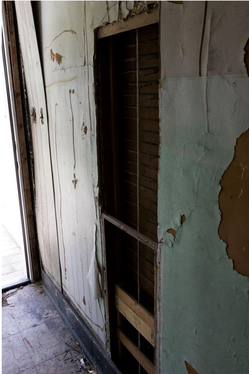
Photo 8 Pulley system used to lift and lower attic staircase, southwest elevation
