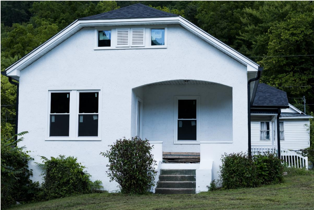
Photo 1 Southwest side of building, showing corner porch, east elevation
