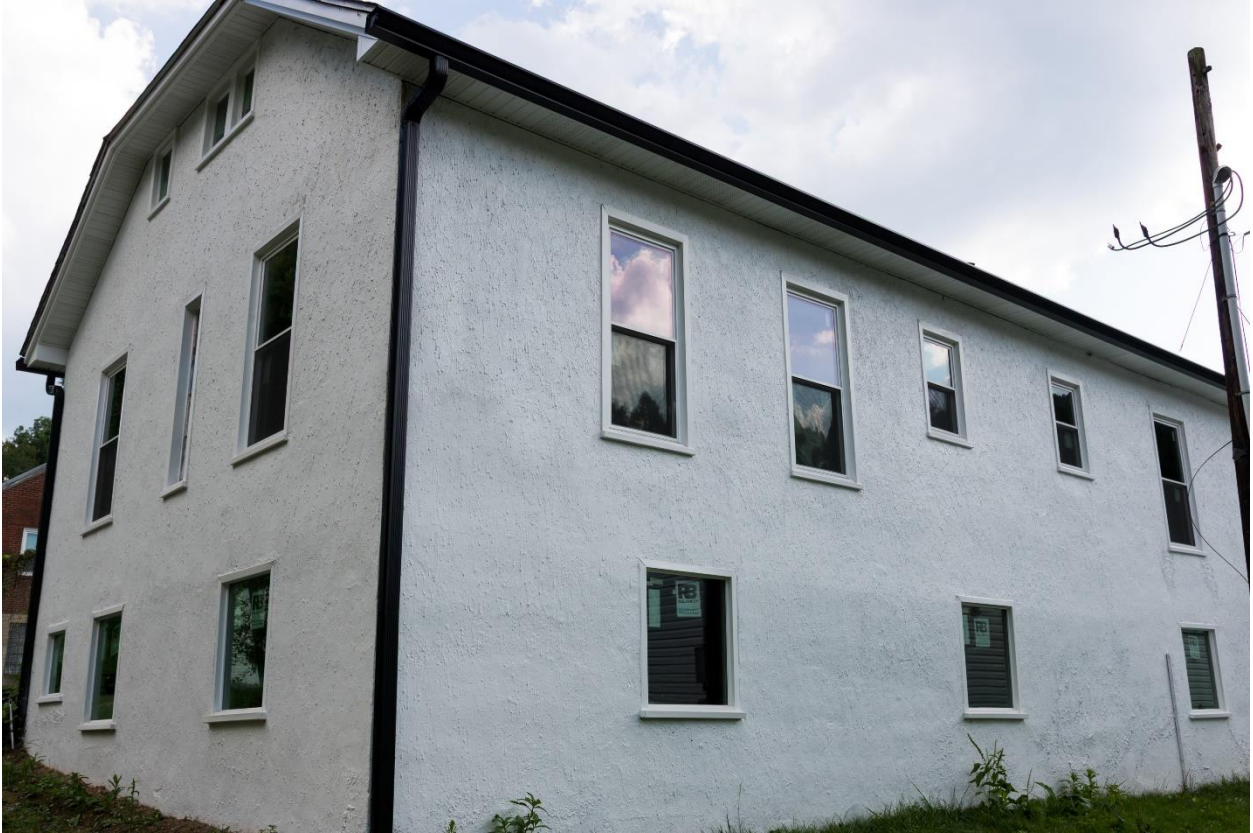
Photo 4 North side of Nurses Home, south elevation
