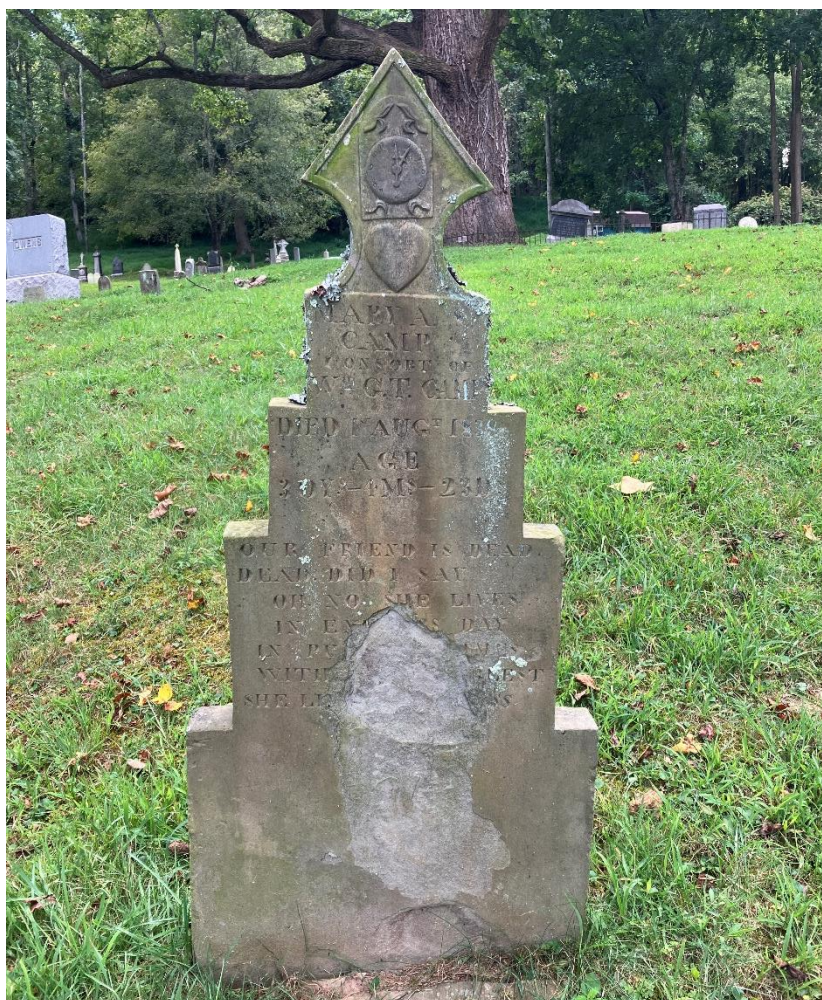
Figure 2 Example of deterioration on this sandstone marker for Mary A. Camp from 1838.
