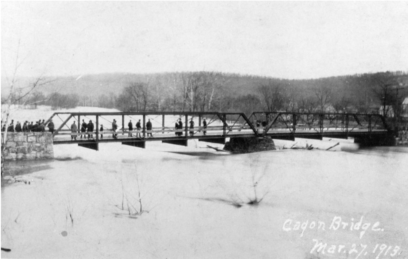
View of the second Capon Bridge, a pony truss bridge
