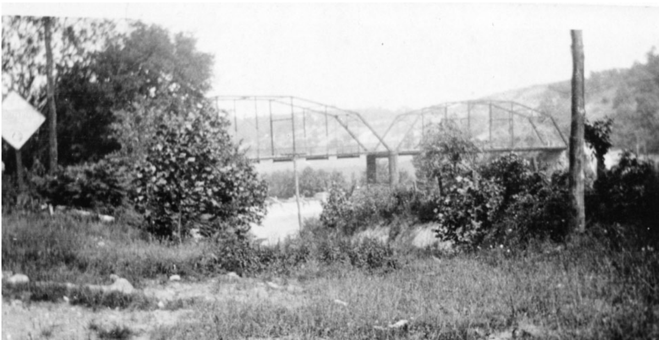
View of the third Capon Bridge, a two span Pratt Through Truss
