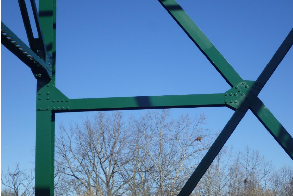
12. 1978 Horizontal Member Added to The Capon Bridge, detail. Note bolts in lieu of rivets.
