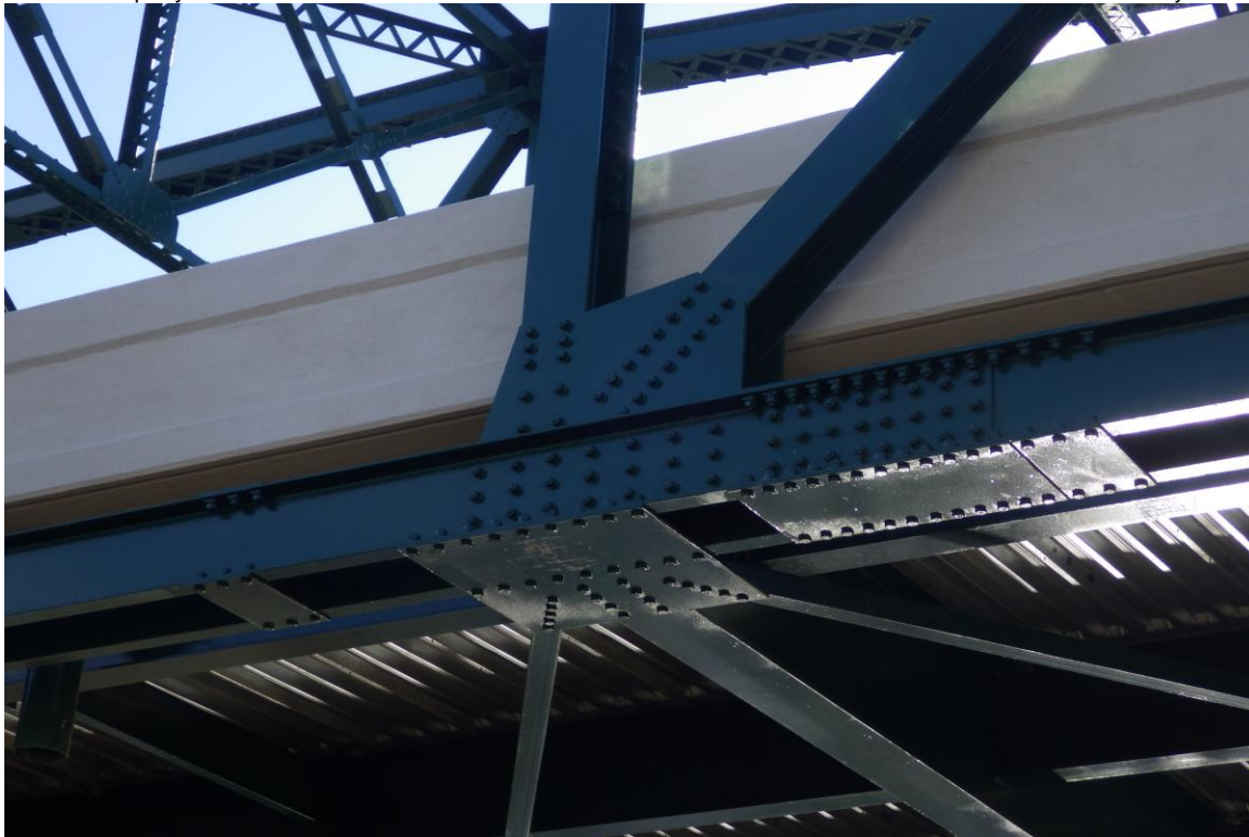
11. Connection at Post to Bottom Chord of The Capon Bridge, detail.
