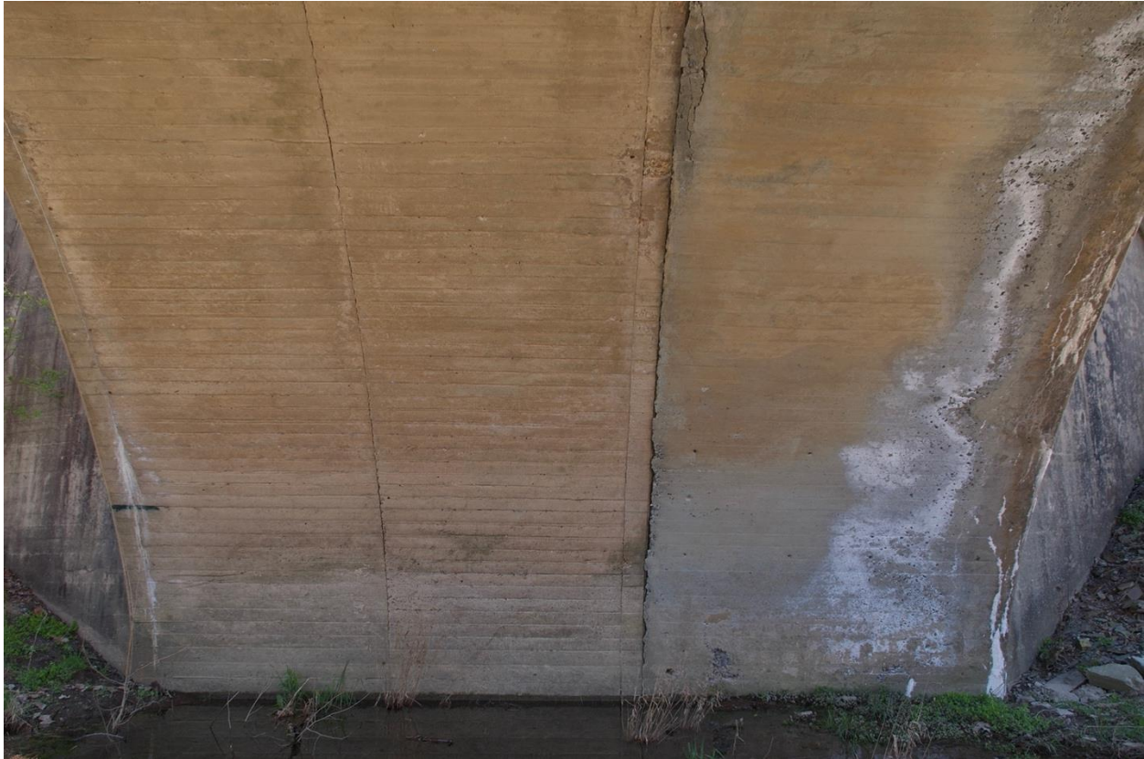
Photo 6. Underside showing form marks of phases (1916 on left, 1935 on right)
