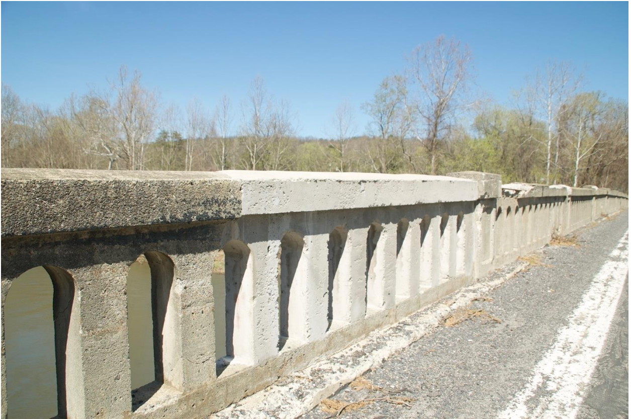
Photo 8. Balustrade detail showing repair
