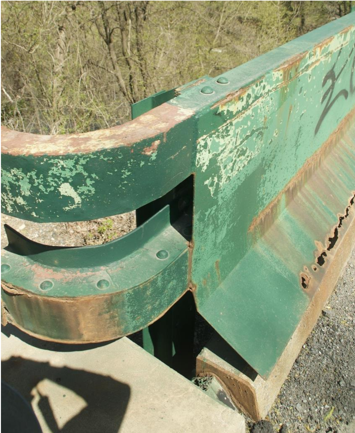
Photo 8. Original riveted guardrail detail with later welded metal plate
