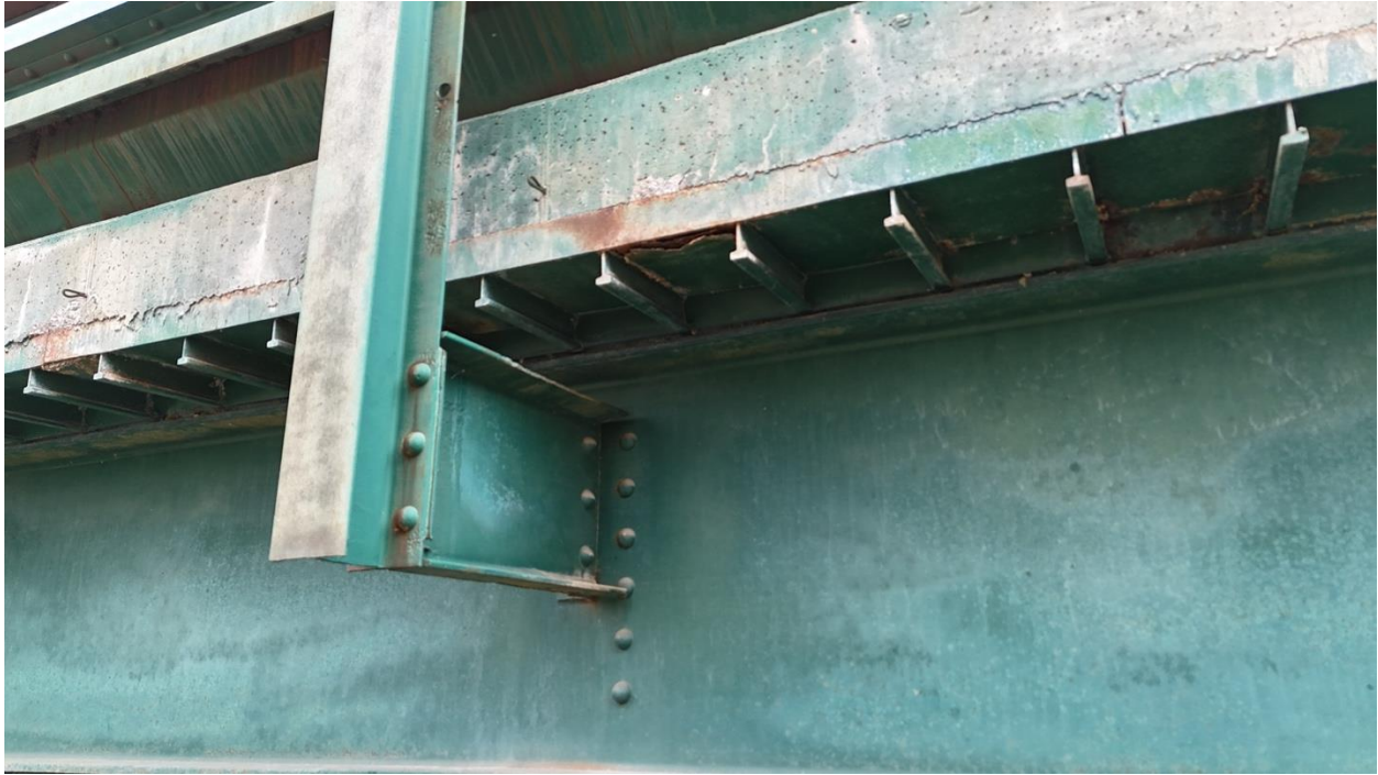
Photo 9. Connection detail showing cantilevered road deck and support strut
