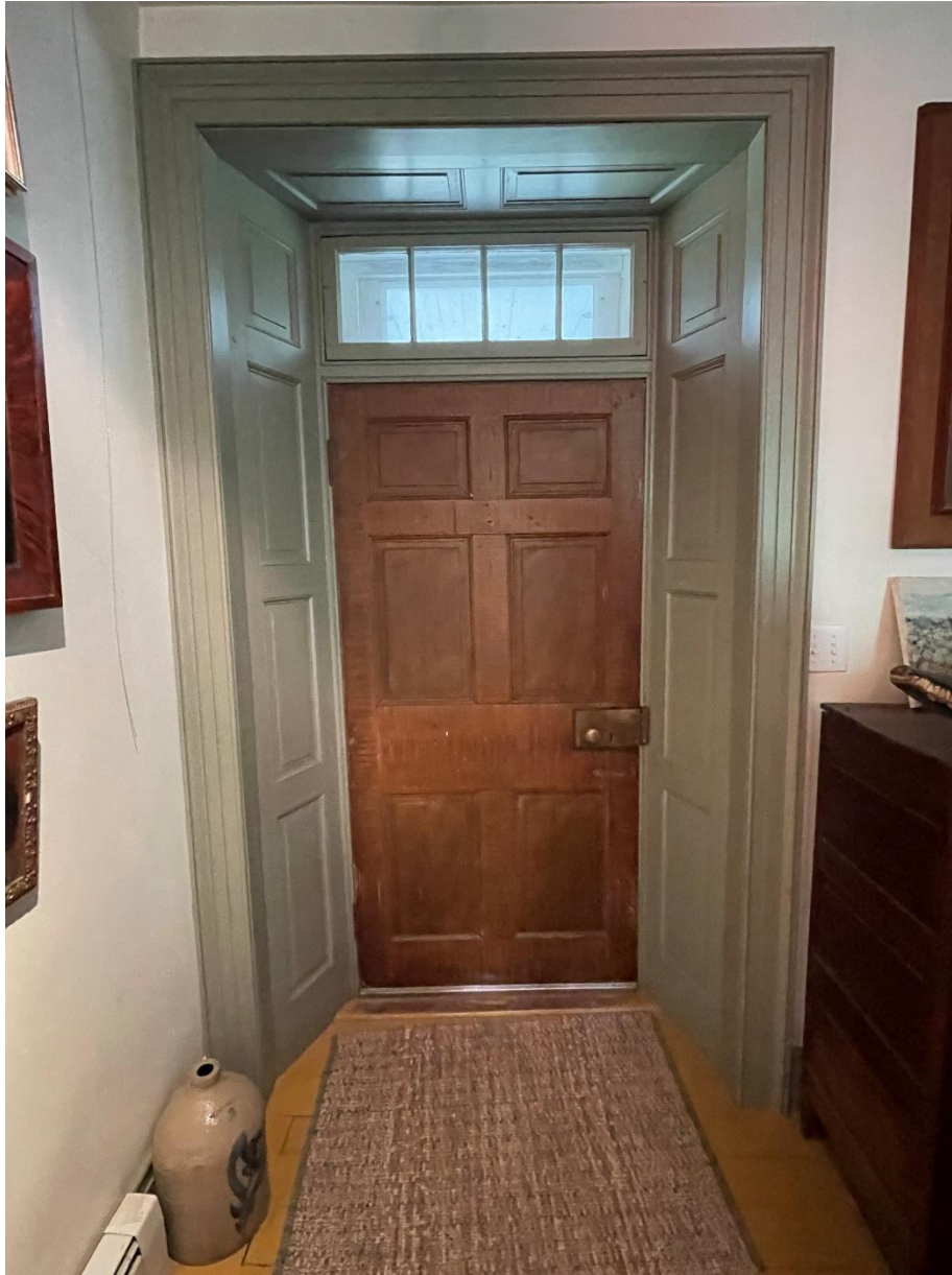
Photo 12. WV_Jefferson_County_Isaac Clymer Farm_012 Issac Clymer House first floor hall. South door with grain-painting. View south.
