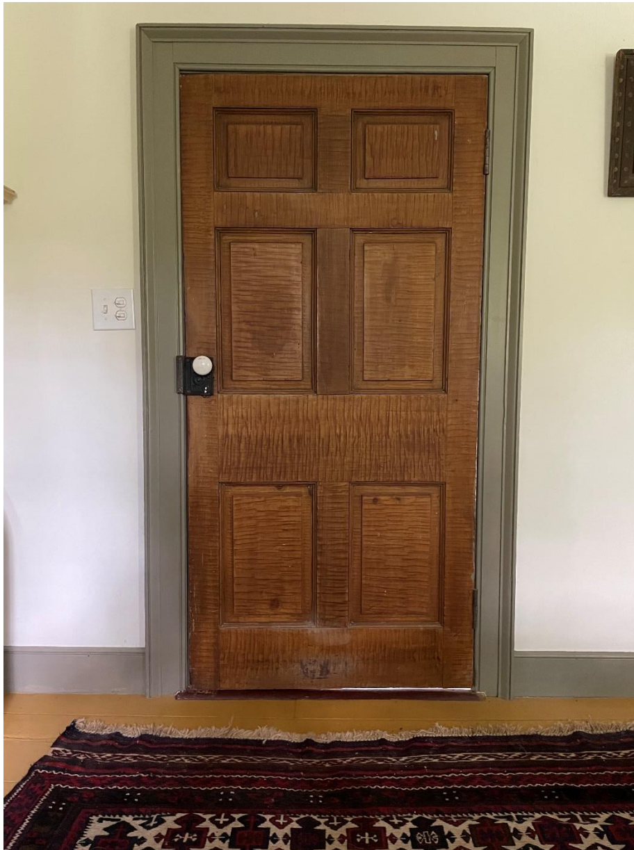
Photo 13. WV_Jefferson_County_Isaac Clymer Farm_013 Issac Clymer House second floor center bedroom. Grain-painted door. View north.
