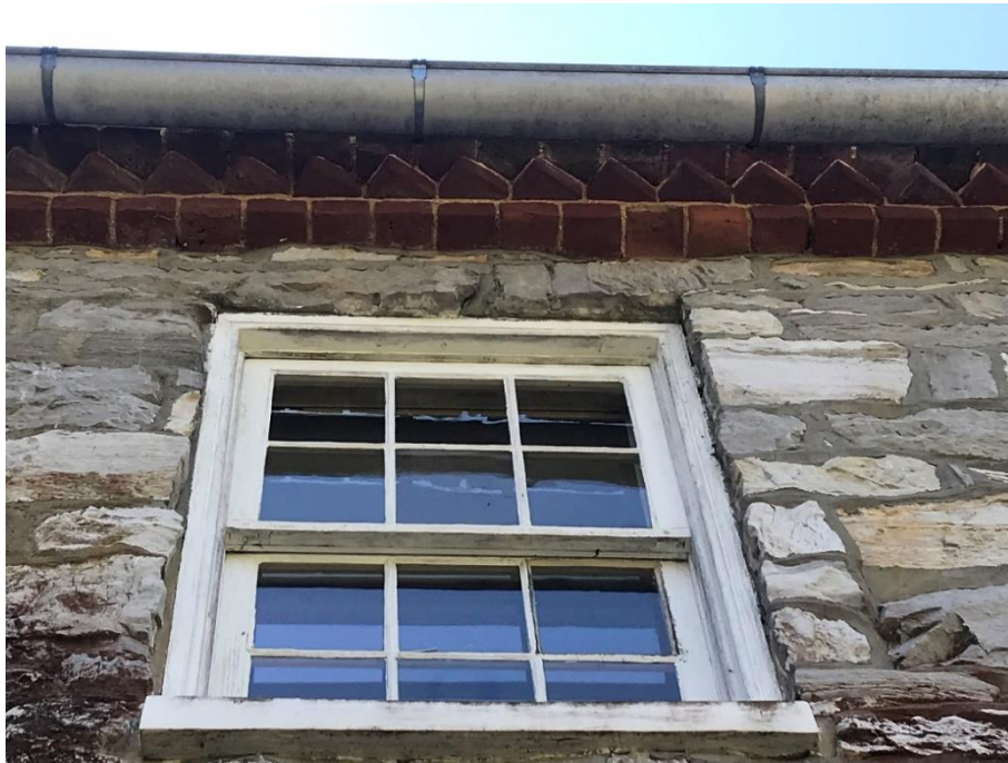
Photo 7. WV_Jefferson_County_Isaac Clymer Farm_007 Corbelled brick soffit on north façade. View south.
