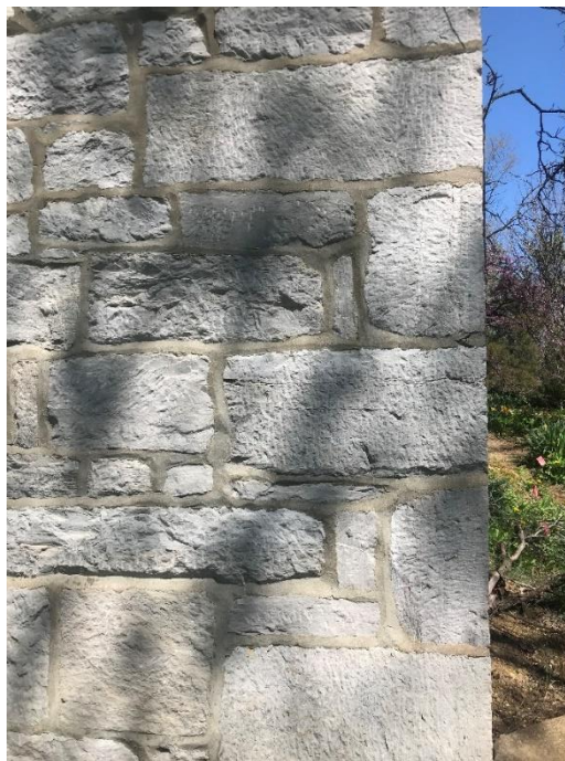
Photo 8. WV_Jefferson_County_Isaac Clymer Farm_008 Southeast corner of Isaac Clymer House showing large dressed limestone quoins. View north.
