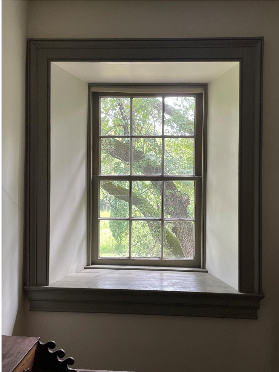
Photo 18. WV_Jefferson_County_Isaac Clymer Farm_018 Isaac Clymer House second floor center bedroom. Plastered window well. View southeast.
