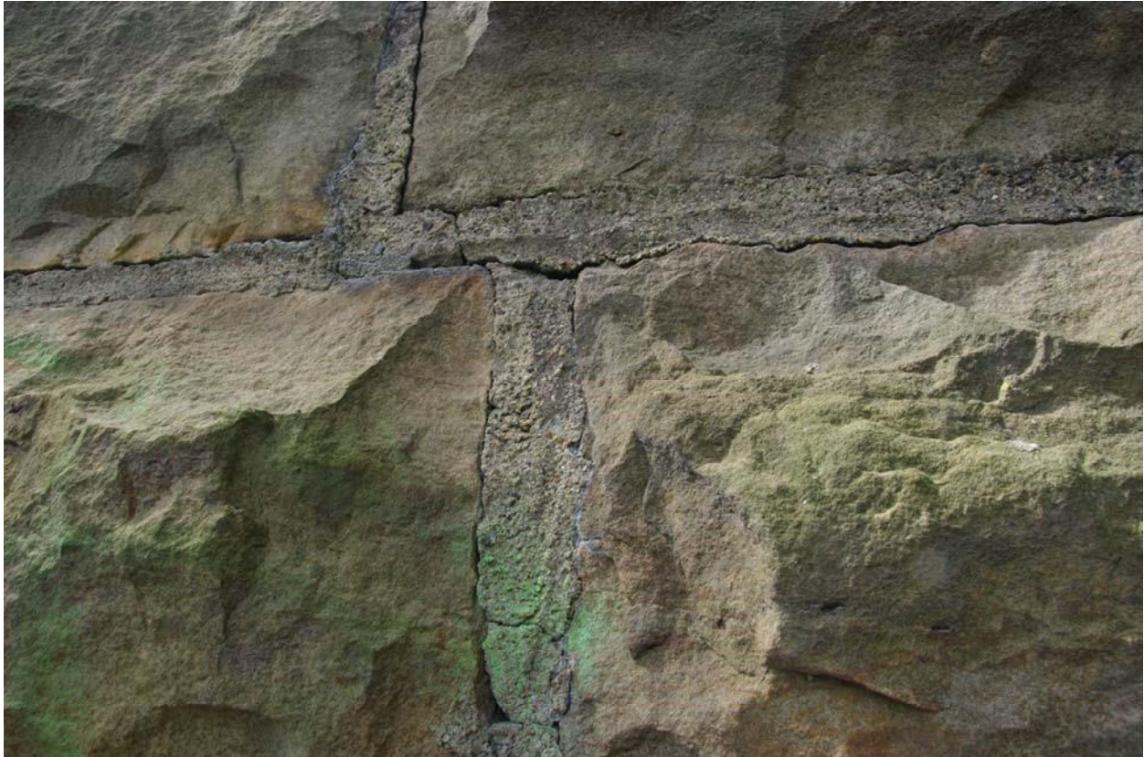
Photo#15. Detail of Richwood Ave Wall mortar and joints
