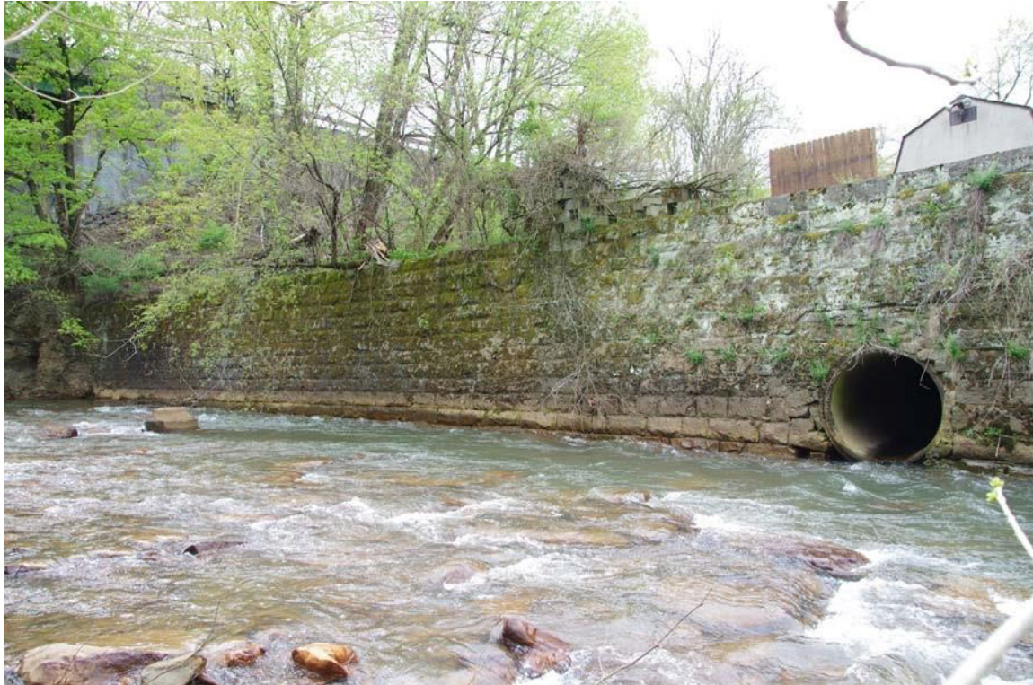
Photo#5. Large circular culvert at bottom of stone wall facing southeast
