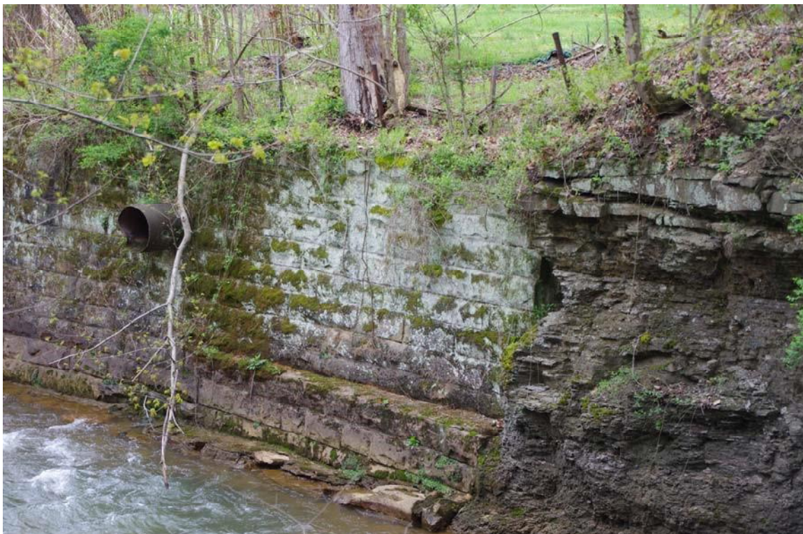
Photo#8. Detail of wall intercepting east abutment of overpass
