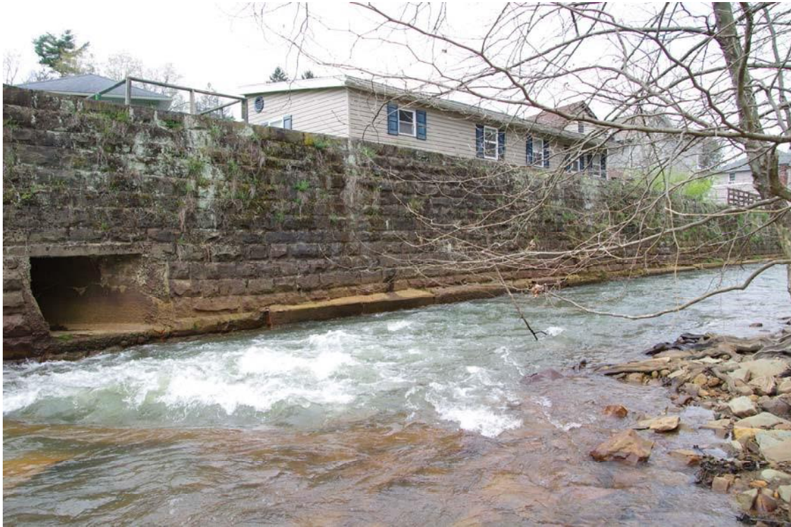
Photo#4. Large rectangular culvert at bottom of stone wall facing southwest
