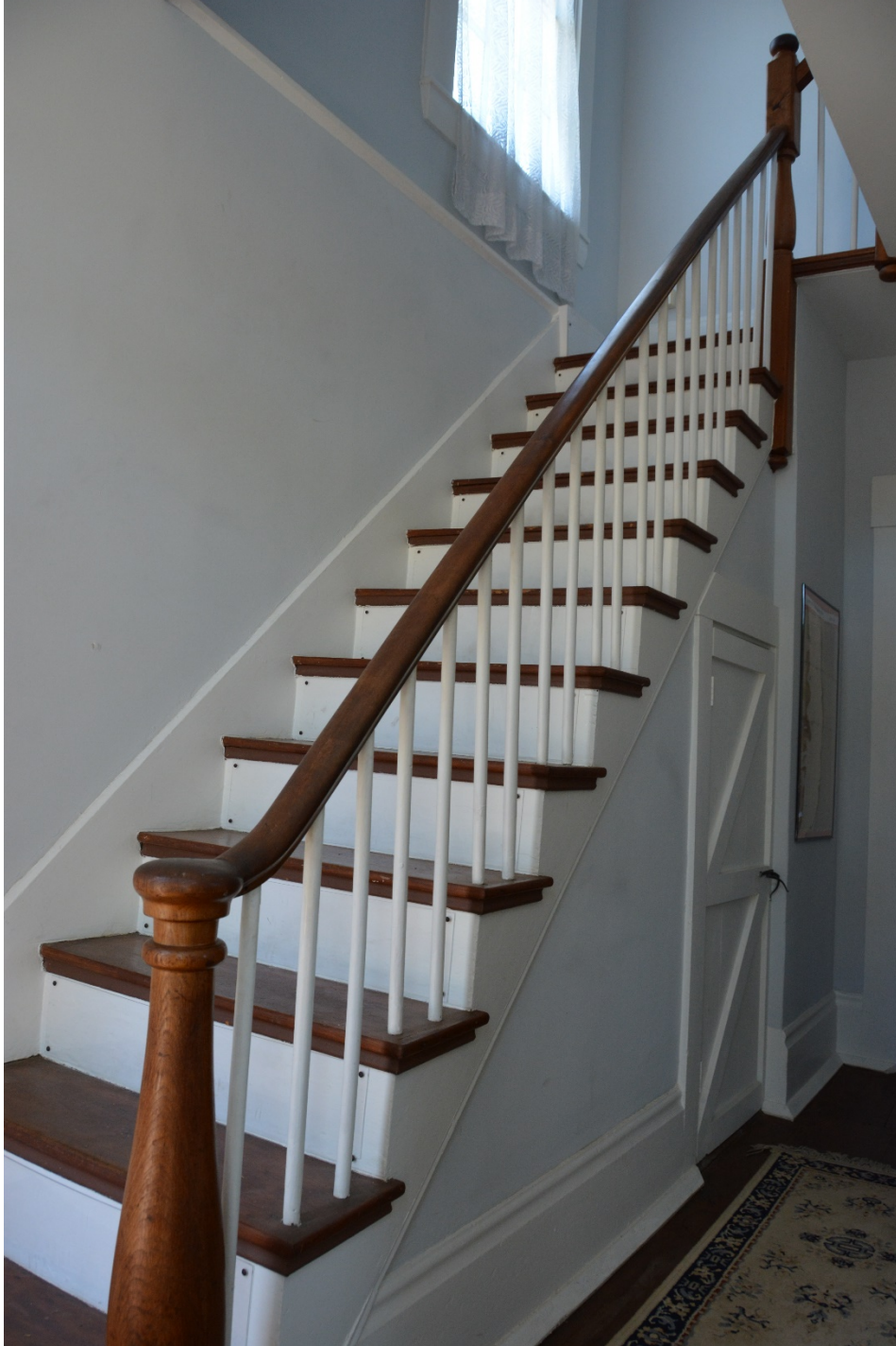
Photo 12 Interior, first floor staircase, southeast elevation
