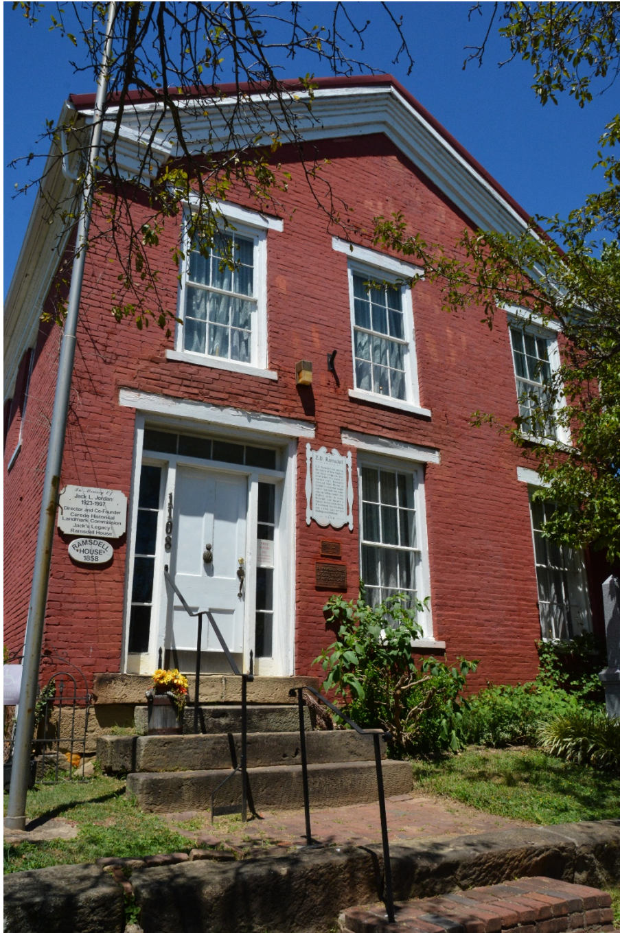
Photo 1 Front of house, southwest elevation
