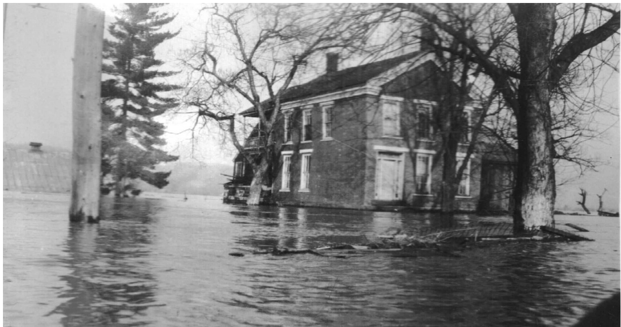
Figure 2 Ramsdell House during the Flood of 1937
