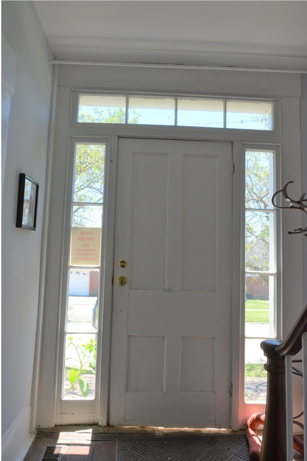
Photo 13 Interior, front door, north elevation
