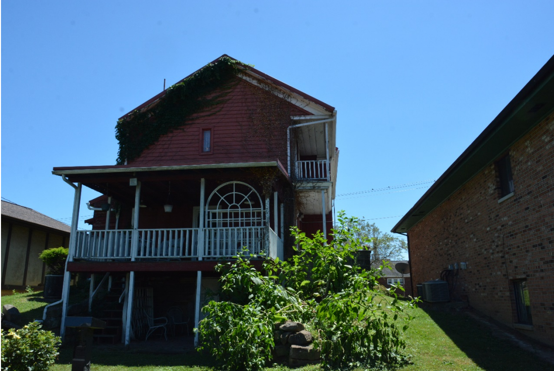
Photo 5 Rear of house, north elevation
