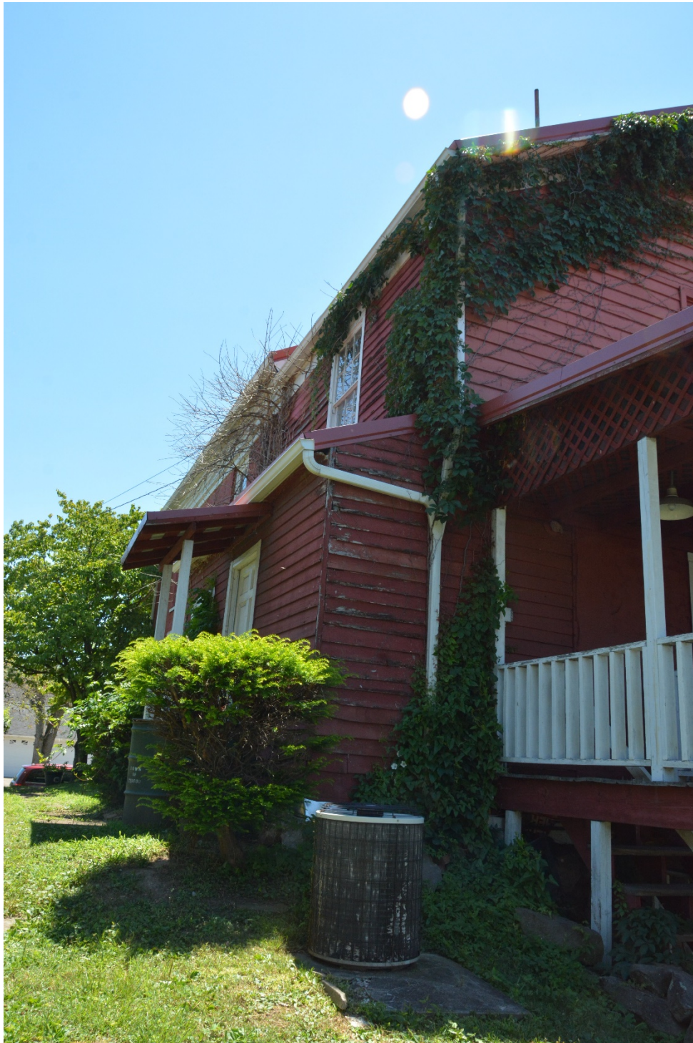
Photo 8 East side of house with kitchenette exterior, northeast elevation
