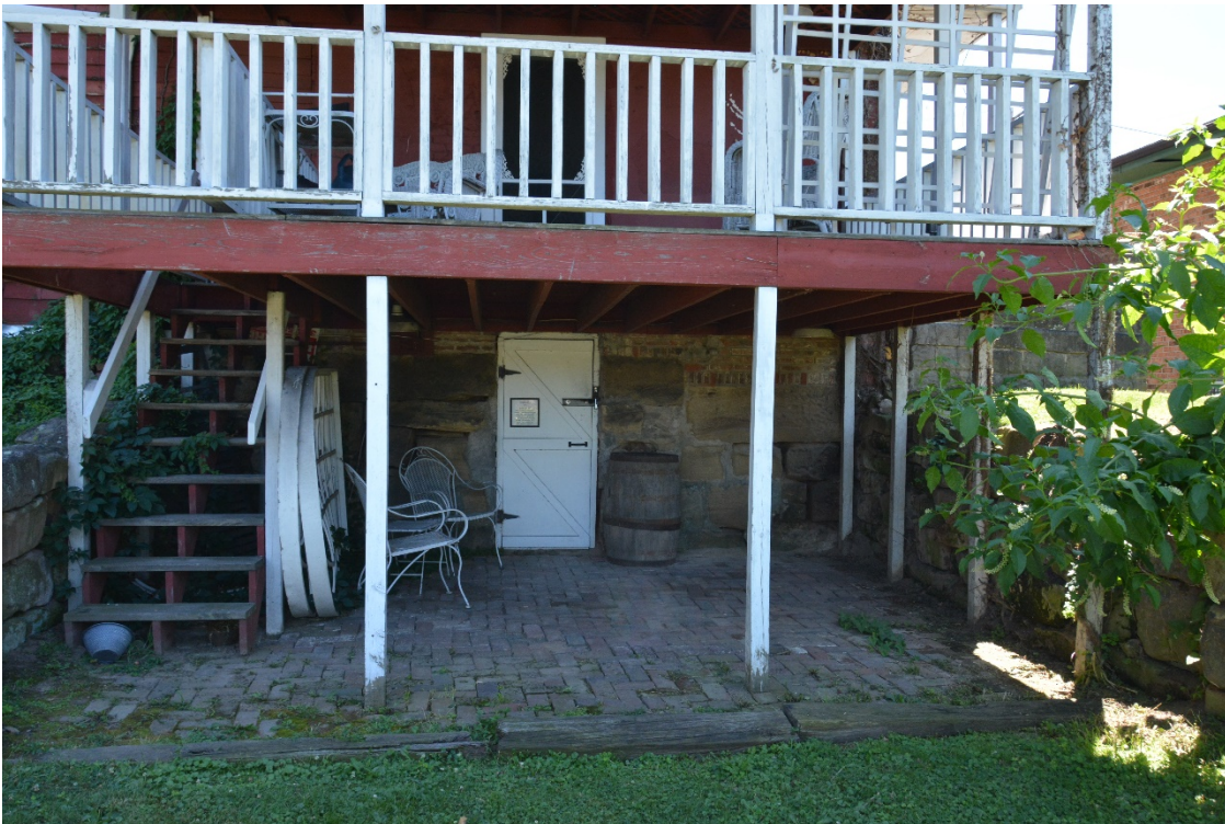
Photo 6 Cellar door beneath rear porch, north elevation
