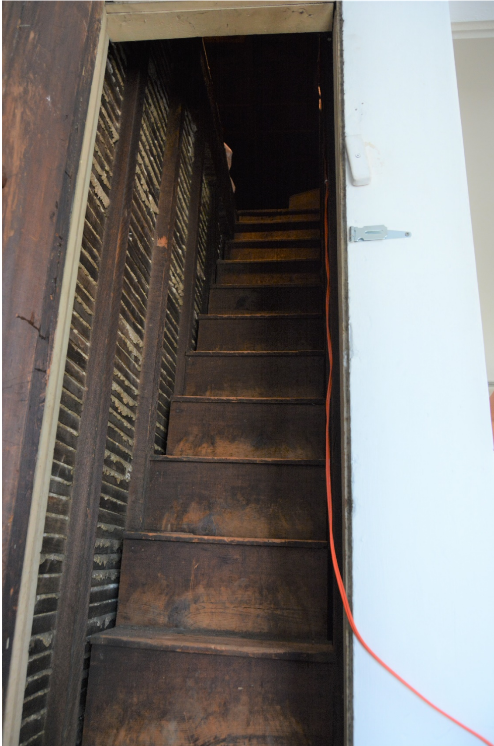
Photo 20 Interior, second floor, stairs to attic, west elevation
