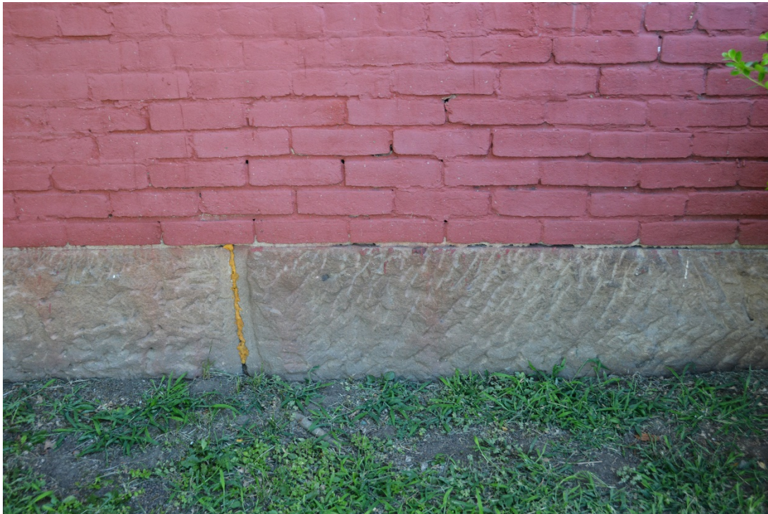
Photo 10 Sandstone foundation, east elevation
