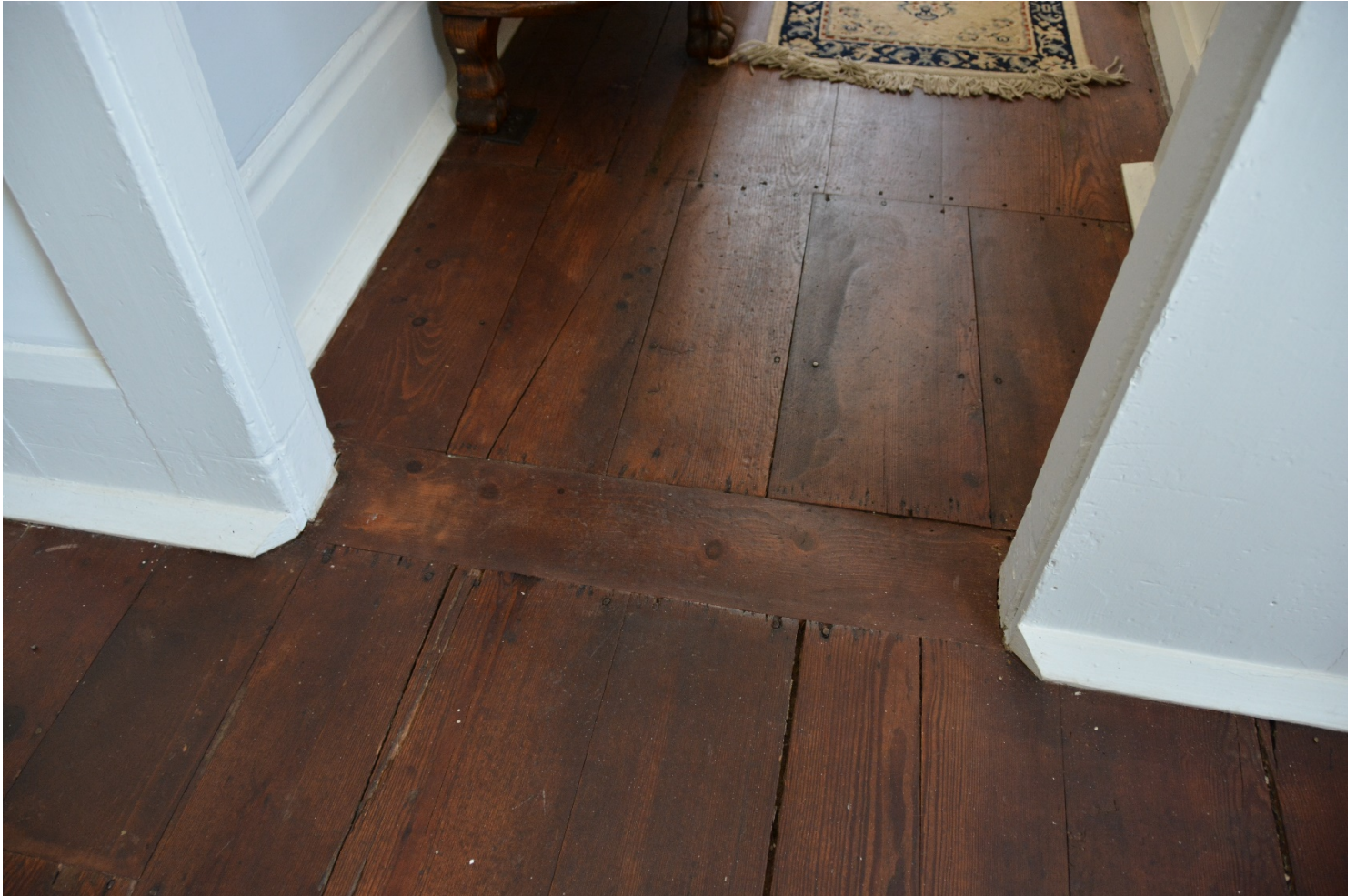
Photo 18 Interior, first floor, wood flooring between Foyer and Room 3, north elevation
