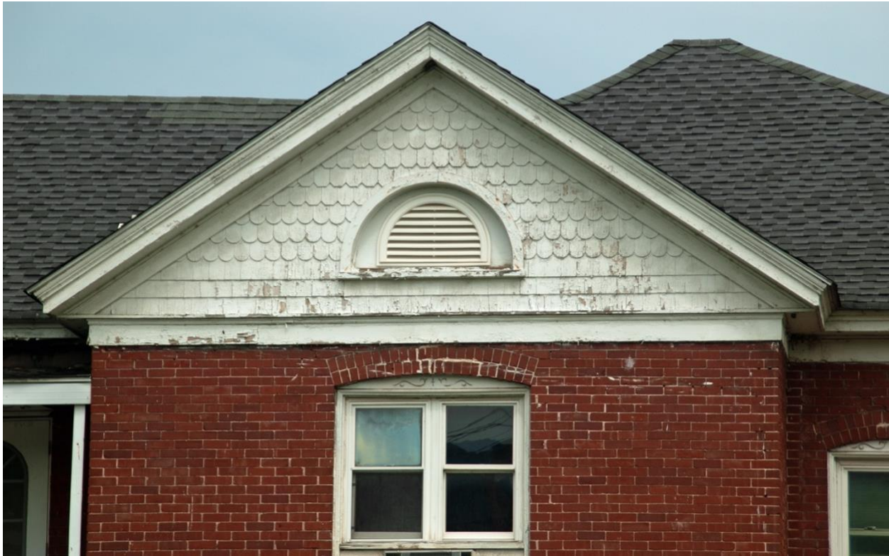
Photo 6. Detail of Gable End, South Elevation
