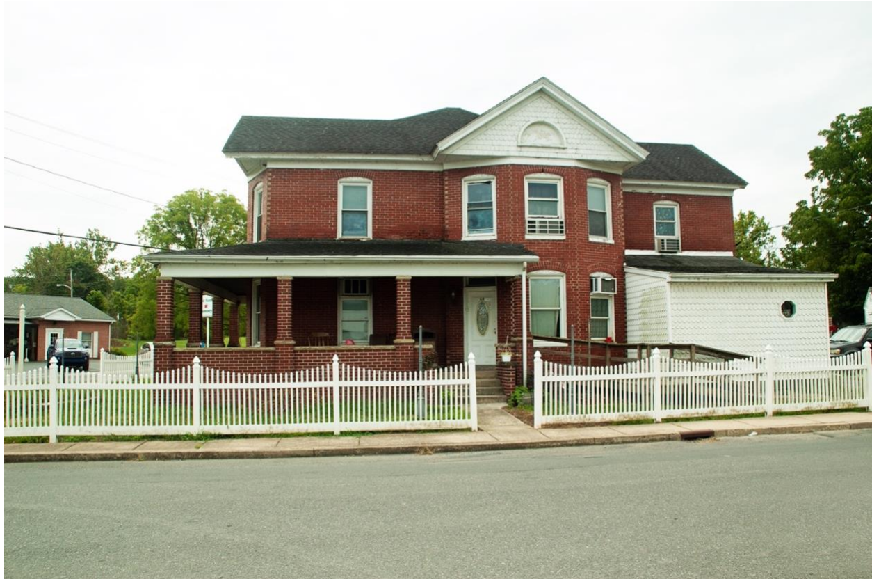
Photo 3. Lee Street Elevation, Facing South
