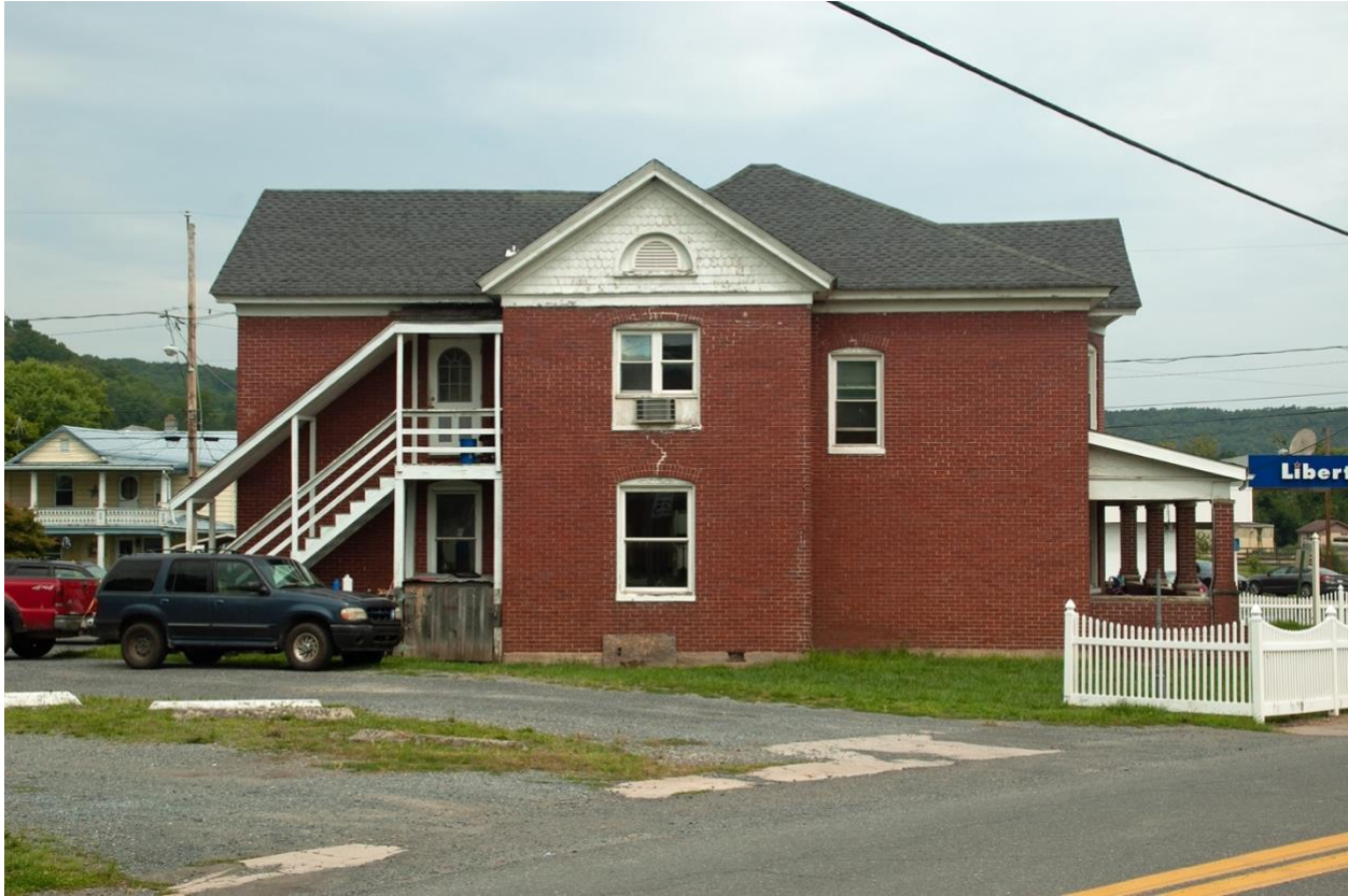
Photo 5. South Elevation Facing North
