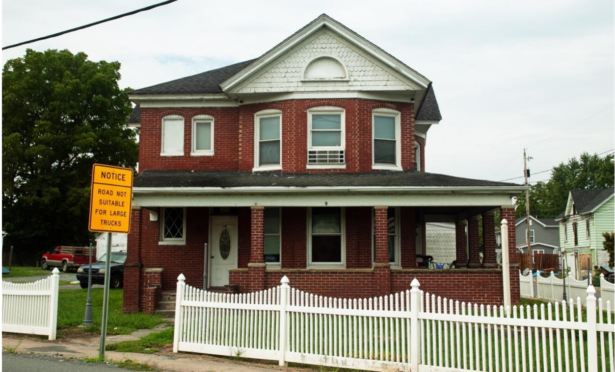
Photo 1. Winchester Street (Main) Elevation, Facing West
