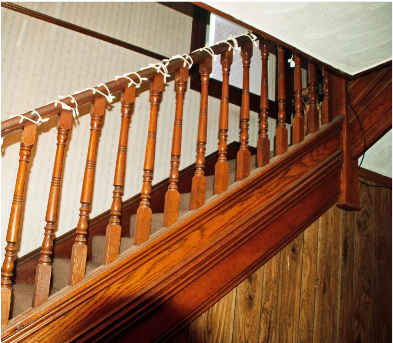
Photo 10. Main Stair Balustrade
