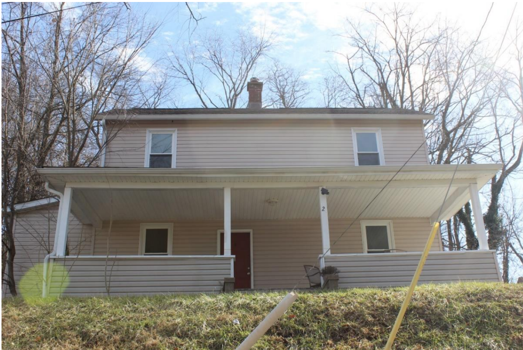
Photo 2: Front View of the Jeannette O. Parker Tourist Home at 2 Cayton Street, camera facing east.
