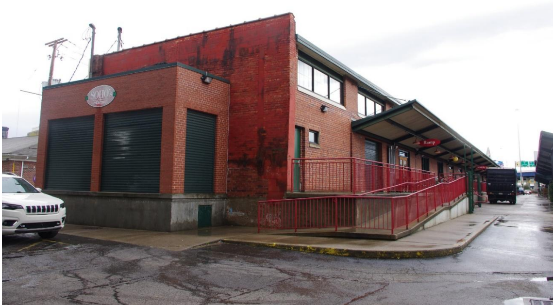
Photo 5. Northeast and southeast elevations, camera facing NW.
