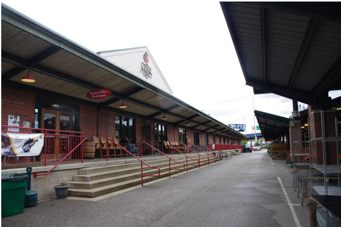
Photo 4. Northeast elevation, camera facing W.
