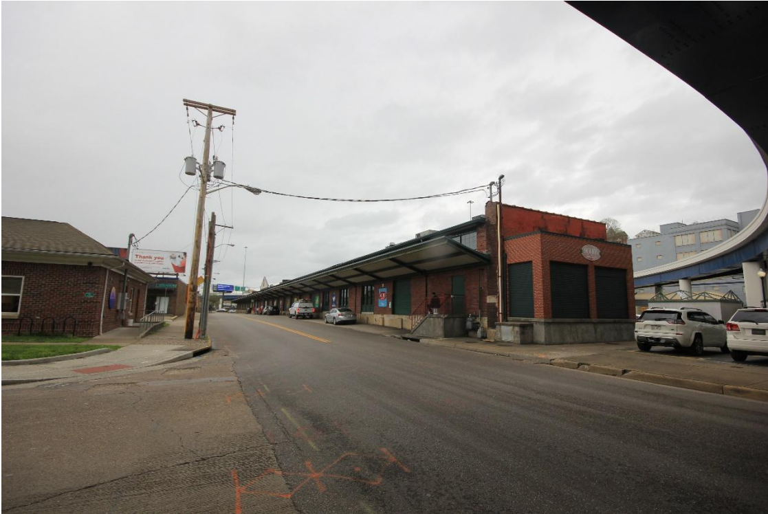
Photo 3. View of southwest (Smith Street) and southeast elevations with interstate ramp at right, camera facing N.
