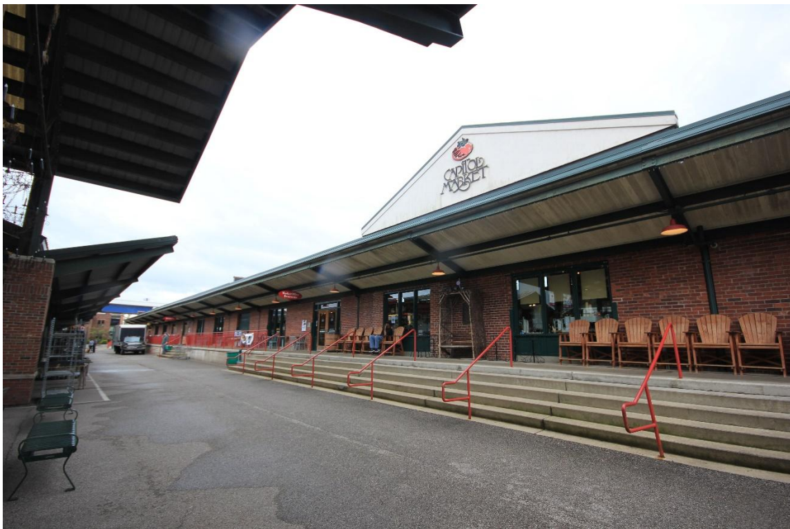
Photo 2. View of northeast elevation, central bays, camera facing SE.
