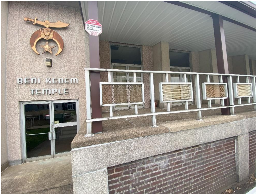
Photo 6: West elevation entrance and terrace railing, camera facing East.
