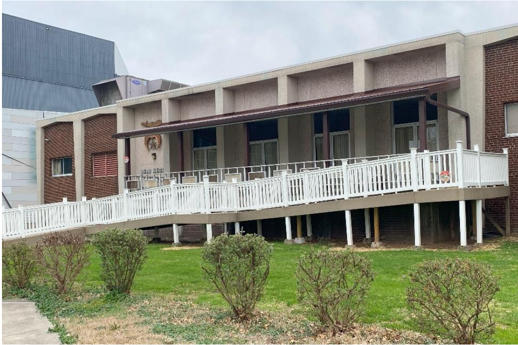
Photo 5: West elevation terrace, camera facing East.
