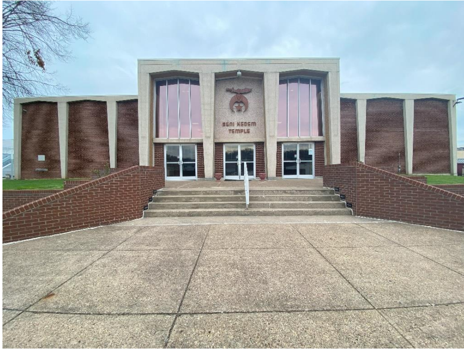
Photo 1: South elevation, camera facing North.
