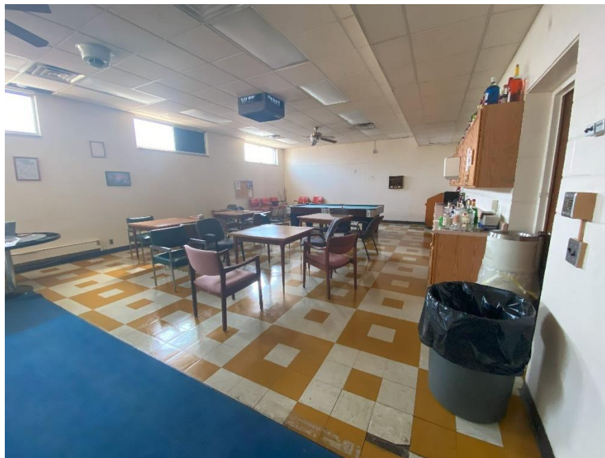
Photo 22: Card room with original two-color floor tiles, camera facing Southeast.
