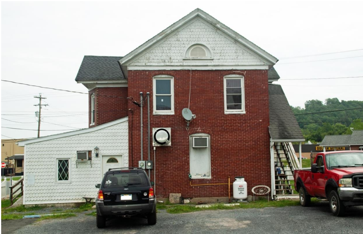
Photo 4. West Elevation, Facing East
