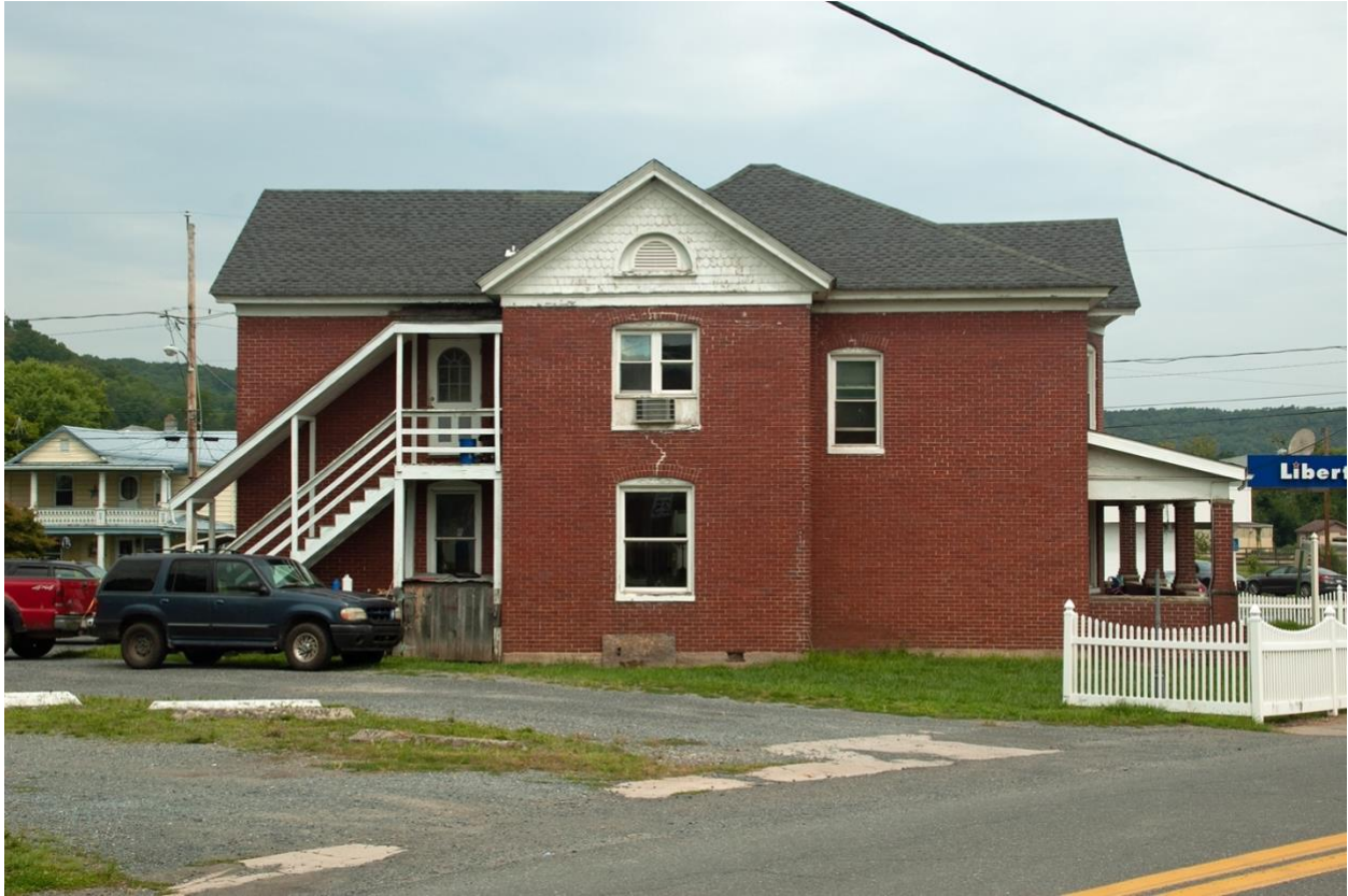
Photo 5. South Elevation Facing North
