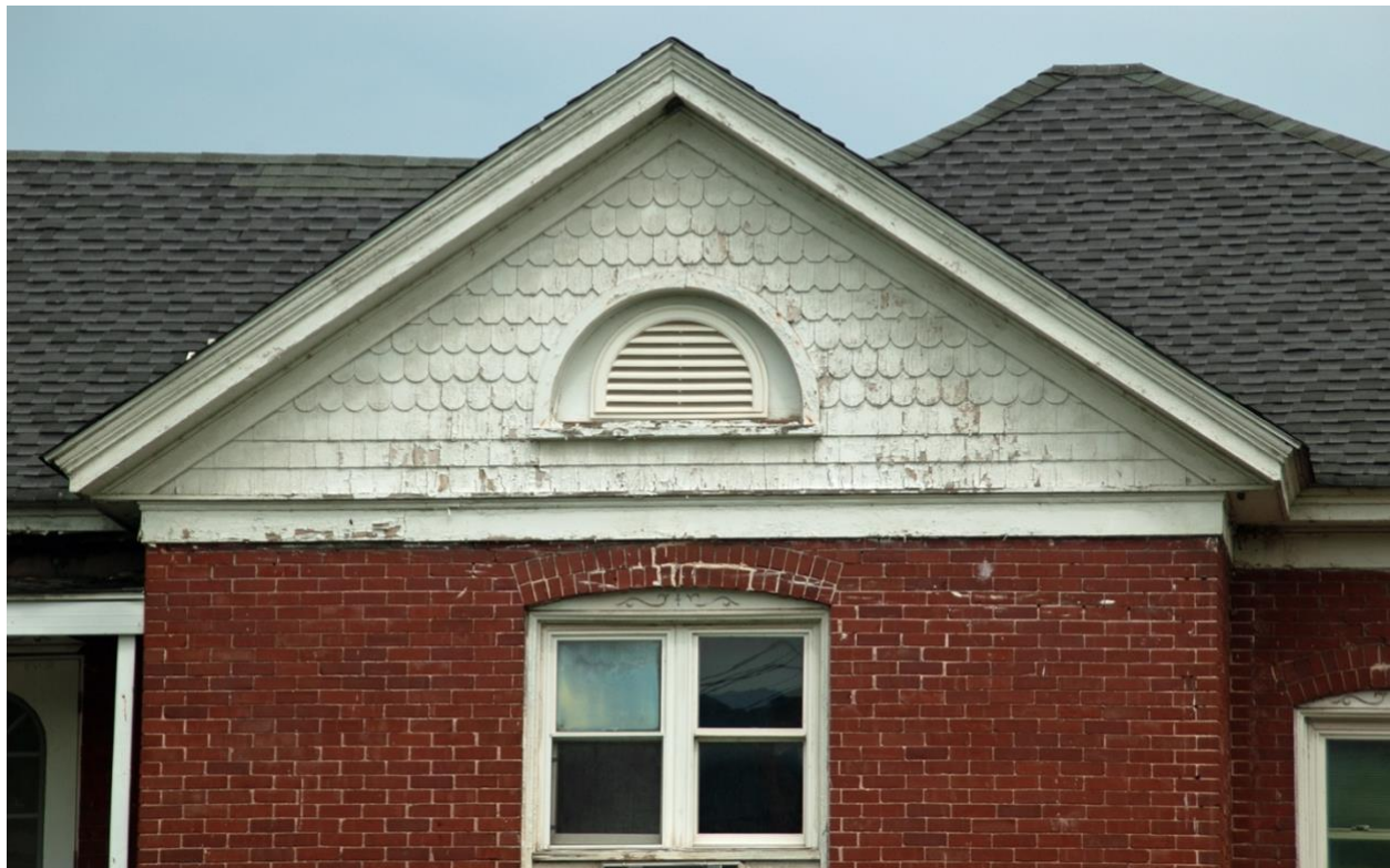
Photo 6. Detail of Gable End, South Elevation
