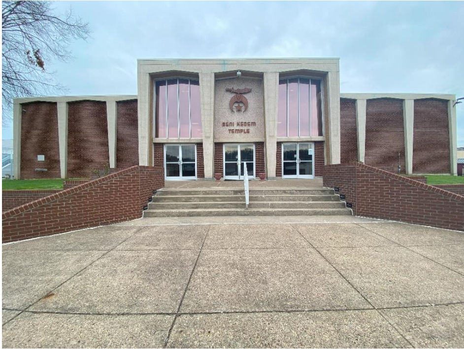
Photo 1: South elevation, camera facing North.
