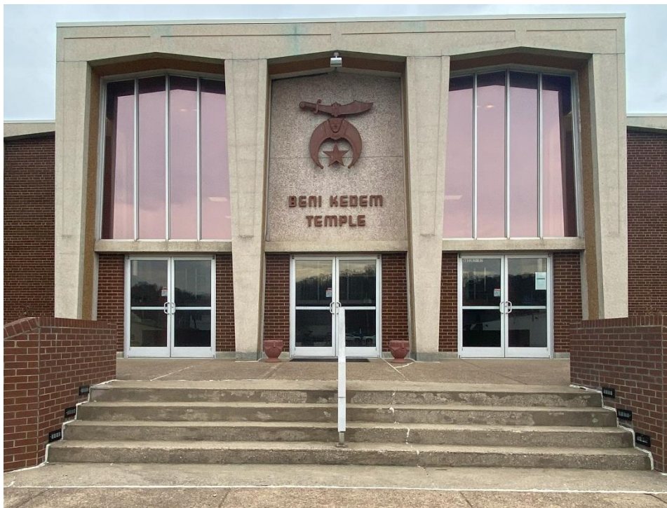
Photo 2: South entrance, camera facing North.
