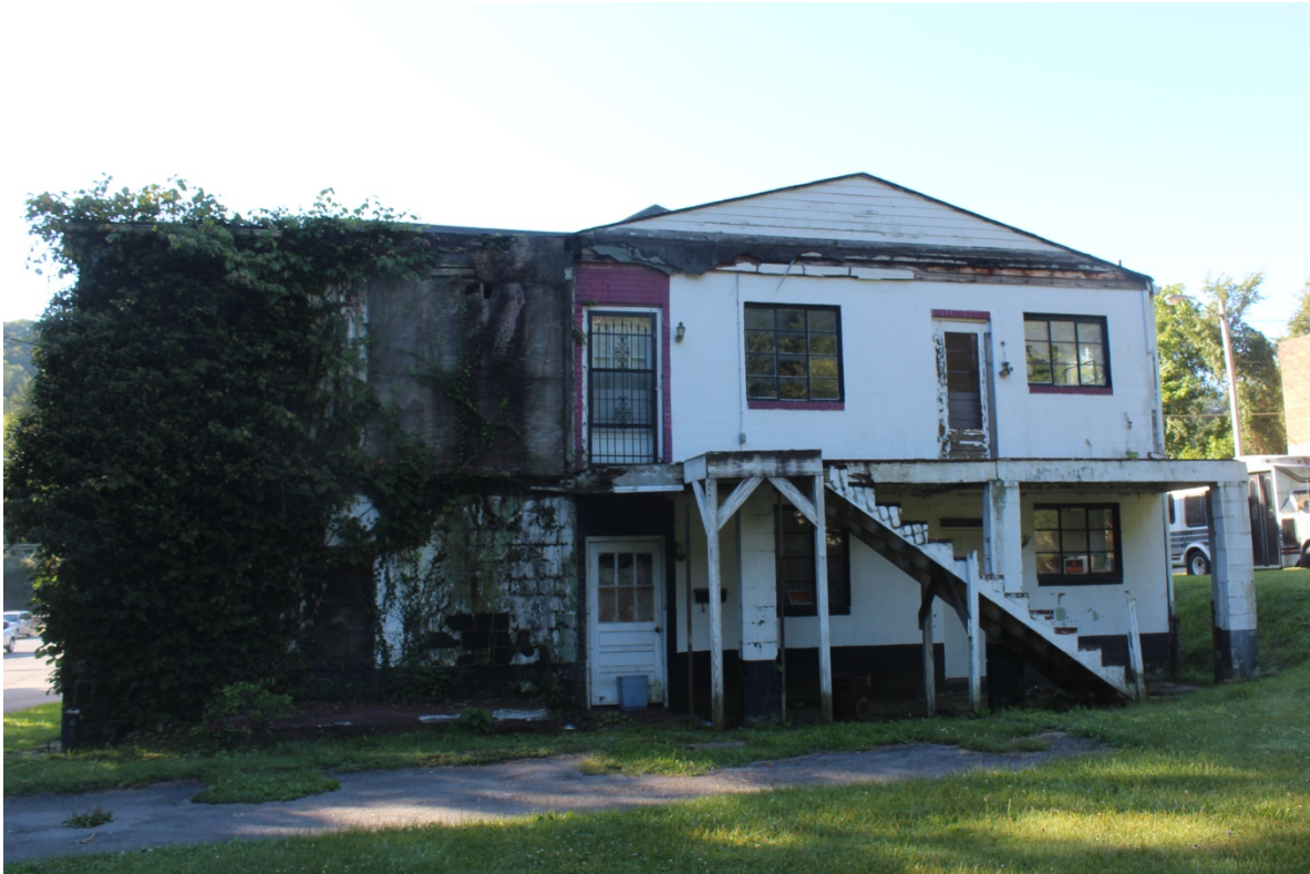
Photo 5: Rear (north) elevation of Hotel Thelma, camera pointing south.
