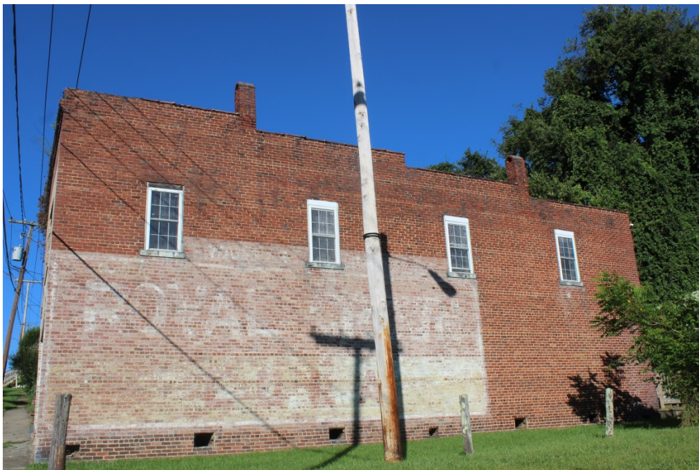
Photo 10: East elevation of Travelers Inn Hotel, camera pointing west.
