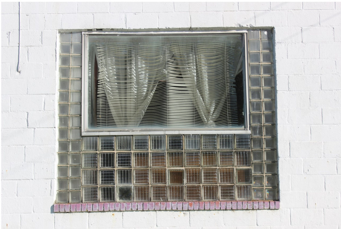
Photo 8: Hotel Thelma window on front elevation, camera pointing north.
