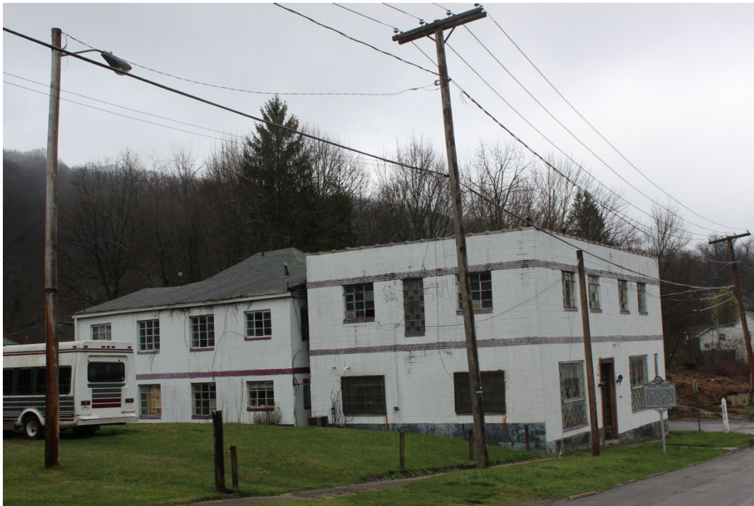
Photo 4: West elevation of Hotel Thelma, camera facing east.
