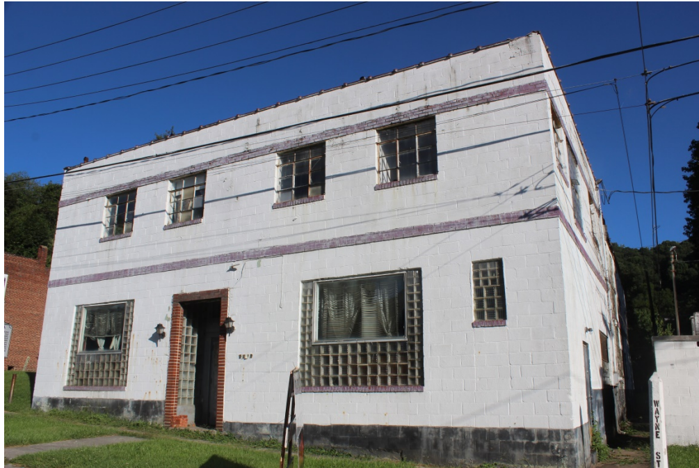
Photo 3: Front (south) elevation of Hotel Thelma, camera pointing northwest.
