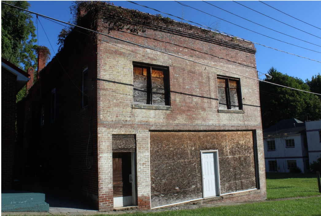
Photo 11: Oblique of Travelers Inn Hotel, camera pointing northeast.
