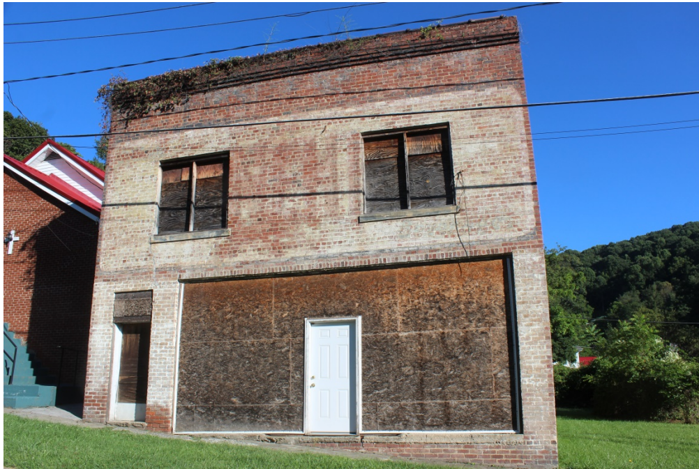
Photo 9: Front (south) elevation of Travelers Inn Hotel, camera facing north.
