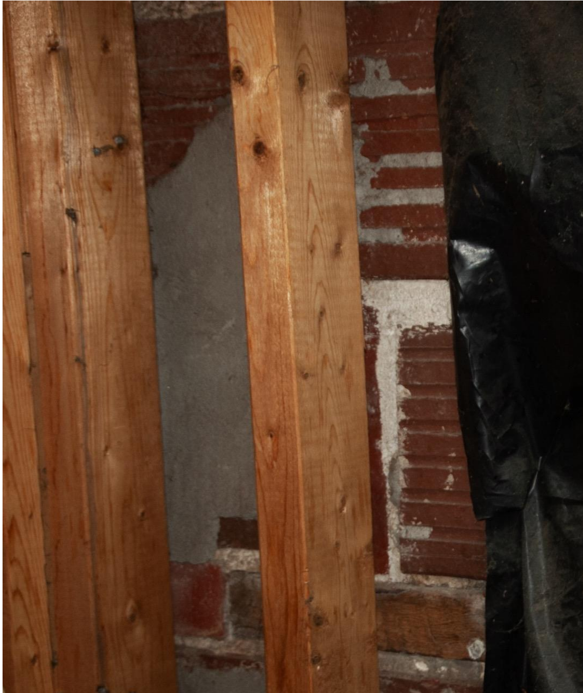
Photo 9. Section of Exposed Terracotta Structural block
