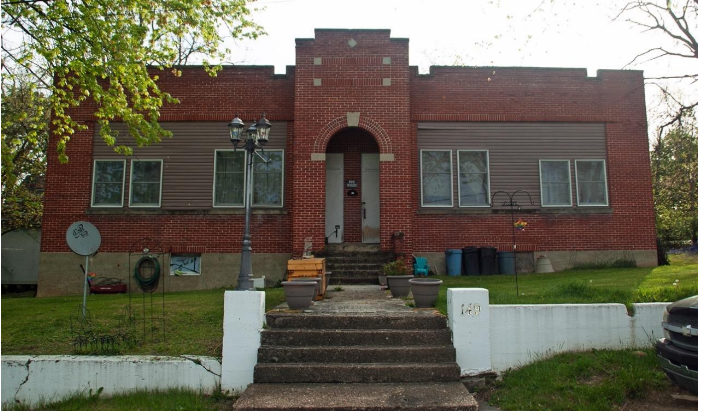
Photo 1. Main Elevation, Facing East
