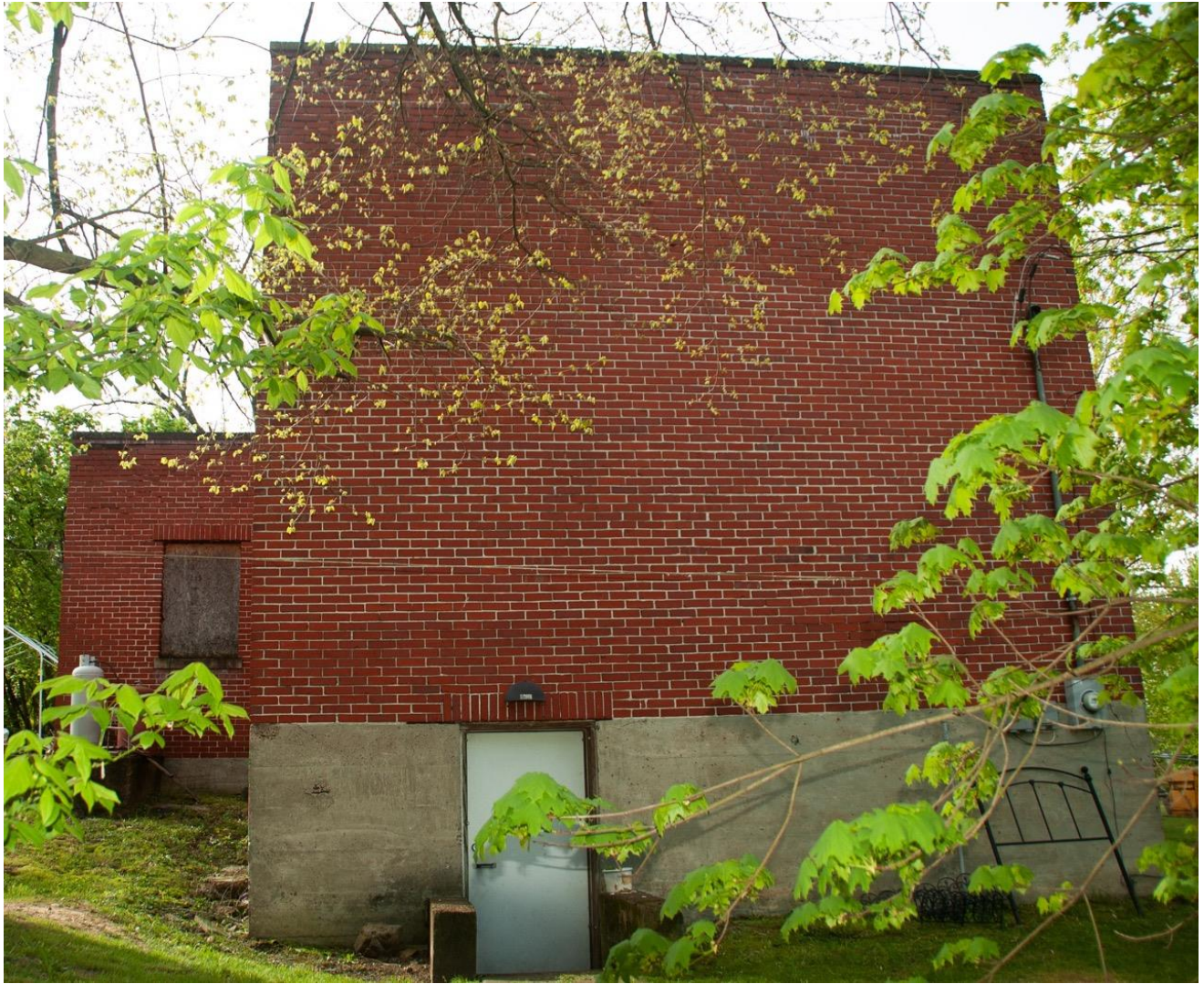
Photo 6. North Elevation, Facing South
