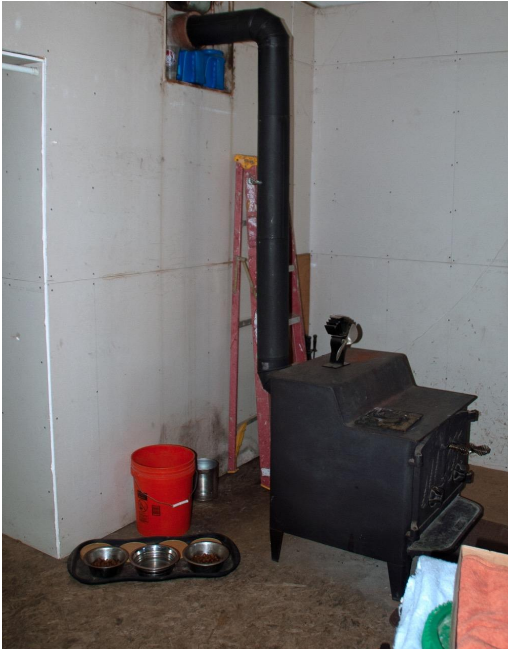
Photo 8. Main Interior Space showing location of woodburning stove
