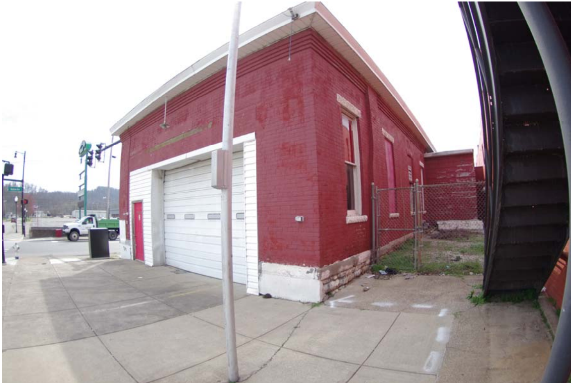
Photo 02 Site 005 looking southwest on 14th St. West.
