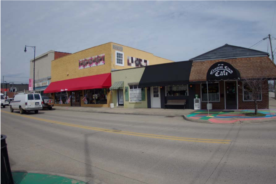
Photo 08 Looking northeast from 14th St. West and 5 Ave.
