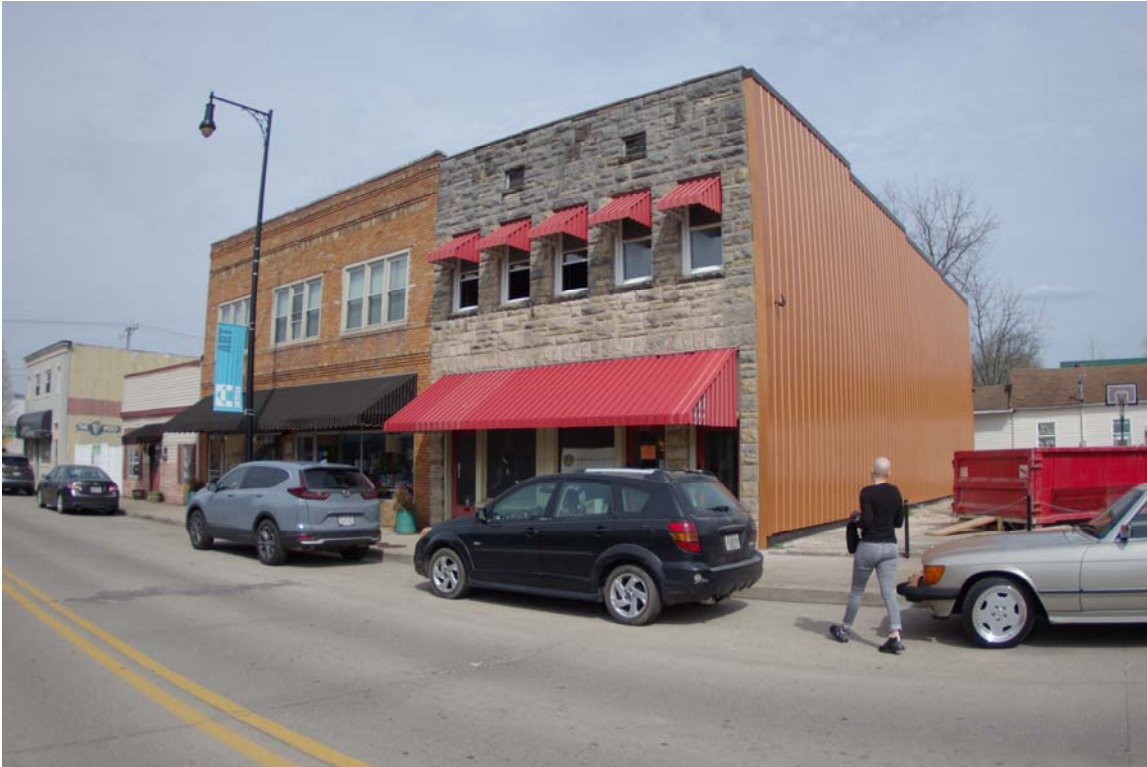
Photo 13 Looking northeast from corner of 14th St. West and Jefferson Ave. Sites 012, 013, 014.
