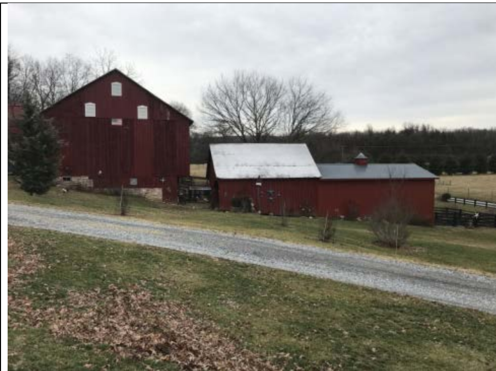
WV_Jefferson County_Woodbyrne_0008. Barn&silos, Corn Crib, Metal Shed, view to east.
