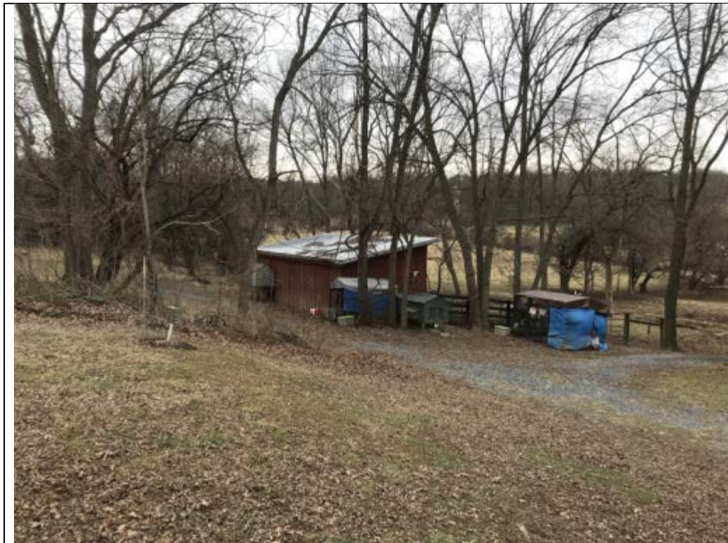
WV_Jefferson County_Woodbyrne_0011. Stable rear, view to southwest.
