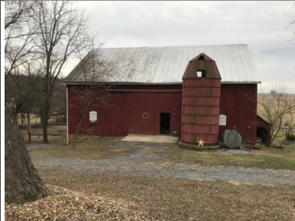
WV_Jefferson County_Woodbyrne_0007. Barn and silo, front façade, view to south.
