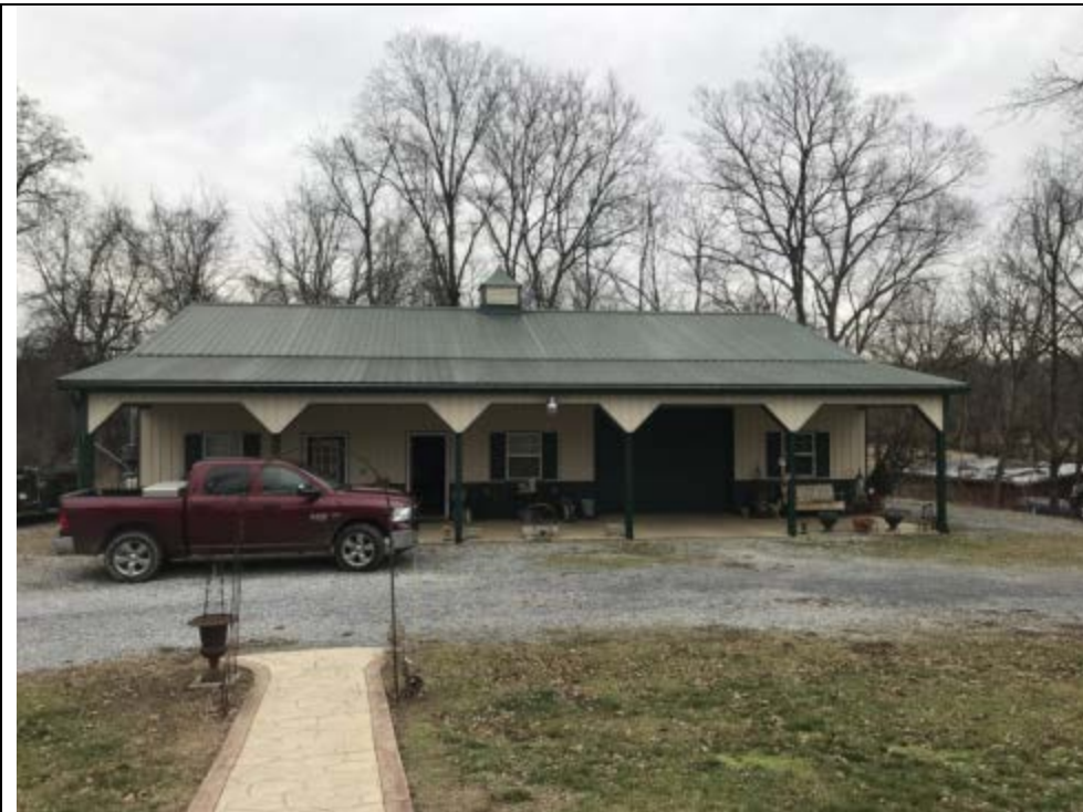
WV_Jefferson County_Woodbyrne_0006. Garage, work shed, front façade, view to east.
