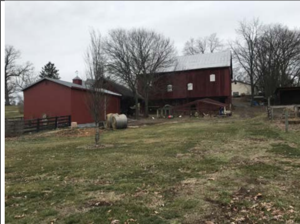
WV_Jefferson County_Woodbyrne_0009. Barn forebay and stock yard, view to north.
