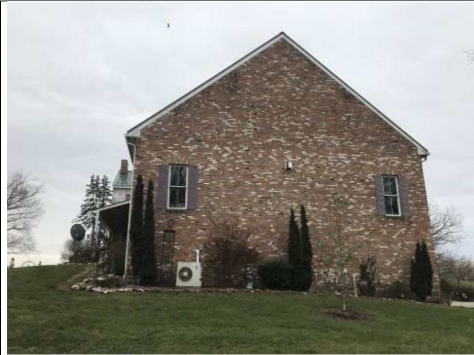
WV_Jefferson County_Woodbyrne_0003. Woodbyrne house, north façade, view to south.
