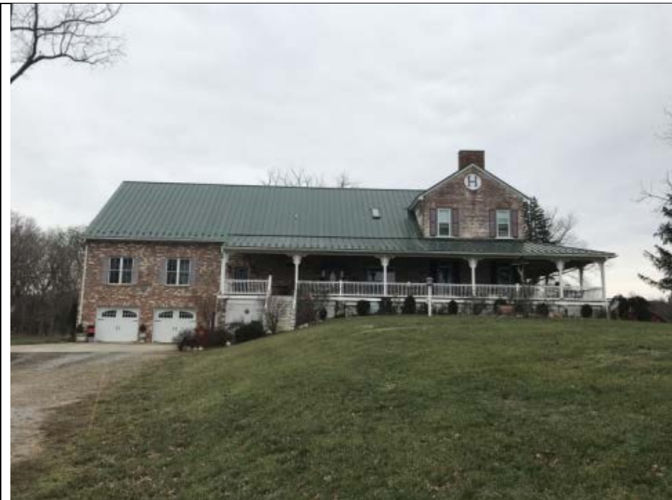
WV_Jefferson County_Woodbyrne_0004. Woodbyrne house, west façade, view to east.
