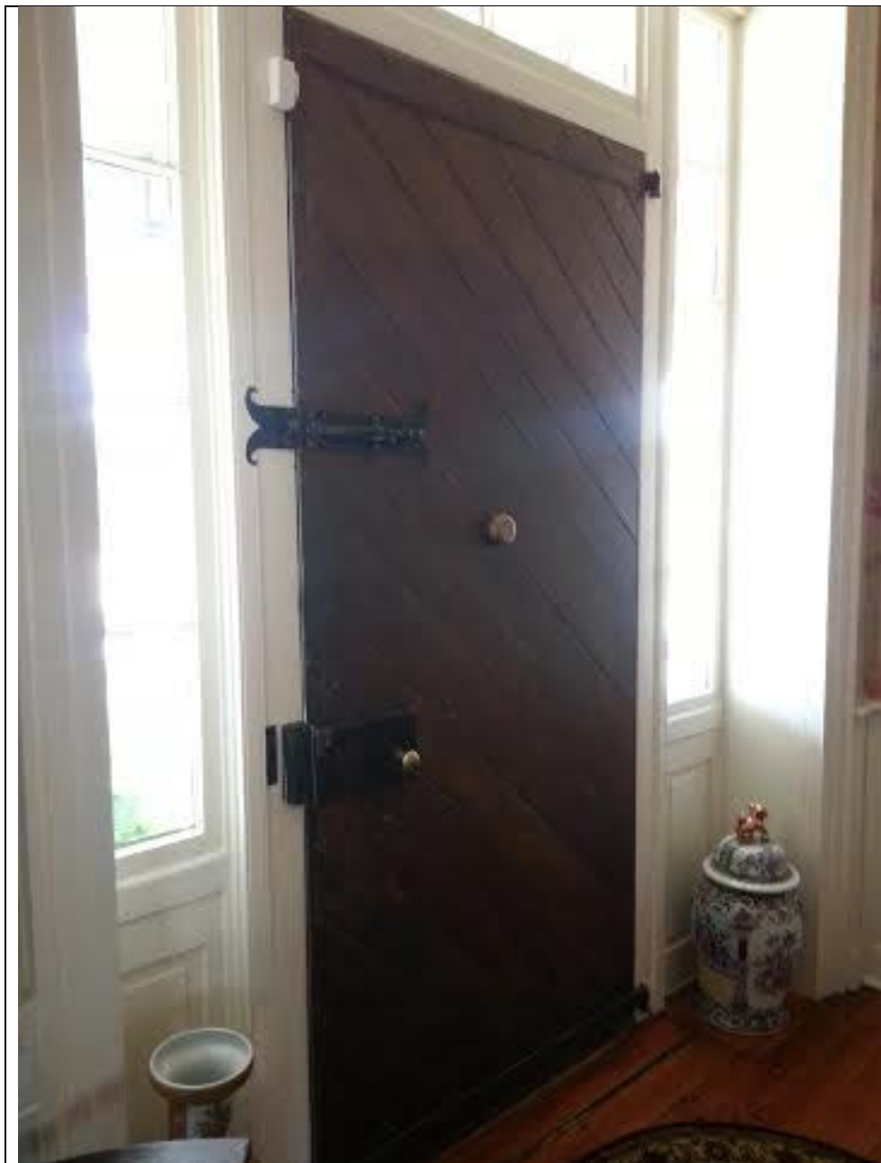
Fig. 17. Diagonally-braced door at main entry (front door). Built for strength and security, the door contains its original box lock.
