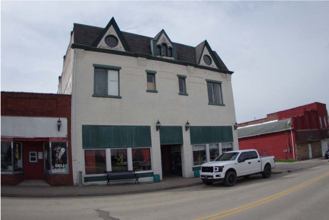
Photo 11 Site 008 looking west on 14th St. West.
