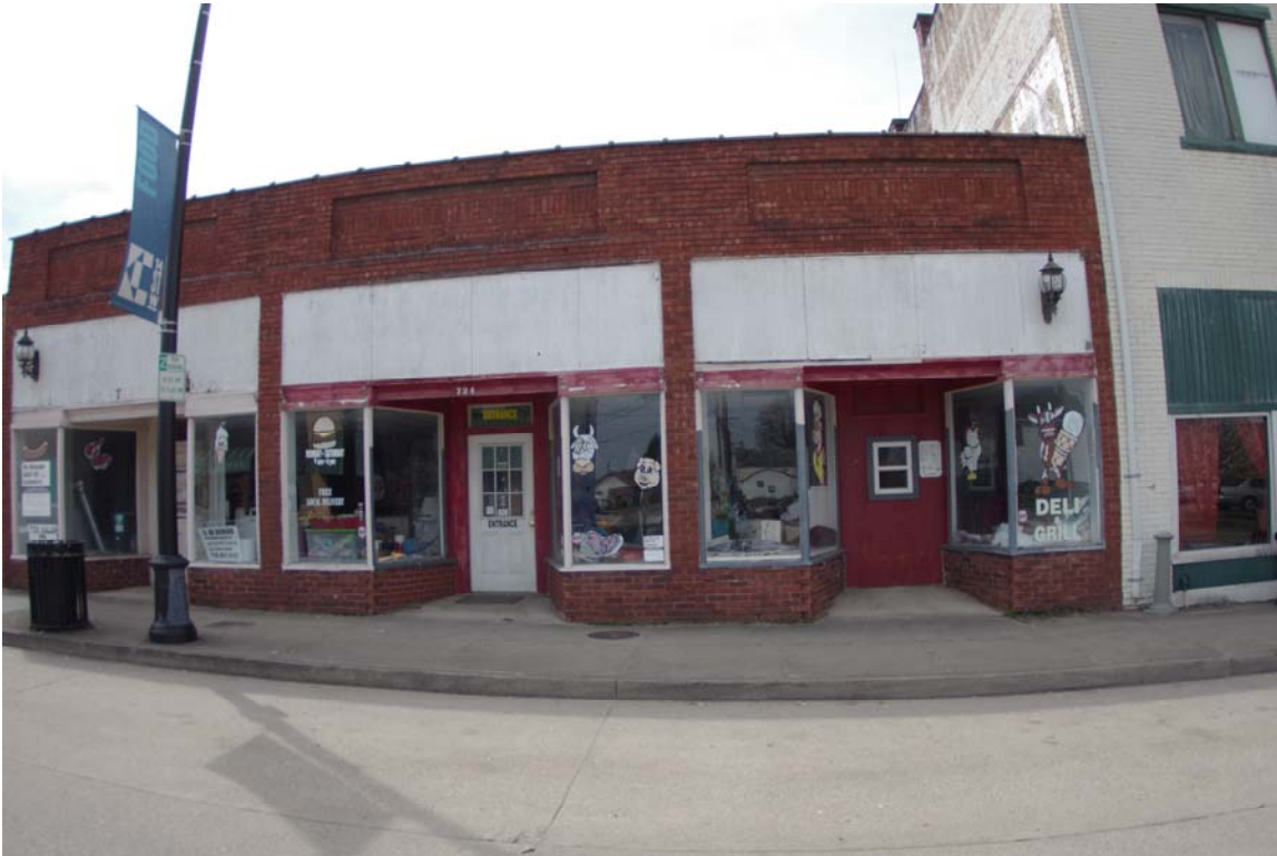
Photo 10 Site 007 looking west on 14th St. West.
