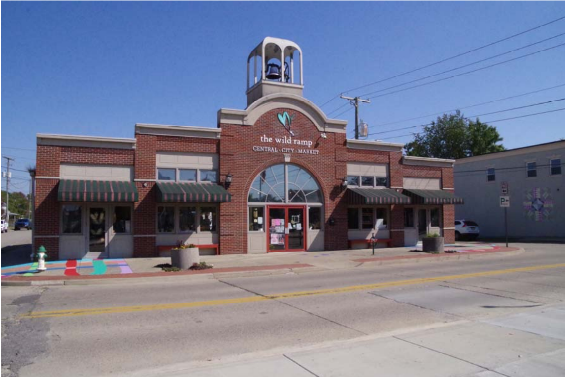
Photo 25 Site 021 looking east on 14th St. West, non-contributing.
