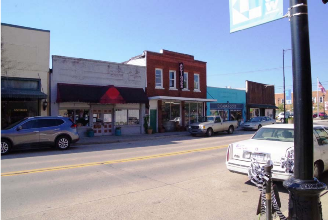
Photo 17 Sites 017, 018, 019 looking west on 14th St. West.
