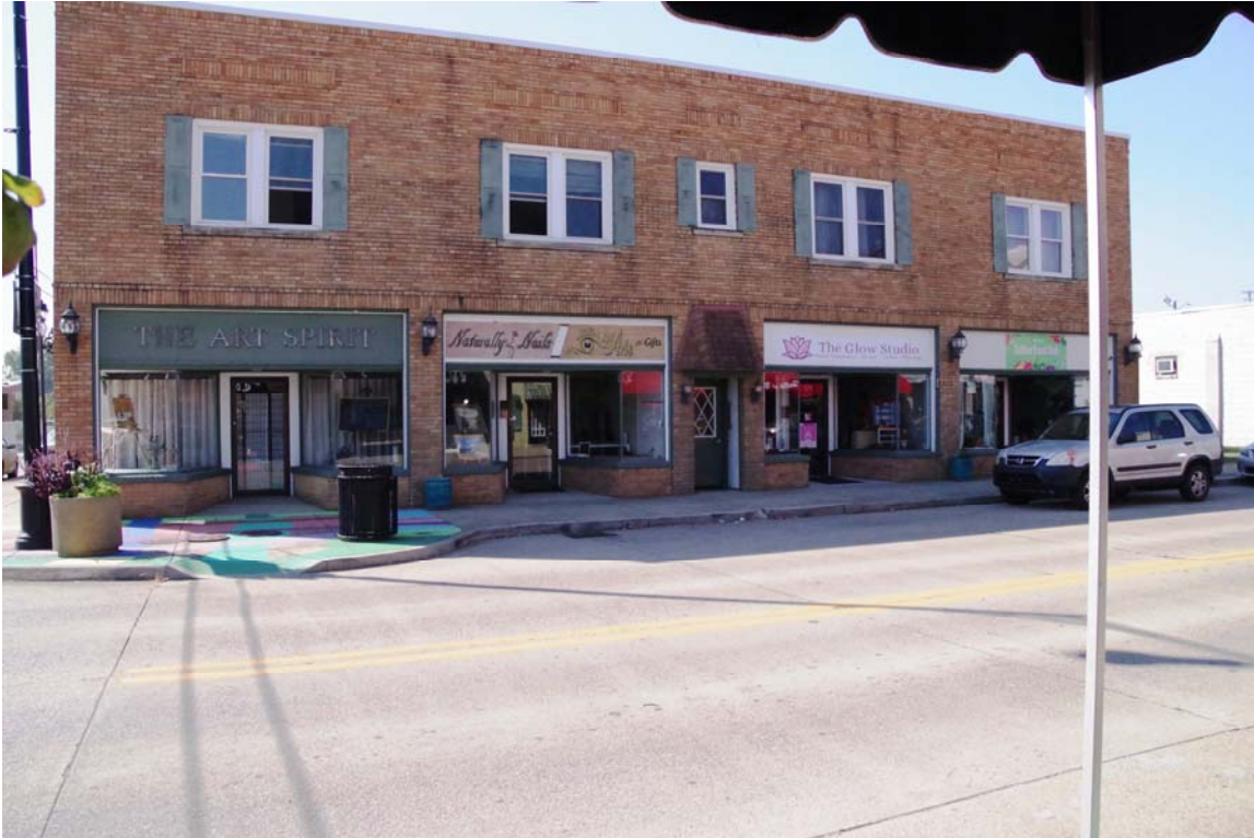
Photo 16 Site 023 looking west on 14th St. West.
