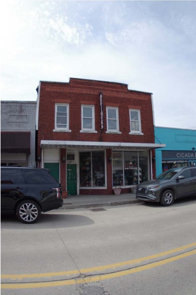
Photo 20 Site 018 looking west on 14th St. West.
