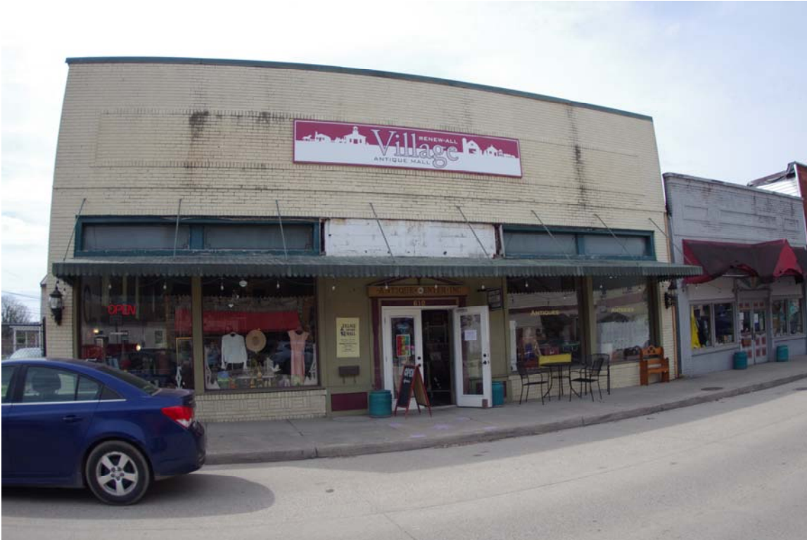
Photo 23 Site 016 looking west on 14th St. West.
