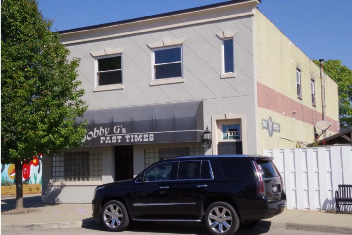
Photo 24 Site 015 looking east on 14th St. West, non-contributing.
