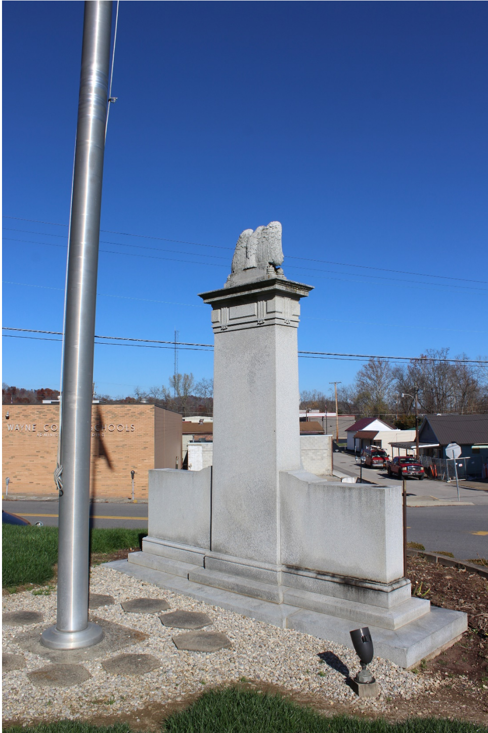
Photo 11 Rear of memorial, southwest elevation
