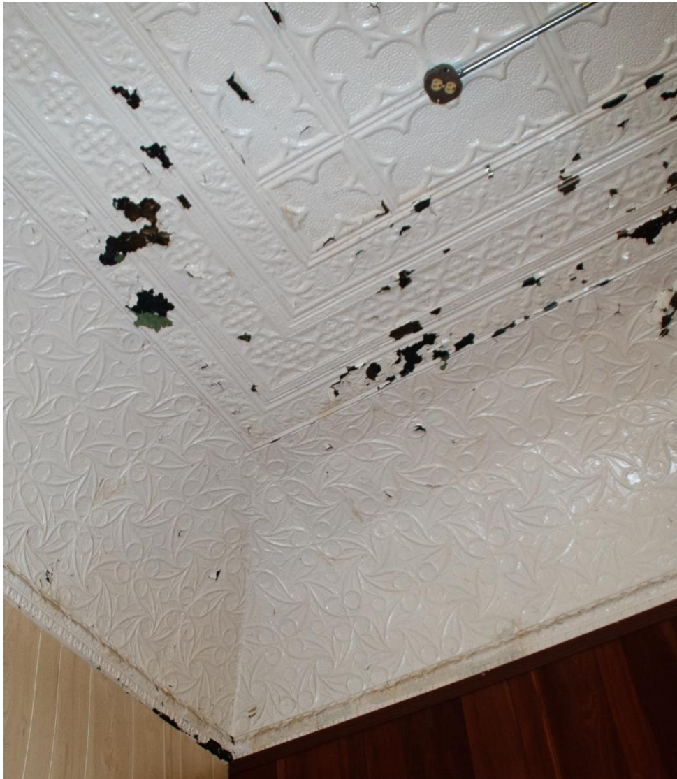
Photo 10. Main Interior Area, Stamped Tin Cove/Ceiling Detail
