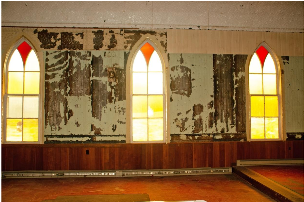
Photo 8. Main Interior Area, Facing East
