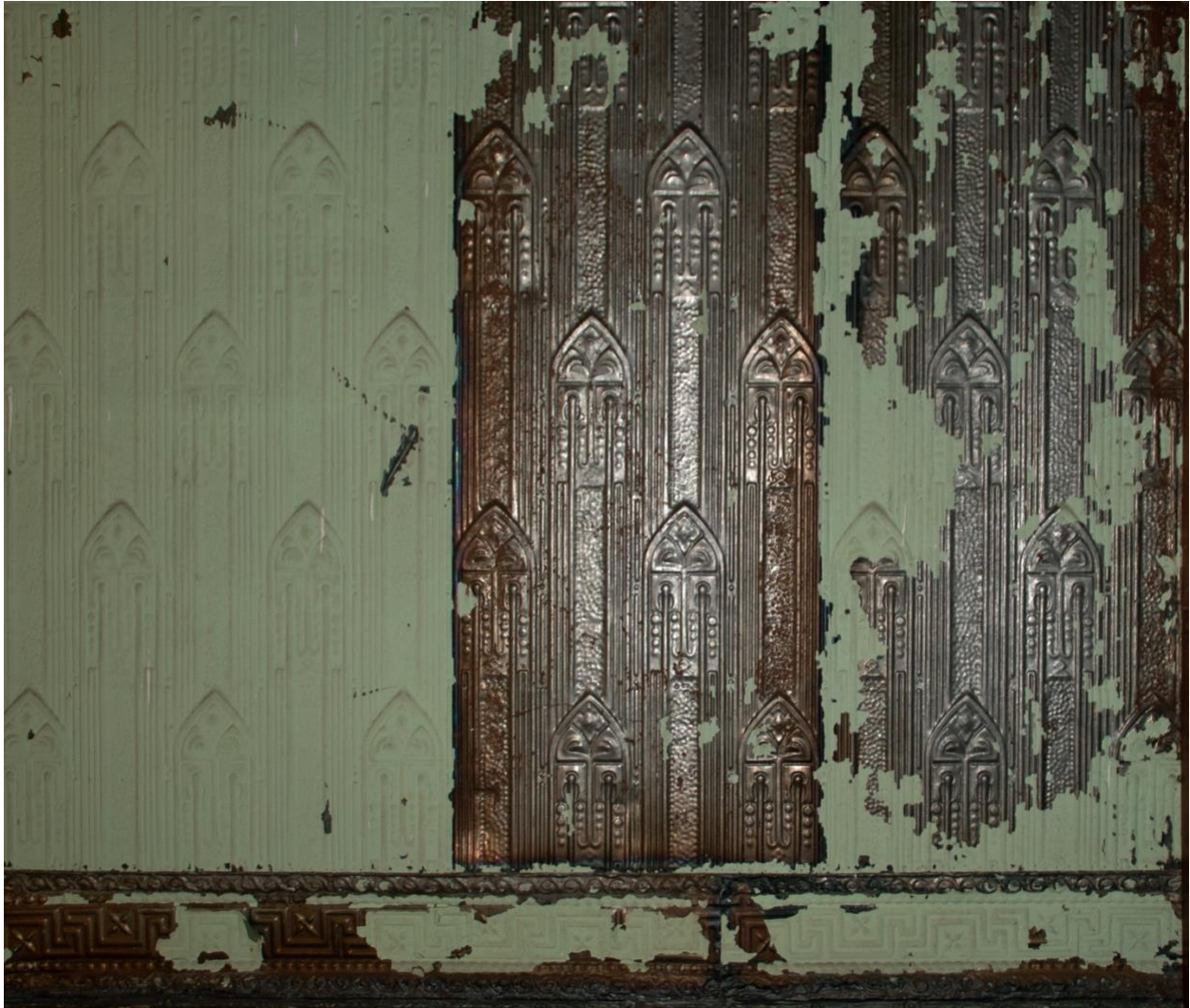
Photo 9. Main Interior Area, Stamped Tin Wall Detail
