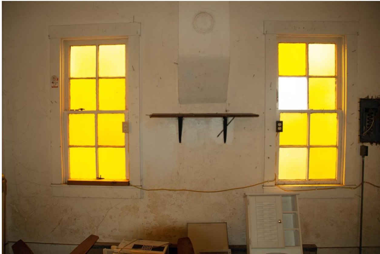
Photo 11. Storage Room/Sacristy, Facing South
