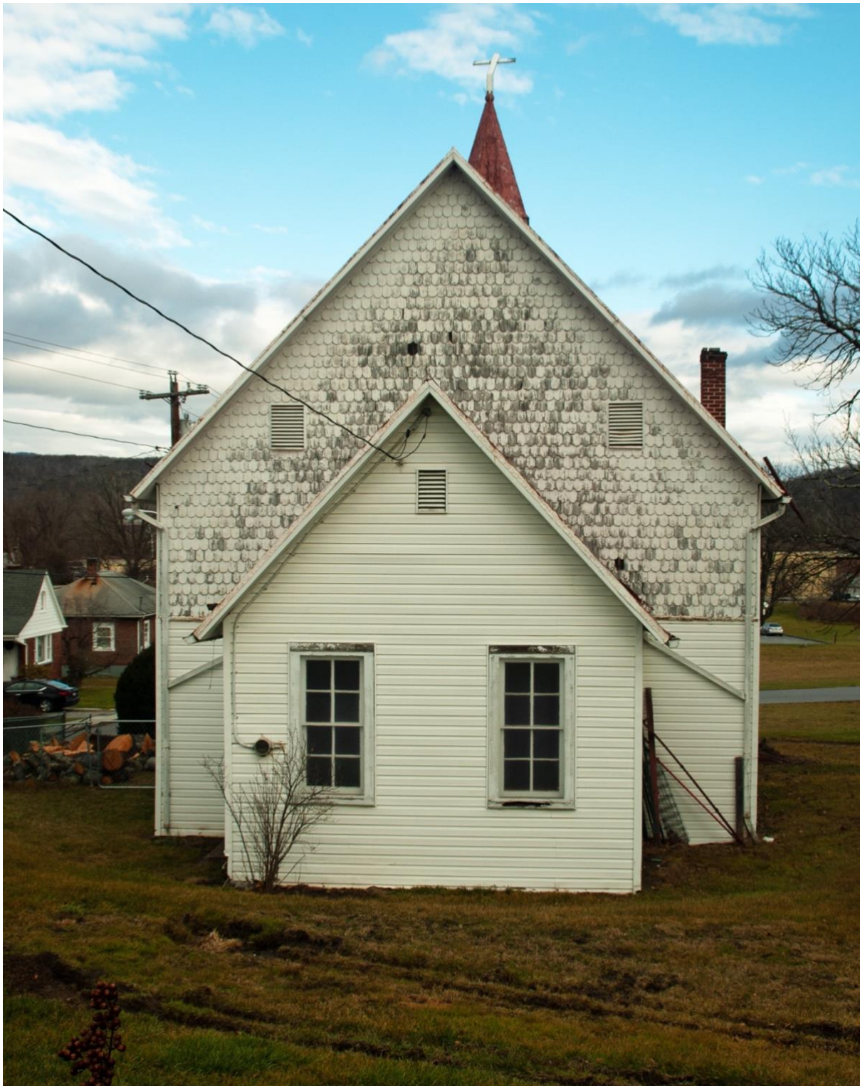
Photo 3. Rear Elevation, Facing North
