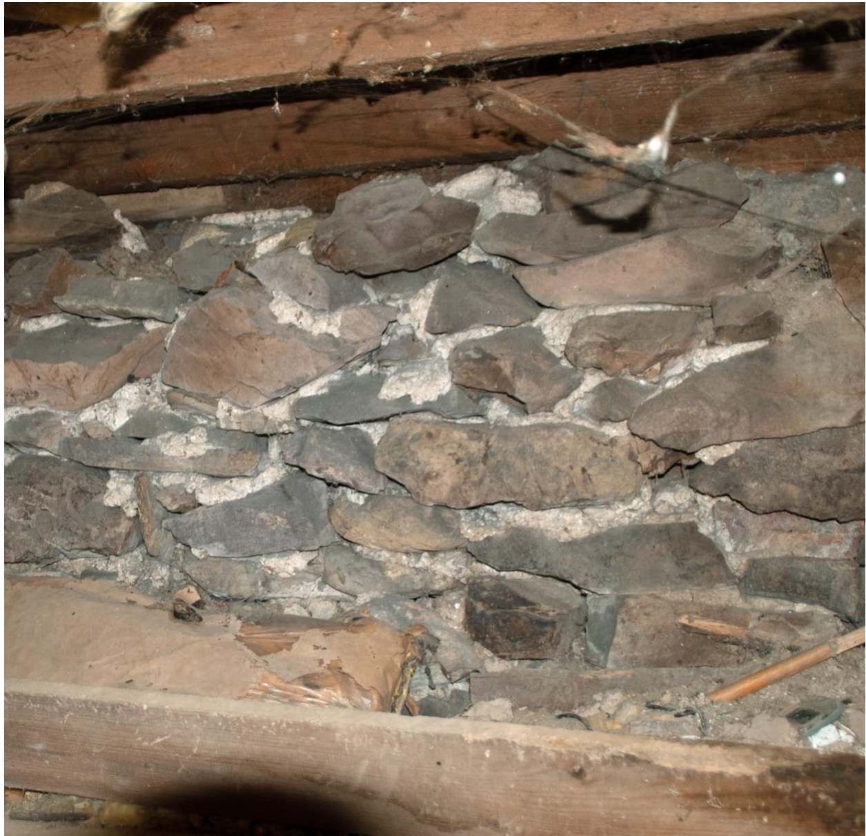
Photo 14. Basement/Crawlspace, Stone Foundation Detail
