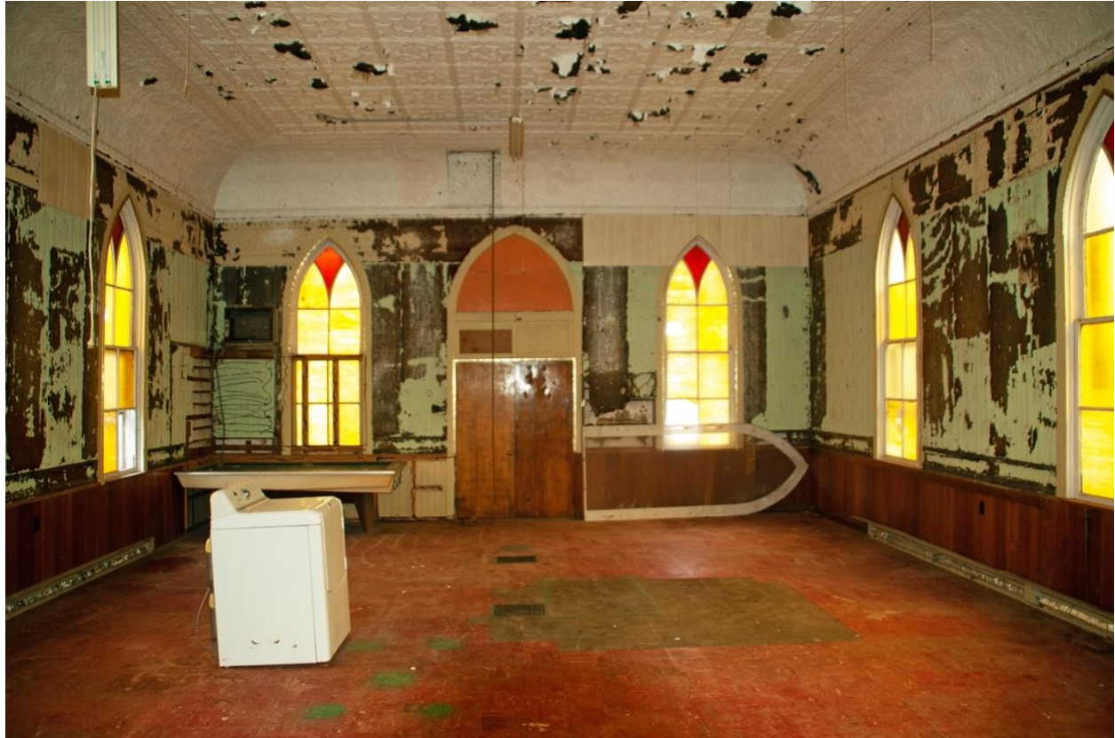
Photo 5. Main Interior Area, Facing North
