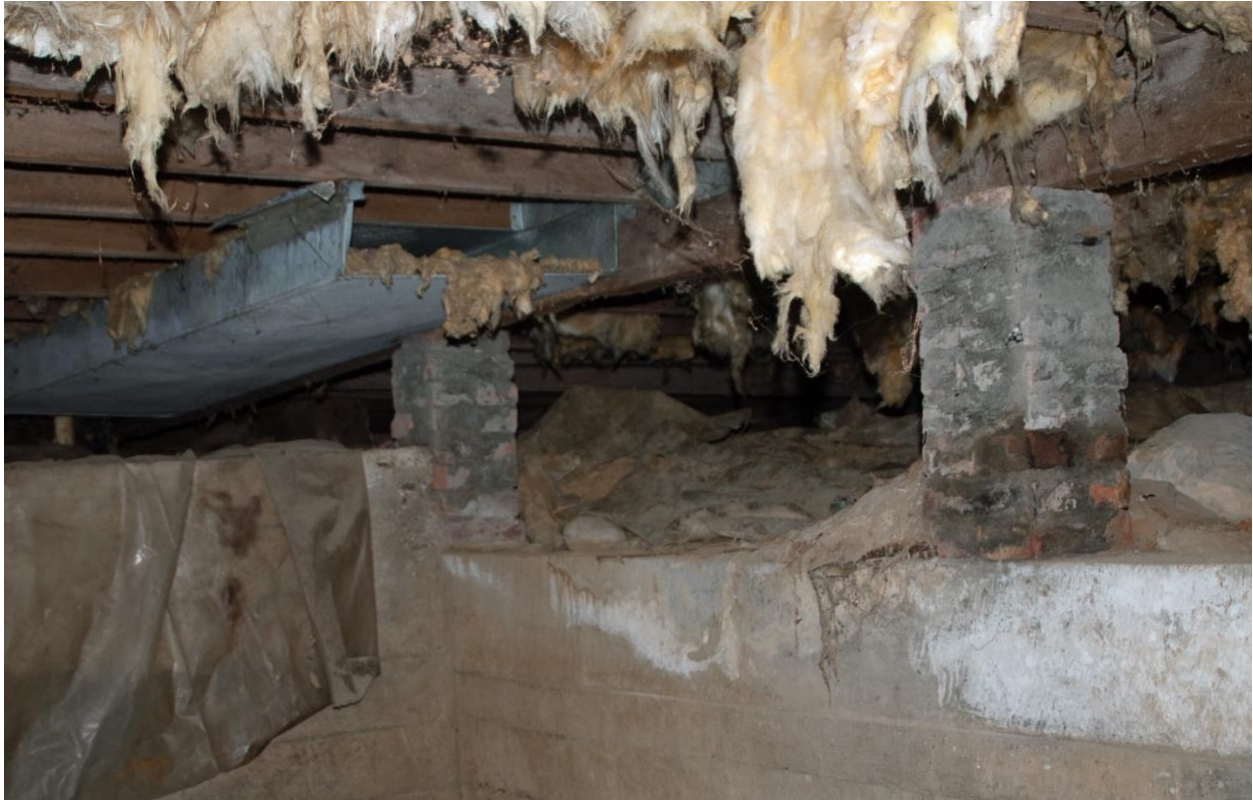
Photo 13. Basement/Crawlspace, Facing Southwest
