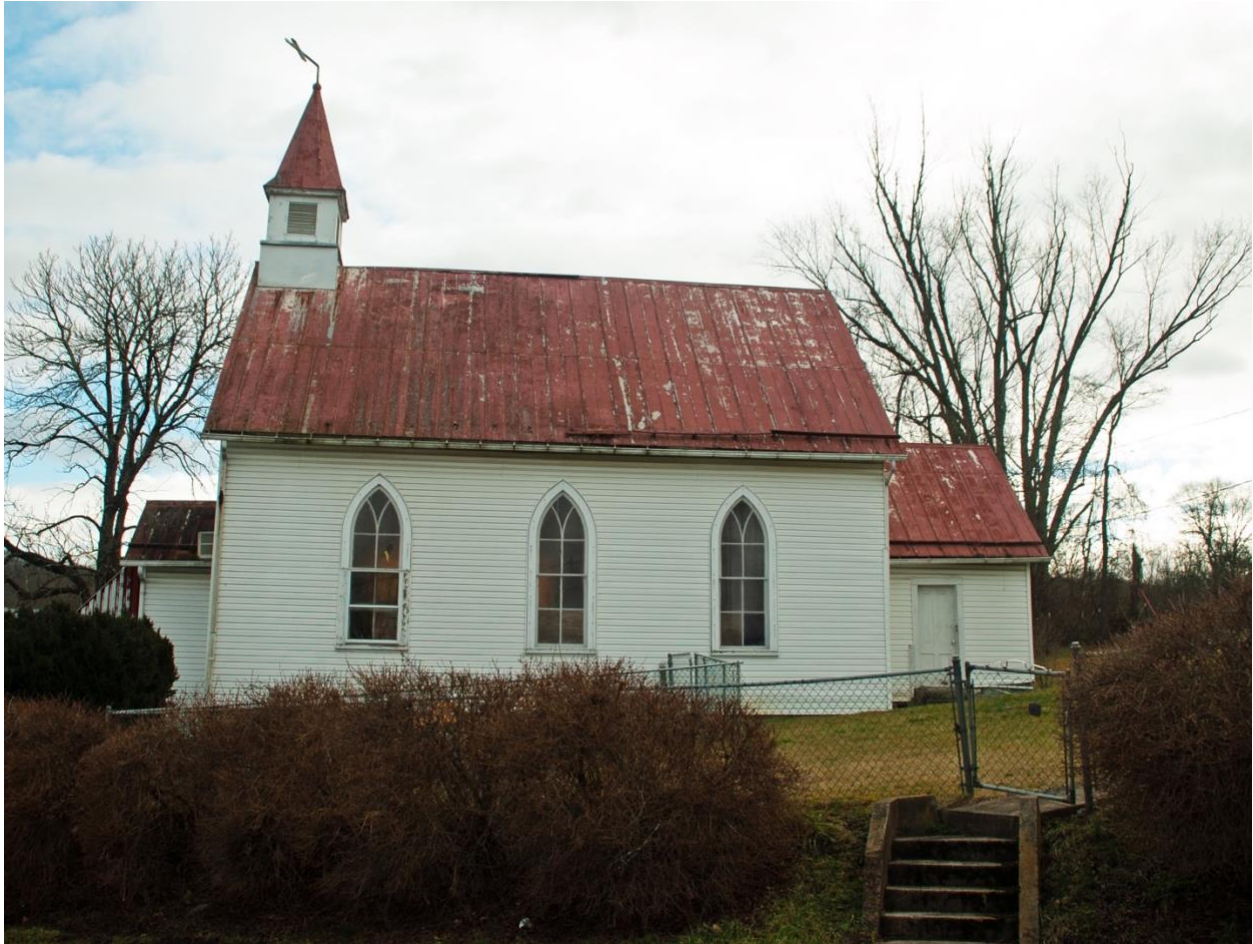
Photo 2. West Elevation, Facing East
