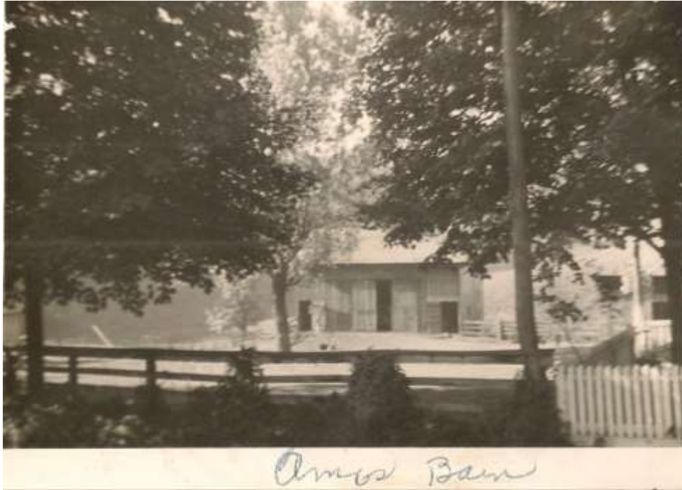
Figure 15: Amos Barn (Resource B) (Historical Photo scanned from Amos archive c. 1925) Camera facing: SW
