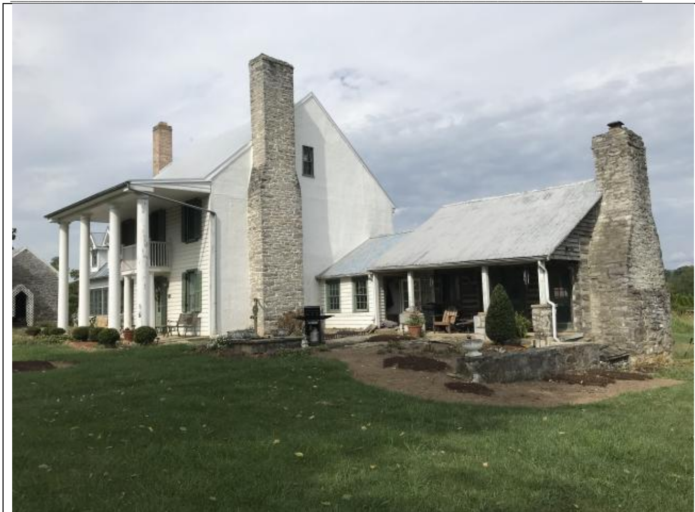
Photo 2. WV_Jefferson County_Fairview-Rees-Daniels Farm_0002. Oblique view to west.
