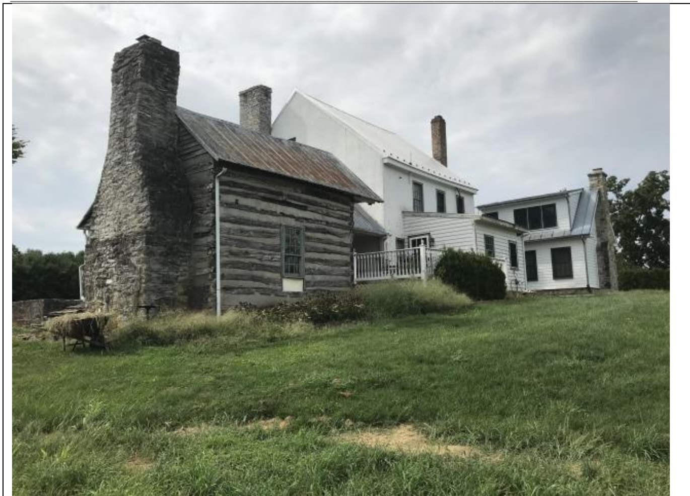
Photo 4. WV_Jefferson County_Fairview-Rees-Daniel Farm_0004. Oblique rear, view to south.
