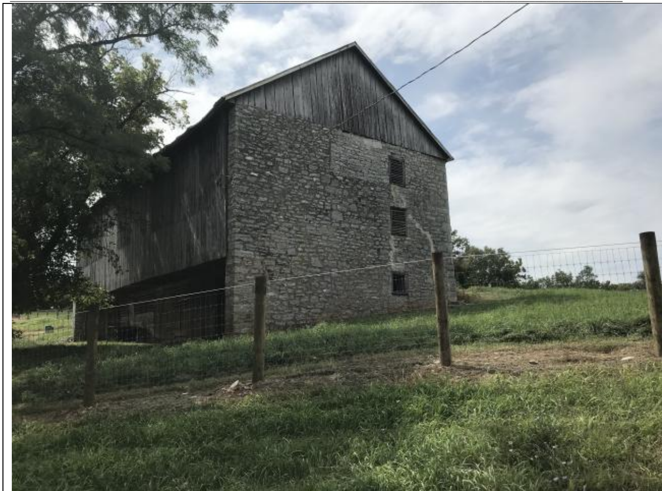
Photo 12. WV_Jefferson County_Fairview-Rees-Daniel Farm_0012. Stone barn oblique, view to west.
