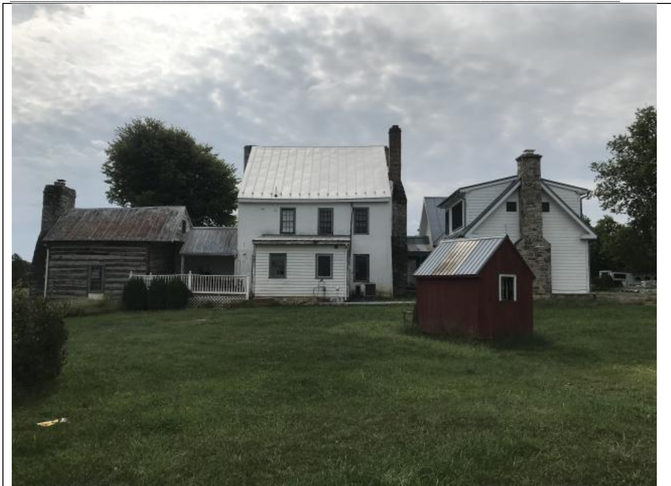
Photo 5. WV_Jefferson County_Fairview-Rees-Daniel Farm_0005. Rear façade, view to southeast.
