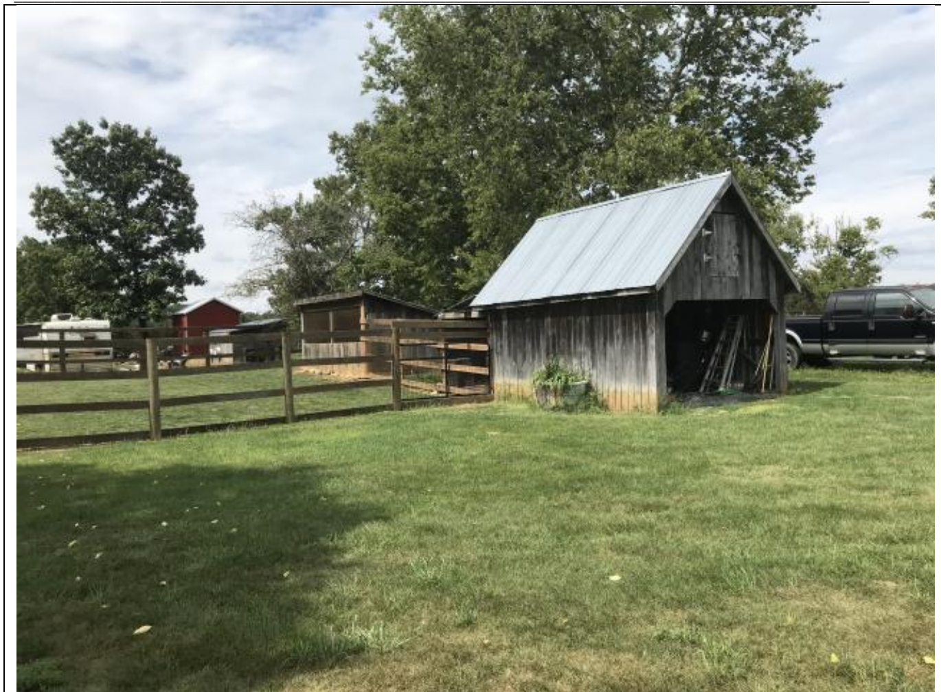
Photo 11. WV_Jefferson County_Fairview-Rees-Daniel Farm_0011. Utility shed/garage, view to west.
