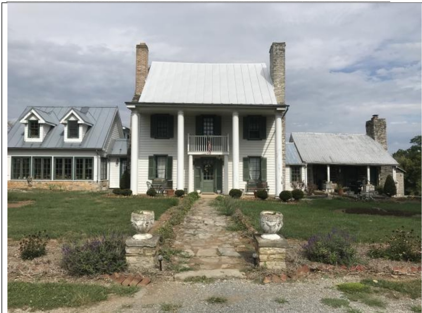
Photo 1. WV_Jefferson County_Fairview-Rees-Daniel_Farm_0001. Front façade, view to northwest.
