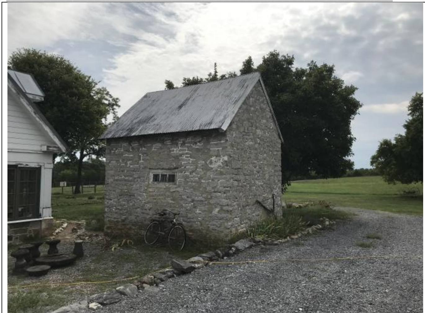
Photo 9. WV_Jefferson County_Fairview-Rees-Daniel Farm_0009. Meathouse west façade, view to southeast.
