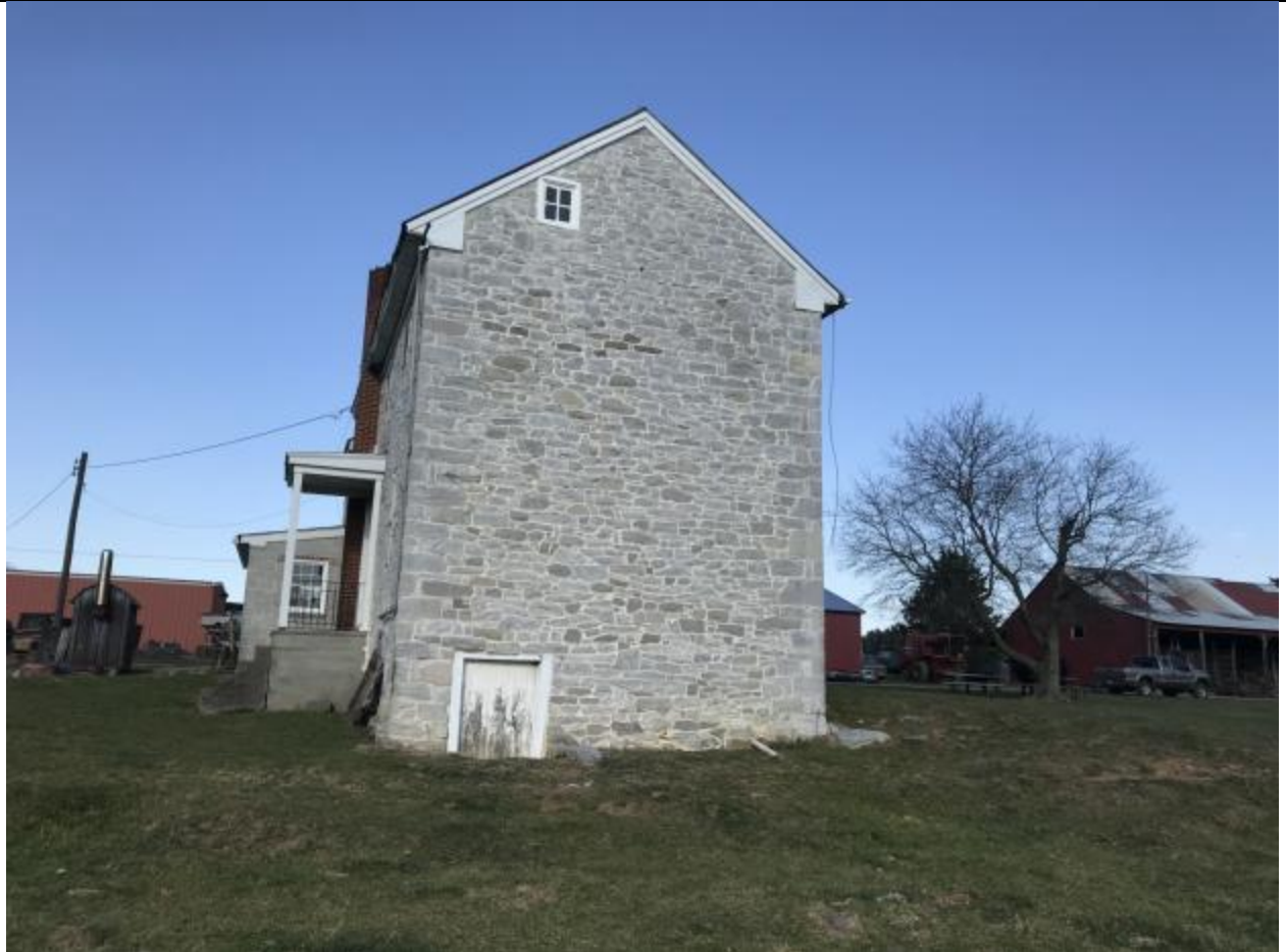
WV_Jefferson County_Rosenberger/Brown Farm_0005. View to southeast. Until 2011, the west façade had an interior chimney that an earthquake destroyed. A small door gives access to the cellar, and a four-panel casement window gives ventilation to the attic.
