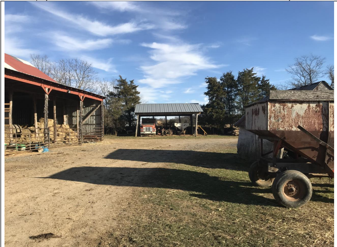
WV_Jefferson County_Rosenberger/Brown Farm_0020. Pole shelter, view to south. Pole shelters of metal roofing supported by poles or 6" x 6" lumber prove an adequate shelter for valuable equipment.
