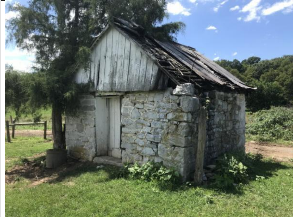
WV_Jefferson County_Rosenberger/Brown Farm_0006. View to northwest. A family cured and stored pork, hams, bacon, beef and venison in their meat house (Fig 13). Thick stone helped keep the structure cool in summer. In style, this meat house has an off-center doorway on its gable end.
