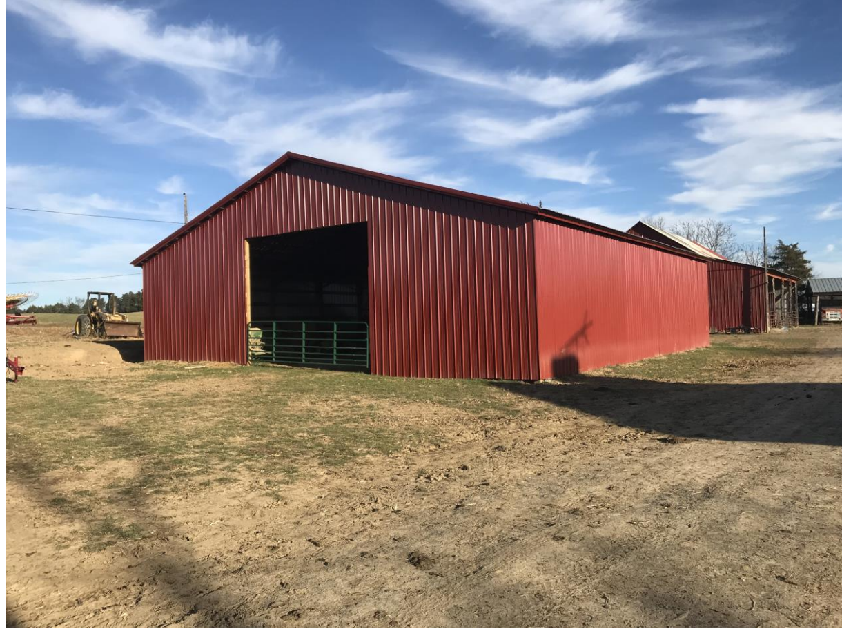
WV_Jefferson County_Rosenberger/Brown Farm_0013. Metal barn, view to southeast. Metal buildings such as this provide shelter for livestock and equipment formerly housed in the Old Barn and other wooden buildings and pole shelters. These provide adequate shelter, can be assembled by family and a small crew, and cost less than a traditional wood, barn-frame barn.
