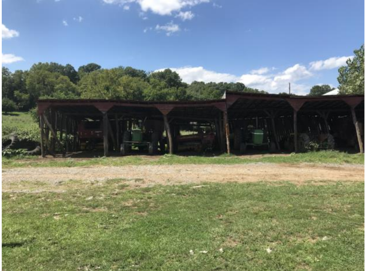
WV_Jefferson County_Rosenberger/Brown Farm_0010. View to north. These sheds help shelter farm equipment from rain and snow.
