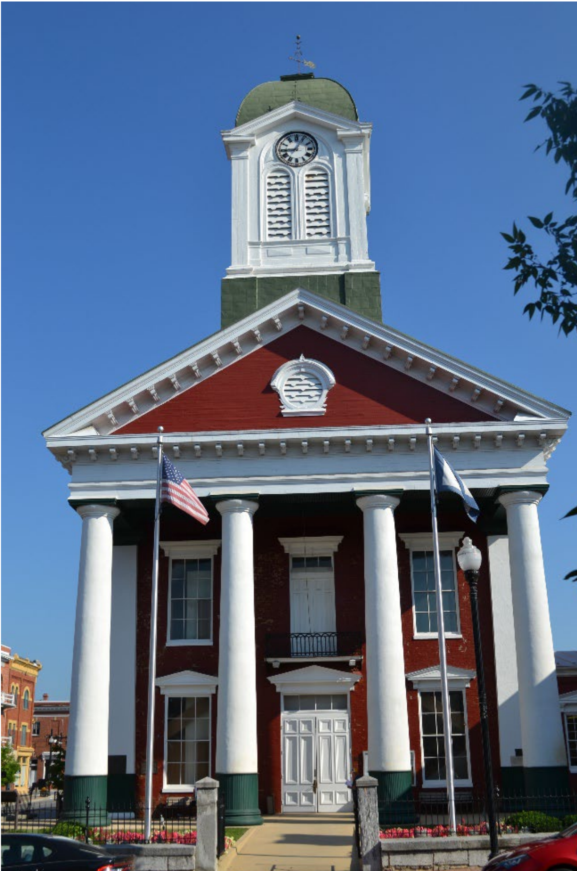
Photo 1. View north of front façade. Photo by Susan Cianci Salvatore, 7/19/2019.
