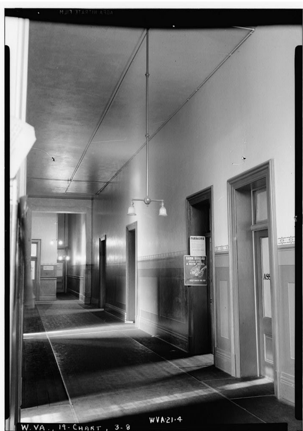
Historic Image 12. Interior, main hallway, 1 st floor looking northeast. Courthouse, George & Washington Streets, Charles Town, Jefferson County, WV. Historic American Buildings Survey (WV-21-4), circa 1936.
