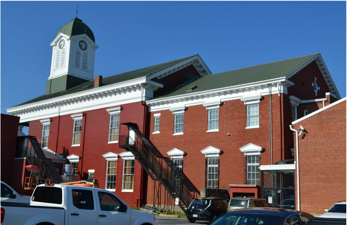
Photo 5. View looking southwest at the east side of the courthouse and the 1910 addition. Photo by Susan Cianci Salvatore, 7/19/2019.
