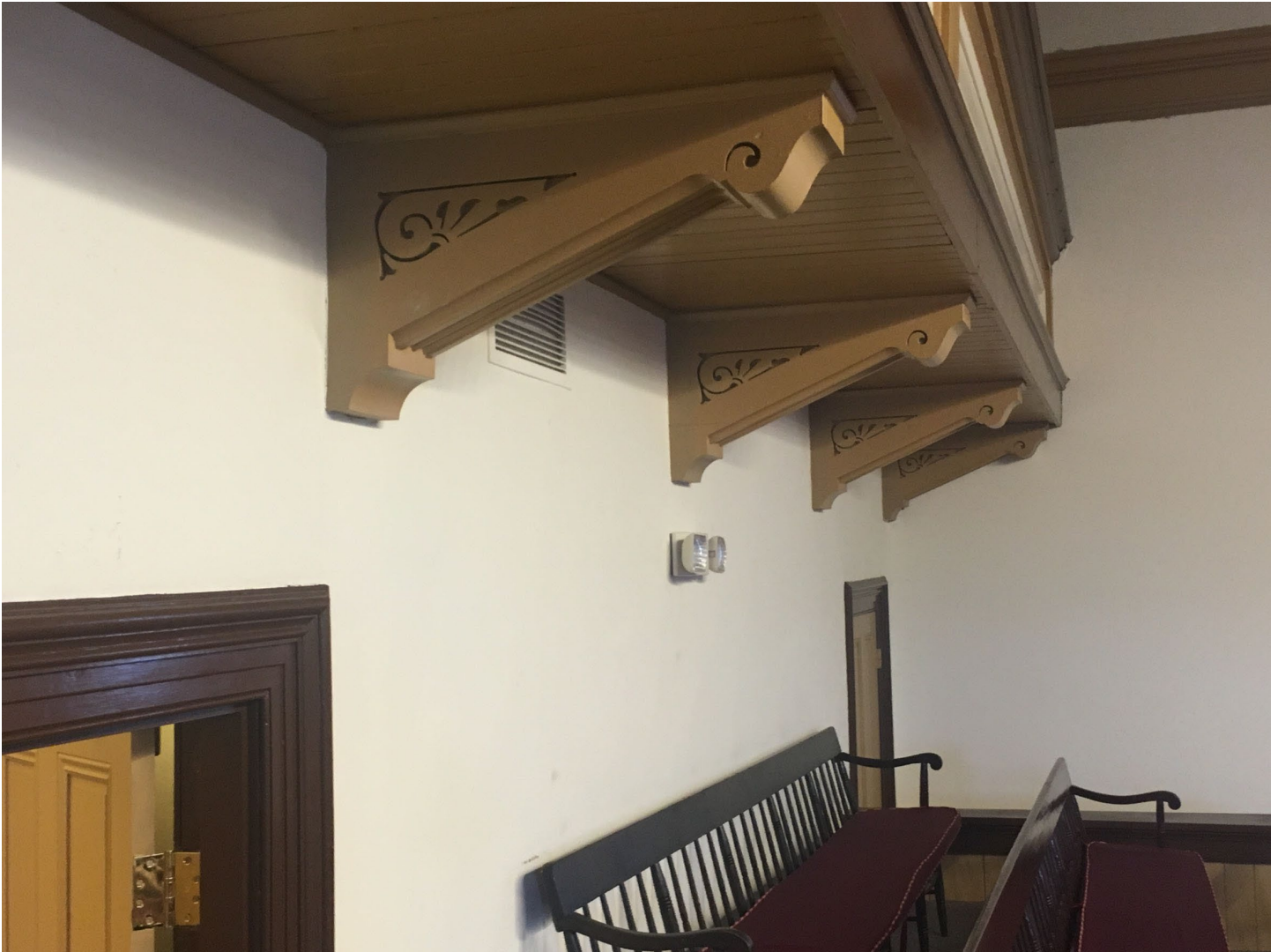
Photo 14. View of decorated brackets under courtroom balcony. Photo by Christopher Hetzel, NPS, 5/7/2018.
