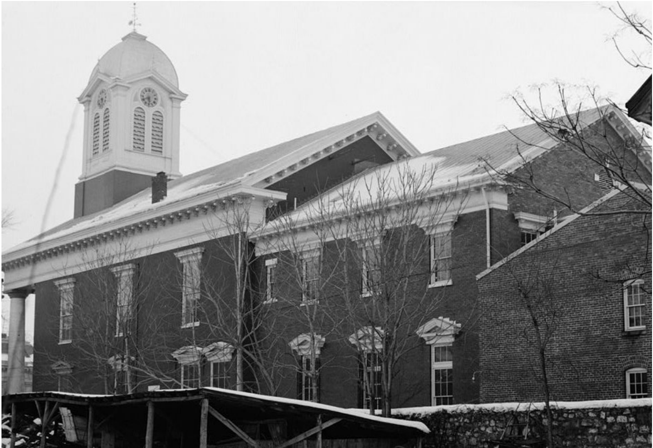
Historic Image 7. East elevation. Courthouse, George & Washington Streets, Charles Town, Jefferson County, WV. Historic American Buildings Survey (WV-21-4), circa 1936.
