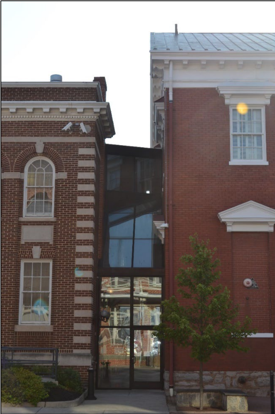
Photo 4. View looking east at 2007 glass hyphen addition between the courthouse addition (right) and the jail (left). Photo by Susan Cianci Salvatore, 7/19/2019.
