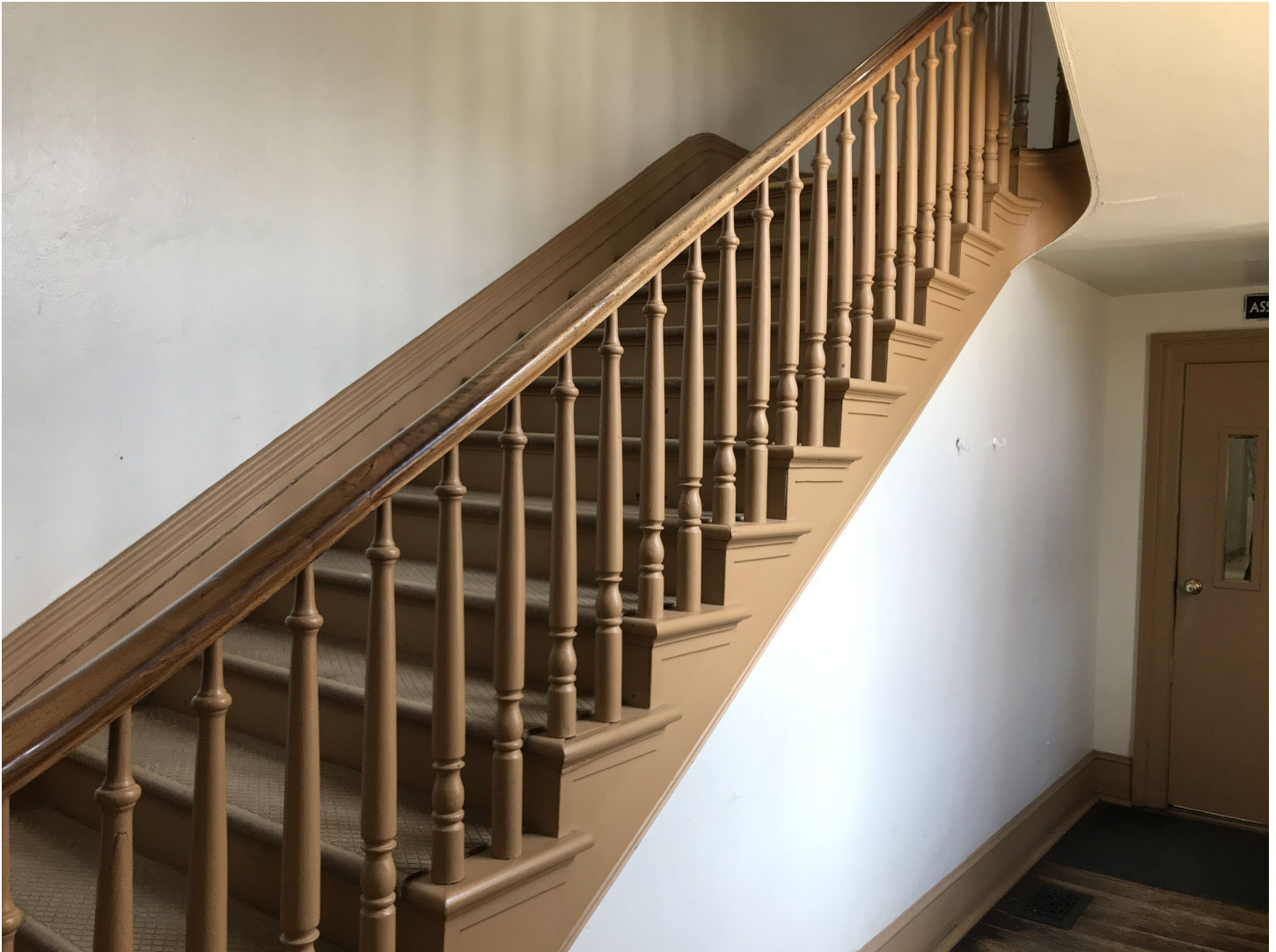
Photo 8. View of staircase on the east side of the foyer leading to the second floor courtroom. Identical staircase is on the west side. Photo by Kathryn Gettings Smith, NPS, 5/7/2018.
