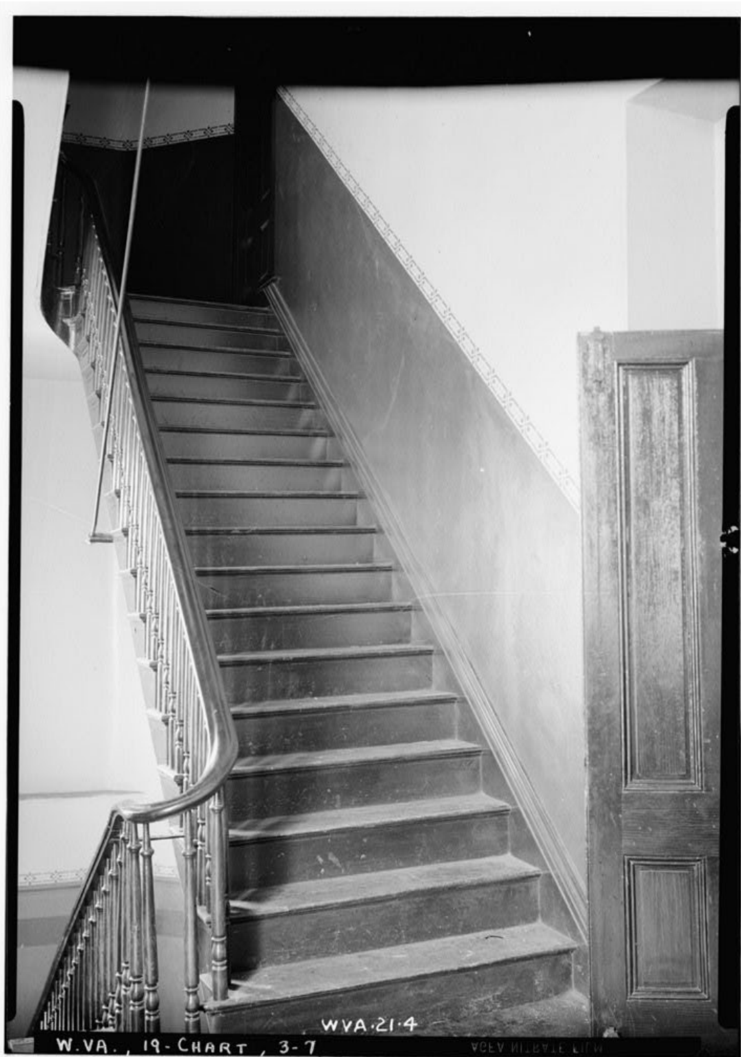
Historic Image 11. Interior, West stair from 2 nd floor to attic. Courthouse, George & Washington Streets, Charles Town, Jefferson County, WV. Historic American Buildings Survey (WV-21-4), circa 1936.
