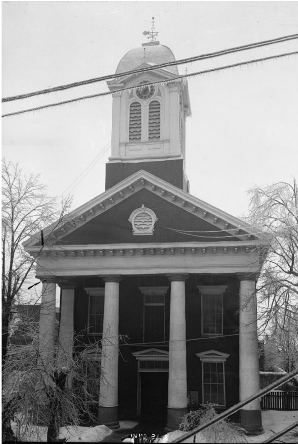
Historic Image 6. South elevation (façade). Courthouse, George & Washington Streets, Charles Town, Jefferson County, WV. Historic American Buildings Survey (WV-21-4), circa 1936.
