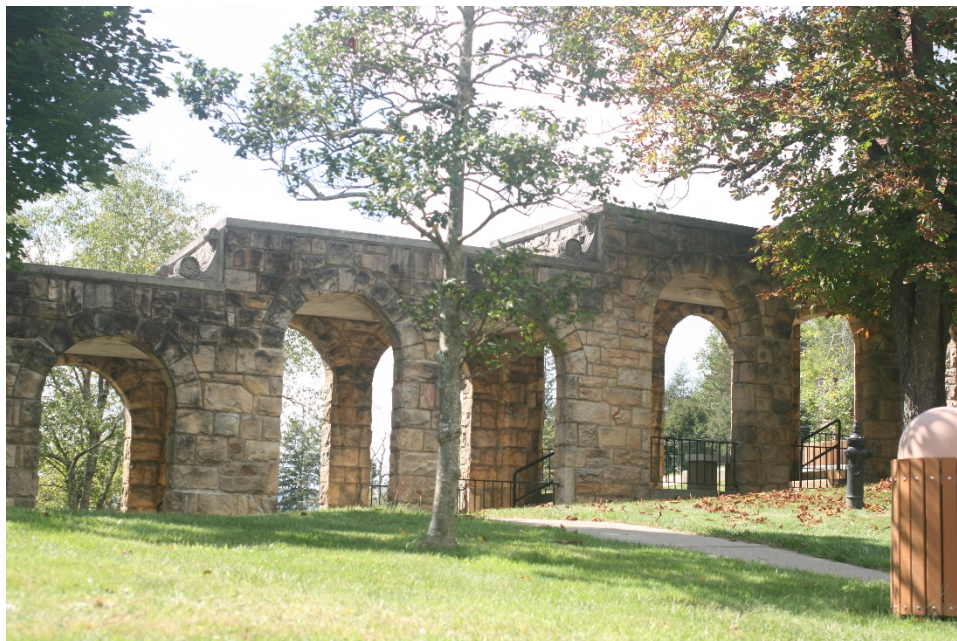
Photo 6 of 19: Rock-faced arcaded stone walkway linking Charles Albert Hall and Liberal Arts Hall, looking northwest.
