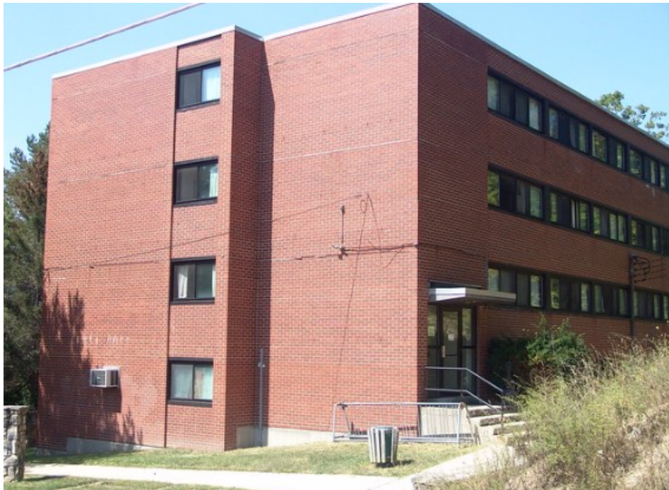
Photo 8 of 19: Darby Residence Hall, southeast perspective, looking northeast.
