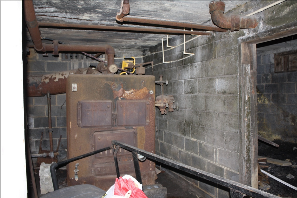
Photo 15. Image of former coal furnace, photographer facing southwest
