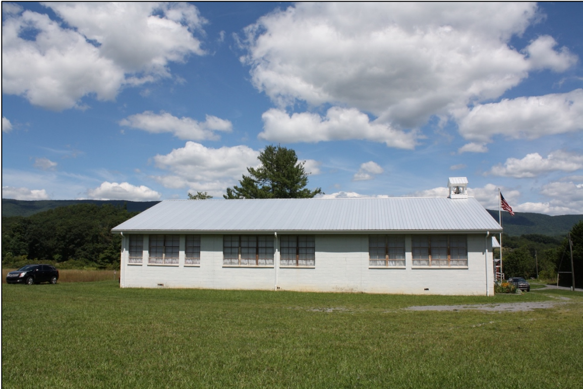
Photo 2. South elevation, photographer facing north
