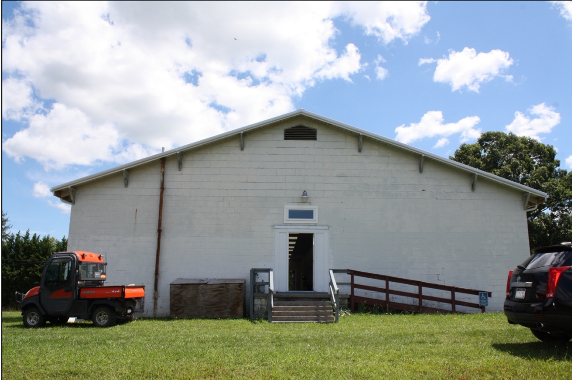
Photo 3. West elevation, photographer facing east
