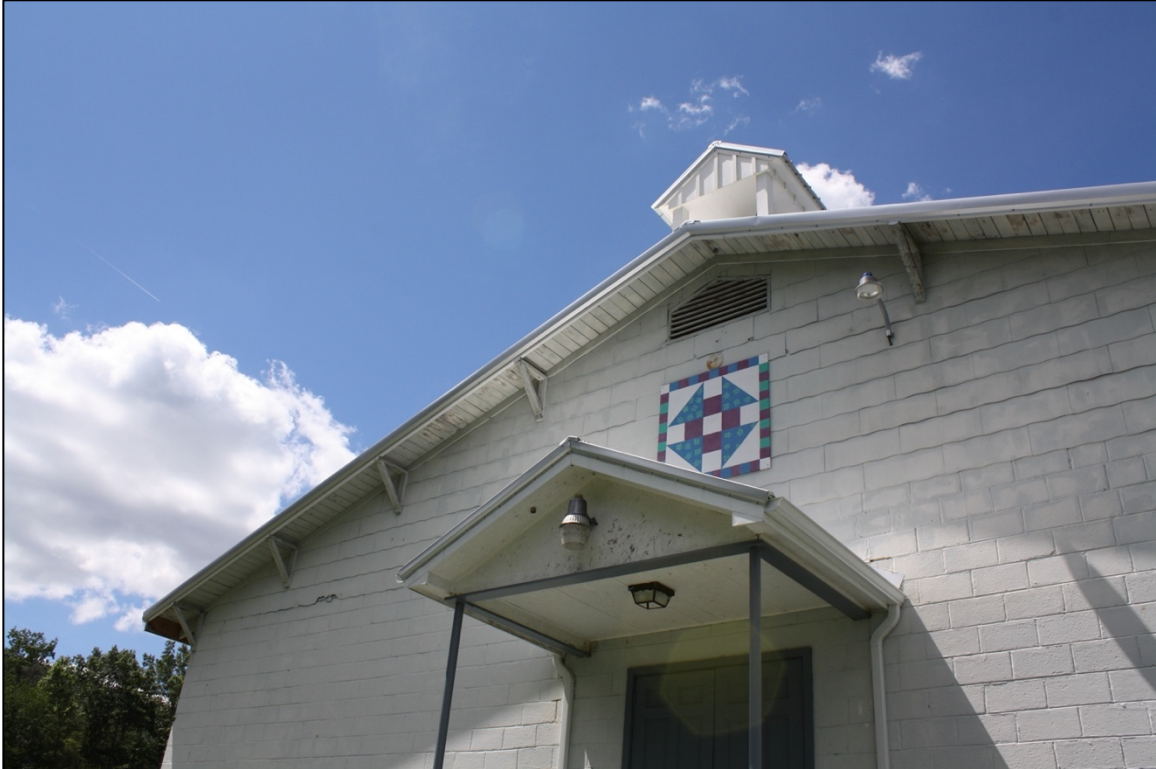
Photo 5. Detail of the façade, photographer facing southwest
