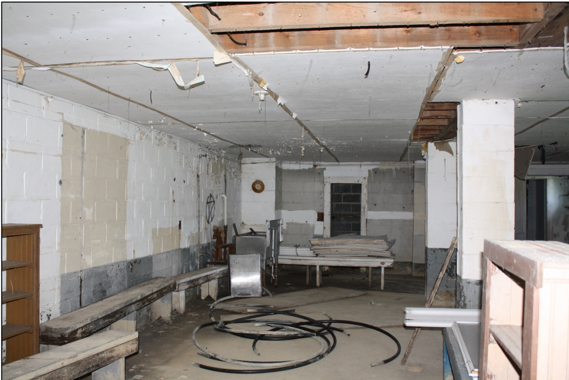
Photo 14. Lower-level kitchen and cafeteria, photographer facing west
