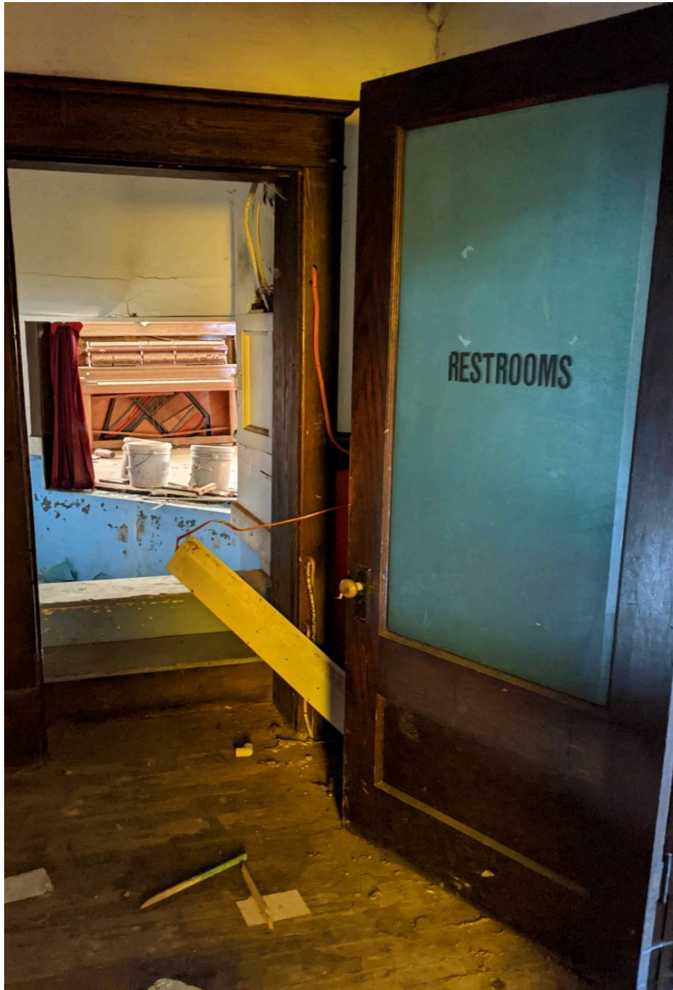
Photo 26 of 33 Interior, entrance to restrooms at rear of building, south elevation
