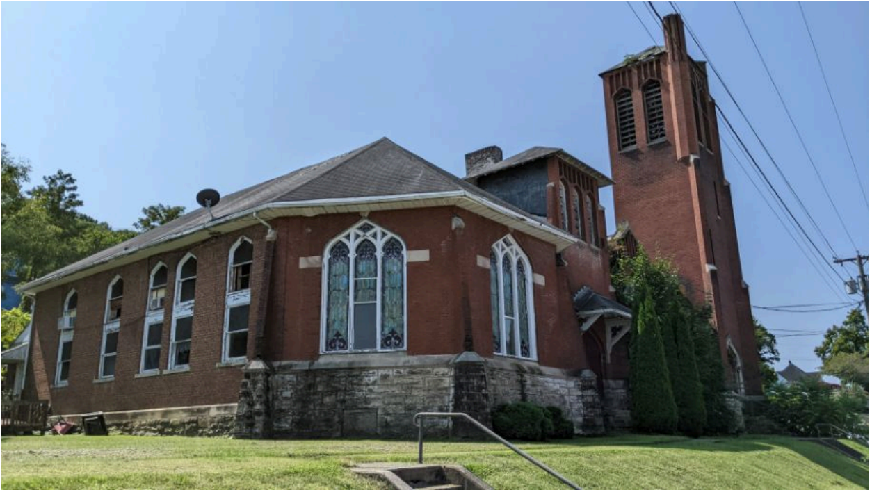
Photo 5 of 33 Exterior, northeast corner of building, southwest elevation
