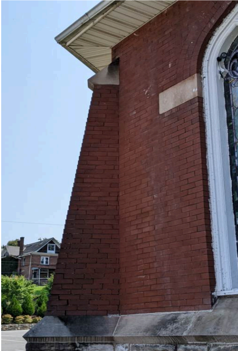
Photo 9 of 33 Exterior, buttress at northeast corner, southeast elevation.
