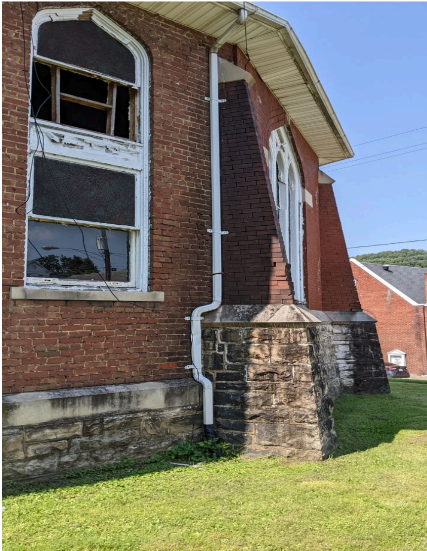
Photo 8 of 33 Exterior, buttresses, Tudor window arch, northwest elevation
