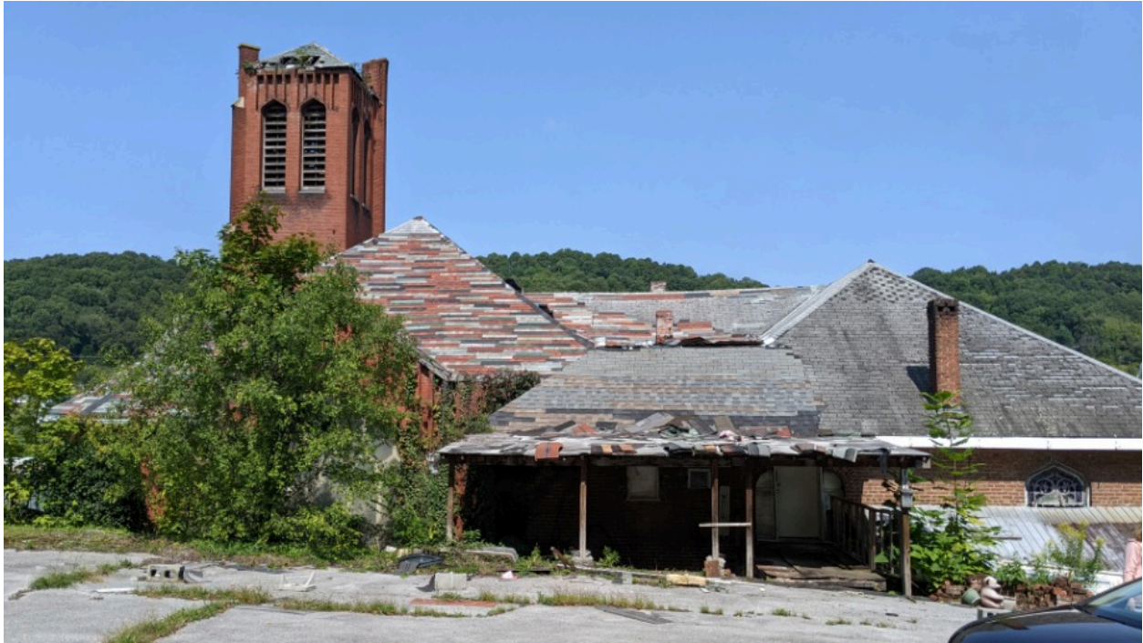
Photo 14 of 33 Exterior, rear of building, north elevation
