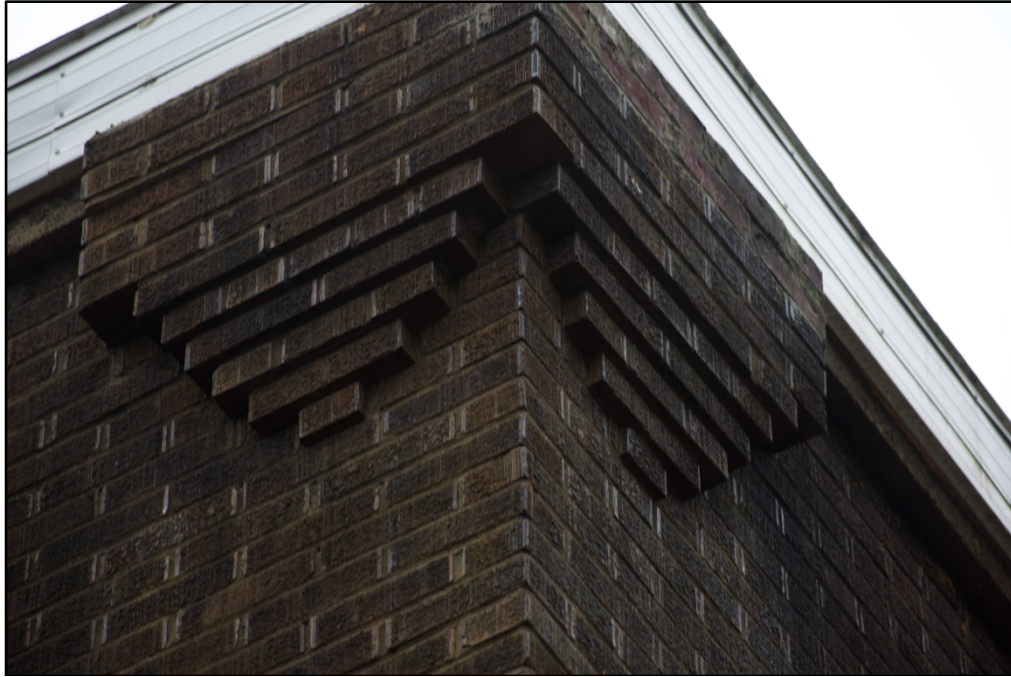
Photo 5. Detail of corbel, facing northwest. Photo by JaLon Staples, taken January 3, 2023.
