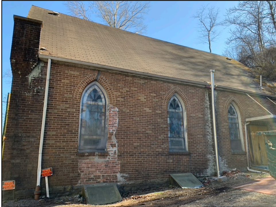
Plate 2. Mount Zion Baptist Church, facing southwest.
