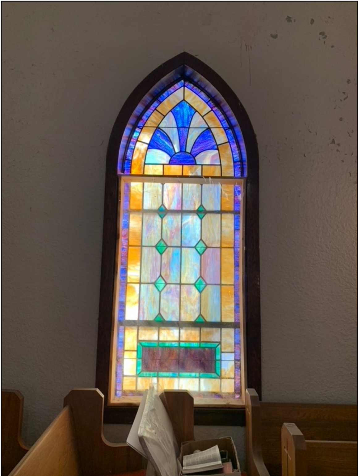
Plate 15. Typical window detail, facing east.
