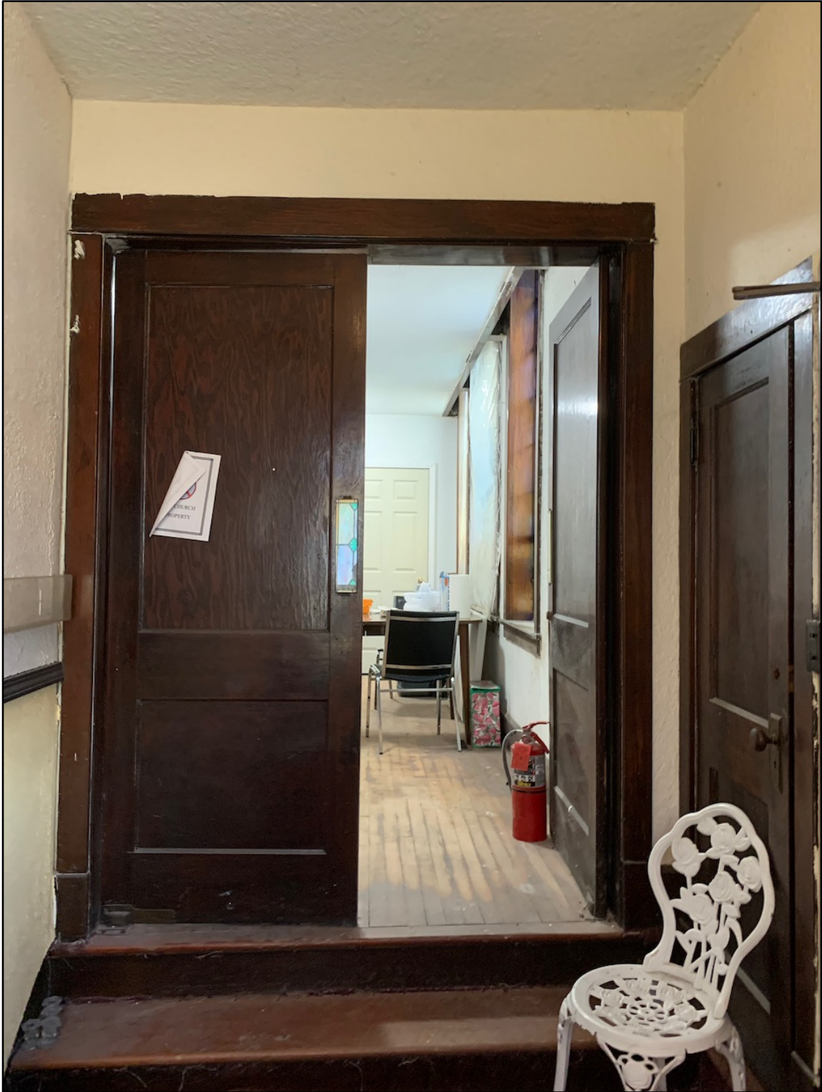
Photo 7. Entry into Narthex from vestibule, facing north.
