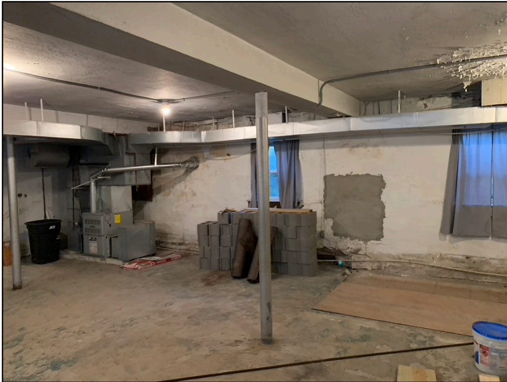
Plate 14. Basement, facing north. Note plywood covering baptismal pool.
