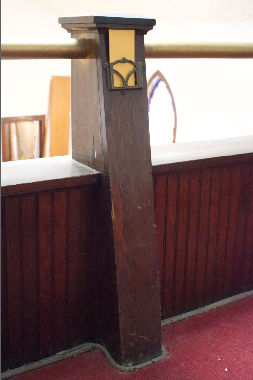
Photo 13. Detail of balustrade, facing northwest. Photo by Jalon Staples, taken January 3, 2023.
